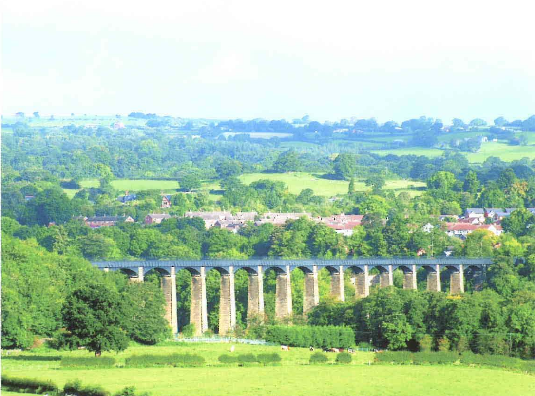
Telford's Pontcysyllte Aqueduct, built between 1795 and 1805, and considered the finest aqueduct built in Britain, carried the canal across the river Dee. Photo: CPAT 1766-50
