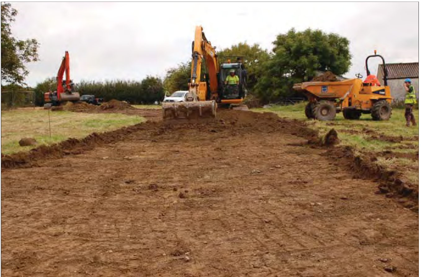
Plate 06: Topsoil strip of main site road. View from the north west.
