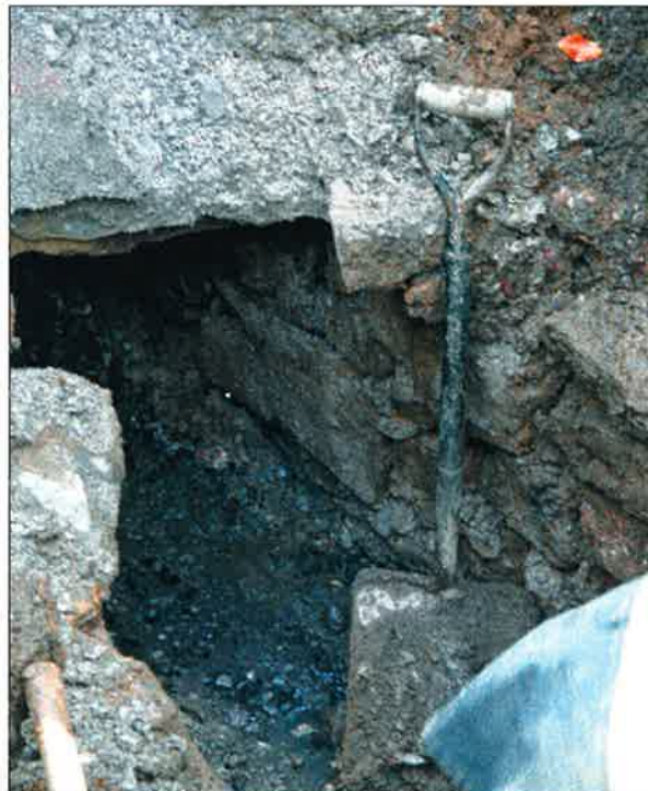
Fig 8. Detail of the culvert (looking south).
