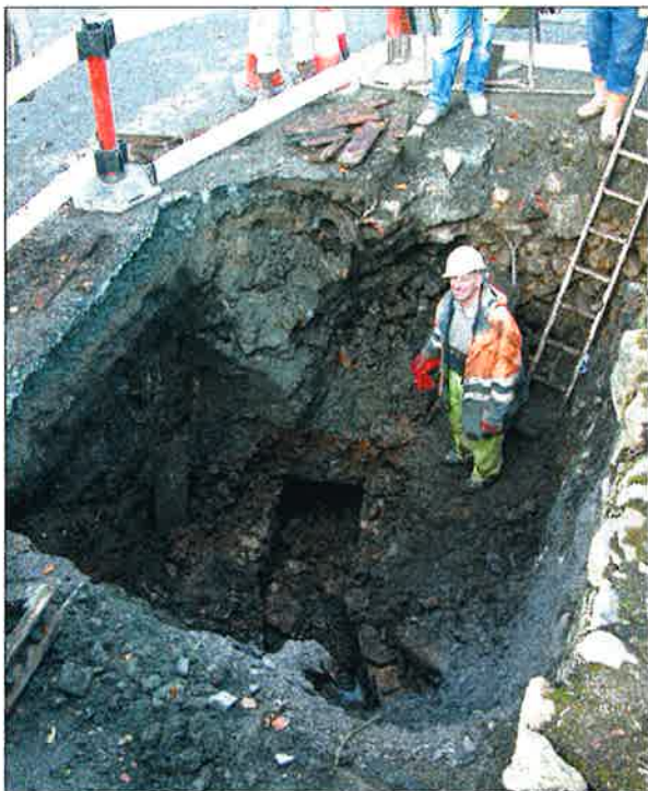
Fig 7. The culvert revealed (looking north).
