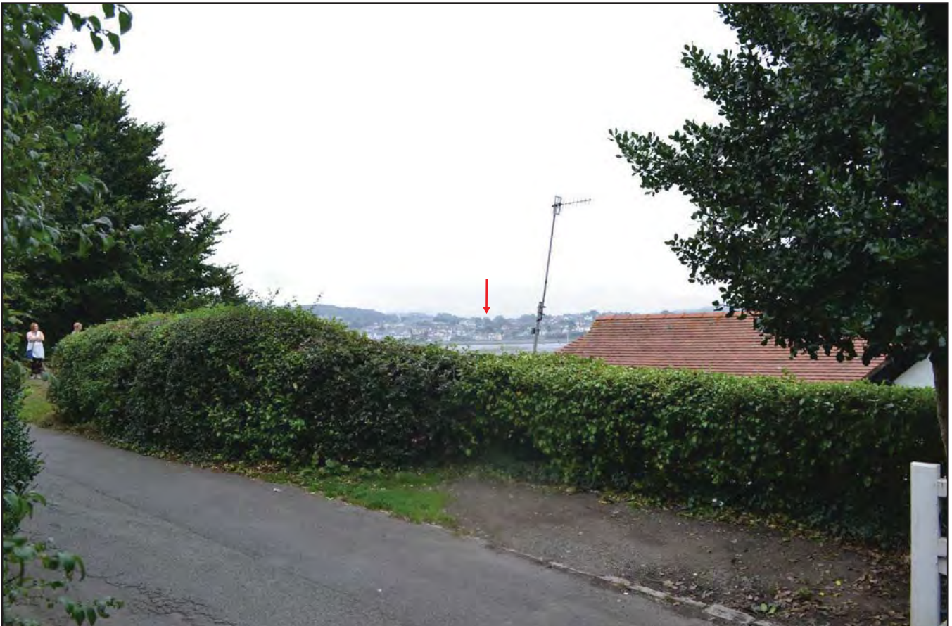
Plate 24: View towards the Proposed Development (direction indicated by red arrow) from LB3363 Bodlondeb Lodge and LB87429 gate piers, gates and walls at entrance to Bodlondeb, viewed from the south-west.
