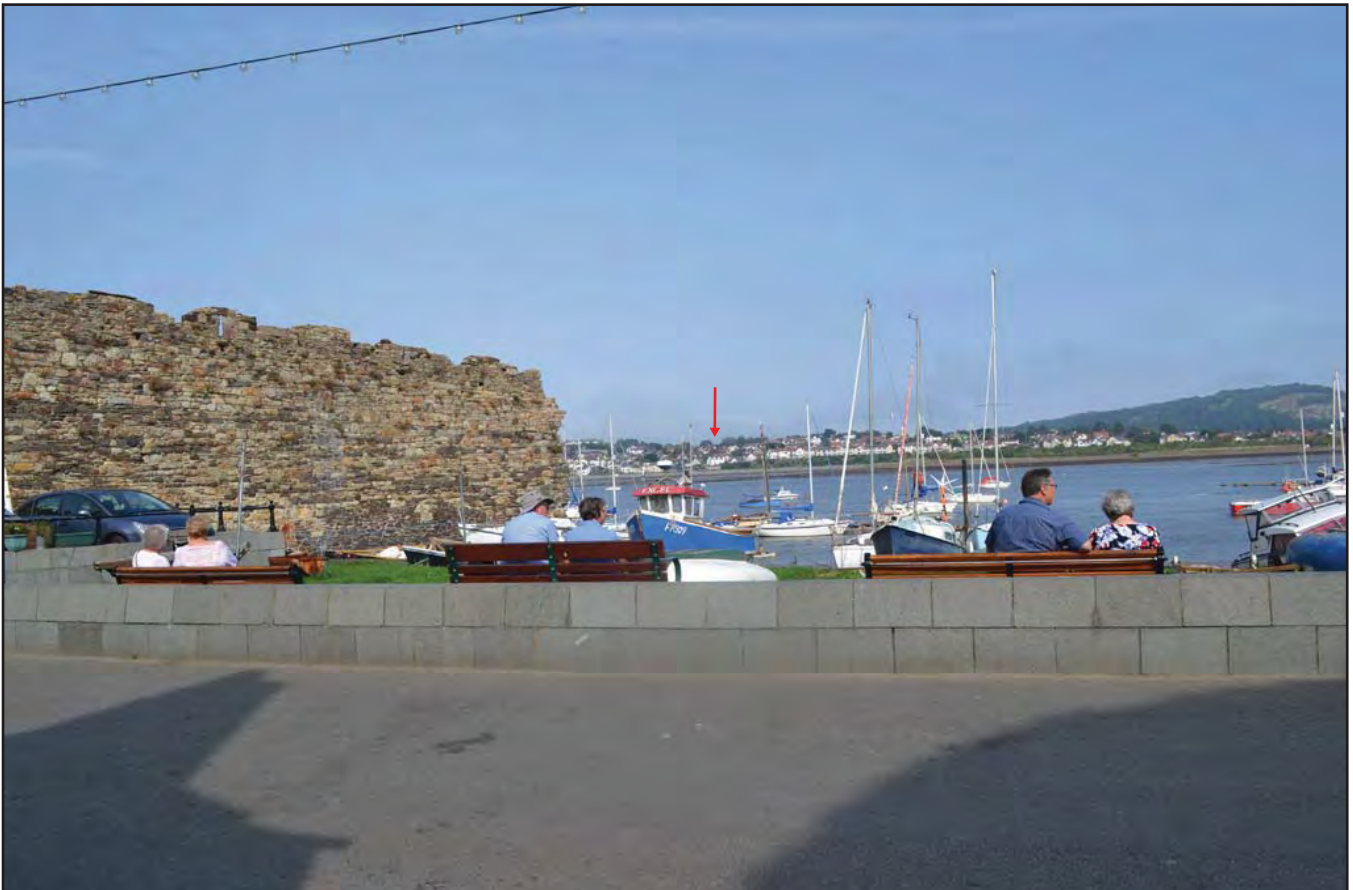
Plate 20: View towards the Proposed Development (direction indicated by red arrow) from the front of LB87363, 12 Lower Gate Street, viewed from the south-west.
