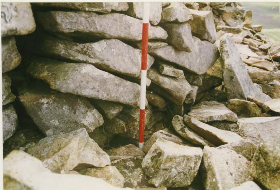
Plate 64, G1022/149/21, Collapse B, outer face, slipped forward face, before conservation.
