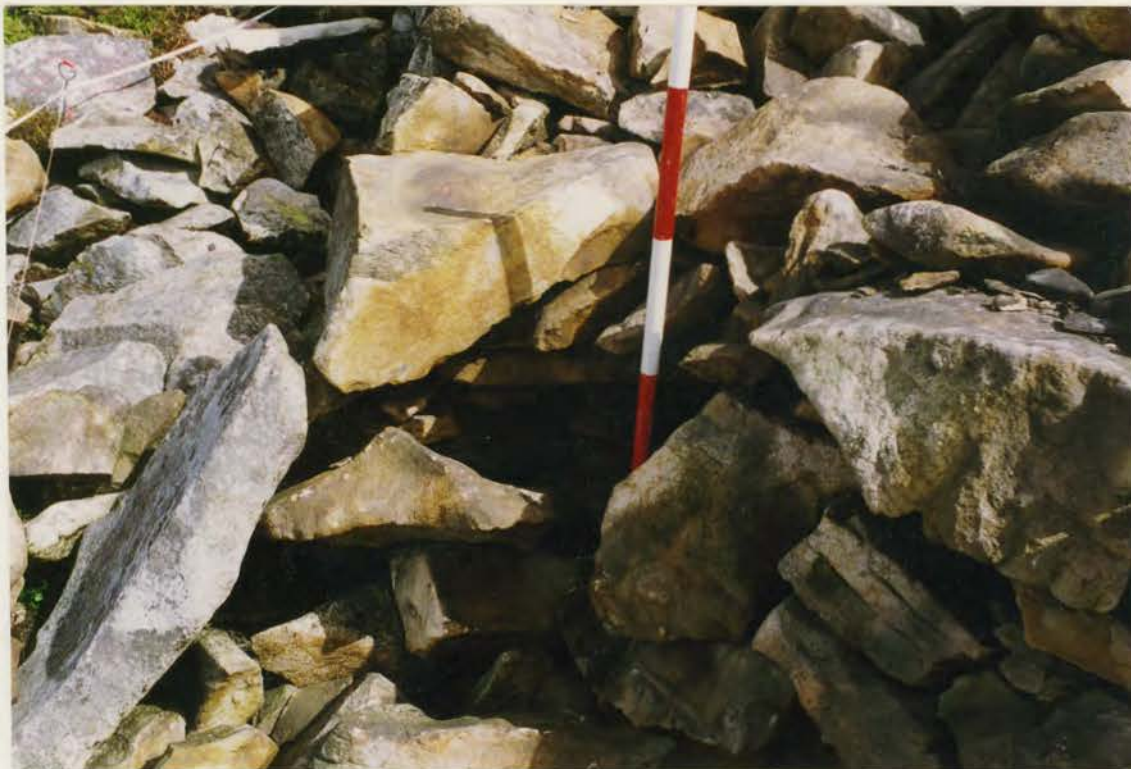
Plate 74, G1022/149/18, Collapse B, slipped forward outer face, after clearance.
