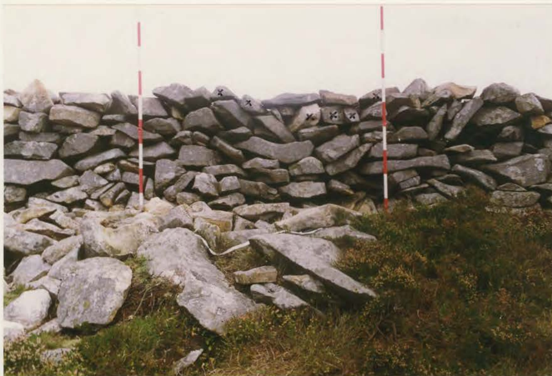
Plate 44, G1022/155/10, Wall B4 to B, after conservation, showing reset stones.
