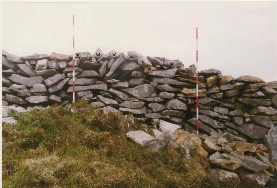
Plate 43, G1022/155/03, Wall B4 to B, after conservation, showing reset stones.
