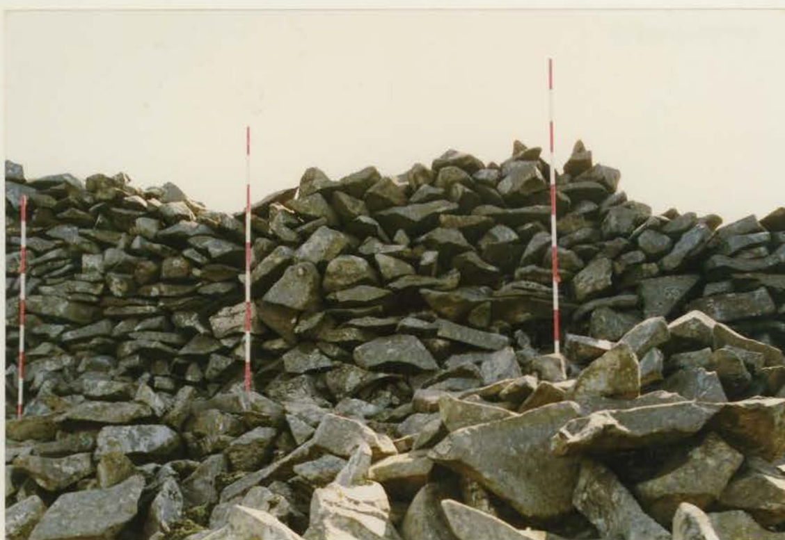
Plate 24 G1022/160/12 ; Collapse H13, showing voids in the facing before conservation.
