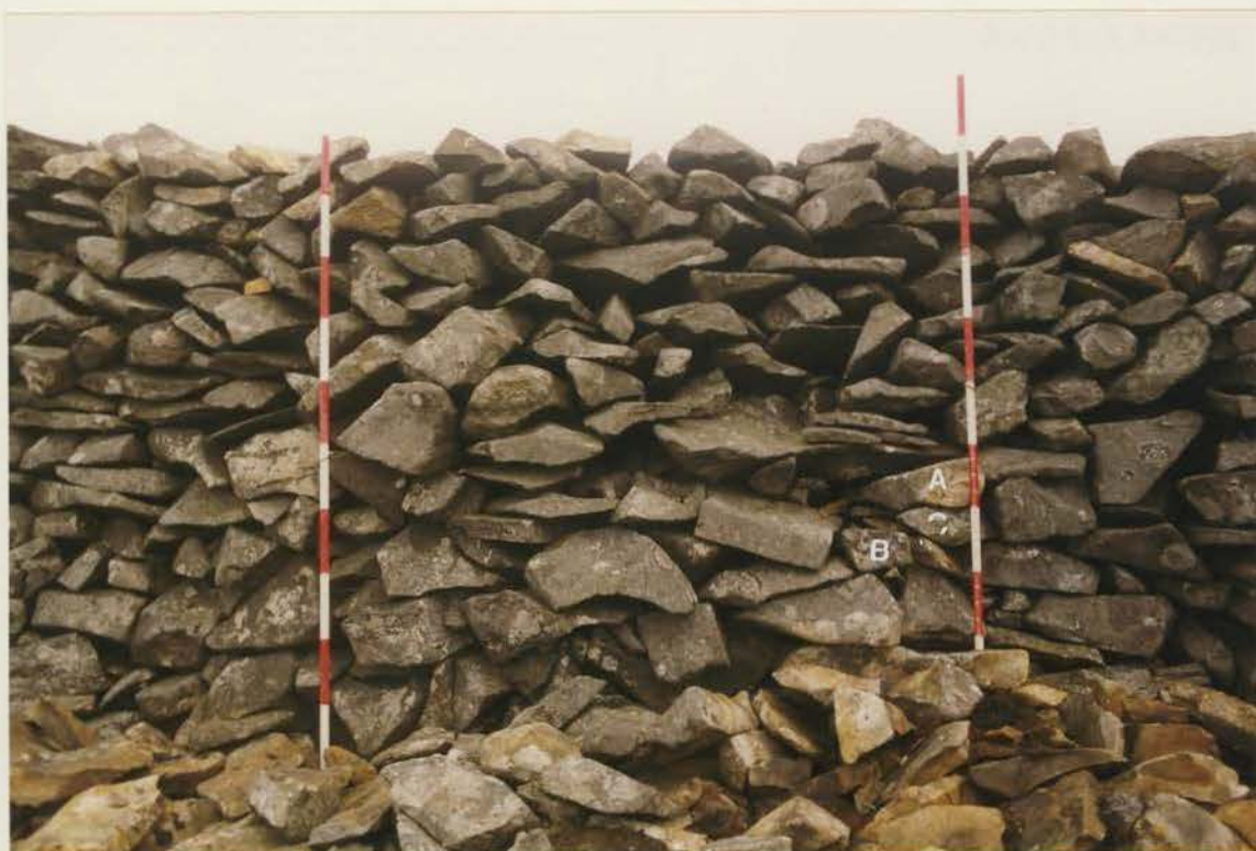
Plate 25 G1022/171/02 ; Collapse H13, showing voids in the facing after conservation.
