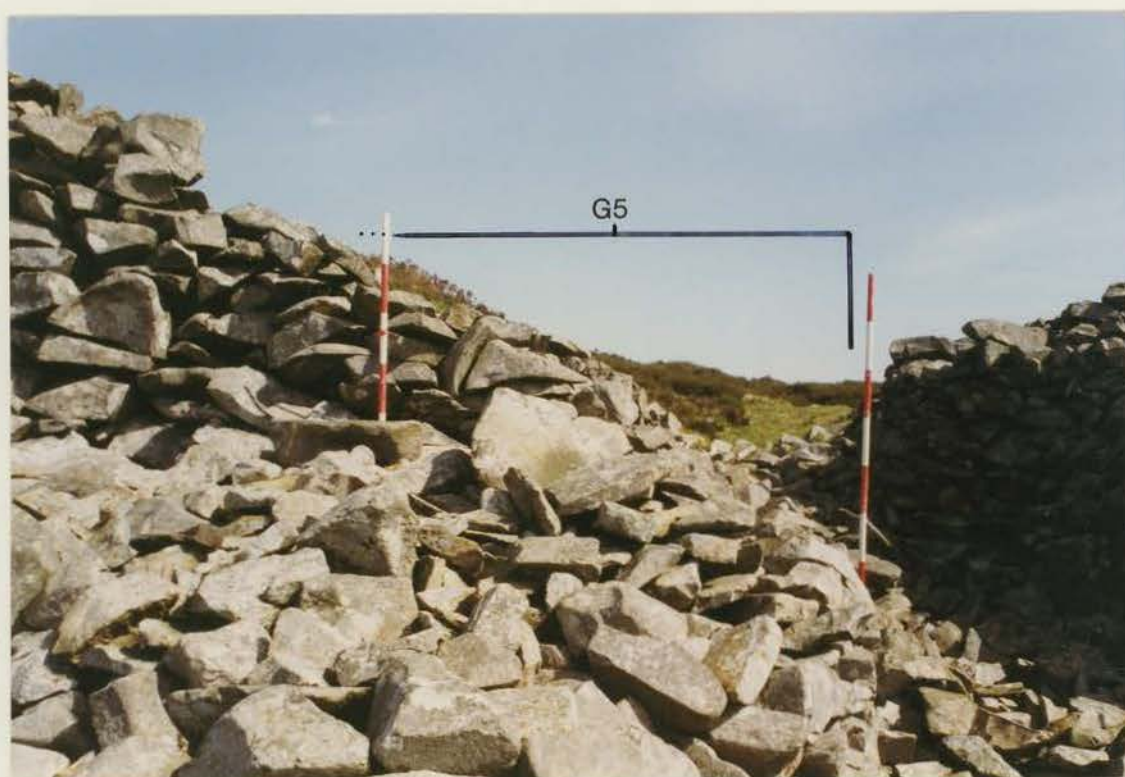
Plate 40 G1022/160/31 ; Collapse G5 before conservation.
