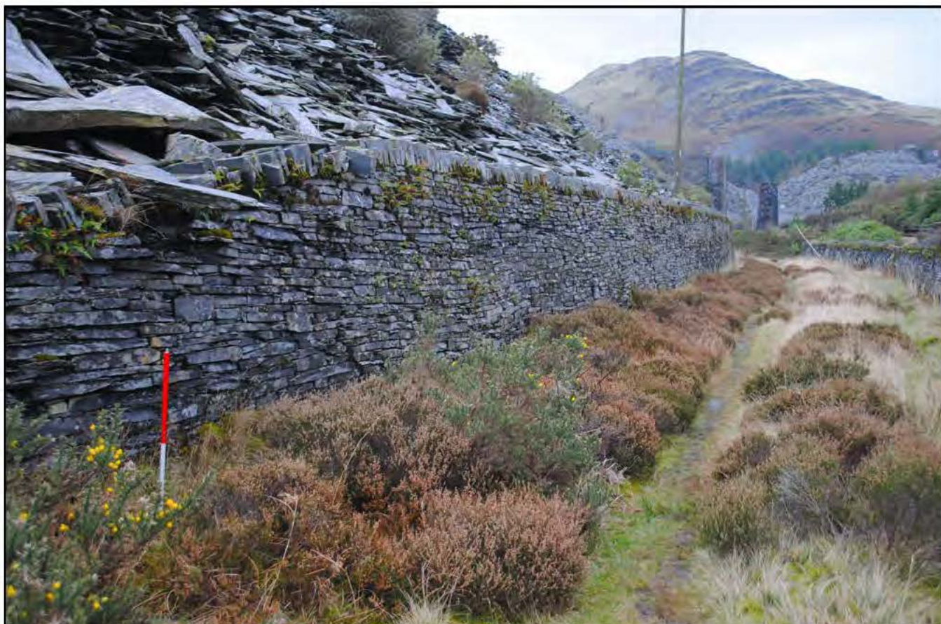
Plate 10: View of drystone slate walling, revetting slate tips. Photograph taken from the east
