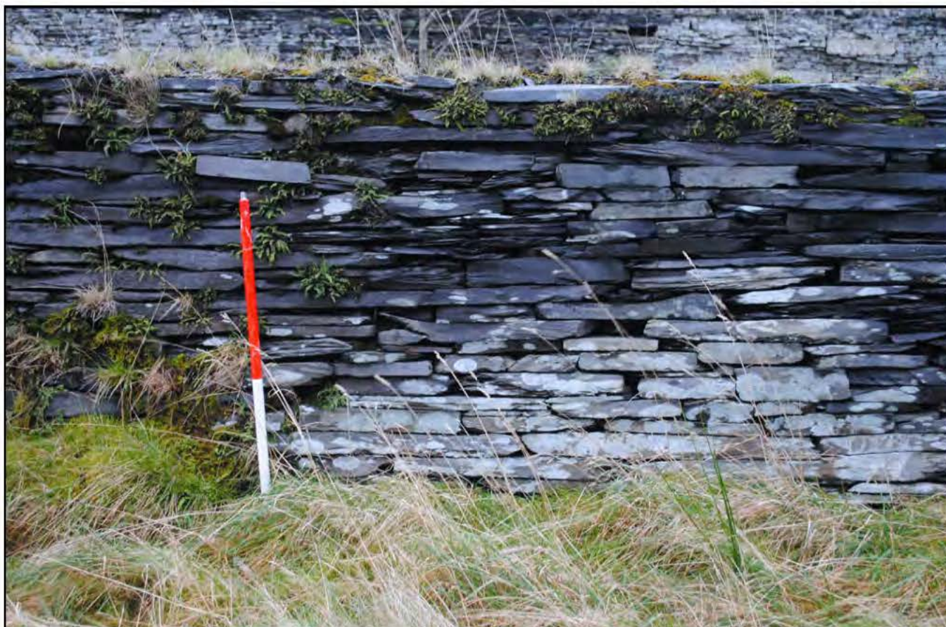
Plate 12: Detailed shot showing slate drystone walling.
