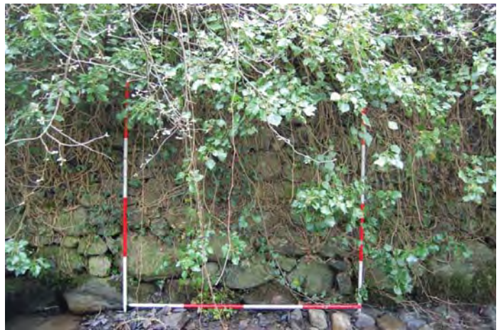
Plate 18: Large boulders forming wall foundation (002) and upper wall (003), from the N
