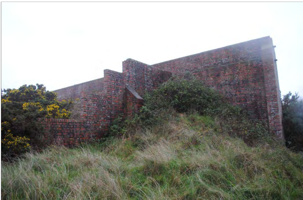
Plate 14: Rifle Range, showing buttressing and revetment RAF Llanbedr (PRN 32273)
