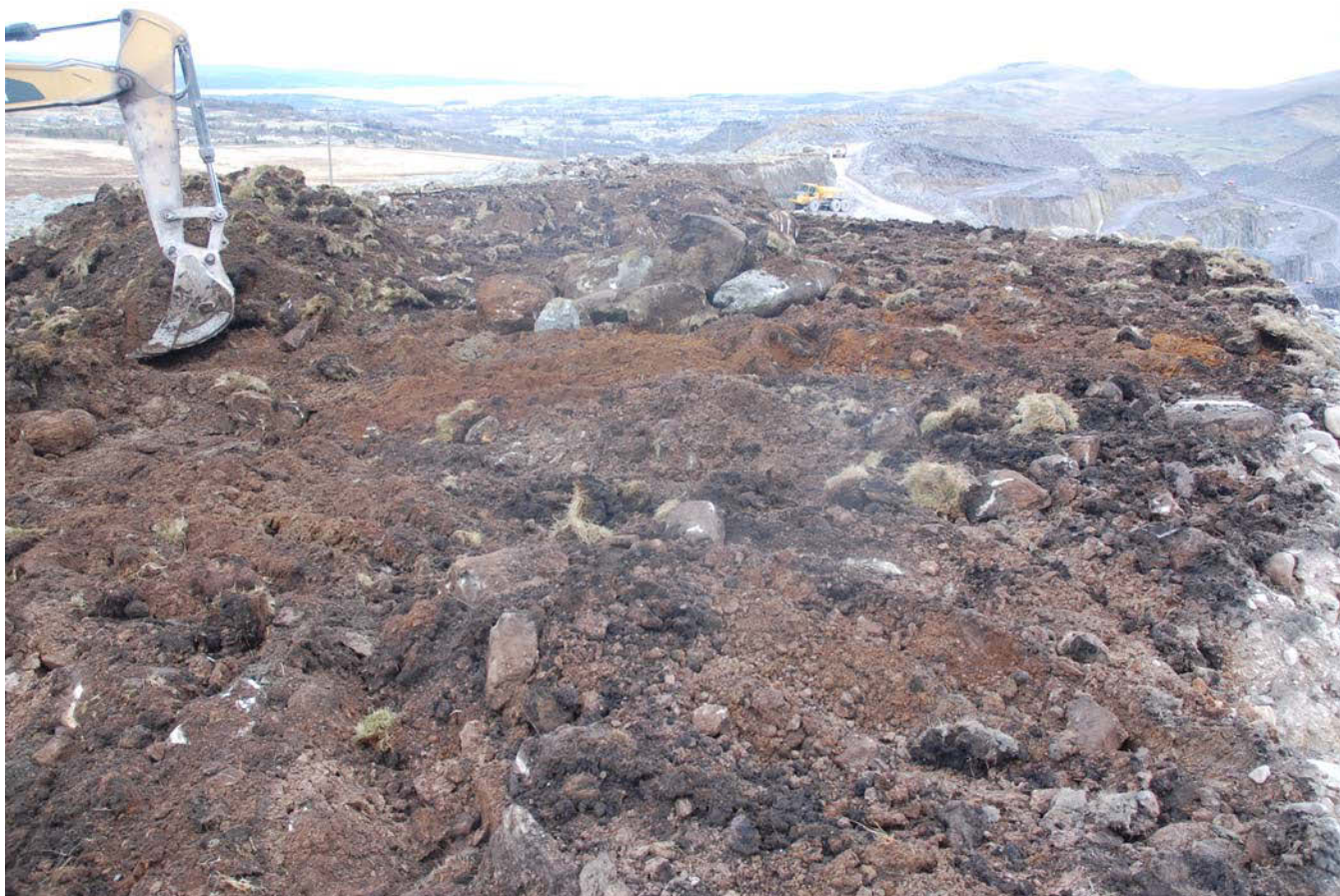
Plate 01: Topsoil Stripping, view from southeast
