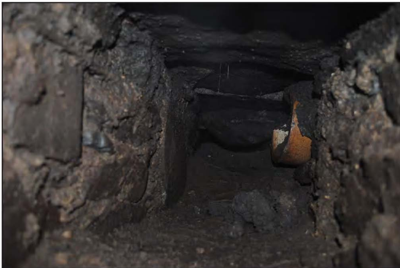
Plate 07: View along the length of the stone constructed drain showing subsequent reuse. A vitreous drain pipe encased with road mastic. The road mastic also appears to have partly sealed the drain as it passes under the A547 (Conway Road).
