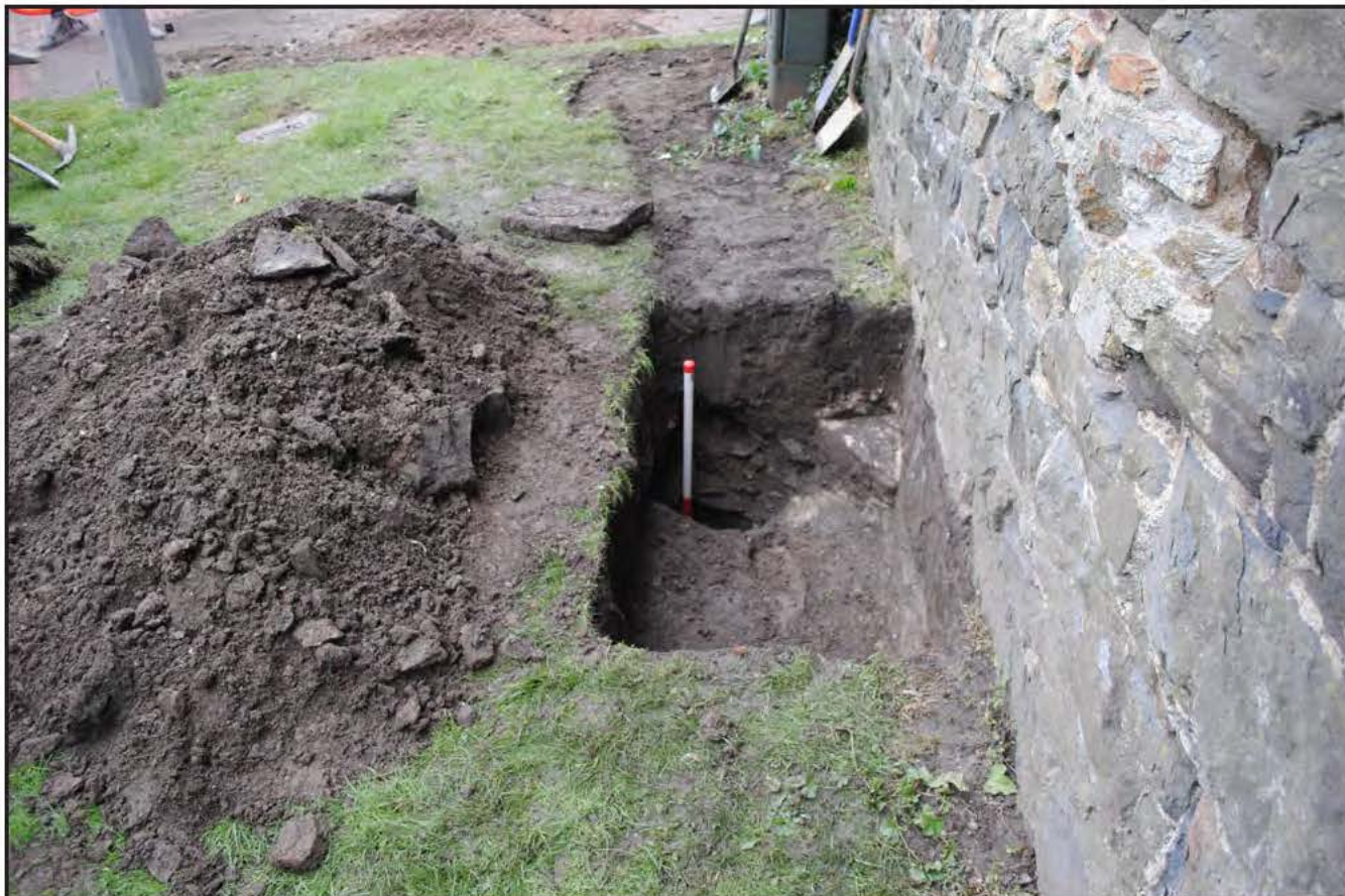
Plate 05: Ranging Pole inserted into the stone constructed drain with the concrete slab which had been placed over it visible in the background. Scale: 1x1m.
