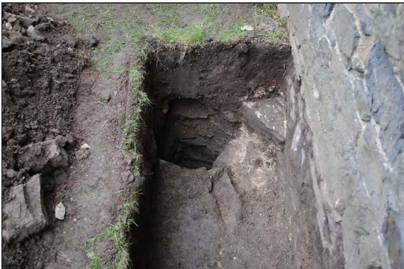
Plate 06: The hard mortar surface visible under the triangular stone, and also on top of the stone forming the north-eastern side of the stone constructed drain.
