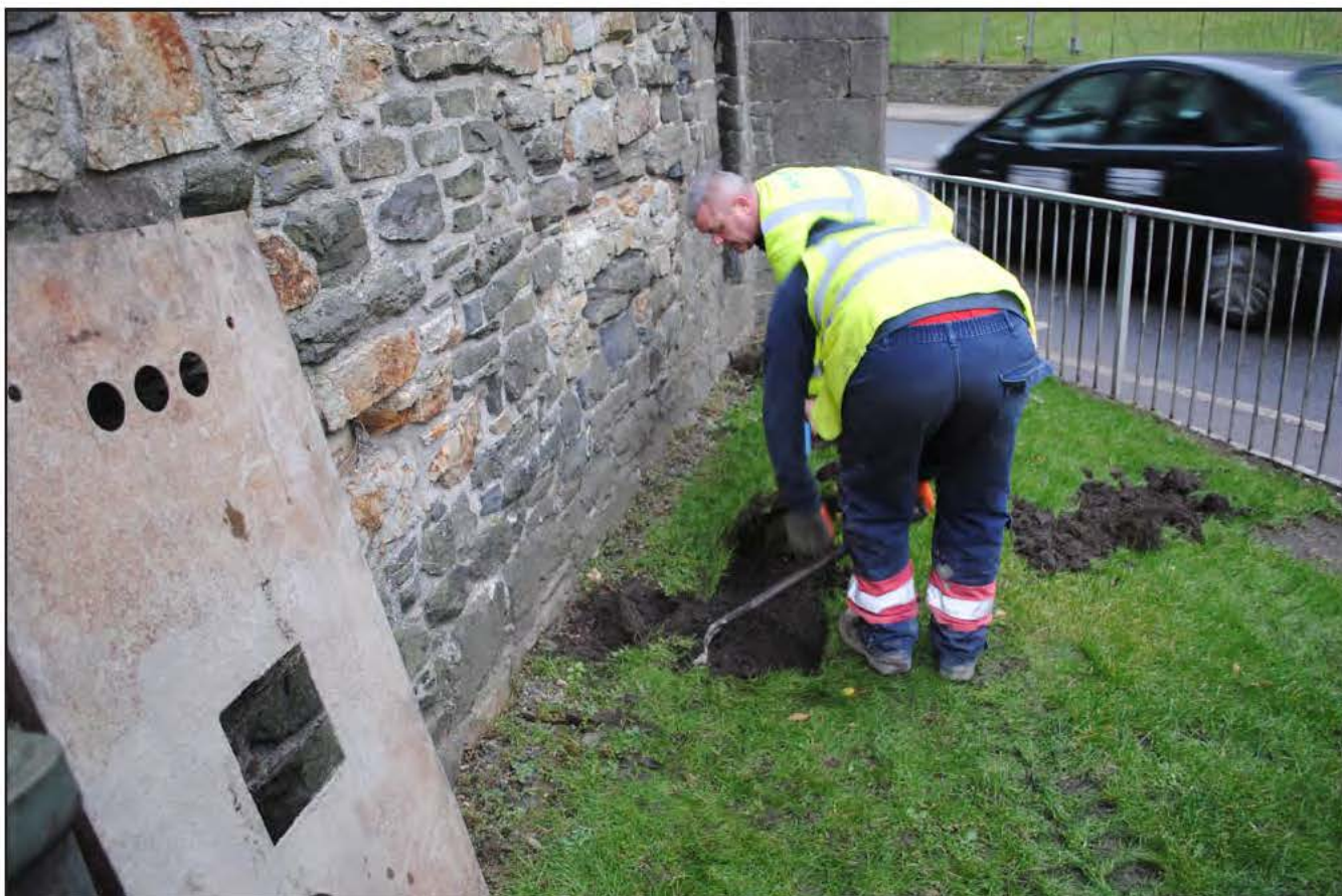
Plate 02: Excavation by Groundworkers of the Proposed Installation location of the BT Openreach Cabinet using a pre-formed template (foreground).
