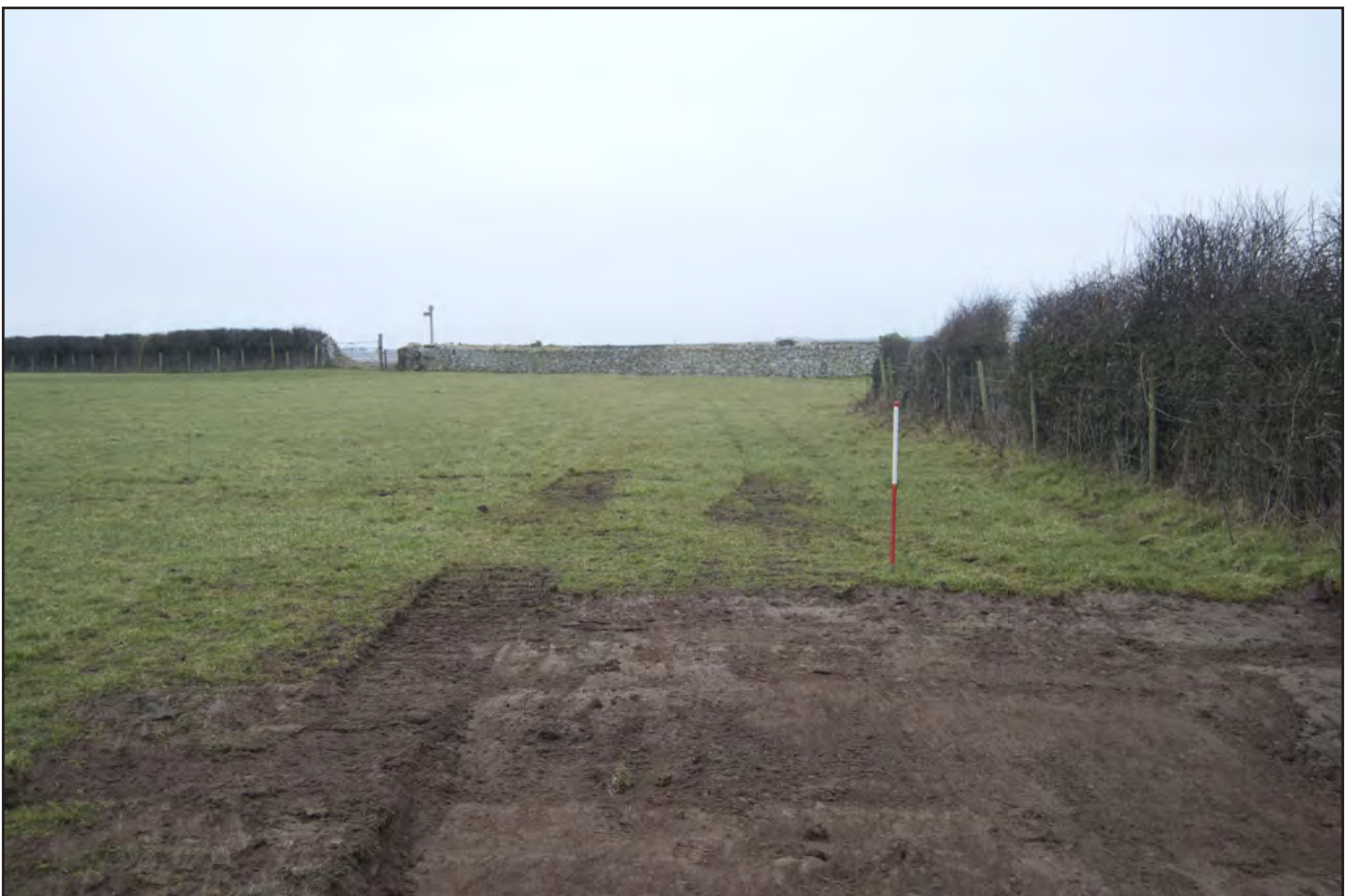
Plate 02: Section of track to be reduced only to turf level and built up to nearly height of wall, roughly 36m in length. 1x1m scale. As seen from the WNW.
