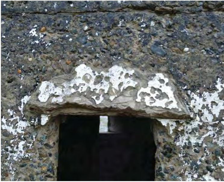
Plate 27. Render hood over embrasure in north-east wall (29/10/2015)
