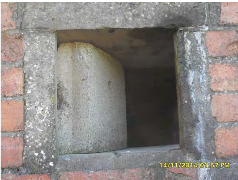
Plate 9. Embrasure plug in partially open position at Egryn, near Llanaber; External view. (Photo taken by Matt Rimmer)
