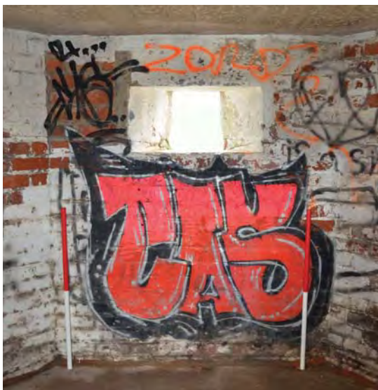
Interior of west wall
