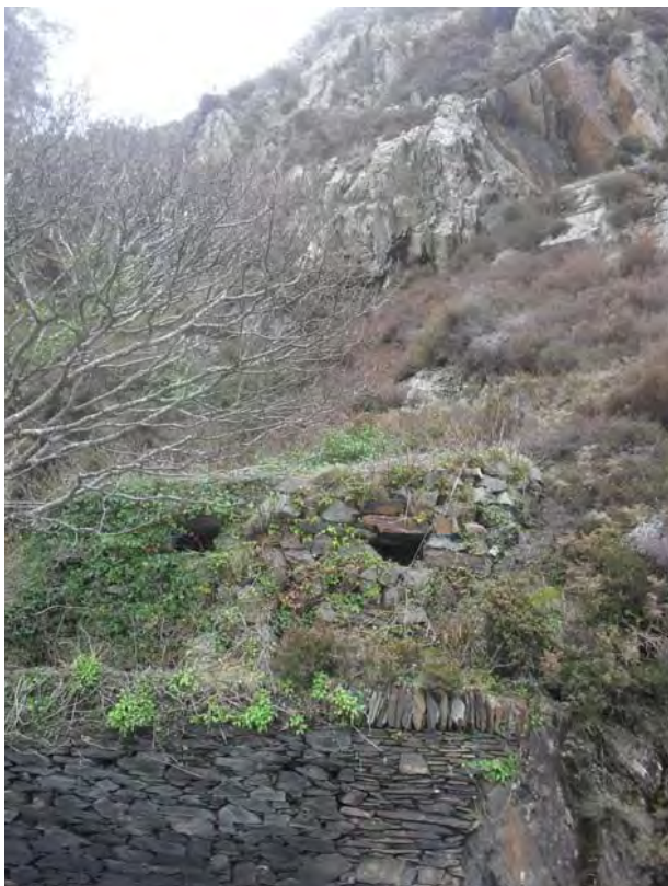
Plate 6. Pillbox built into the rocky hillside, at Aberamffra, Barmouth (Photo taken by Matt Rimmer)
