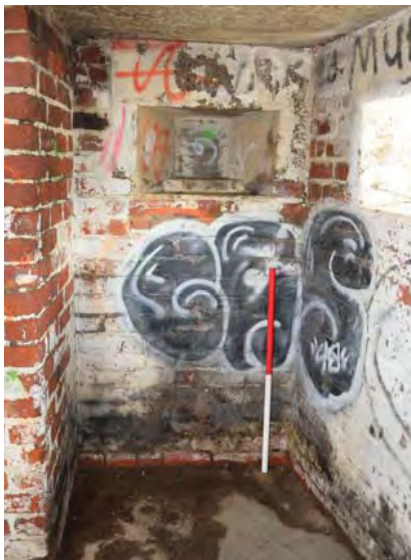
Interior of east wall south of door
