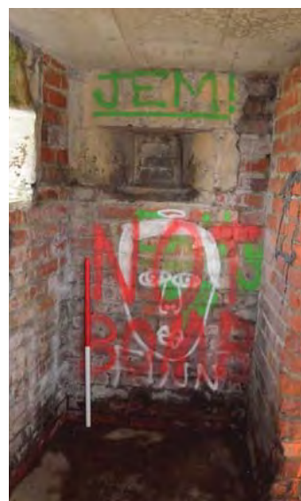
Interior of east wall north of door
