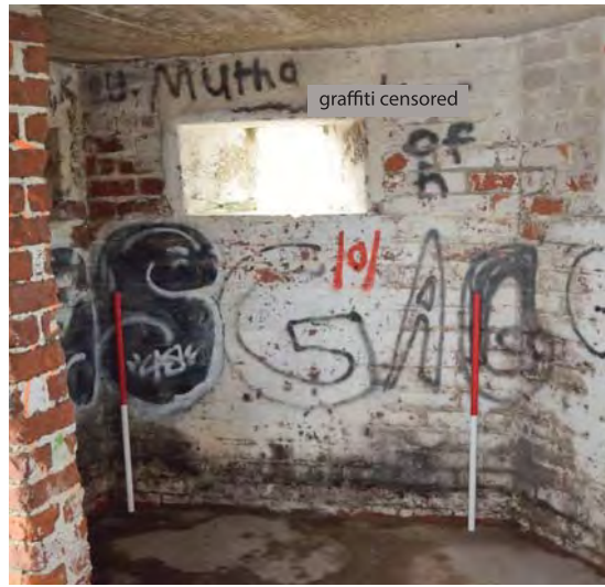
Interior of south-east wall
