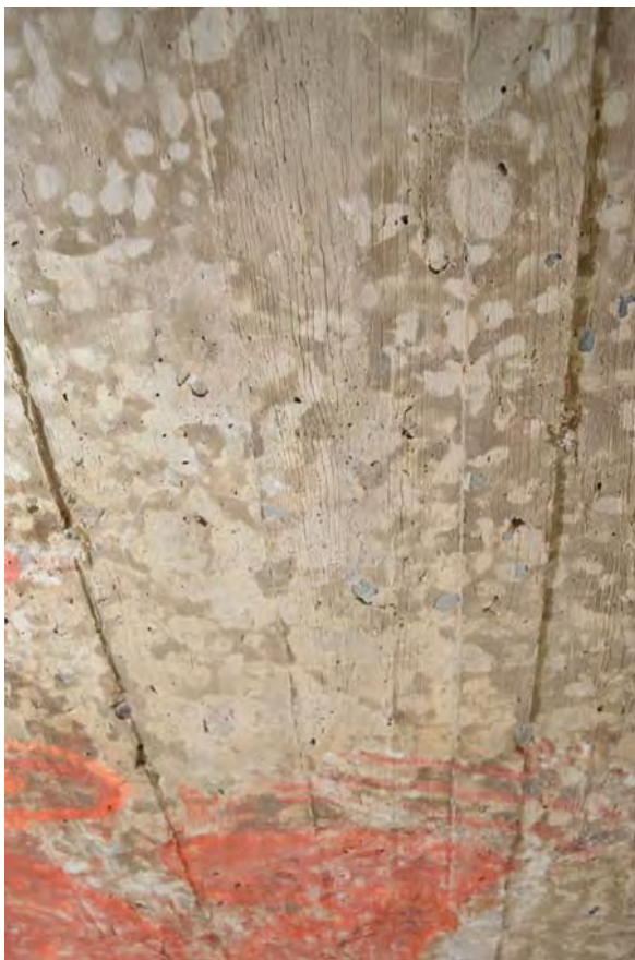
Plate 21. Cast of planks with wood grain in ceiling of pillbox PRN 34151 (27/10/2015)
