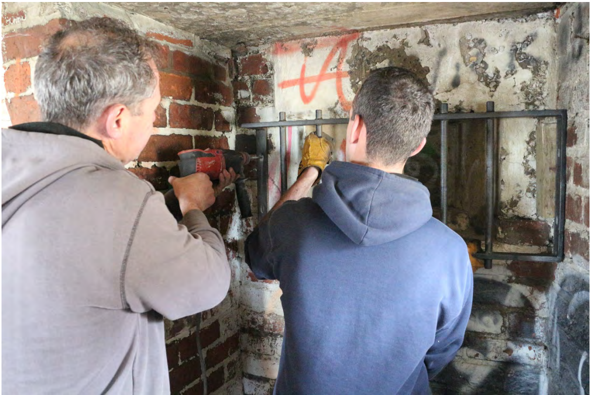
Drilling mortar joints for fixing points for the embrasure grilles, IMG_8320, 27.10.2015
