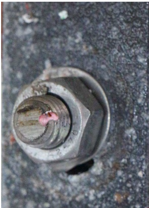
Steelwork fixings, before (left) and after (right) installation of A2 stainless steel armour rings, IMG_9805 and IMG_9806, 03.03.2016
