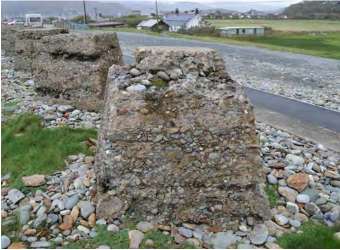
Plate 40. Eroding anti-tank blocks south of pillbox PRN 34151. The construction in layers with beach pebbles can also be seen picked out by the erosion (29/10/2015)
