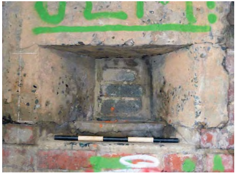
Plate 24. Interior of blocked embrasure at north end of east wall (27/10/2015)
