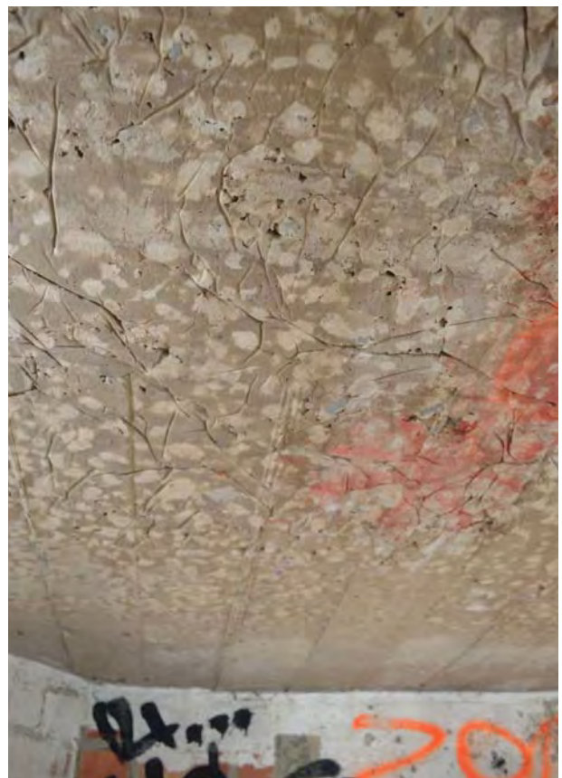
Plate 22. Cast of tar paper with over planks in ceiling of pillbox PRN 34151 (27/10/2015)
