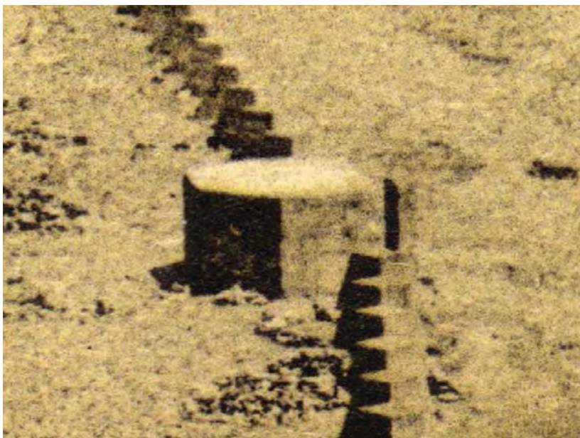
Plate 12. Enlargement from the above image, showing the external blast wall to the rear of the pillbox PRN 34150
