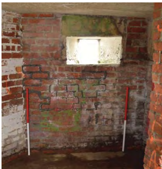
Interior of north-east wall
