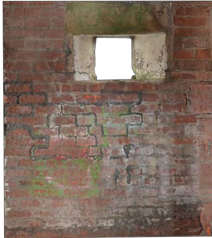
Internal elevation of north-east wall
