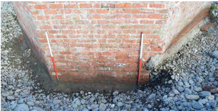
Plate 25. Detail of concrete foundations from west (26/10/2015)
