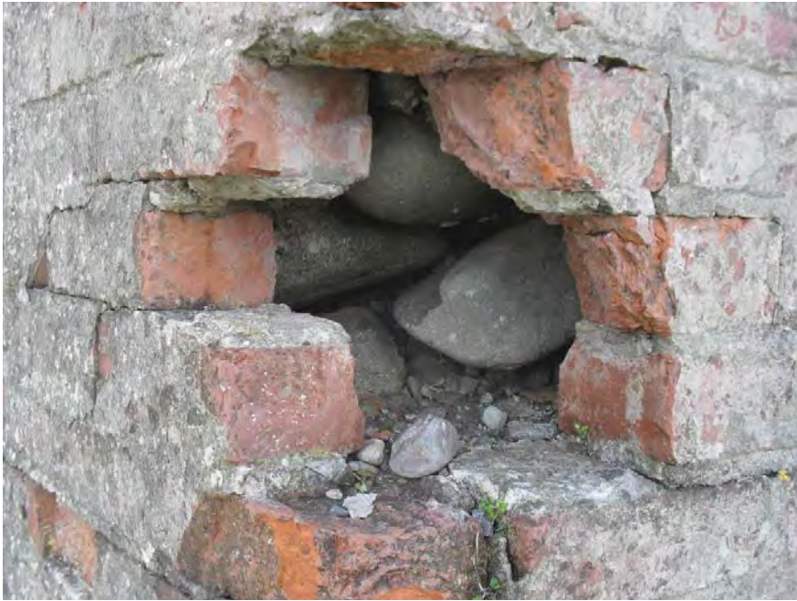
Plate 4. Pebble and concrete core to pillbox wall, as seen in southernmost pillbox (PRN 34150) before its destruction. (Photo taken by Matt Rimmer 2013)
