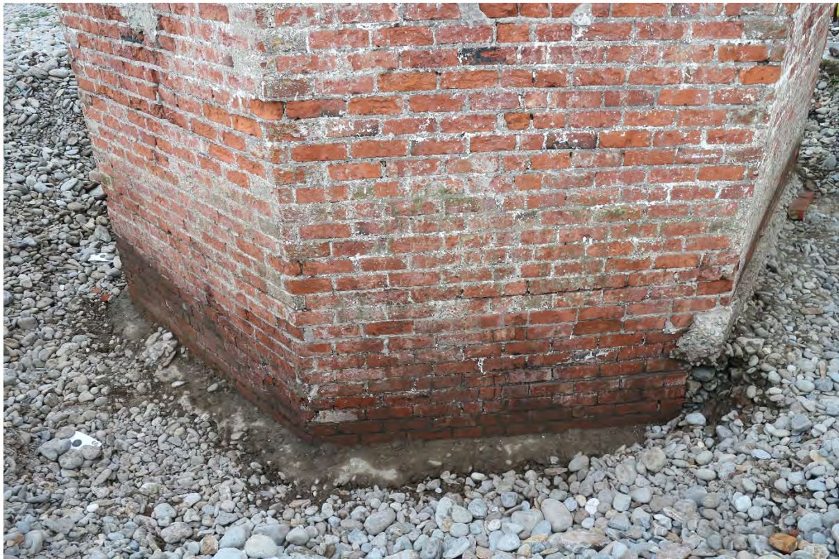
Fully revealed footings and lower brickwork courses, IMG_8296, 26.10.2015
