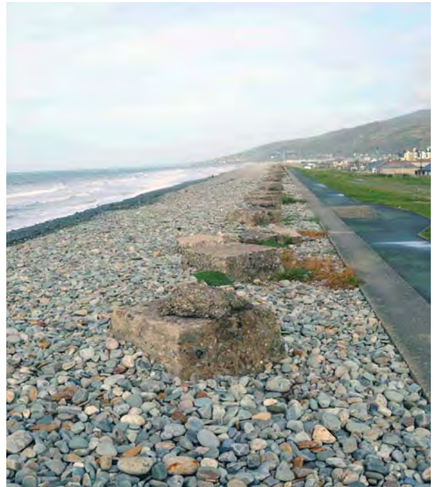
Plate 37. Anti-tank blocks north of pillbox PRN 34151 largely buried. These also have cement from building the sea wall dumped on top of them (29/10/2015)
