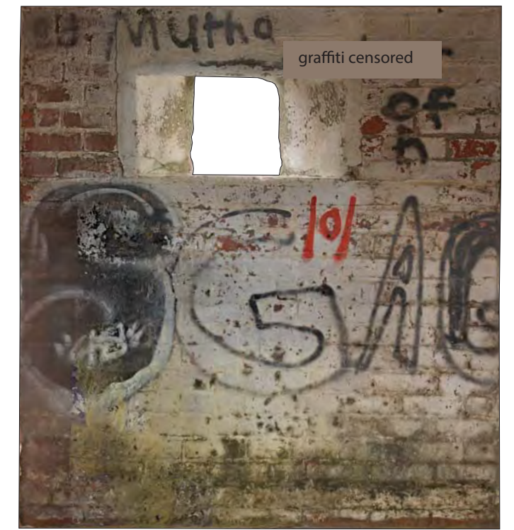
Internal elevation of south-east wall
