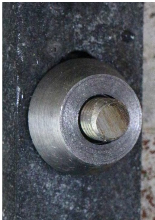
Steelwork fixings, before (left) and after (right) installation of A2 stainless steel armour rings, IMG_9805 and IMG_9806, 03.03.2016
