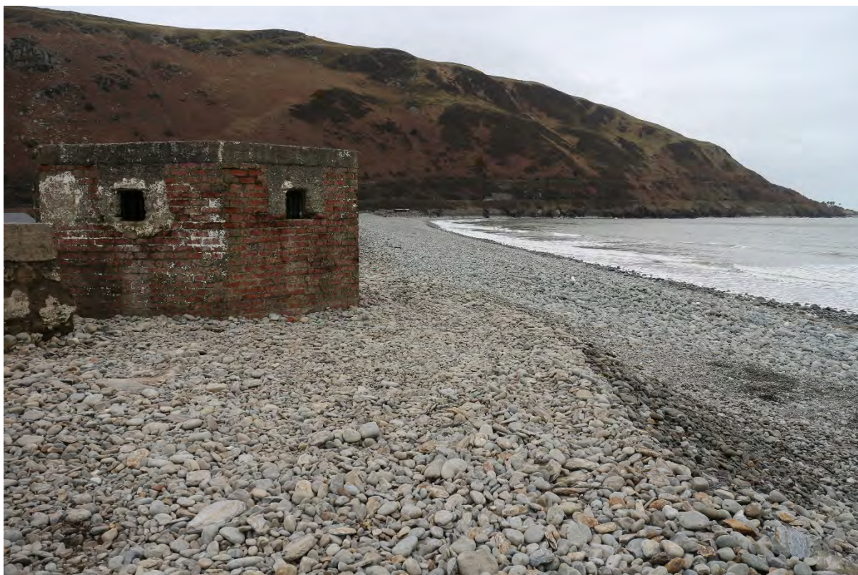
Shingle beach seaward of pillbox, following small-scale re-profiling, IMG_9827, 03.03.2016
