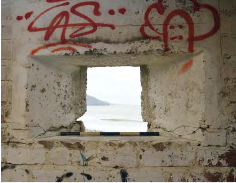
Plate 23. Interior of embrasure in south-west wall (27/10/2015)
