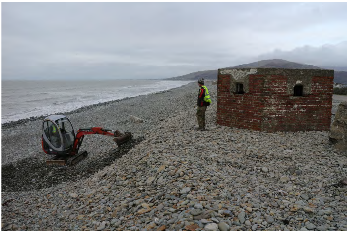
Re-profiling shingle following completion of exterior works, IMG_9824, 03.03.2016
