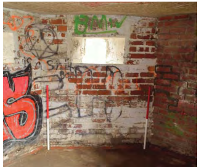
Interior of north-west wall
