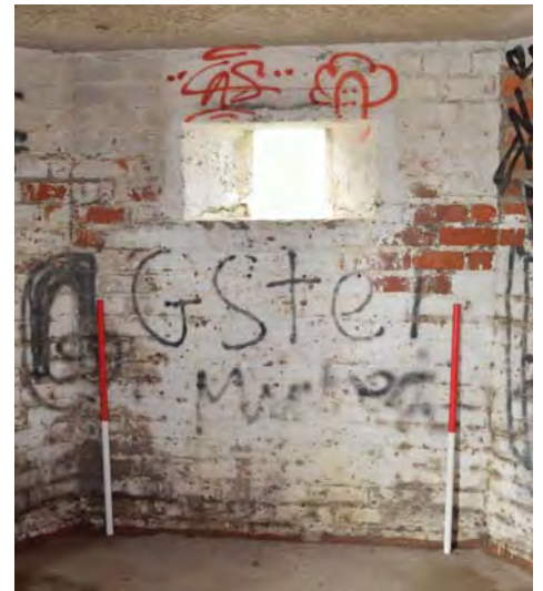
Interior of south-west wall
