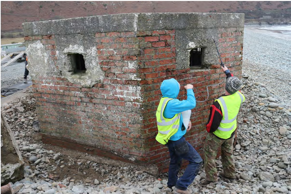
Applying Kingfisher Storm Seal, IMG_9800, 03.03.2016
