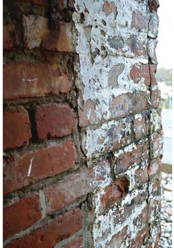
Plate 28. Junction of interior passage wall and main exterior wall (29/10/2015)
