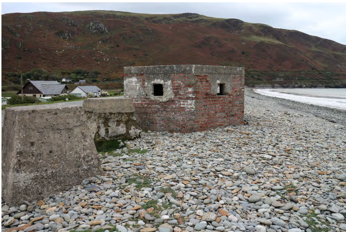
Shingle beach seaward of pillbox, before erosion during Storm Imogen, IMG_8272, 26.10.2015
