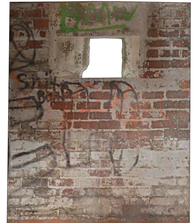
Internal elevation of north-west wall
