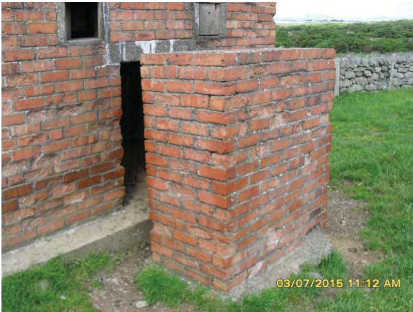
Plate 10. Intact example of an external blast wall protecting the entrance to the pillbox at Egryn, near Llanaber, Barmouth (Photo taken by Matt Rimmer)
