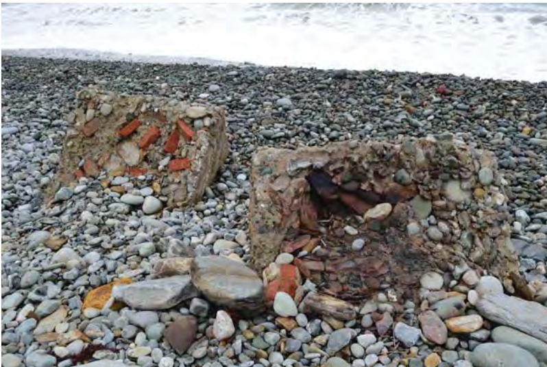
Plate 38. Anti-tank blocks at the southern end of the line toppled and moved. These show their construction using beach pebbles and bricks (29/10/2015)
