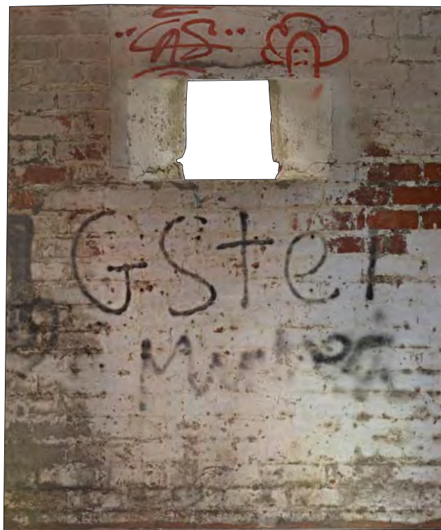
Internal elevation of south-west wall
