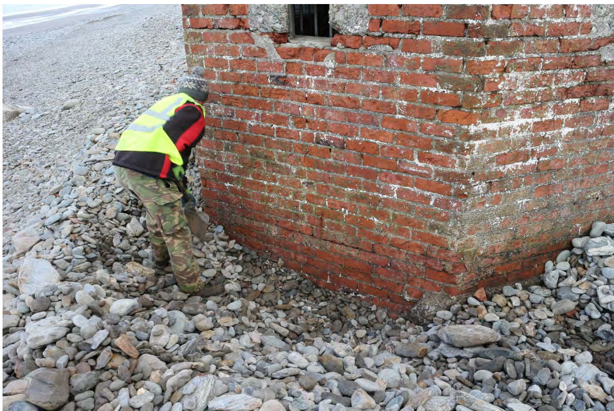
Removing beach pebbles from lower brickwork faces by hand, IMG_9776, 03.03.2016
