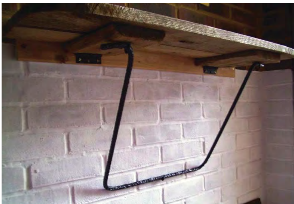
Plate 15. Another design of folding shelf found in some pillboxes; Image courtesy of Tim Denton of the Pillbox Study Group
