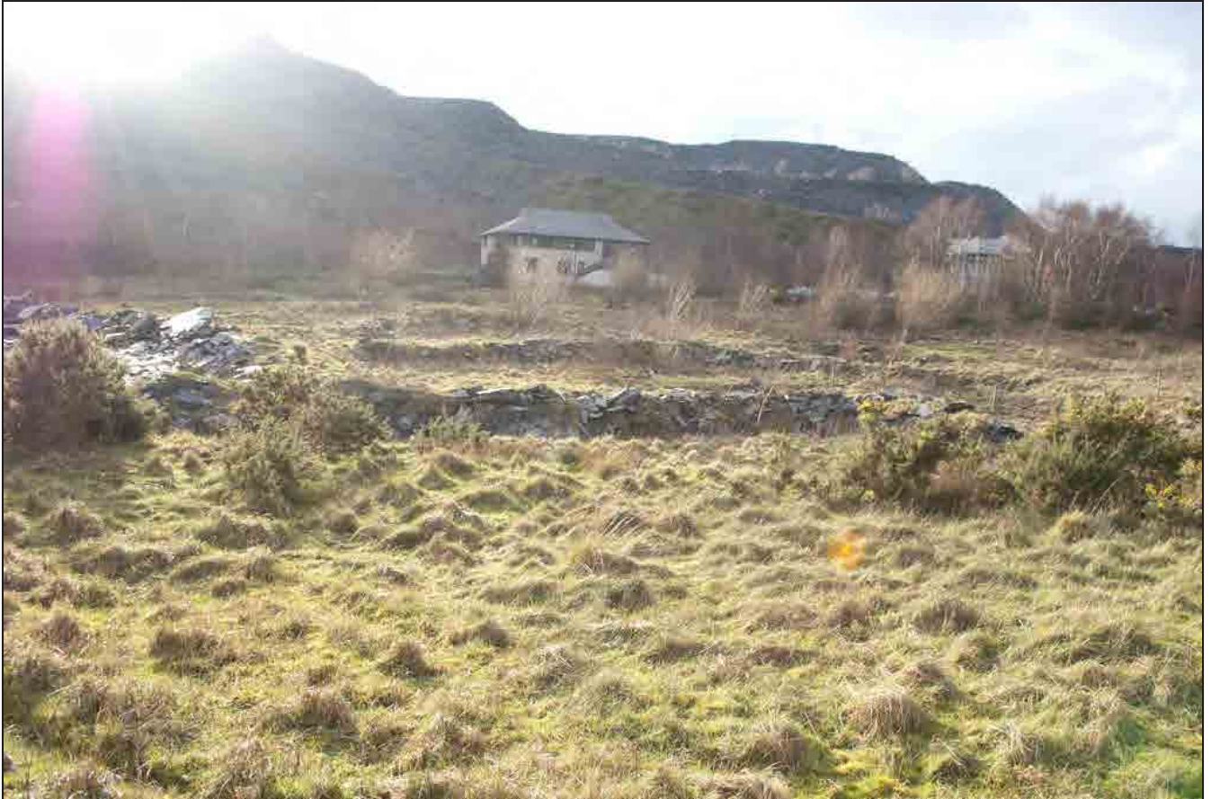
Plate 05: General view of the slate built earthwork showing the slight graduation in height. View from the Northeast.
