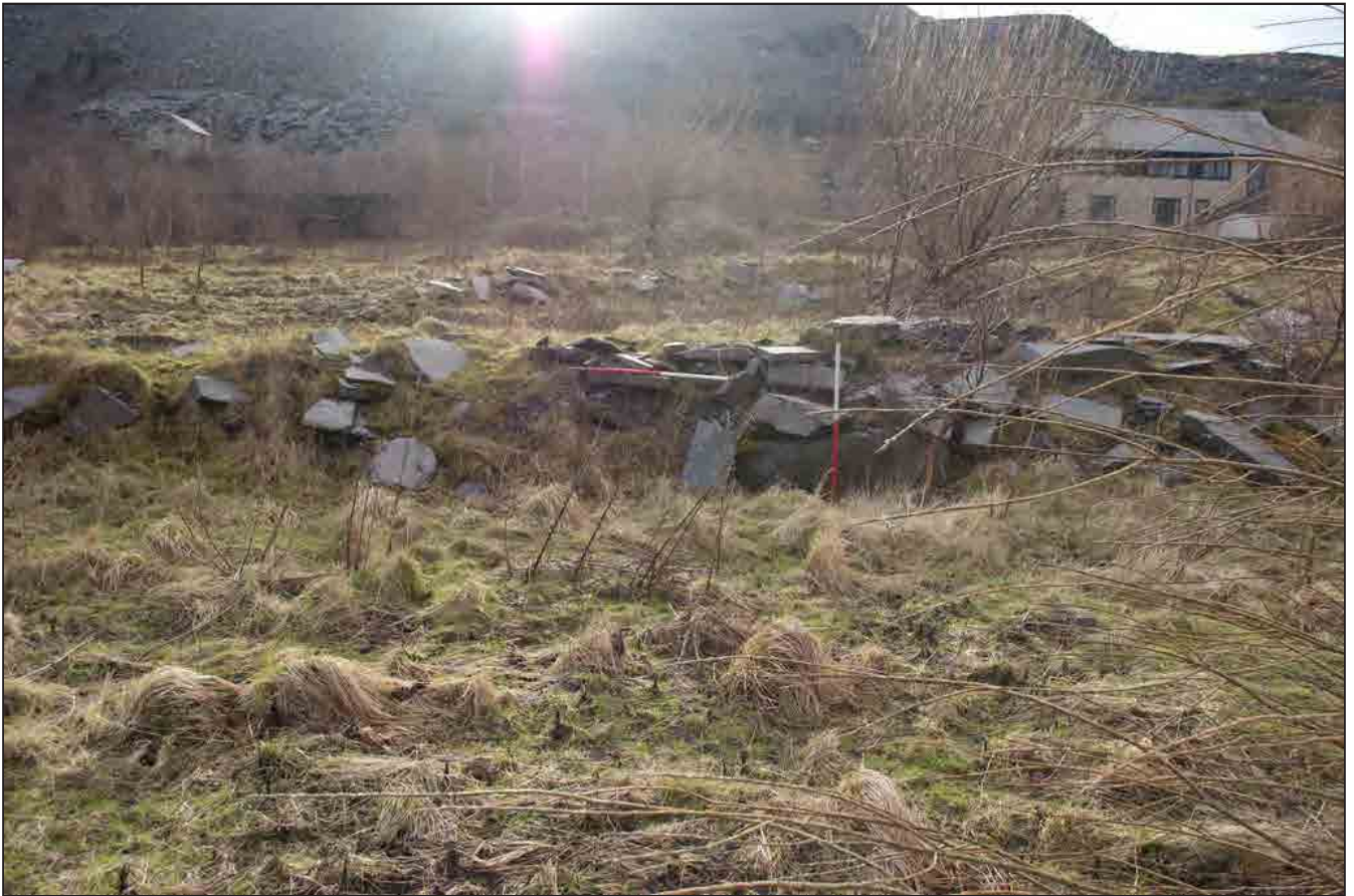
Plate 03: A close up of a low un-bonded section of wall formed of poorly sorted blocks of slate, standing up to a meter in height View from the North; scale 2 x 1m.
