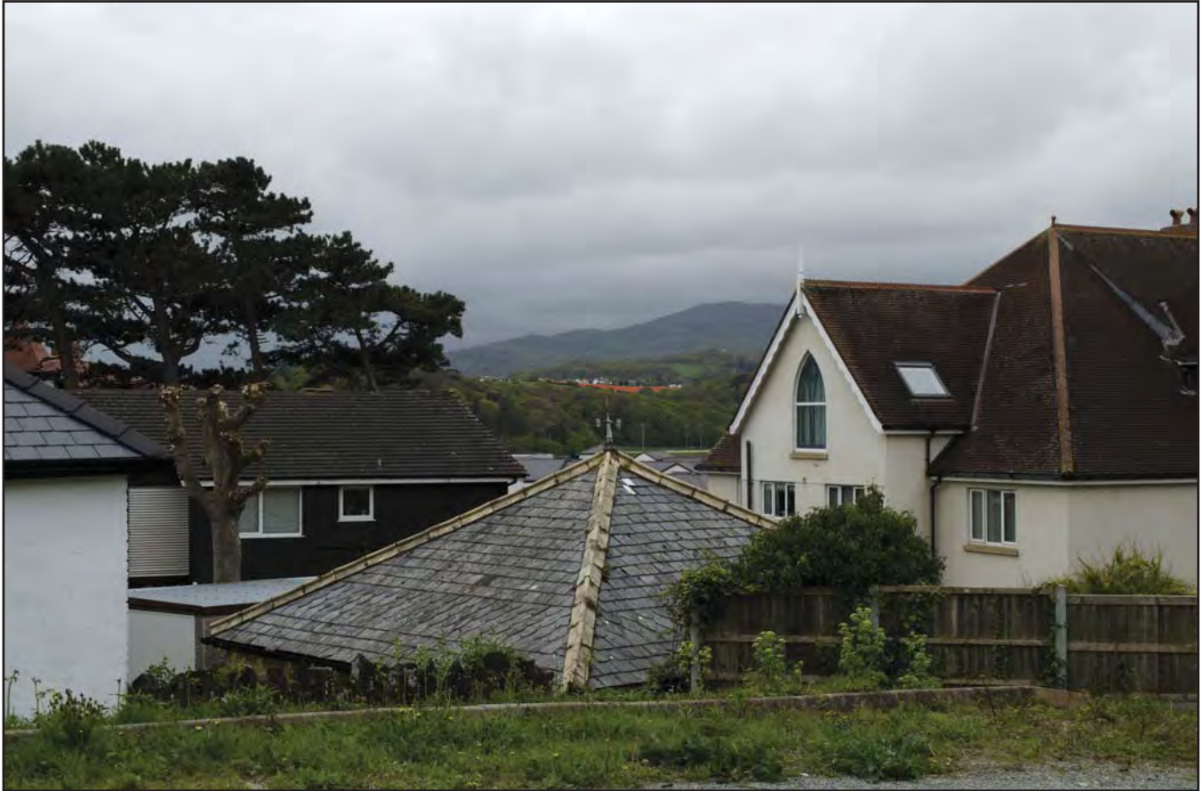
Plate 17: View towards the Proposed Development from land to the south of All Saints Church, Deganwy. The approximate extent of the footprint of the Proposed Development is highlighted in red. Viewed from the north-east
