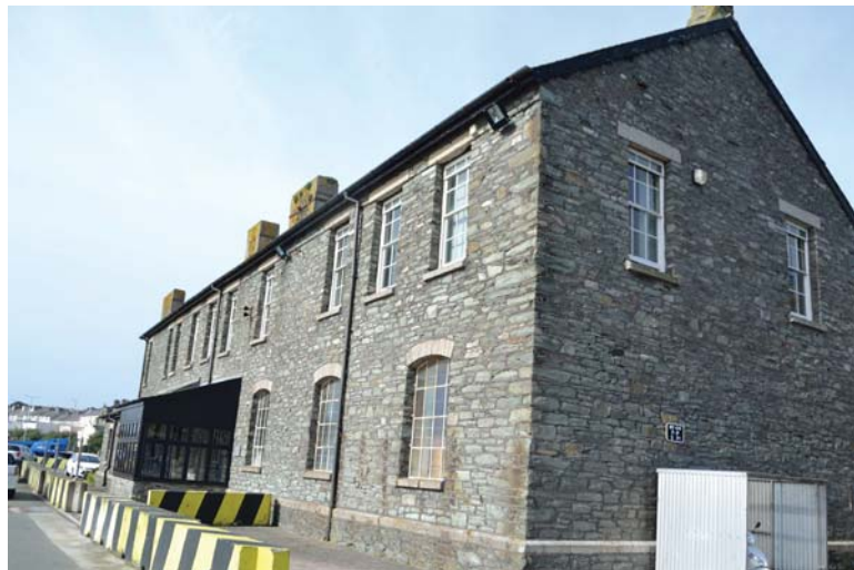
Plate 18. The offices and stores in Marine Yard
