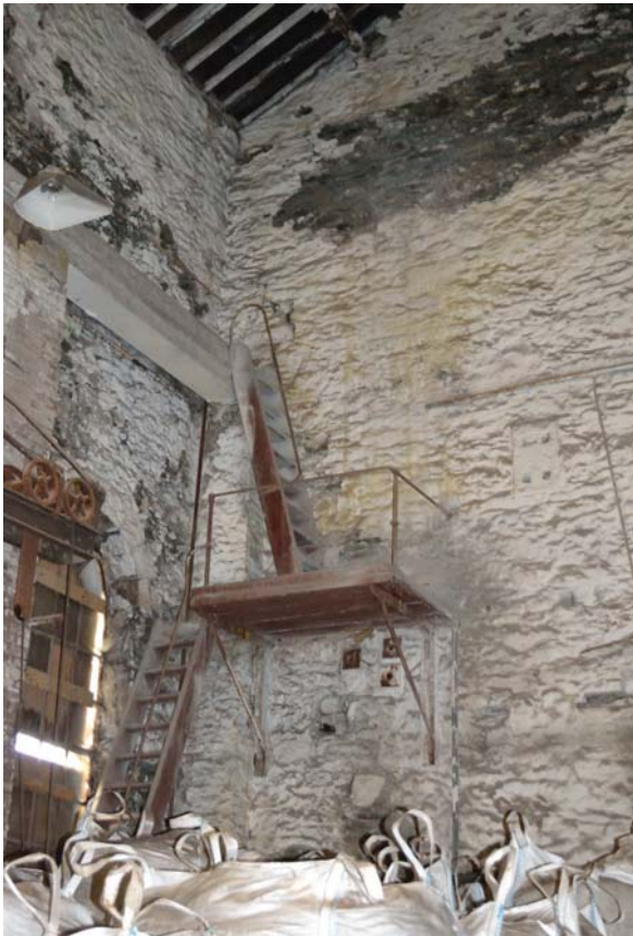
Plate appII.11. Stairs leading to crane in boiler shop (PRN 11824)
