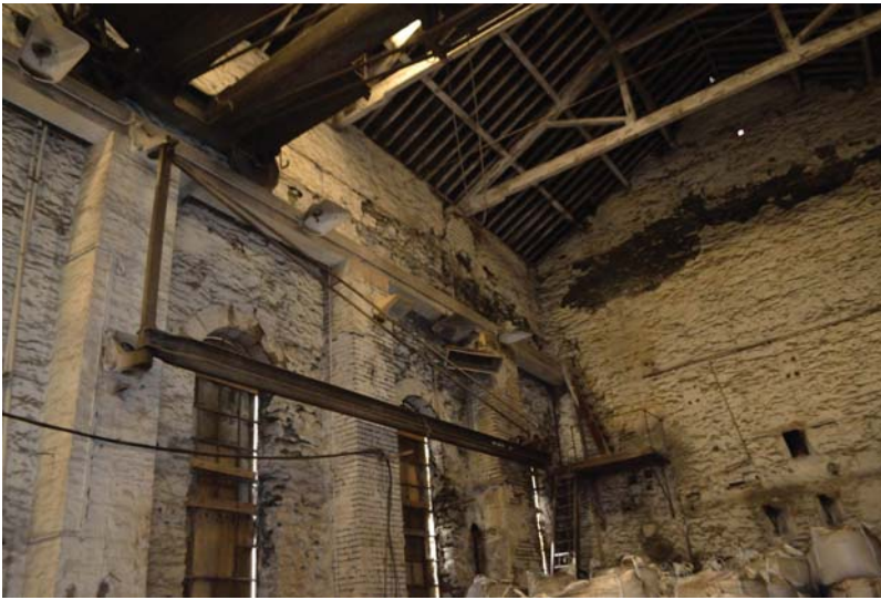
Plate appII.9. Winch on east elevation of boiler shop (PRN 11824)
