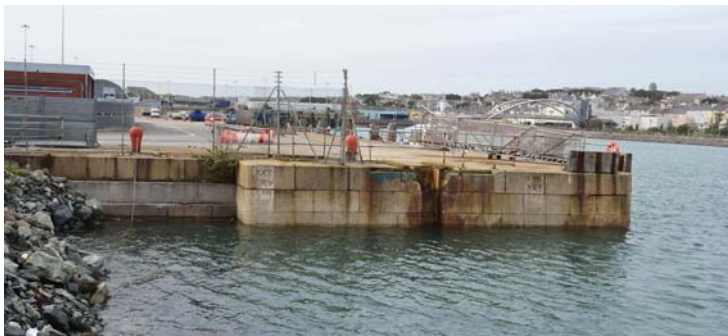
Plate 15. Part of the entrance wall to the large graving dock (PRN 16083)
