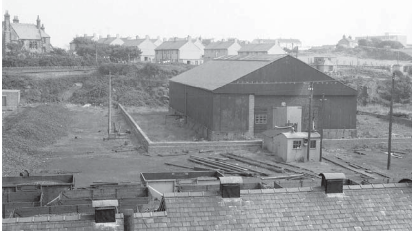
Plate 14. The Pontoon House Workshop showing the bund wall around it (image kindly provided by John Cave)
