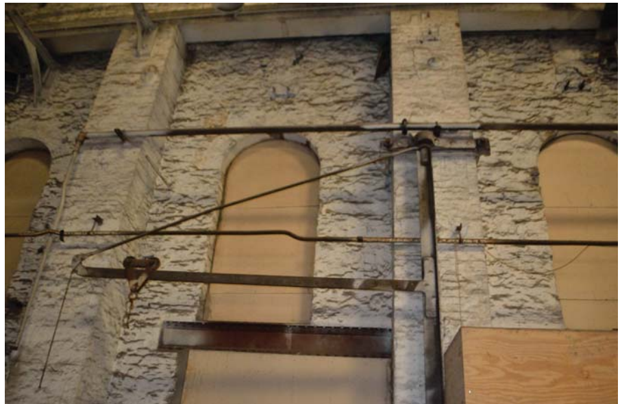
Plate appII.10. Winch on north-east elevation of boiler shop (PRN 11824)
