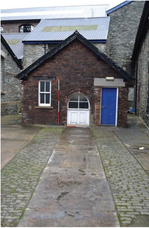
Plate appII.1. Engine house for sheerlegs (PRN 33999)
