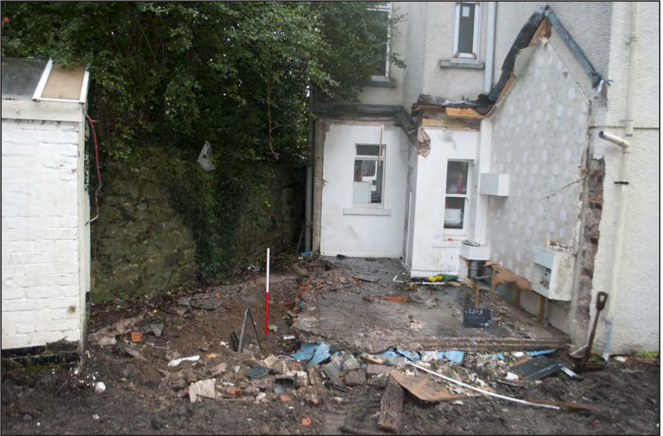
Plate 4: View of conservatory area subsequent to wall footing removal; slate floor in place; scale: 1x1m (archive reference: G2573_011).
