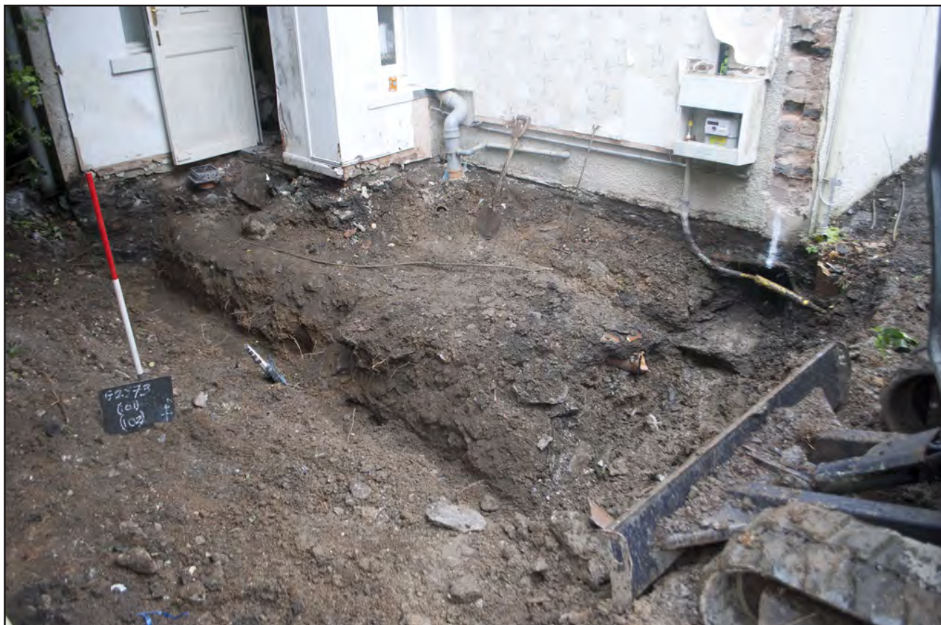
Plate 5: Angled view of new foundation trenches post-excavation; scale: 1x1m (archive reference: G2573_019).
