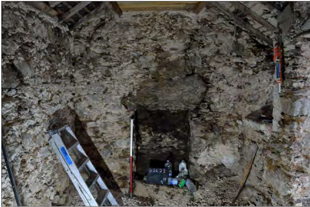
Plate 21: North wall of cottage - render removed to expose stone work; scale: 1x1m (archive reference: G2623_065).
