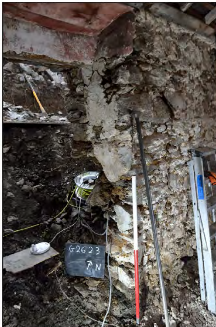
Plate 22: Opening at rear, western end of the cottage, for new doorway; scale: 1x1m (archive reference: G2623_080).
