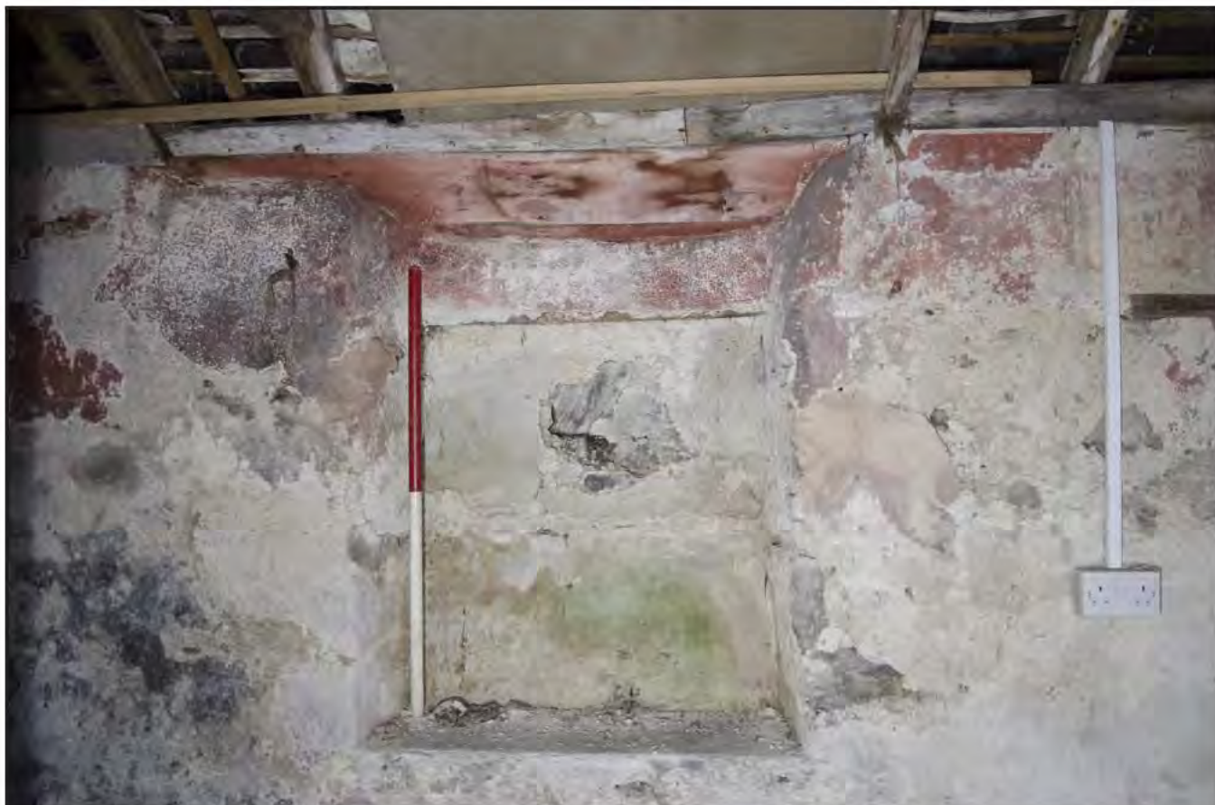
Plate 13: Blocked window in western wall; scale 1x1m (archive reference G2623_022).
