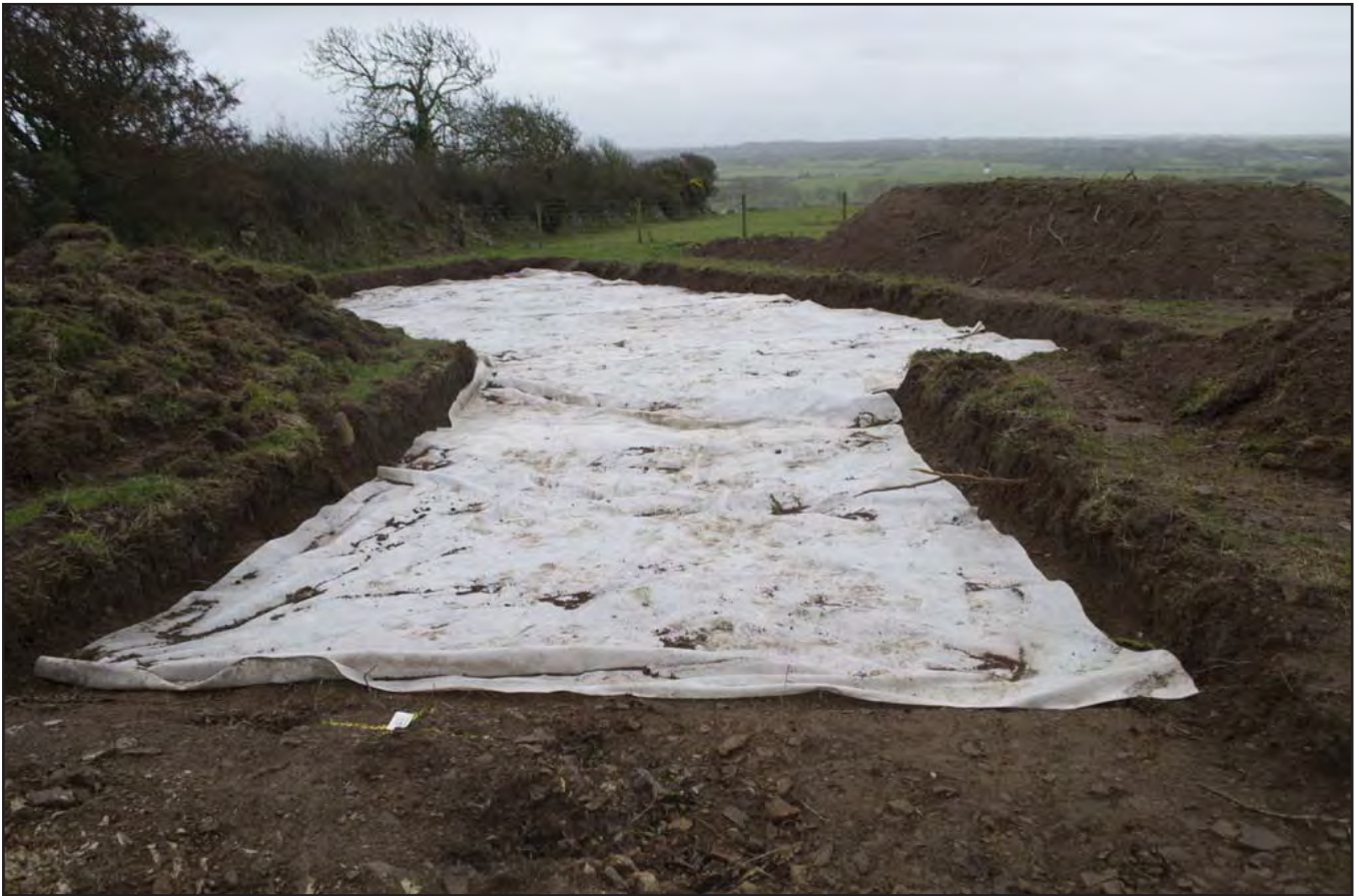
Plate 17: Herringbone drainage field - geotextile membrane prior to backfilling; scale: not used (archive reference: G2488_071).
