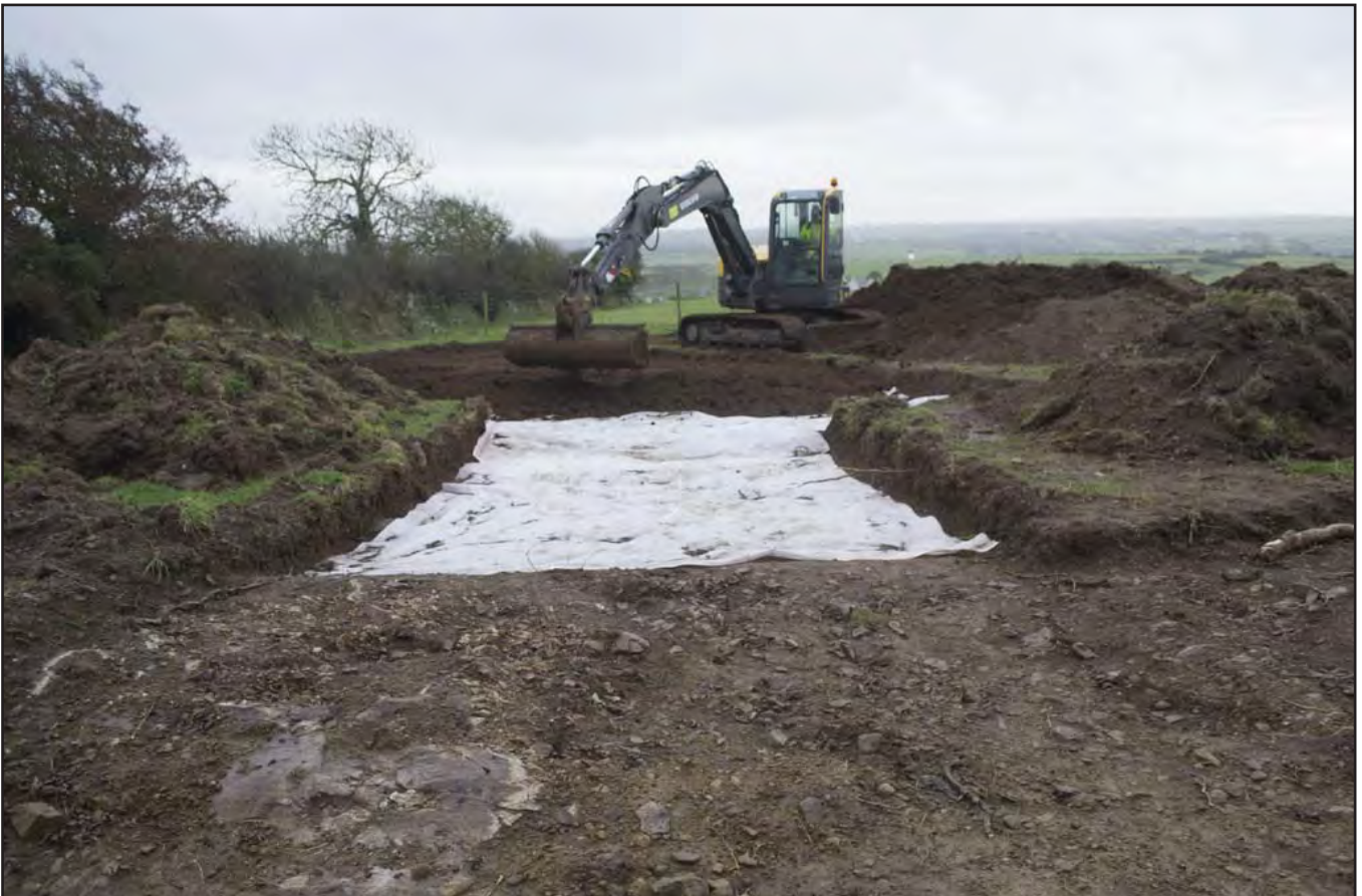
Plate 18: Herringbone drainage field - during backfilling over geotextile membrane; scale: not used (archive reference: G2488_072).
