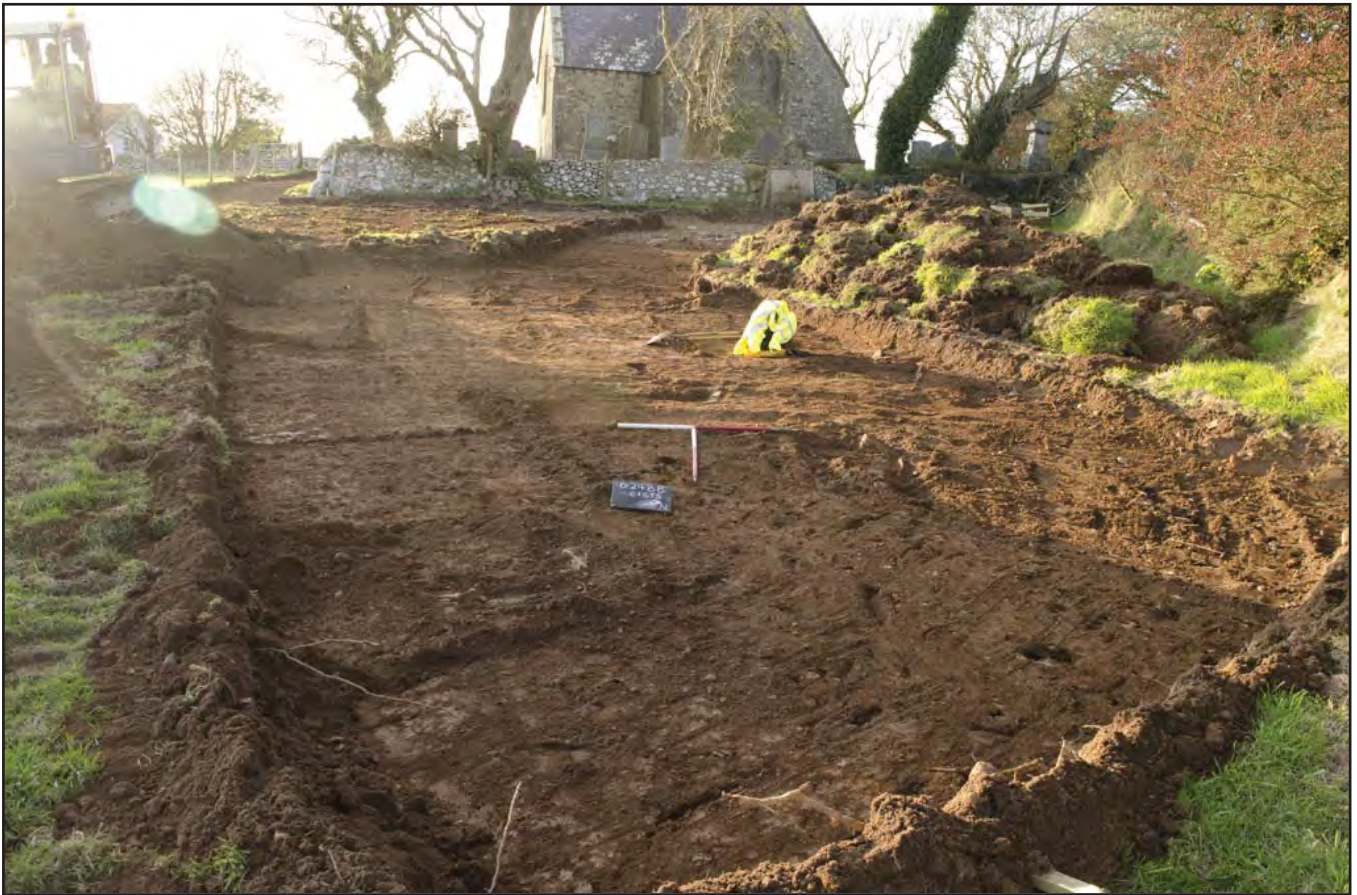
Plate 05: Herring bone drainage field - post topsoil strip; scale: 2x1m (archive reference: G2488_038).
