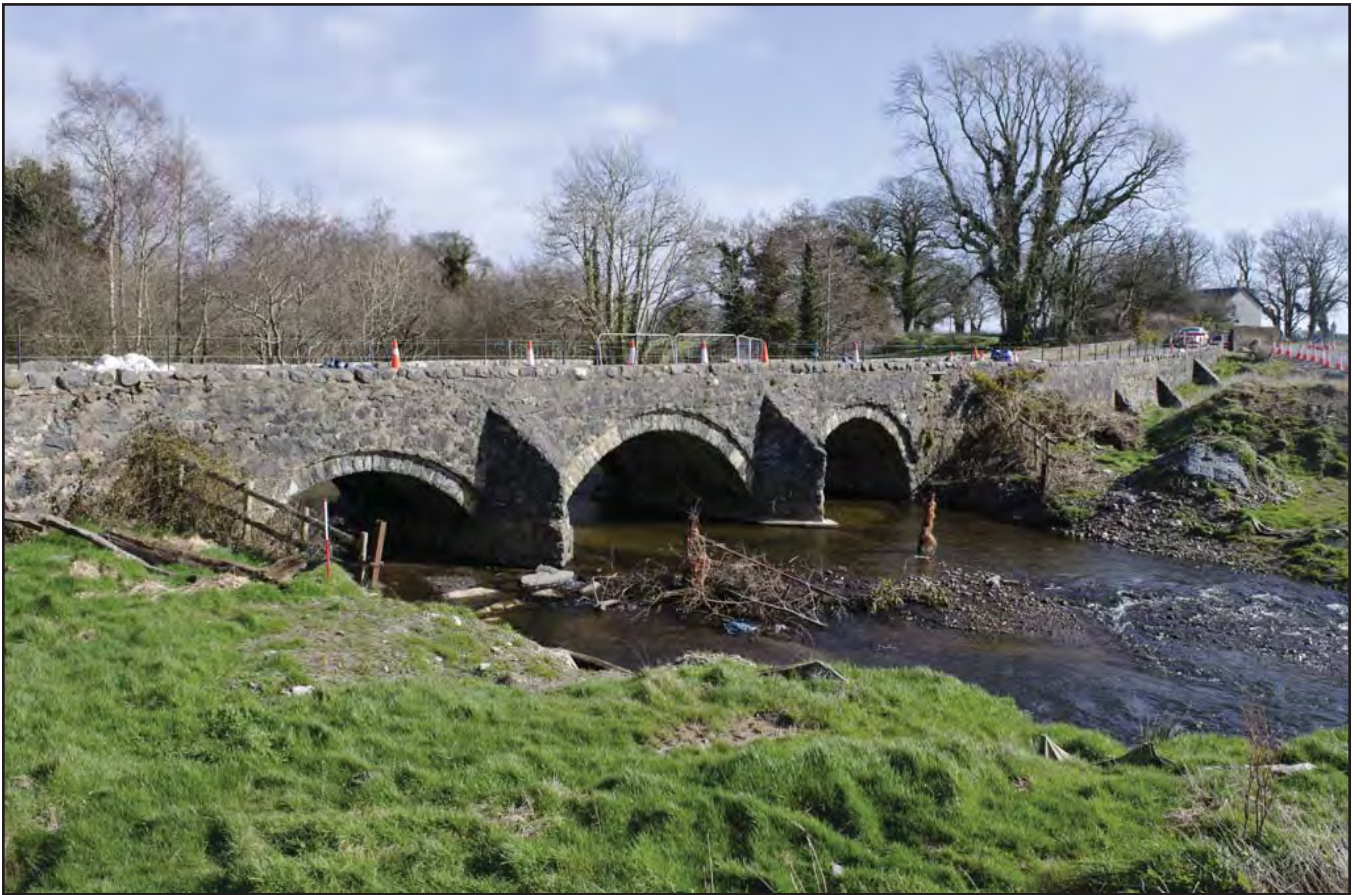
Plate 1: G2644_Pont_Bodfel; scale SW; view of south side of Pont Bodfel showing concrete repair to the base of SE bridge cutwater (archive reference: G2644_027).
