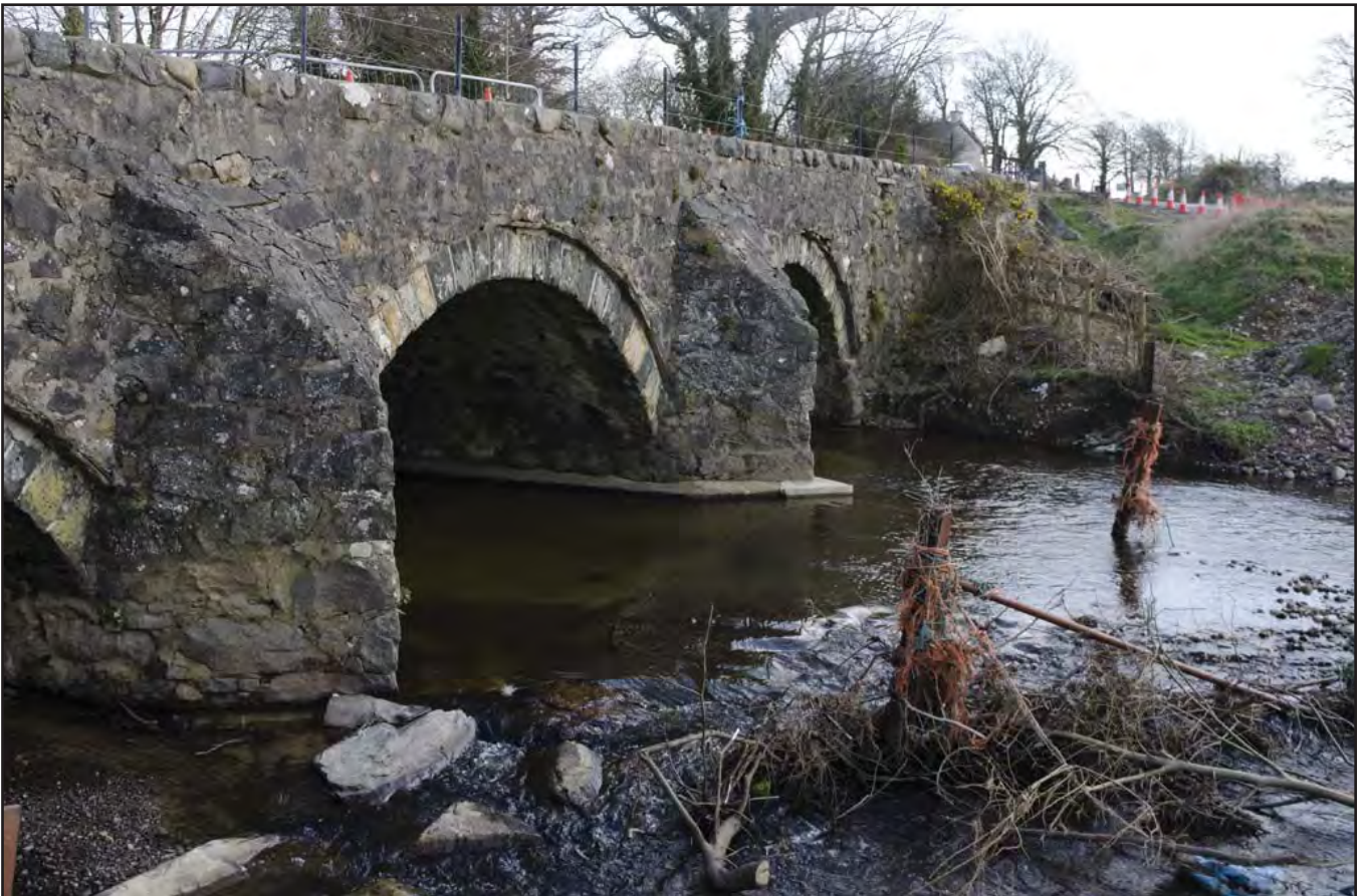
Plate 4: G2644_Pont_Bodfel; scale W; Angled view of bridge cutwaters on the south side, showing recent repair (archive reference: G2644_028).
