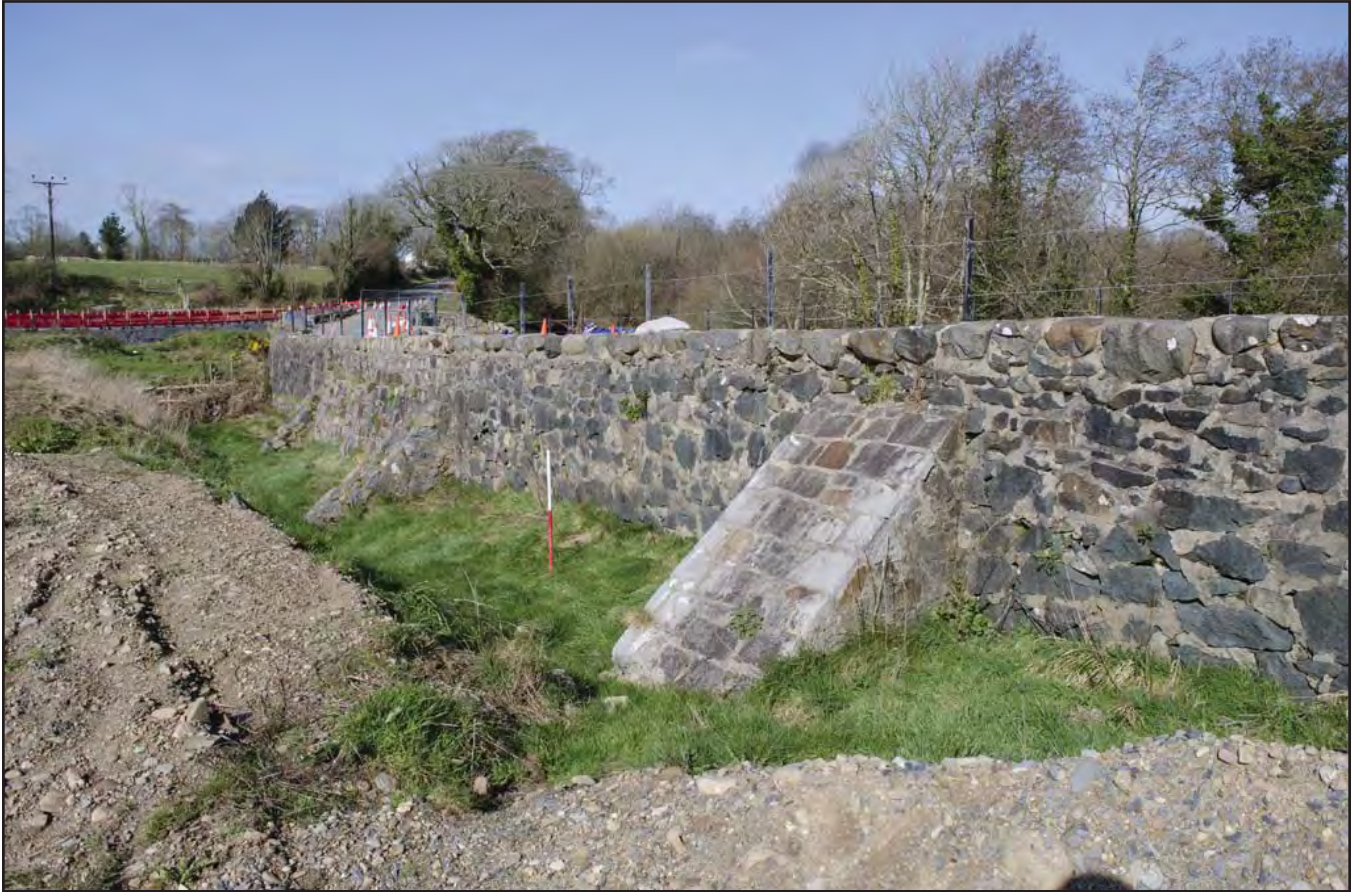
Plate 3: G2644_Pont_Bodfel; scale SE; view of modern buttressing on the south side of bridge approach (archive reference: G2644_025).
