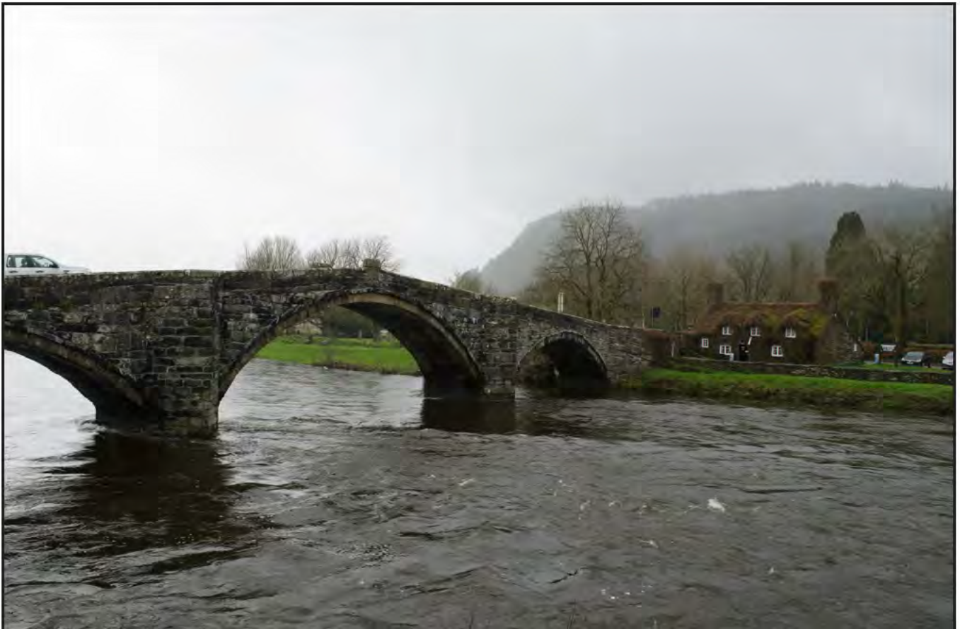
Plate 12: View toward toilet block and of Pont Fawr DE025 from the Wall to the North of Pont Fawr LB 3163, viewed from the north-northeast (Viewpoint 4; archive ref G2650_016).
