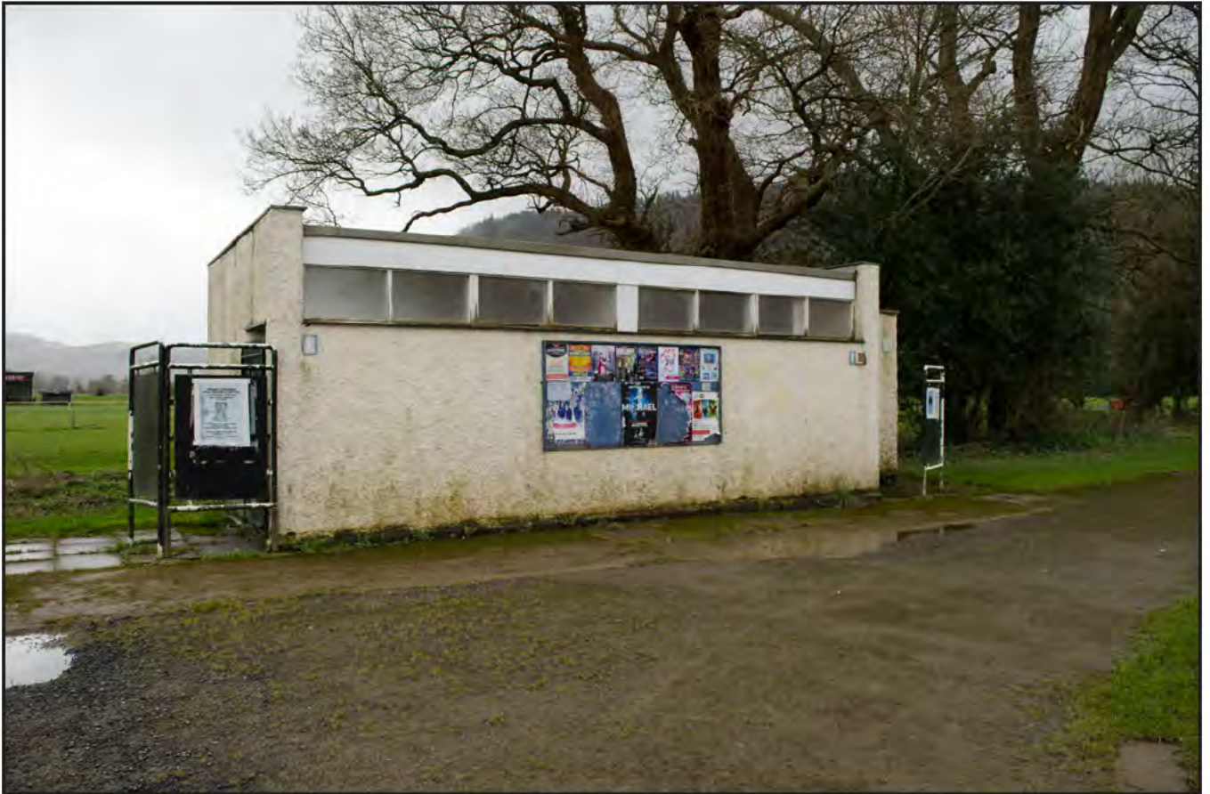
Plate 05: Current toilet block, viewed from the north (archive ref G2650_001).
