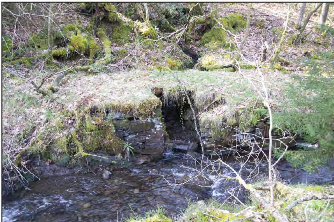
Plate 9: Tramway with culvert for stream; no scale; view from NE (archive reference: G2682_017).
