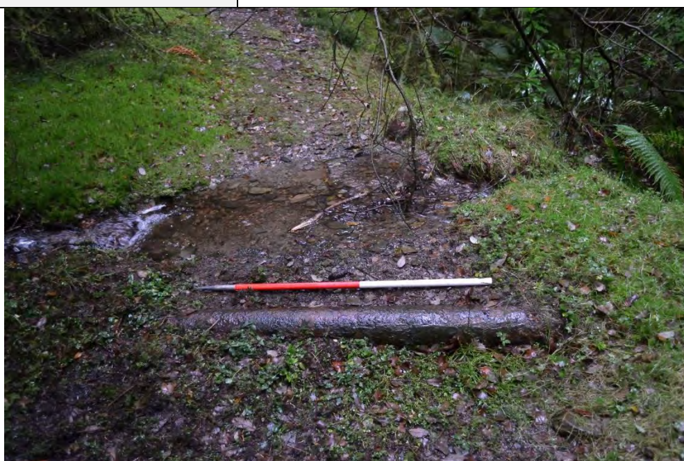
Cast iron water pipe crossing the forest track from SE (archive reference: G2754_0004)
