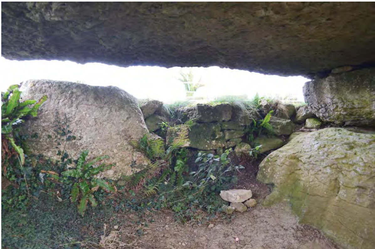
Plate 22. Inside the northern side of the chamber showing small blocks filling the gap (photo reference number G2767_068)
