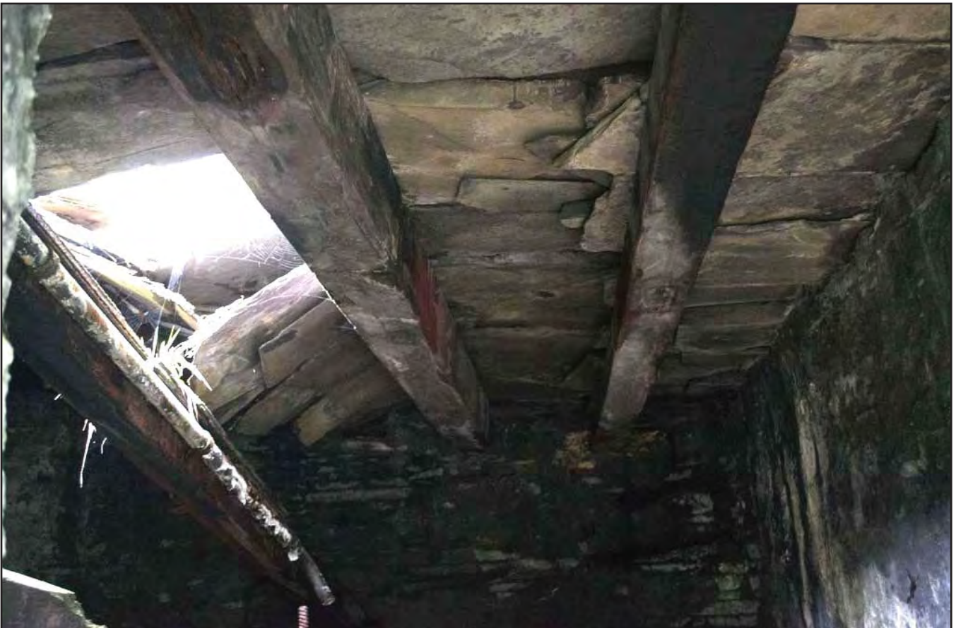
Plate 44: Vivian Quarry Utility Unit & Blast Shelter - View of collapsed roof above machinery in the utility unit; scale not used; view from S (archive reference: G2805_049).
