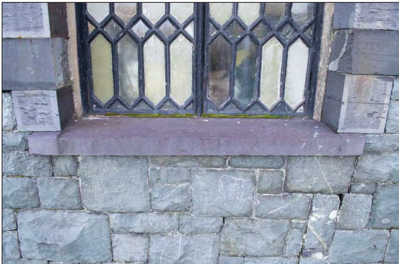
Plate 15: Fire Queen Locomotive Shed - Closeup of tooling on sill in eastern most window of southern lateral wall; scale not used; view from S (archive reference: G2805_015).
