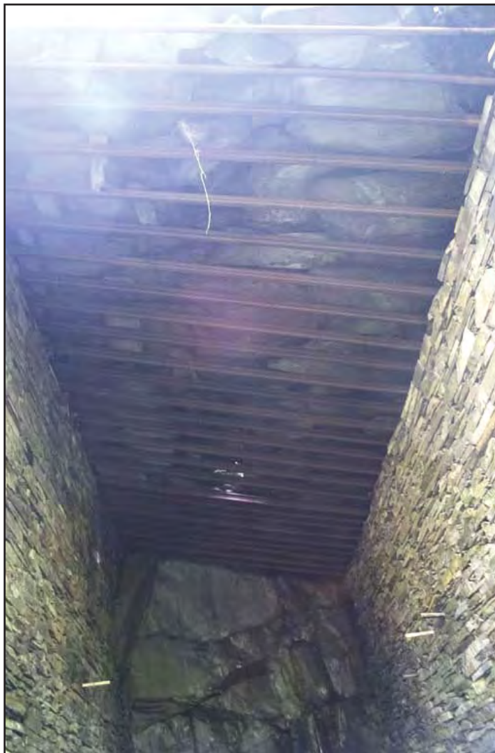
Plate 52: Vivian Quarry Storage Barn - Shot of roof from interior showing recycled rail tracks used as roof rafters; scale not used; view from NW (archive reference: G2805_046).
