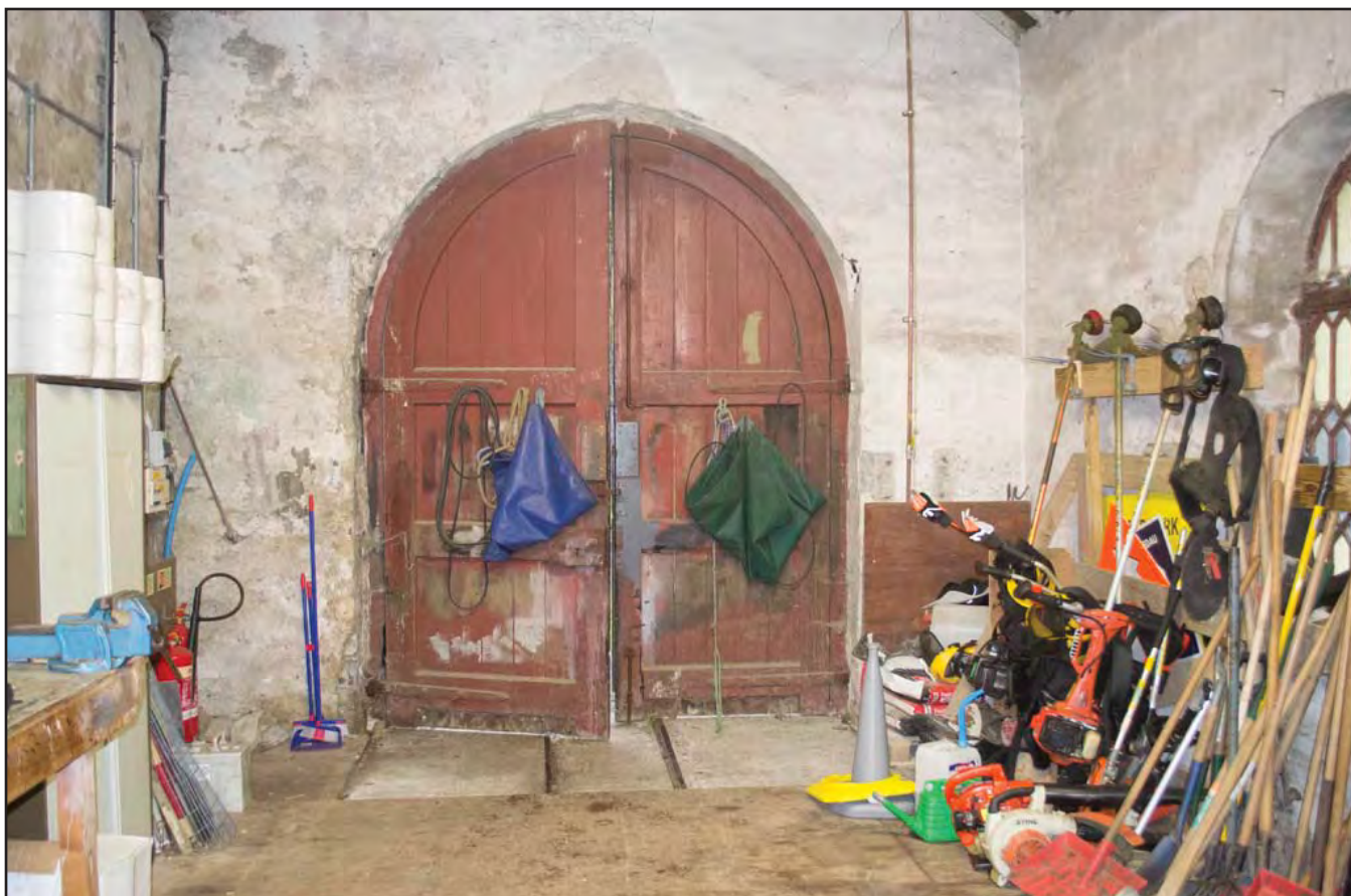
Plate 24: Fire Queen Locomotive Shed - View of inside of main doors to locomotive shed showing cut portions to allow doors to open fully; scale not used; view from W (archive reference: G2805_052).
