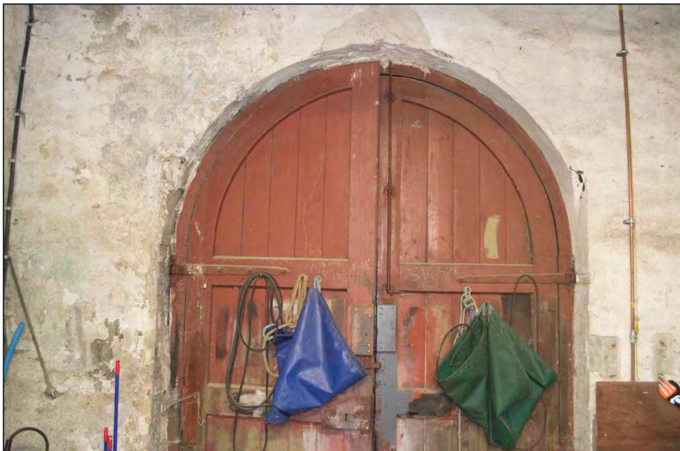
Plate 23: Fire Queen Locomotive Shed - View of inside of main doors to locomotive shed showing cut portions to allow doors to open fully; scale not used; view from W (archive reference: G2805_051).
