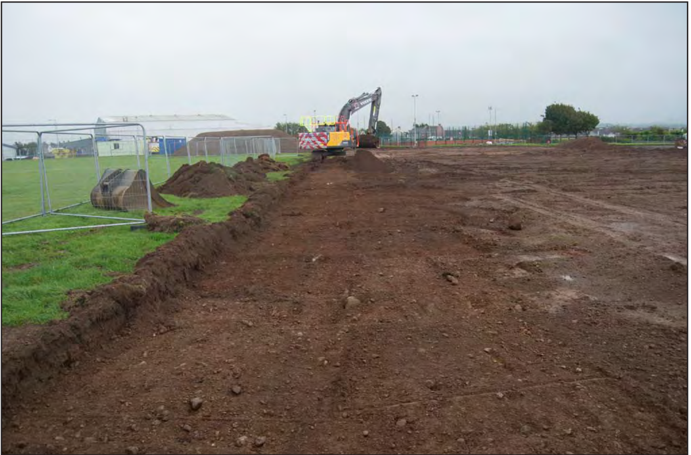
Plate 5: General view of topsoil and subsoil removal of strip of land next to playing field; scale not used; view from W (archive reference: G2780_59).
