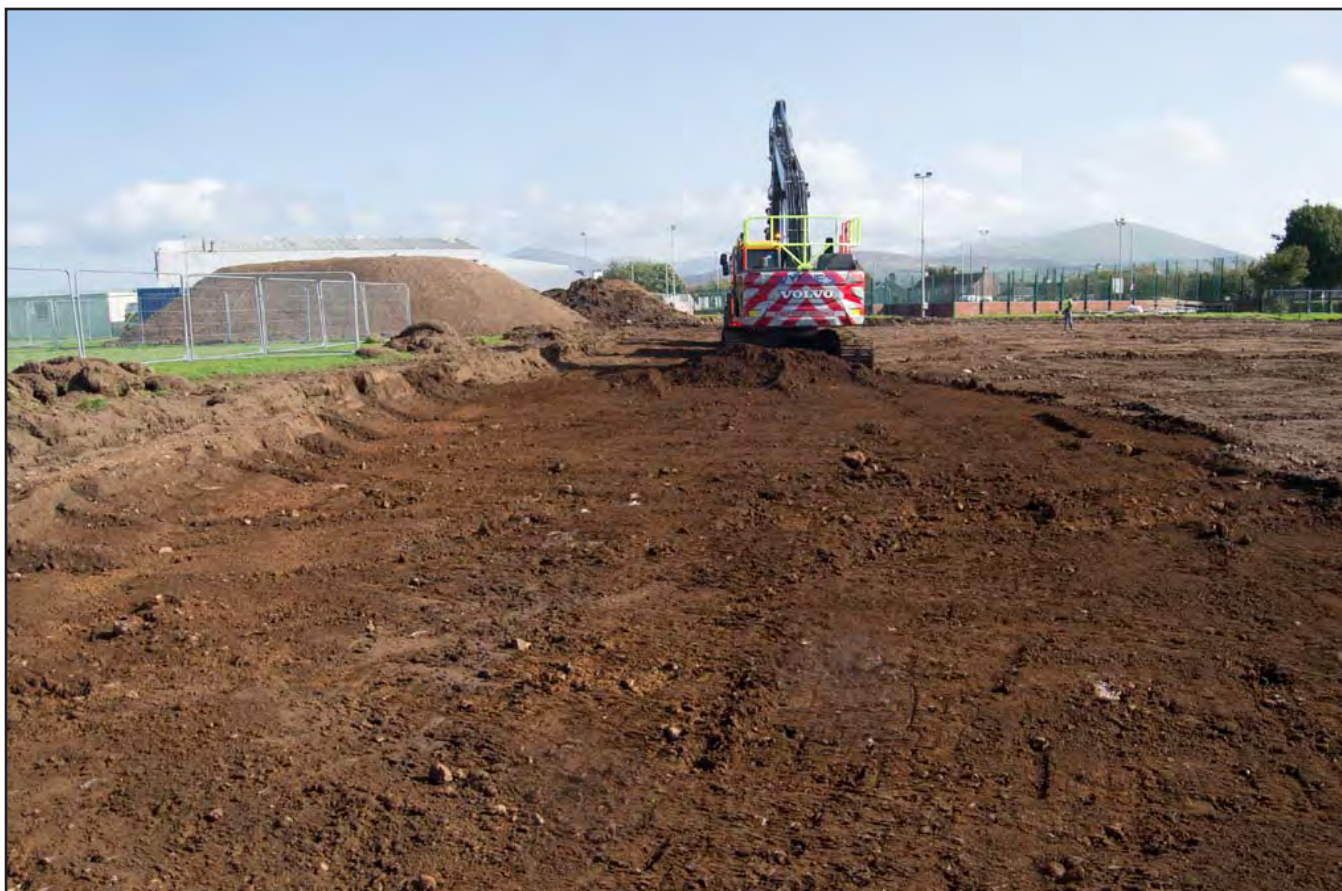
Plate 16: General view of de-turfing and removal of subsoil of strip of land next to playing field; scale not used; view from W (archive reference: G2780_63).
