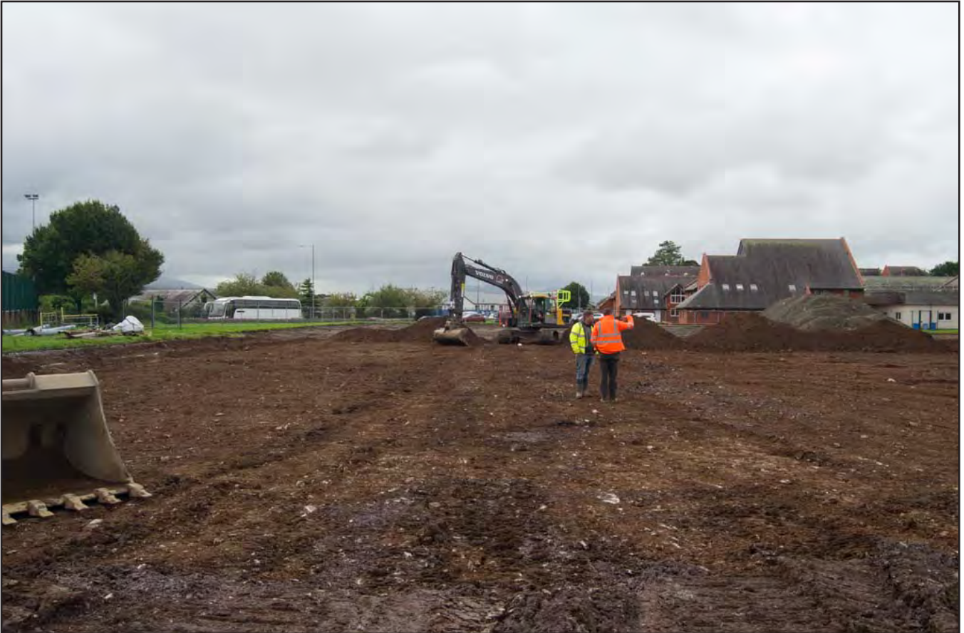
Plate 4: General view of area after removal of haul road and subsoil (102), showing gravel deposit (109); scale not used; view from NNE (archive reference: G2780_45).
