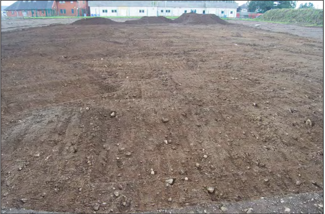
Plate 3: View of site at ESE end to required level; scale not used; view from ESE (archive reference: G2780_033).
