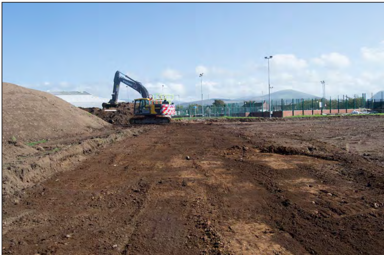
Plate 7: General view of removal of topsoil and subsoil of strip of land next to playing field; scale not used; view from W (archive reference: G2780_65).
