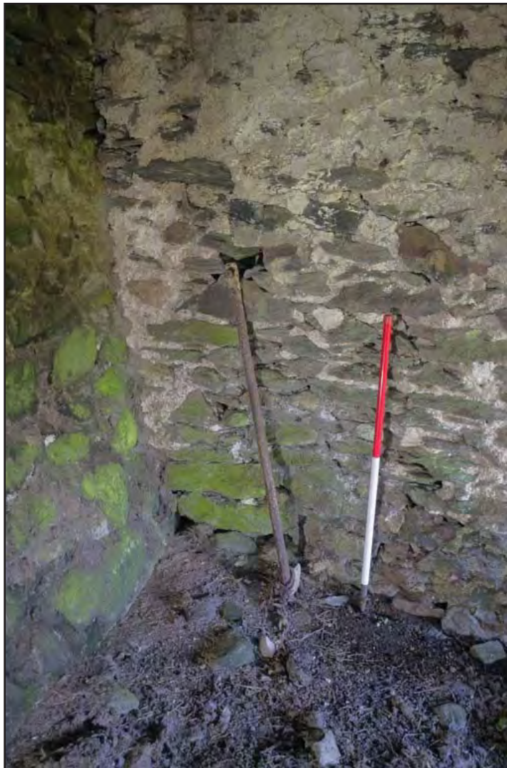
Plate 21: Room 2 interior - Close-up of bar in western wall. Note southern lateral wall to right is bulging at base; scale 1m; view from ENE (archive reference: G2807_016).
