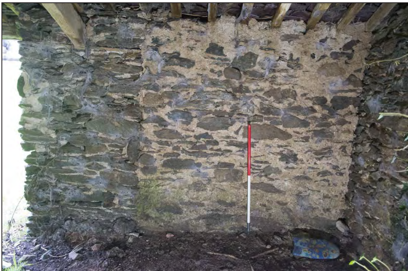
Plate 18: Room 1 interior - Shot of northern lateral wall showing separation in stonework up to northeast corner; scale not used; view from S (archive reference: G2807_012).
