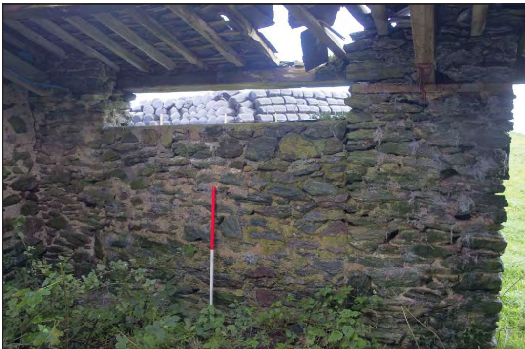
Plate 15: Room 1 interior - Shot of opening to west of northern lateral wall. Now partially filled in; scale 1m; view from SE (archive reference: G2807_009).
