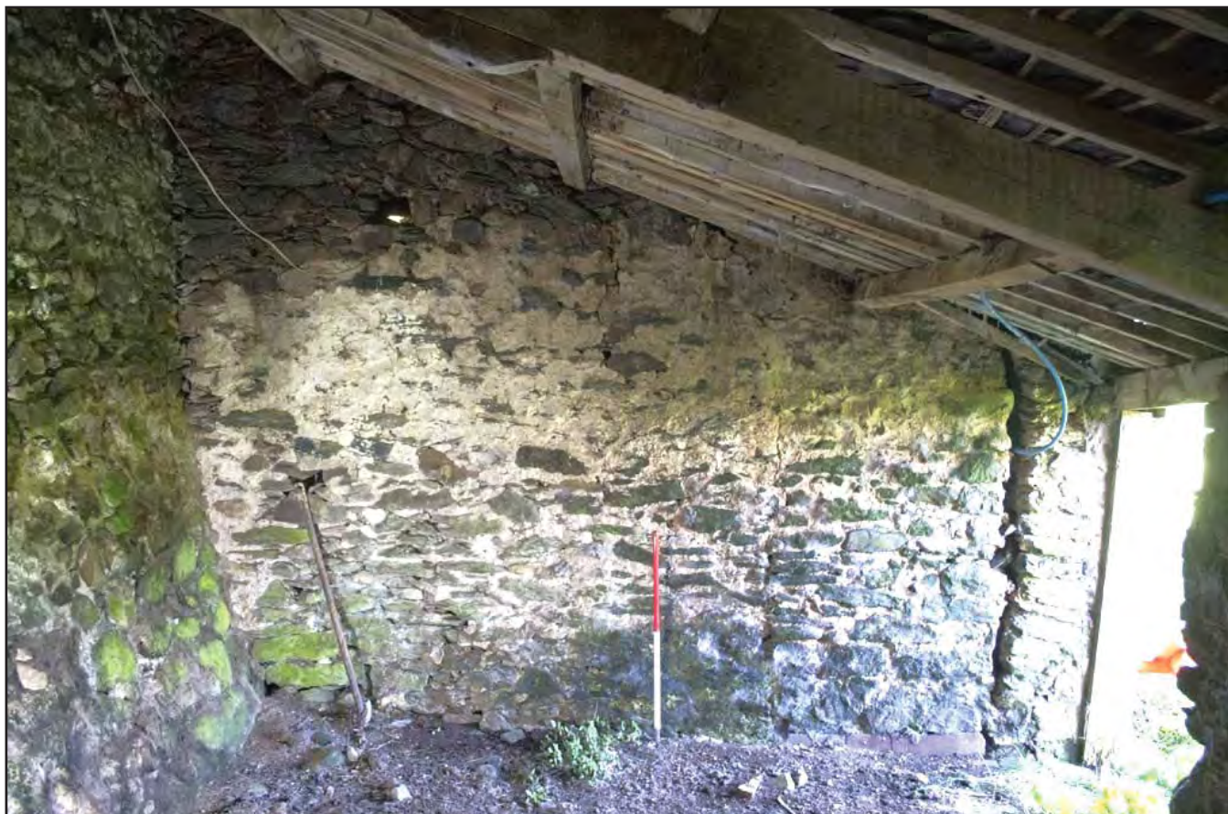
Plate 07: Room 1 interior - Shot of western gable end showing filled in doorway to right and metal bar and chain to left; scale 1m; view from E (archive reference: G2807_014).
