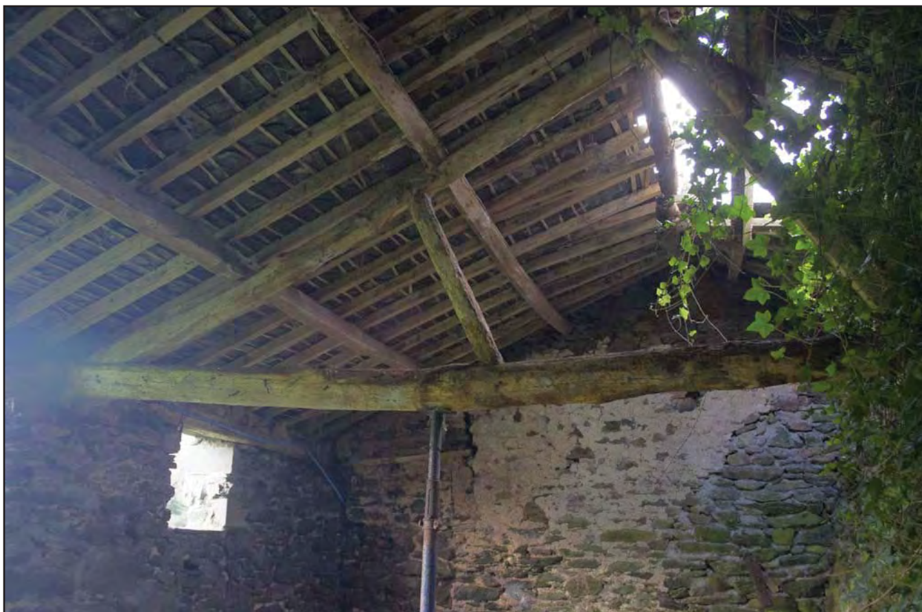
Plate 36: Room 3 interior - Close-up of rotten roof beams; scale not used; view from ESE (archive reference: G2807_031).
