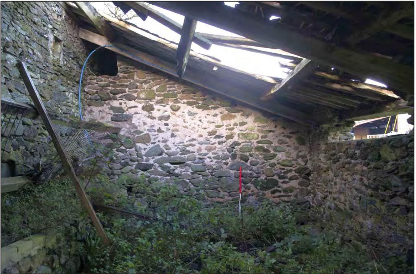
Plate 09: Room 1 interior - Western gable end. Shot of interior showing troughs to left & collapsed roof; scale 1m; view from E (archive reference: G2807_003).
