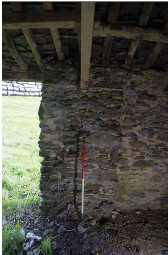
Plate 14: Room 1 interior - Shot of eastern side of doorway in northern lateral wall showing stonework narrowing of entrance (portrait shot); scale 1m; view from S (archive reference: G2807_008).
