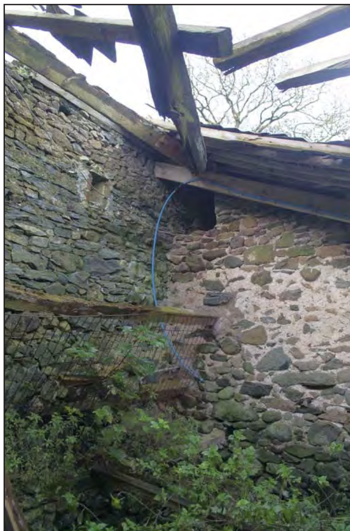
Plate 16: Room 1 interior - Portrait shot showing hole in top of southwest corner of western gable interior. Also shows trough and roof collapse; scale 1m; view from NE (archive reference: G2807_010).
