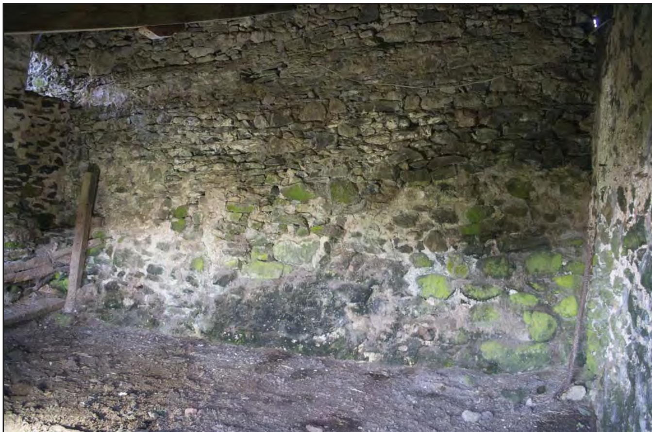
Plate 25: Room 2 interior - Shot of southern wall showing large stones bulging at base with smaller masonry above; scale not used; view from NNE (archive reference: G2807_020).
