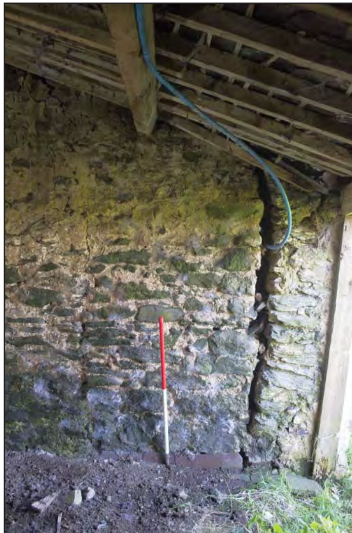
Plate 20: Room 2 interior - Close-up portrait of filled in doorway with crack in it with cable going through western gable; scale 1m; view from E (archive reference: G2807_015).
