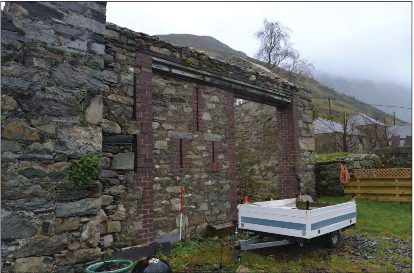
Plate 9: Room 3 - shot of composite construction material in large entrance to Room 3; scale 1m; view from N (archive reference: G2809_009).
