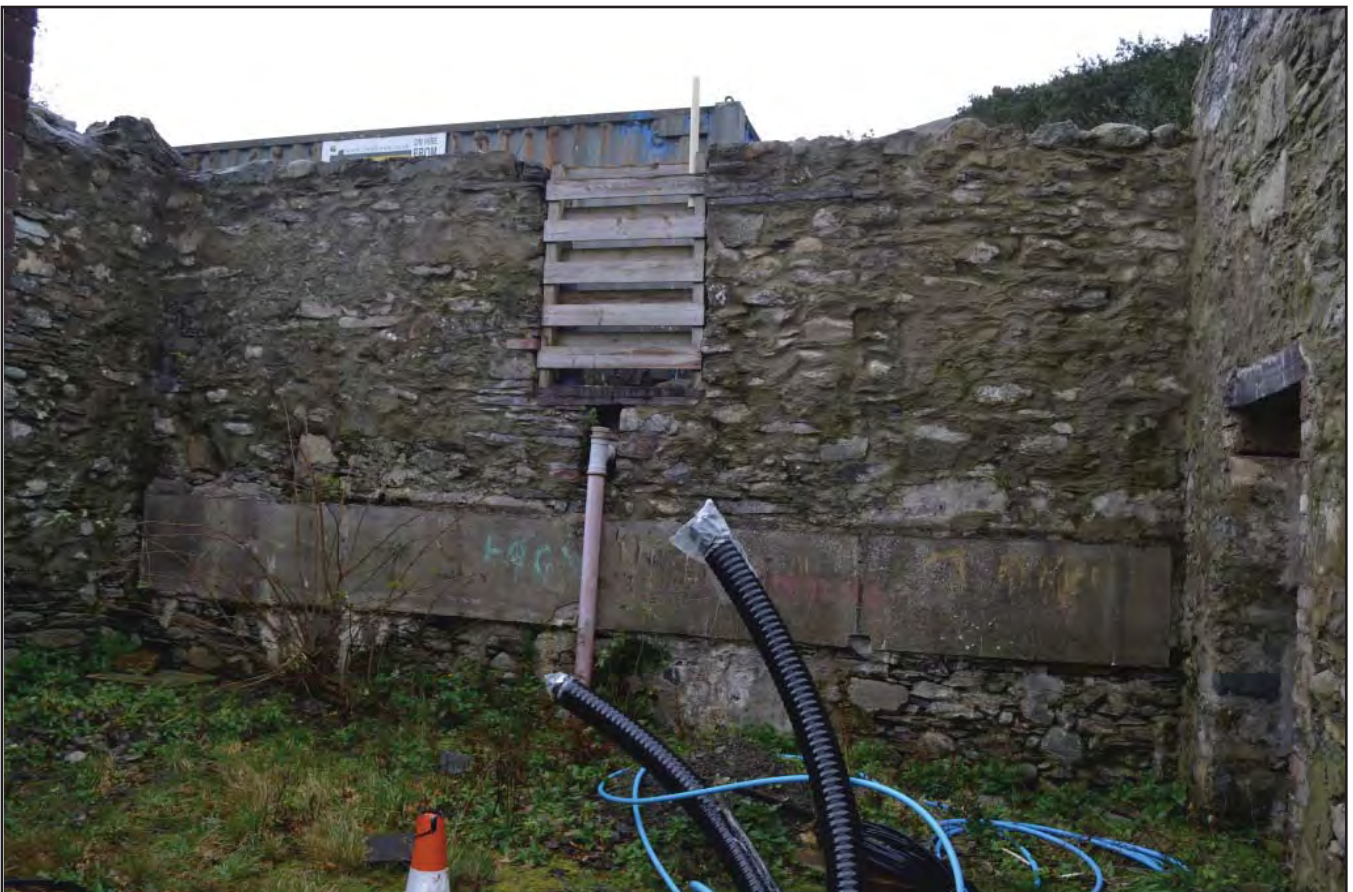
Plate 22: Room 3 - Northeastern interior wall showing concrete backing and modern plastic water pipe (possible drainage); scale none; view from SW (archive reference: G2809_022).
