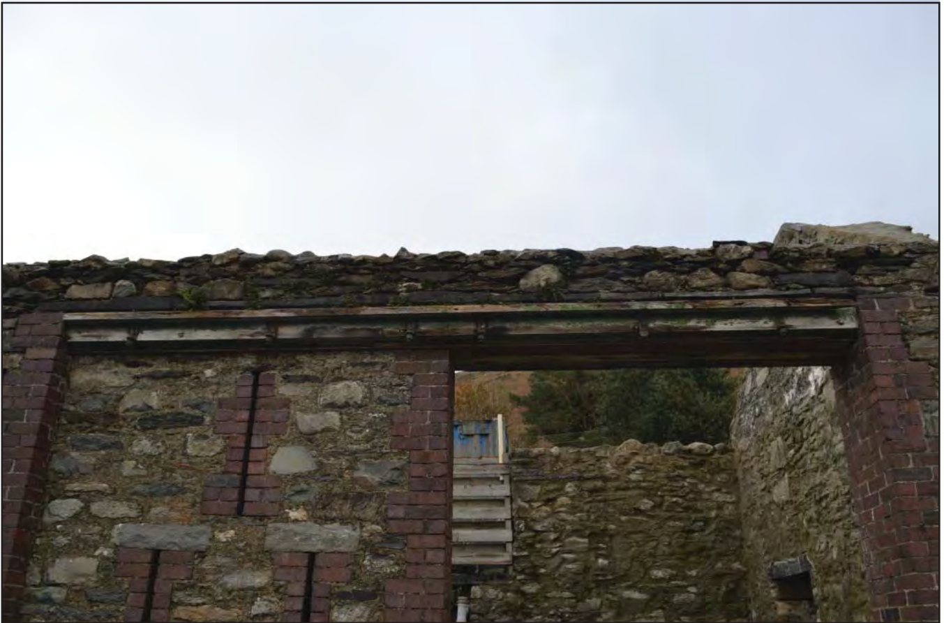
Plate 19: Room 3 - Shot showing original wooden fittings above large entrance to Room 3 with metal rollers for sliding doors; scale none; view from SW (archive reference: G2809_019).
