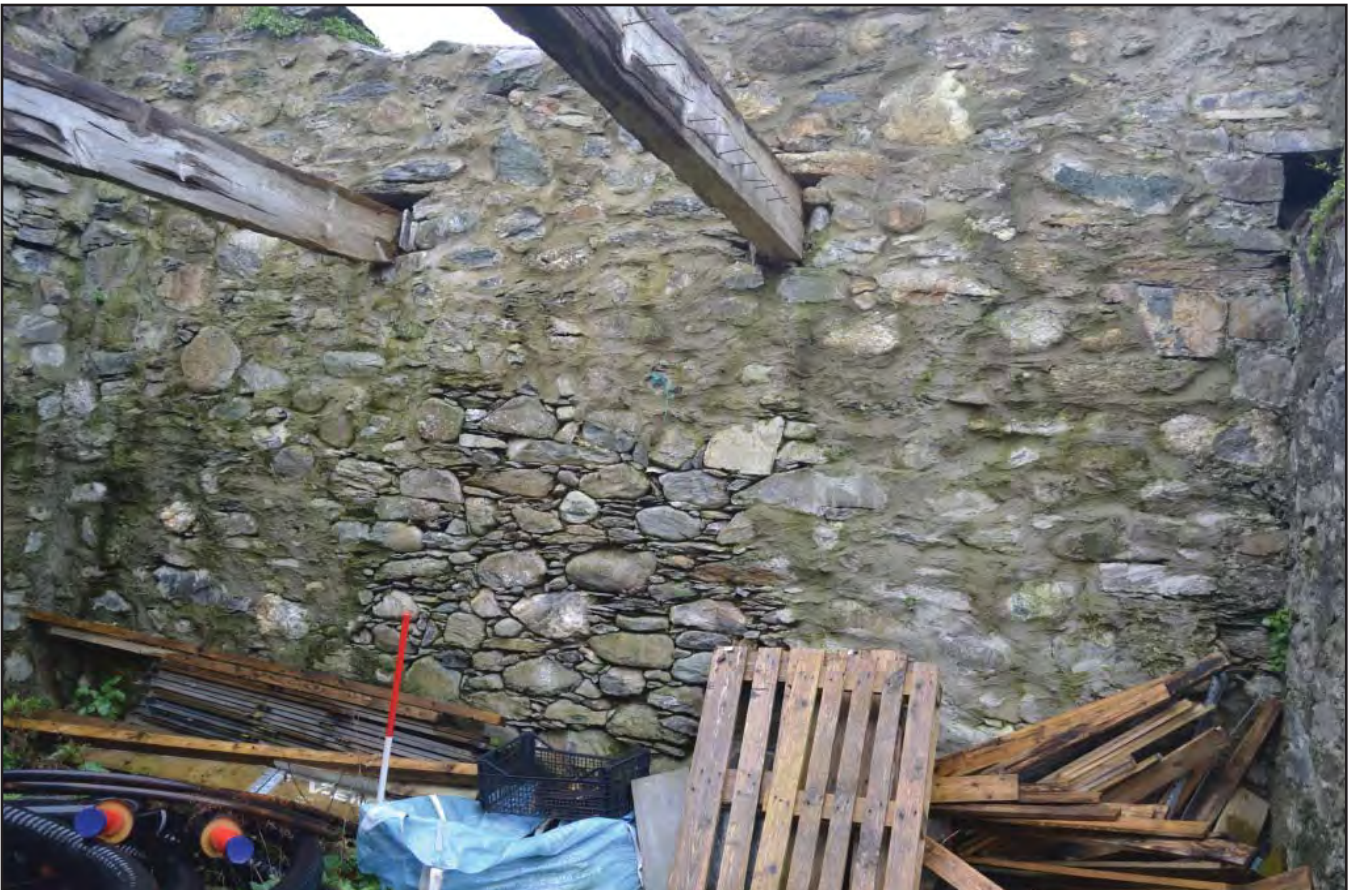
Plate 8: Room 2 - Shot of interior of Room 2 showing possible filled in access to Room 3; scale 1m; view from N (archive reference: G2809_008).
