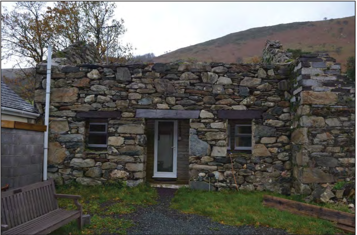
Plate 21: Room 1 - Shot of room 1 showing slate windowsill and stone construction; scale none; view from SW (archive reference: G2809_021).
