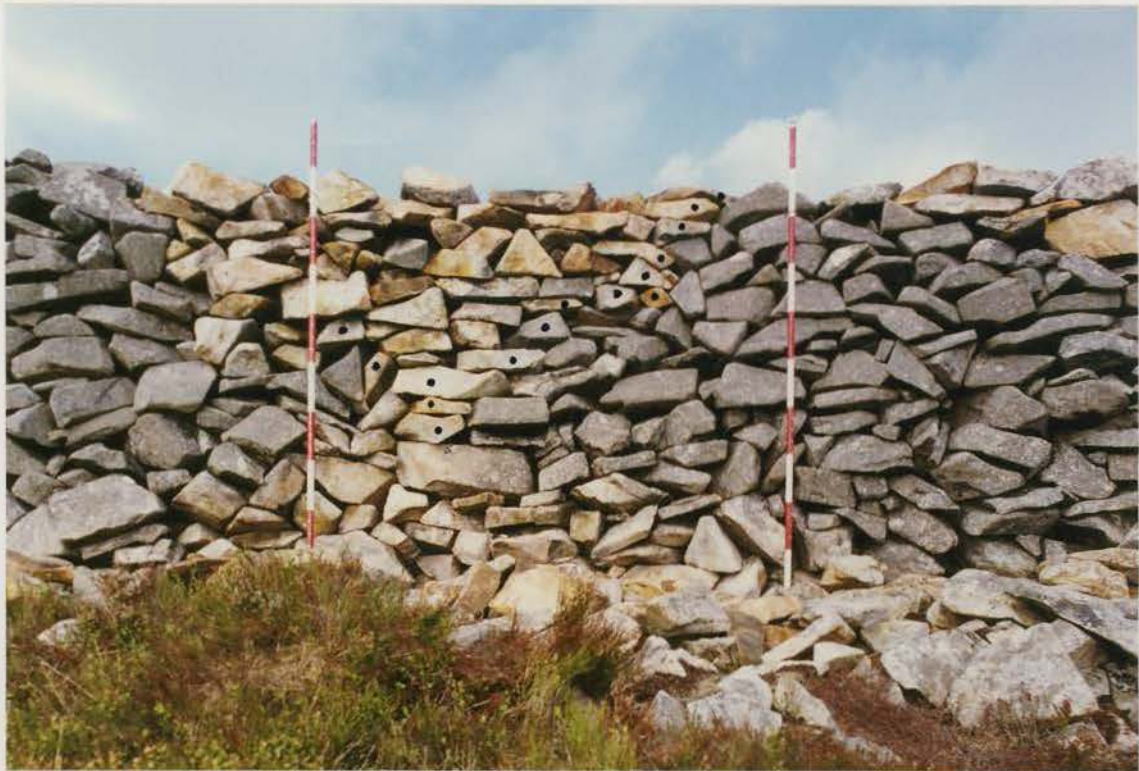
Plate 59 G1022/209/13 ; Collapse V1 after conservation.
