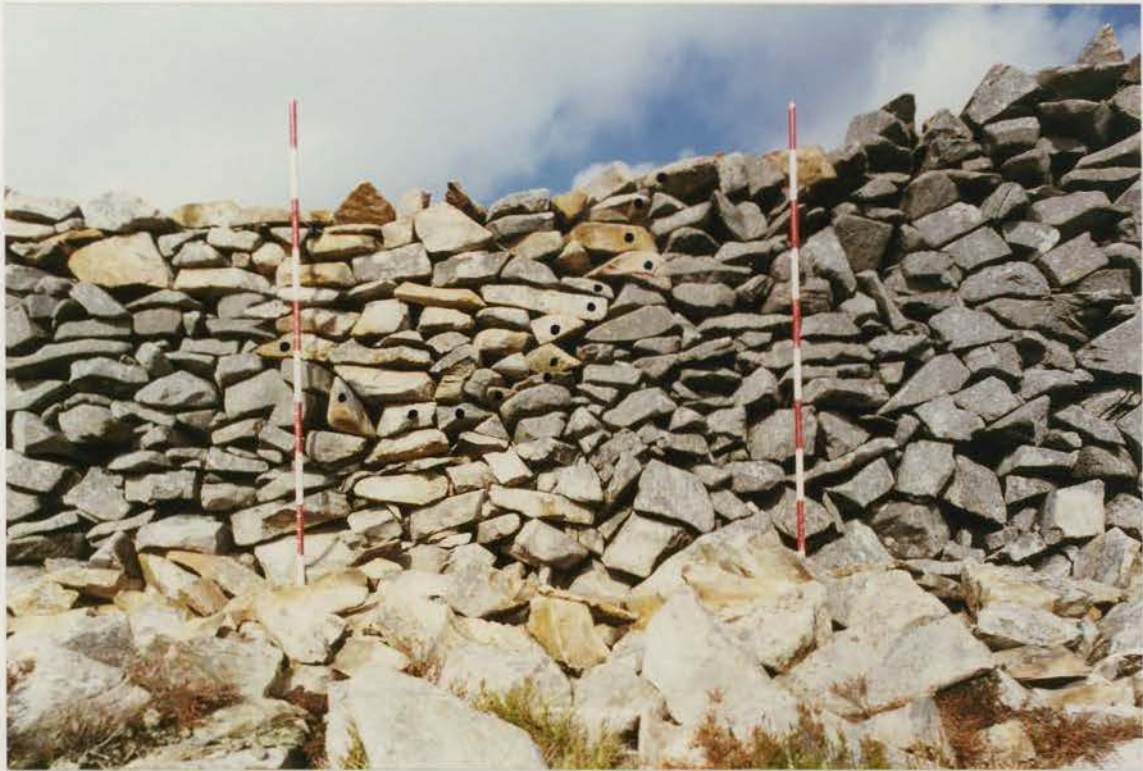
Plate 55 G1022/209/09 ; Collapse V after conservation.
