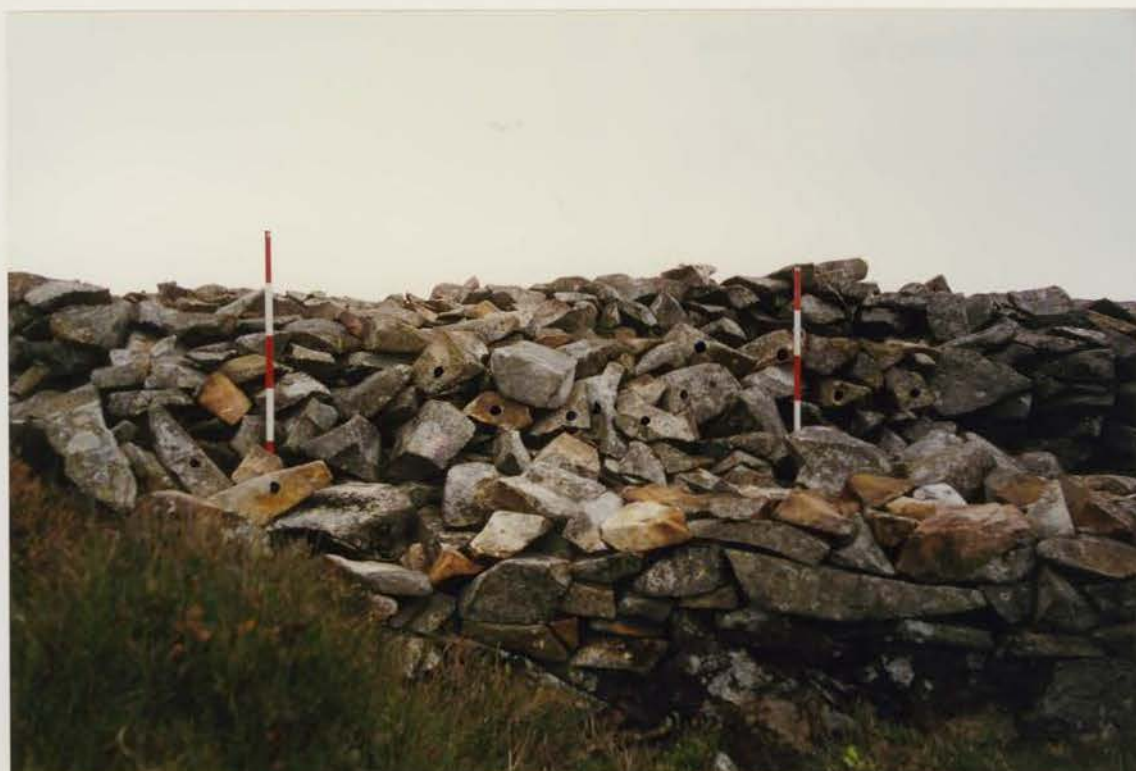
Plate 116 G1022/209/31 ; Collapse V5 after conservation.
