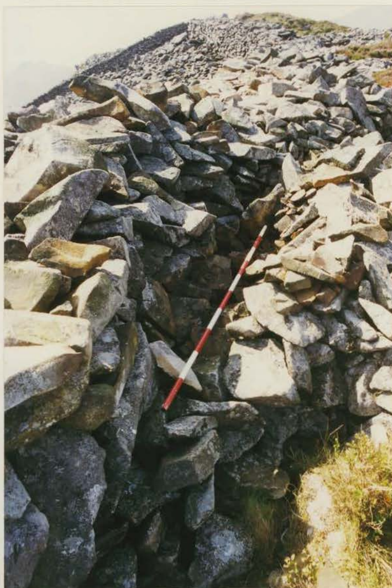
Plate 108 G1022/206/08; Collapse V4, eastern end, after clearance.
