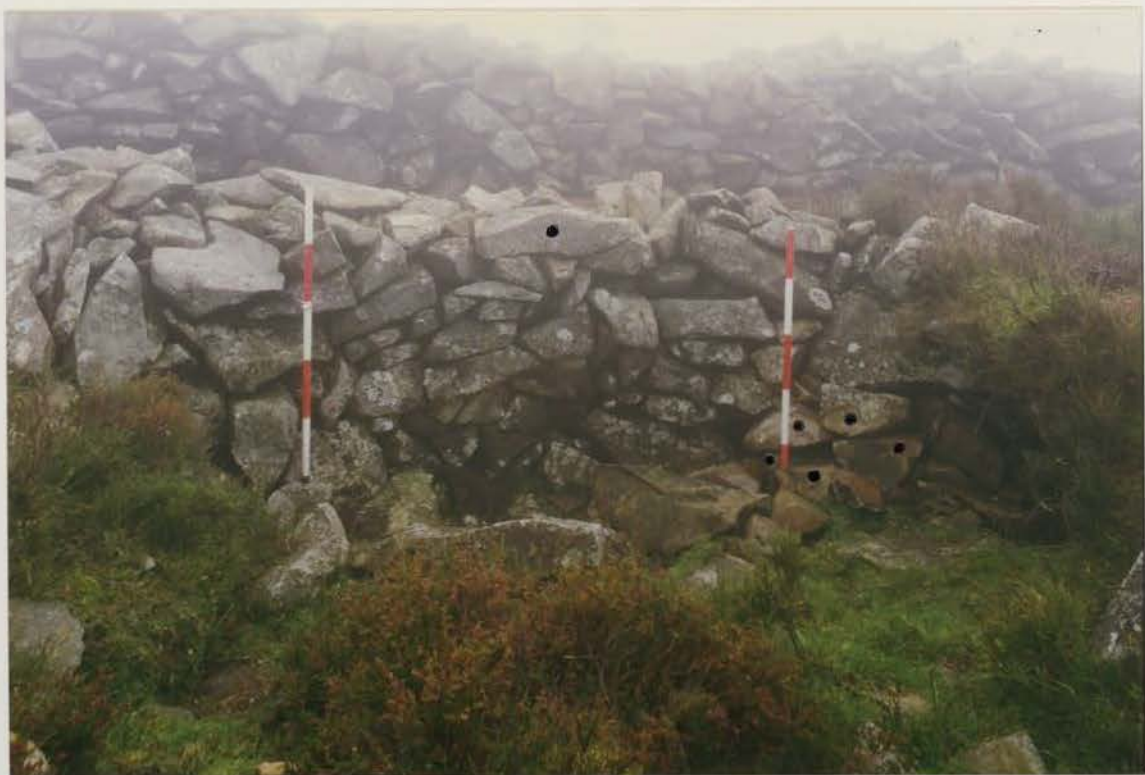
Plate 168 G1022/212/15 ; Collapses 107a and 107d after conservation.
