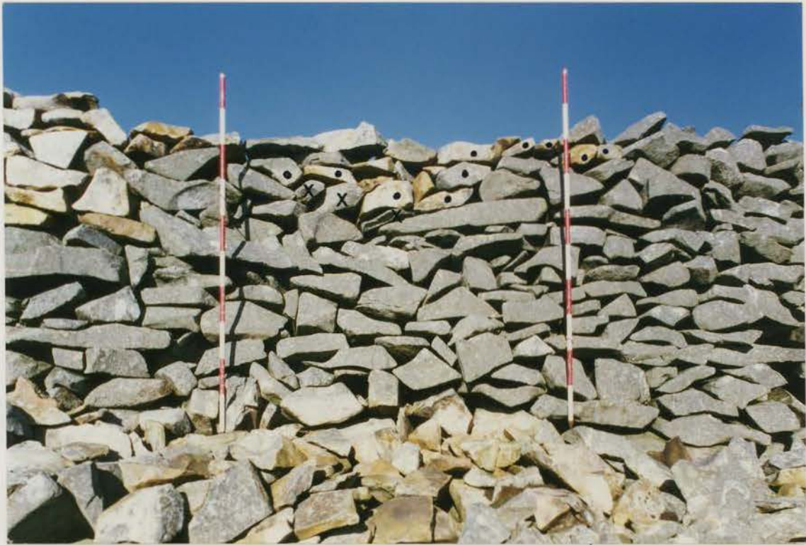
Plate 79 G1022/211/07 ; Collapse W2 after conservation.
