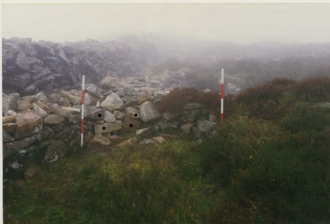
Plate 166 G1022/212/11 ; Collapse 108a after conservation.
