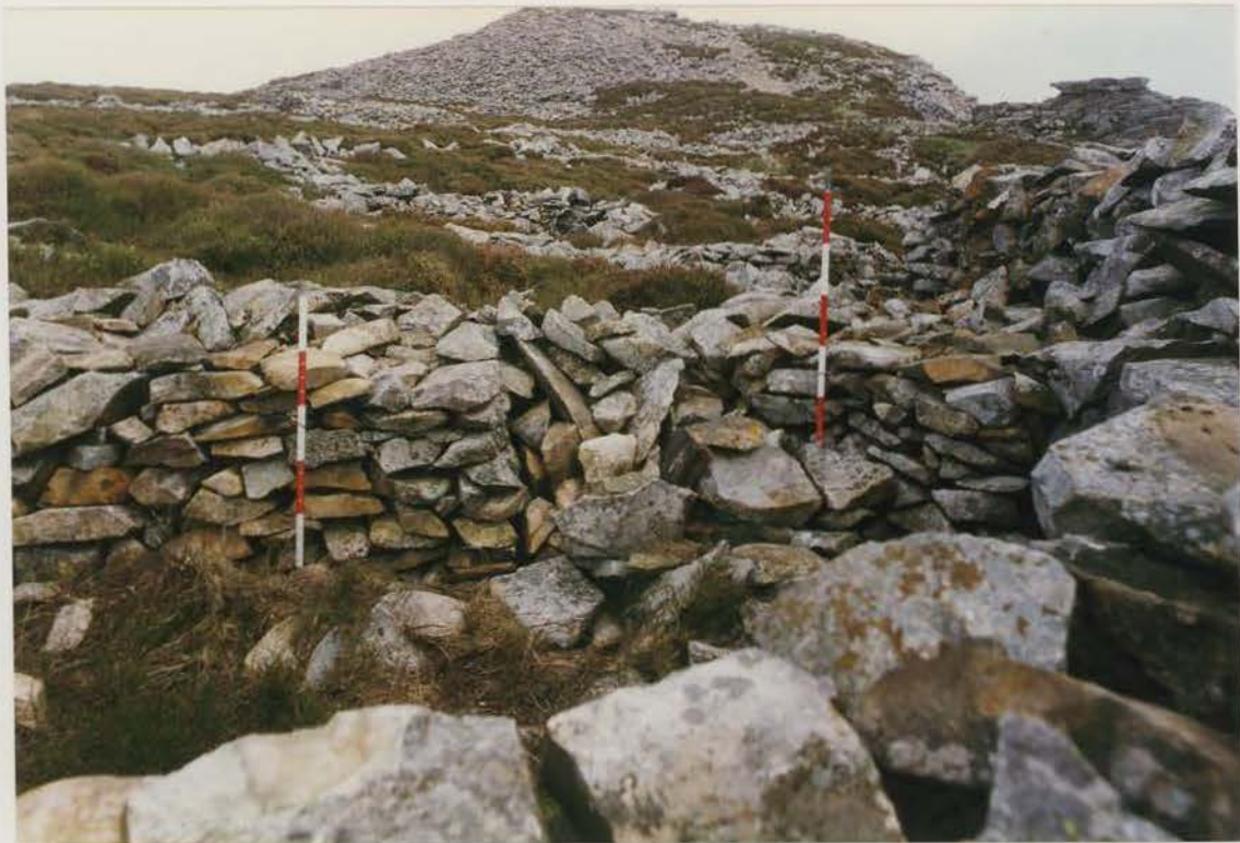
Plate 190 G1022/208/01 ; Collapses 41a and 41b after conservation.
