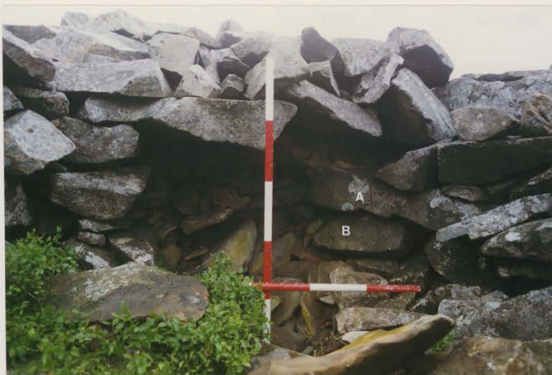
Plate 229 G1022/204/01 ; Collapse 10c after clearance.
