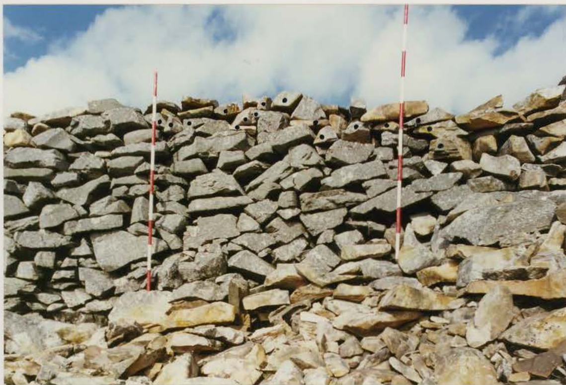
Plate 48 G1022/209/03 ; Collapse U1 after conservation.
