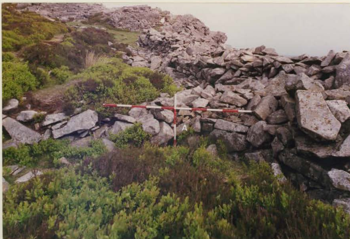
Plate 156 G1022/199/07; Collapse 45Ad before conservation.
