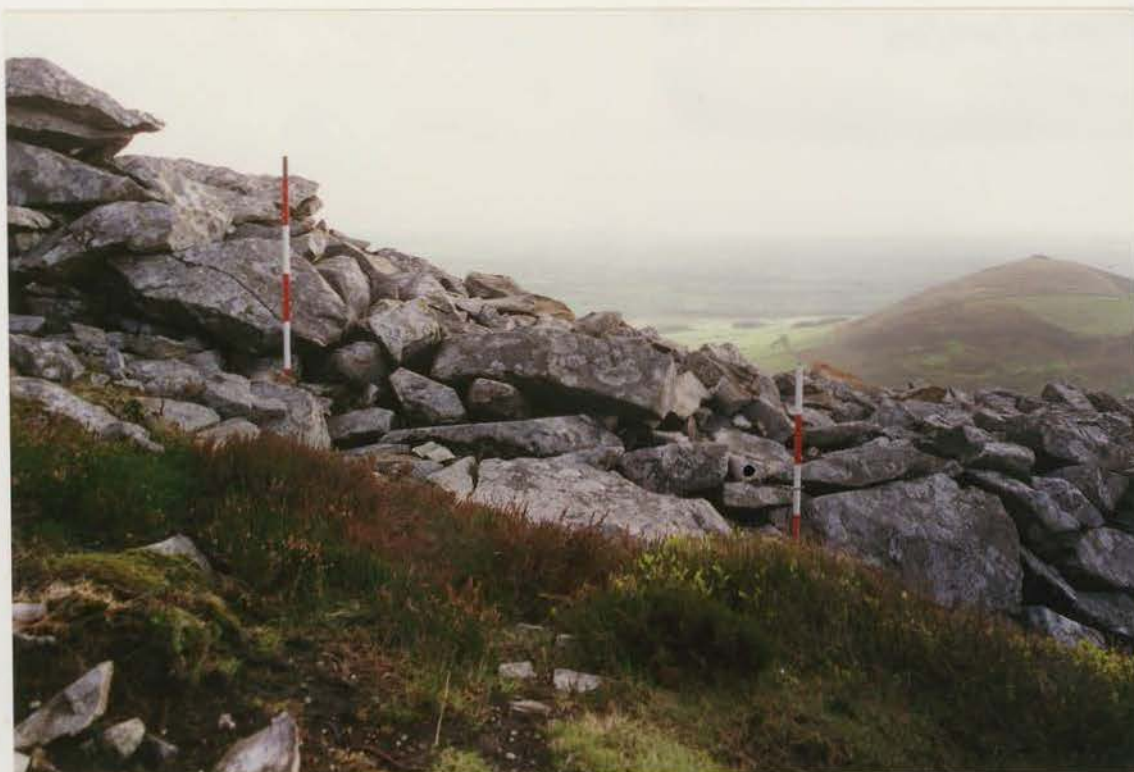
Plate 25 G1022/208/04 ; Collapse S9 after conservation.
