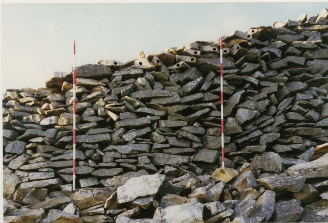
Plate 18 G1022/212/07 ; Collapse S5 after conservation.
