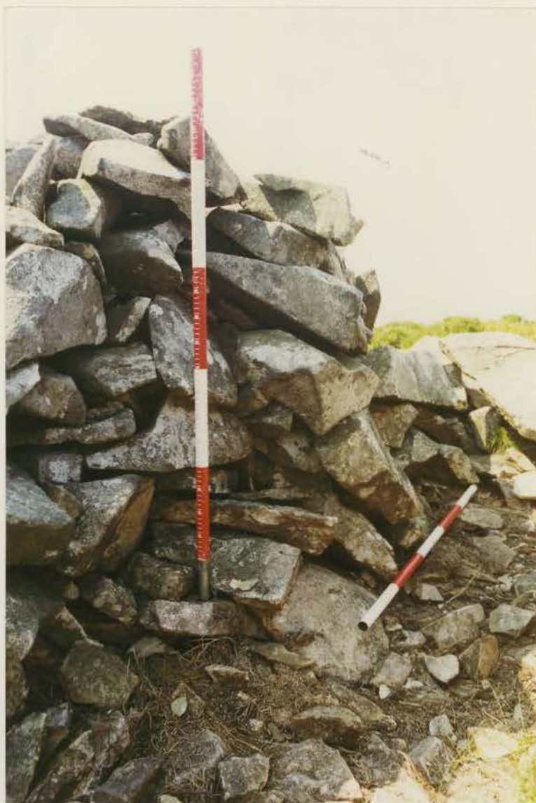
Plate 218 G1022/203/22; Collapse 9d before conservation.
