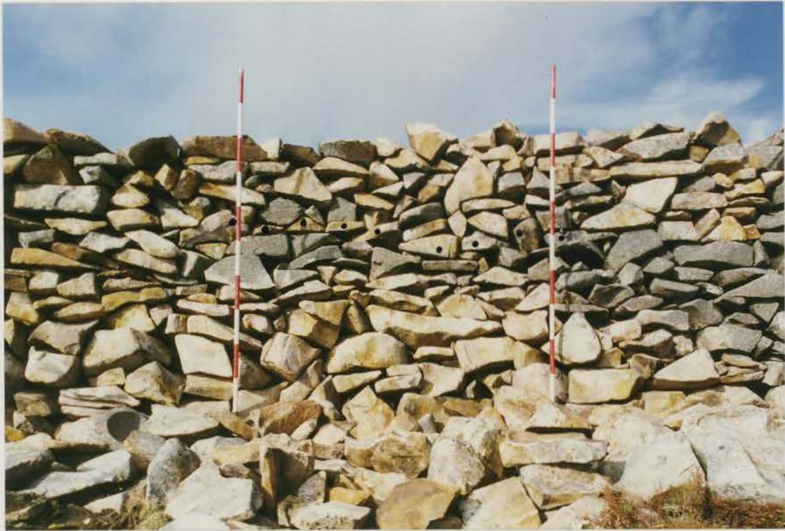
Plate 67 G1022/209/20; Collapse V2 after conservation.
