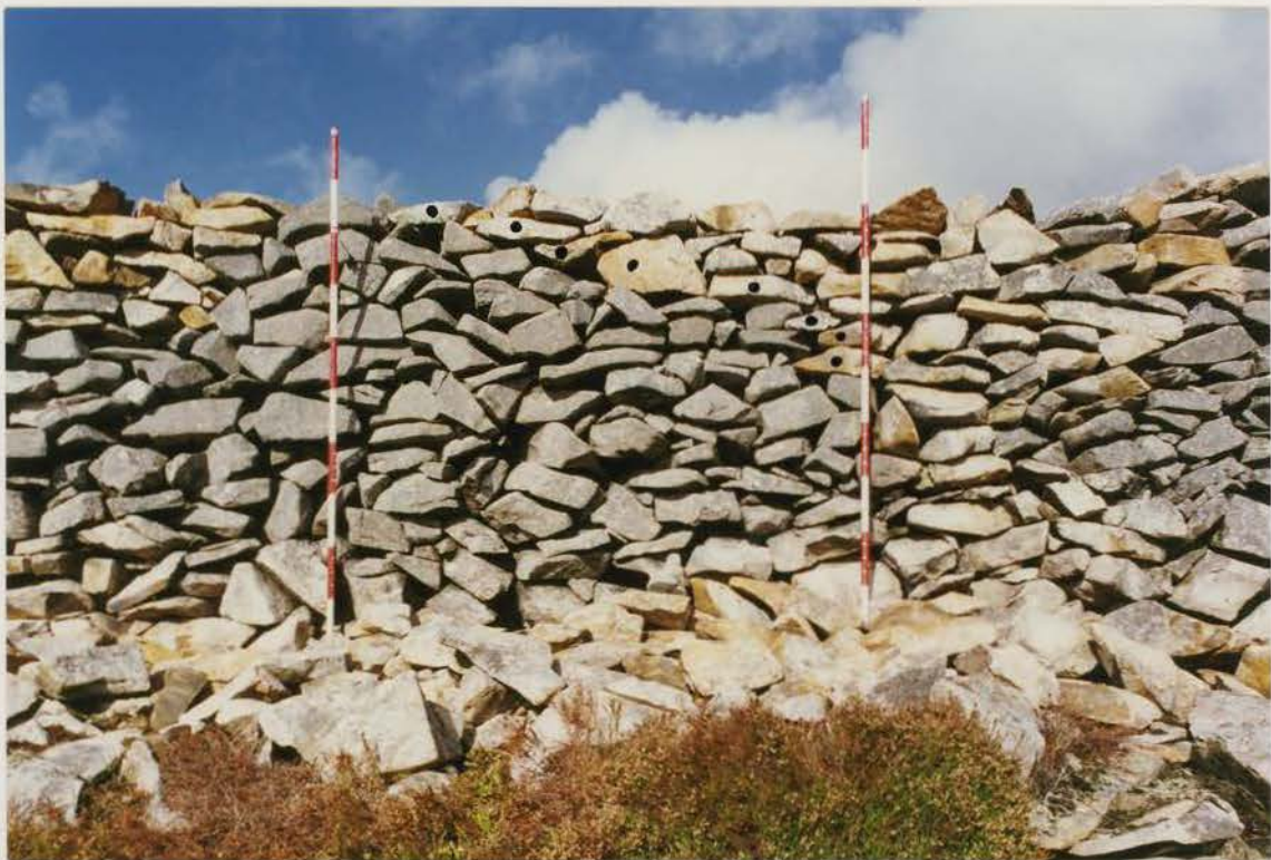
Plate 56 G1022/209/11 ; Collapse V after conservation.
