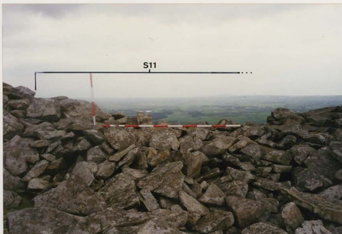
Plate 30 G1022/194/24 ; Collapse S11 before conservation.
