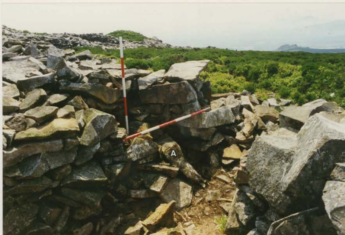
Plate 219 G1022/203/26 ; Collapse 9d after clearance.
