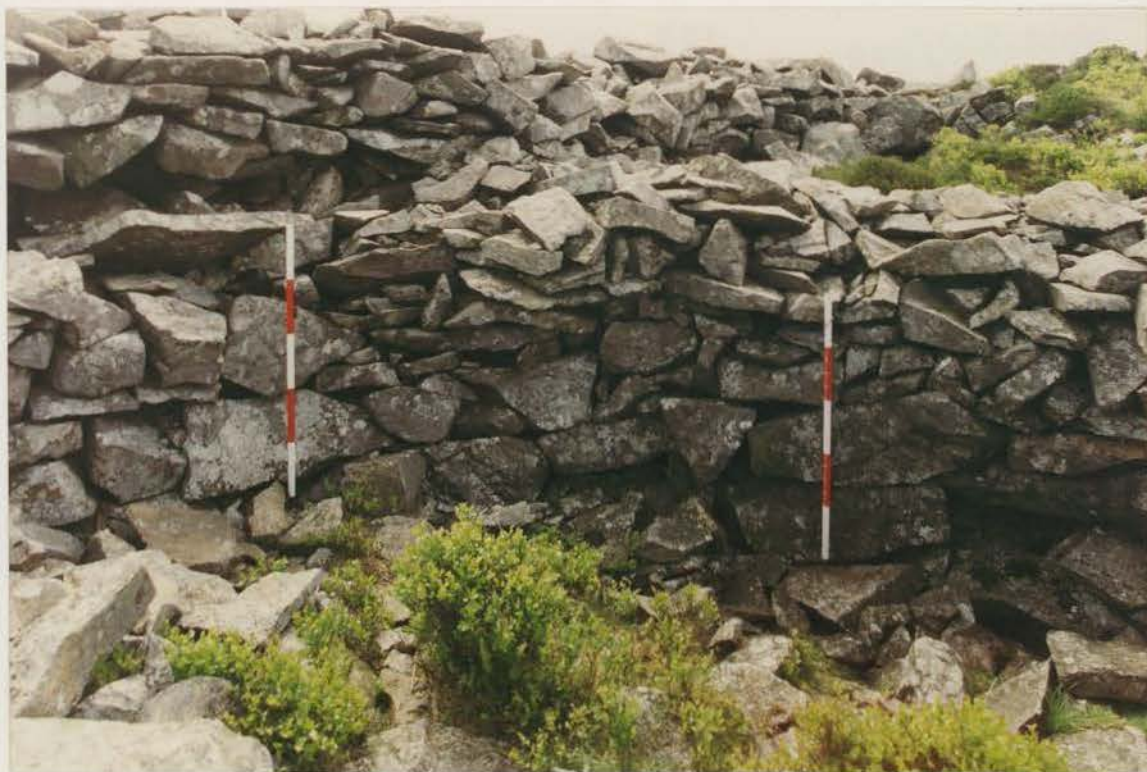
Plate 193 G1022/200/22a; Collapse 41c (NW.) before conservation.
