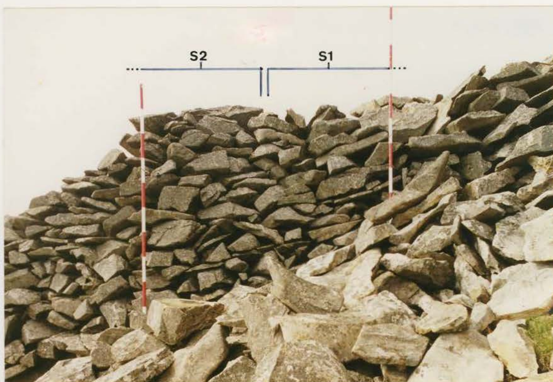
Plate 4 G1022/193/18 ; Collapse S1 before conservation.
