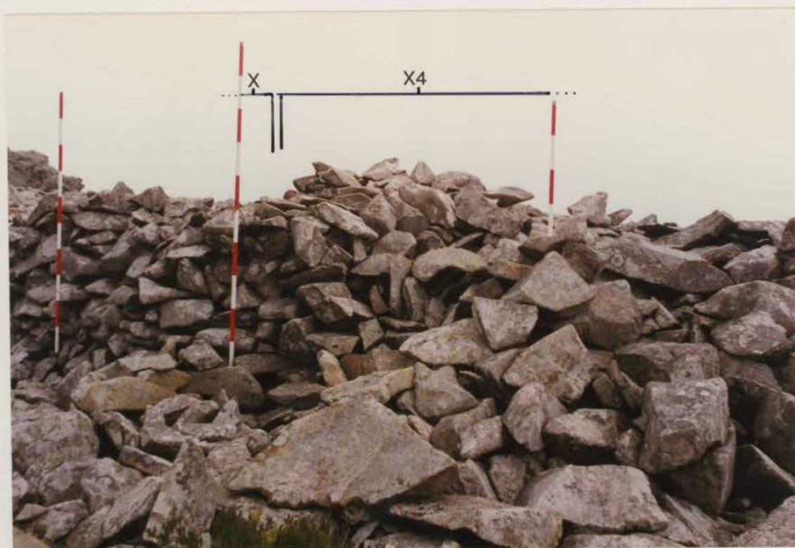
Plate 134 G1022/196/18 ; Collapse X4 before conservation.
