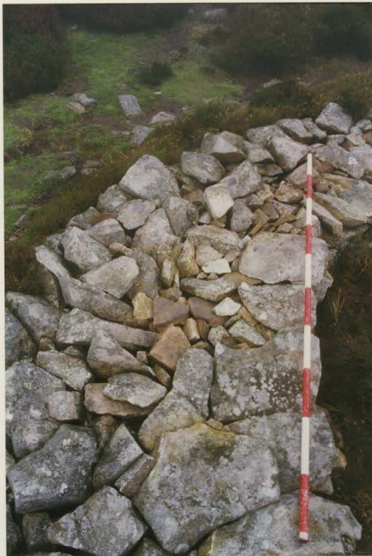
Plate 155 G1022/212/30; Collapse 45Aa, wall top, after conservation.
