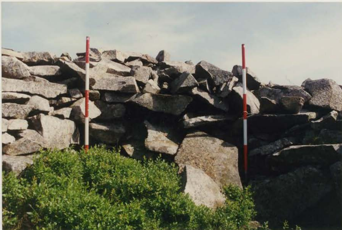
Plate 228 G1022/201/28 ; Collapse 10c before conservation.
