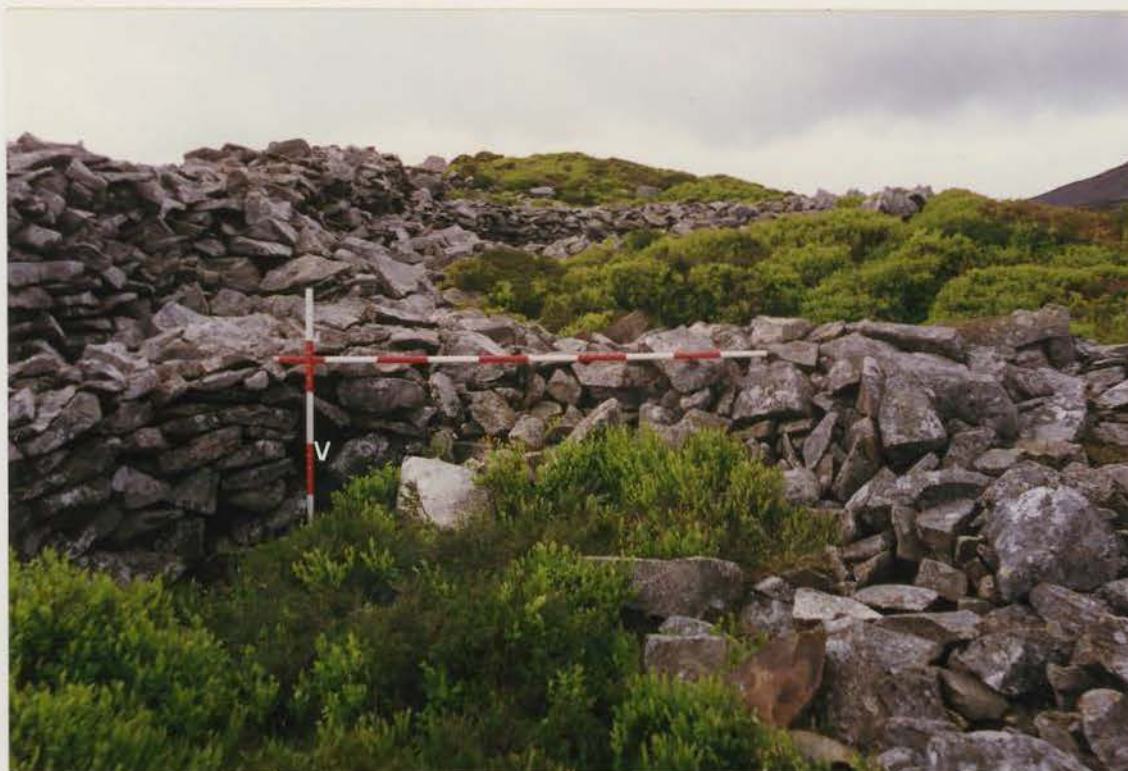
Plate 183 G1022/199/34 ; Collapses 42a and 42b before conservation.
