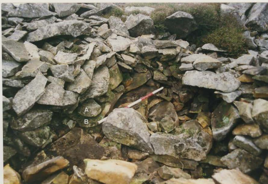
Plate 192 G1022/207/06 ; Collapse 41b during conservation.
