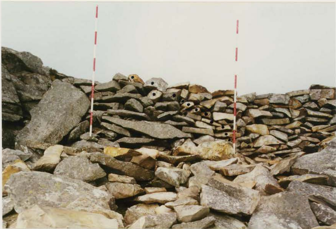
Plate 41 G1022/207/26 ; Collapse S6 after conservation.
