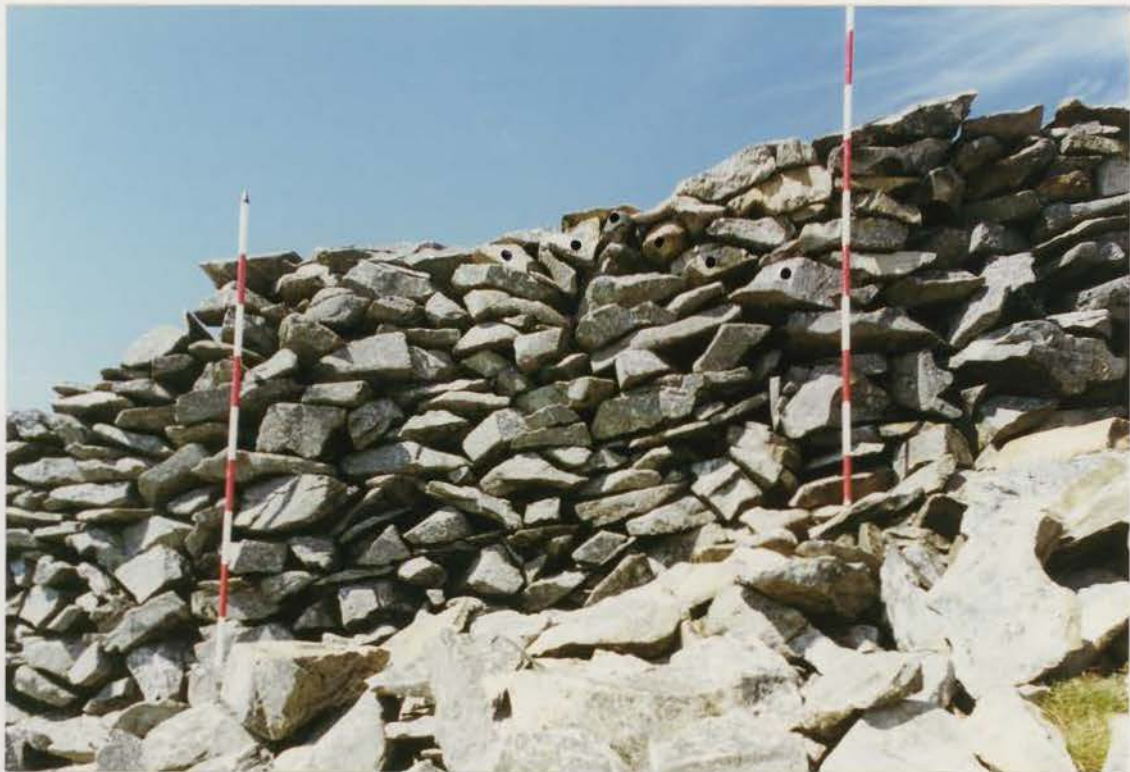
Plate 8 G1022/205/15 ; Collapse S1 after conservation.
