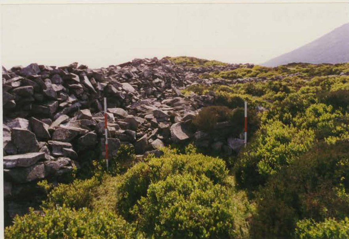
Plate 163 G1022/199/16 ; Collapse 108a before conservation.
