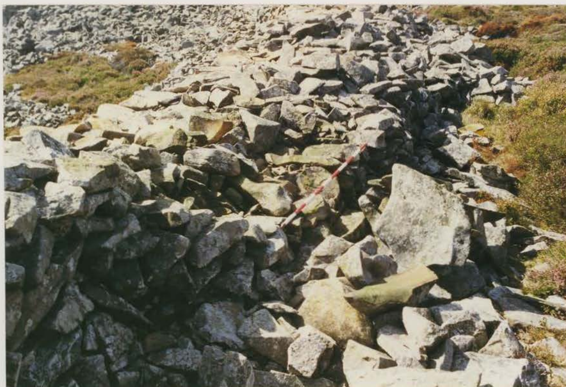
Plate 100 G1022/206/03 ; Collapse V, inner face, after clearance.
