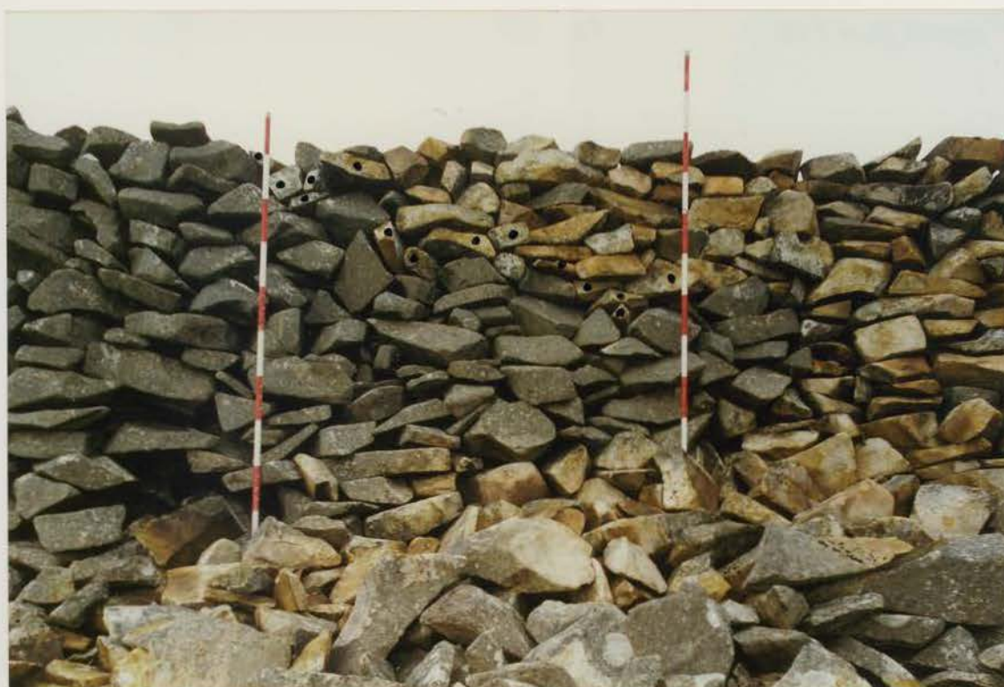
Plate 76 G1022/210/18 ; Collapse W after conservation.
