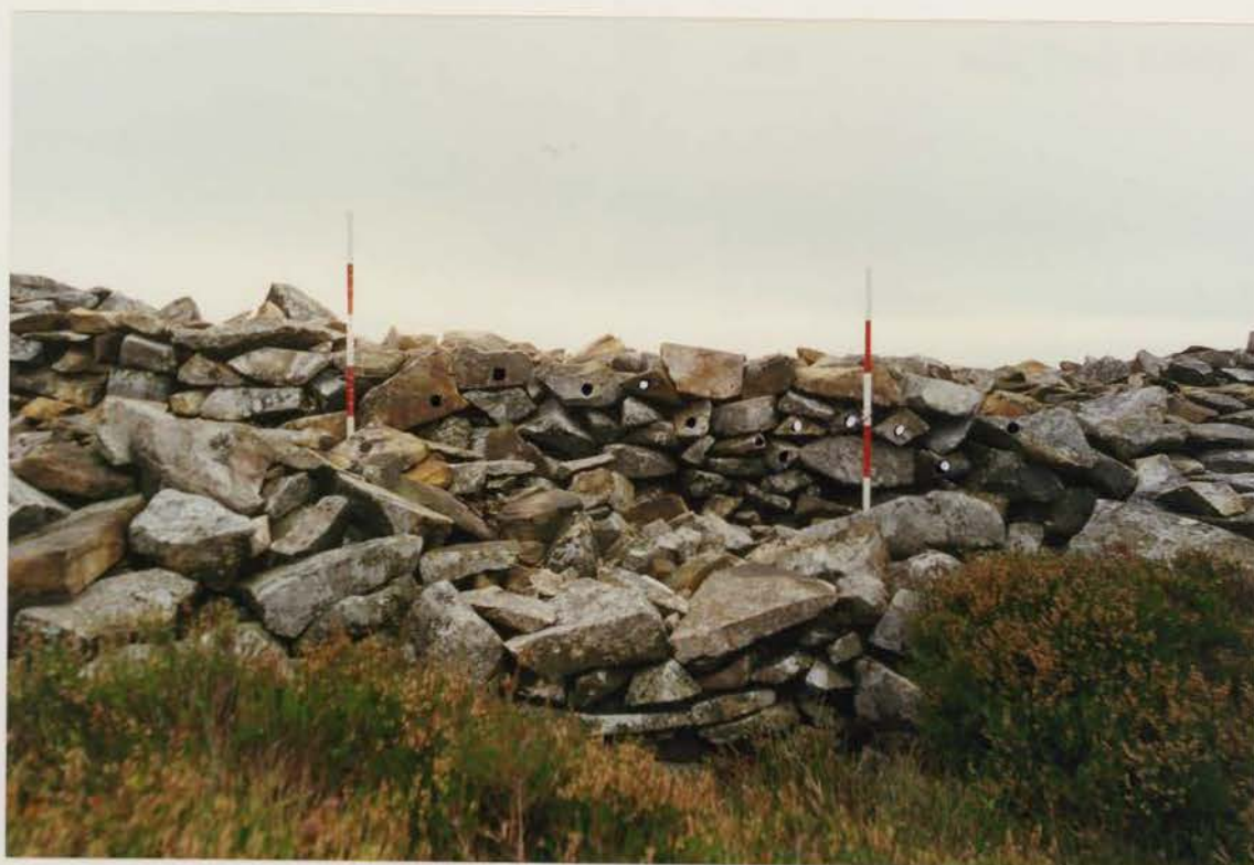
Plate 112 G1022/209/26 ; Collapse V4, after conservation.
