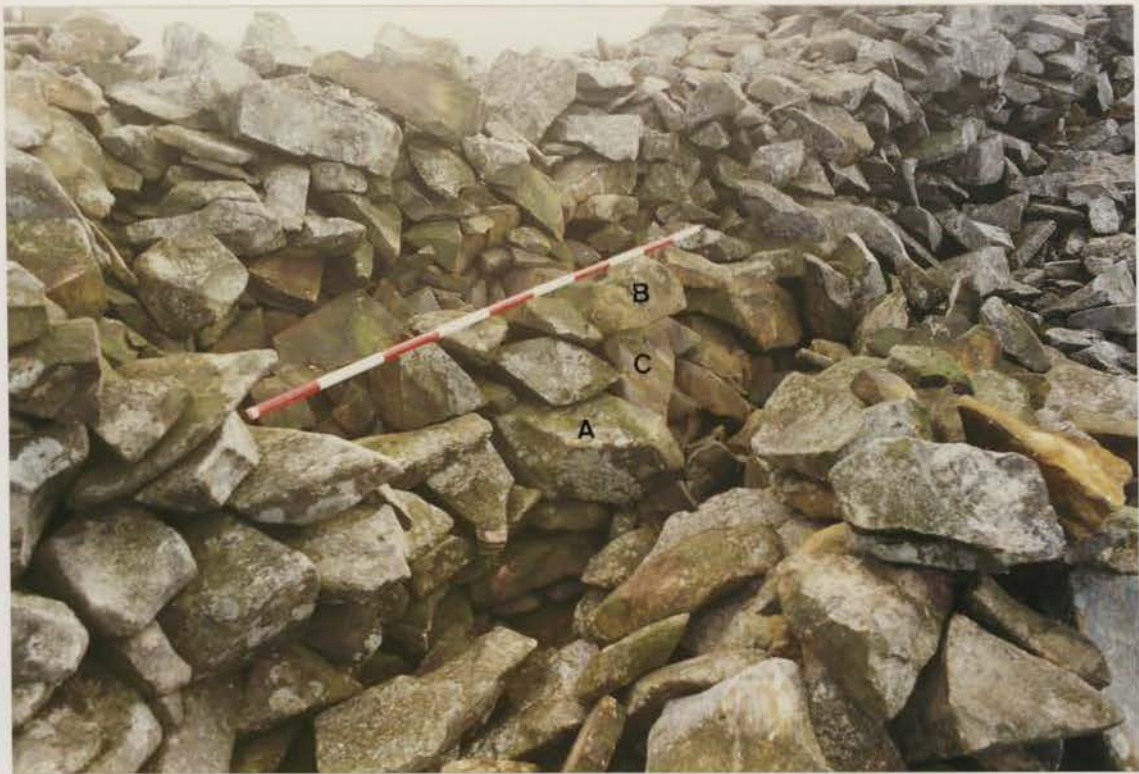
Plate 136 G1022/206/25 ; Collapse X4 after clearance.
