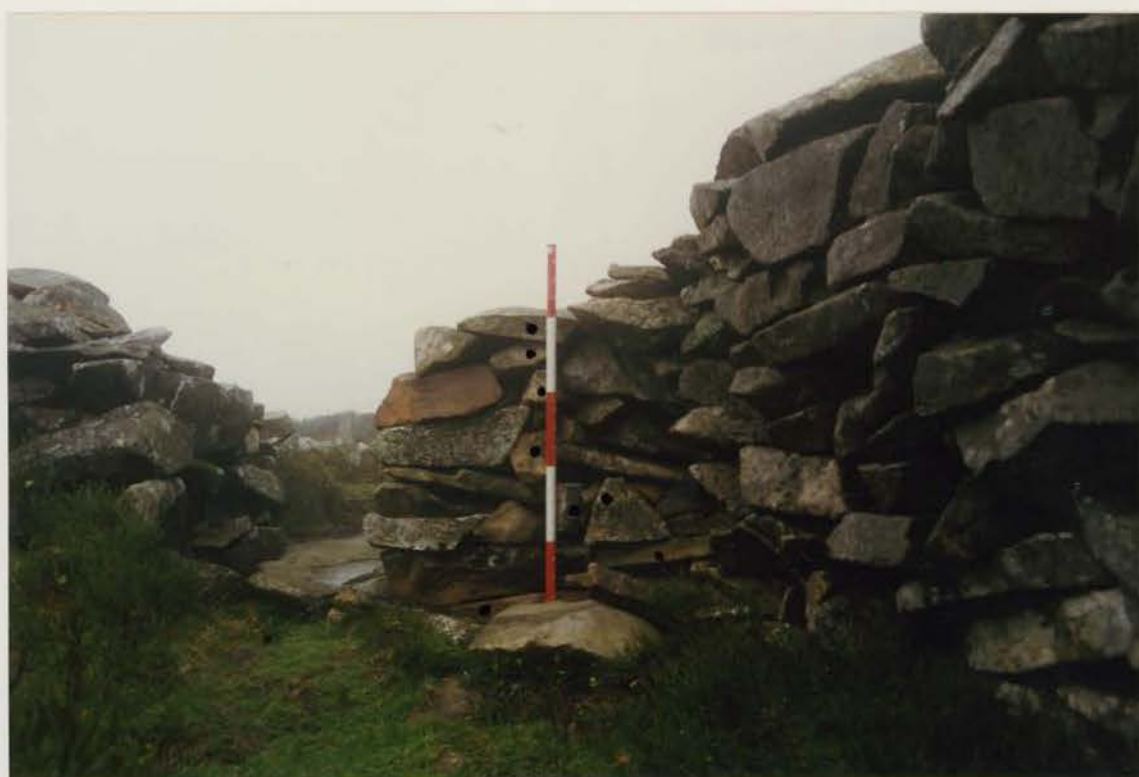
Plate 226 G1022/213/12 ; Collapse 10a after conservation.
