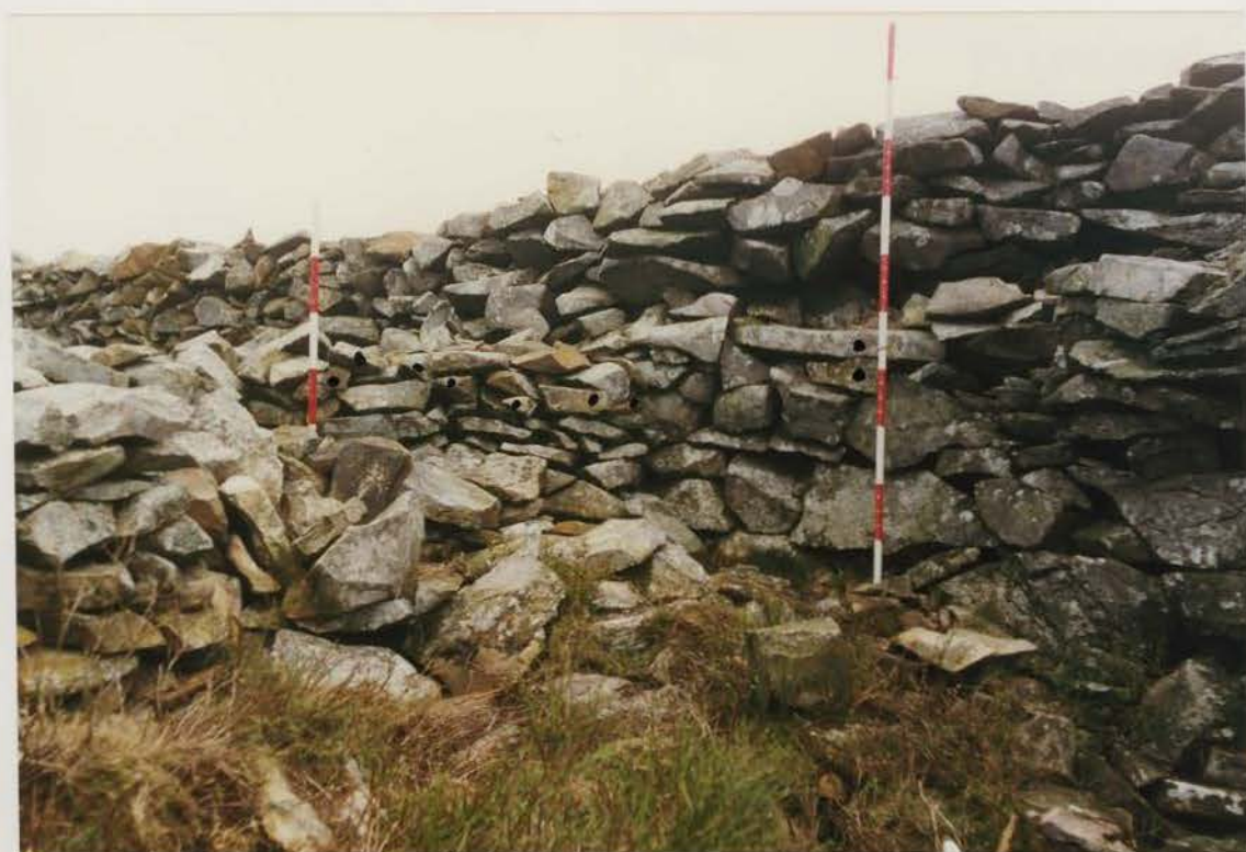
Plate 200 G1022/207/29 ; Collapses 41d and 41e after conservation.
