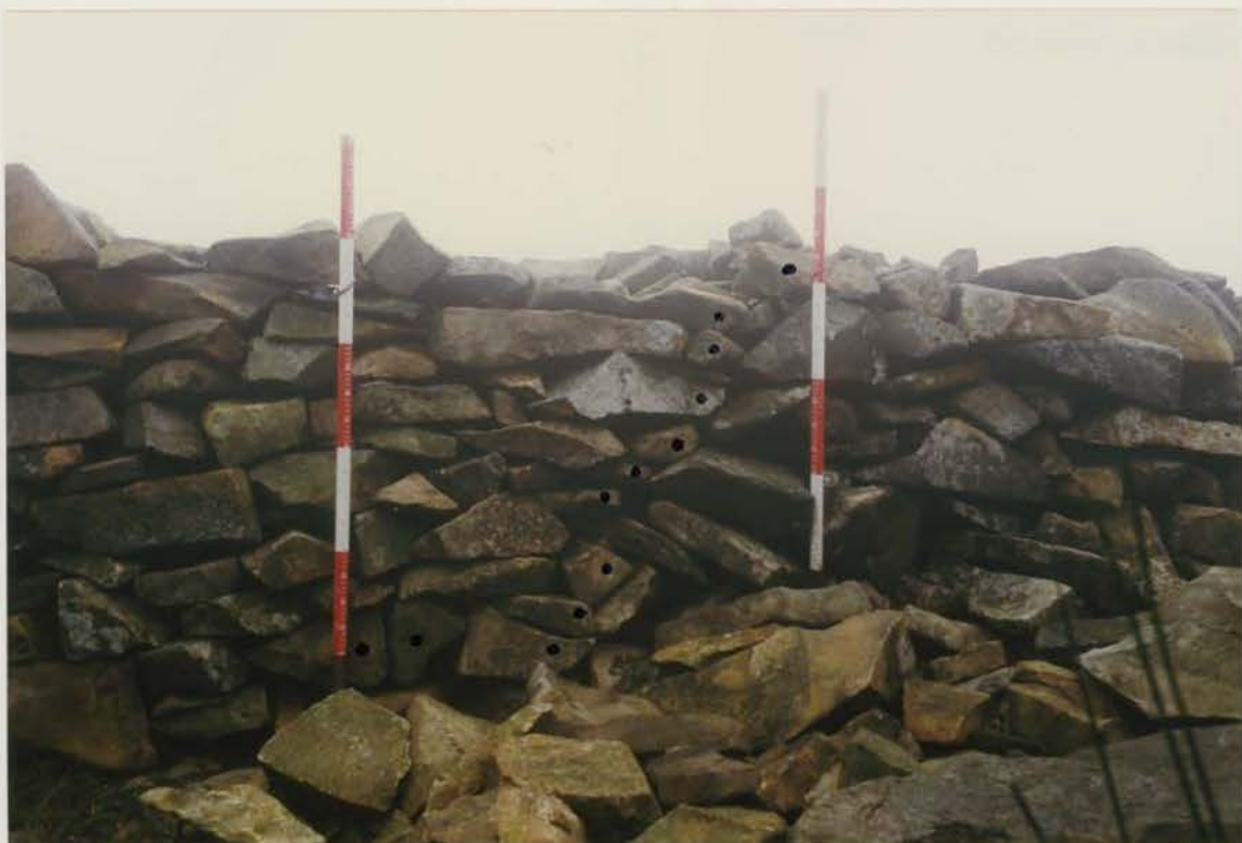
Plate 214 G1022/213/03 ; Collapse 9b (SW.) after conservation.
