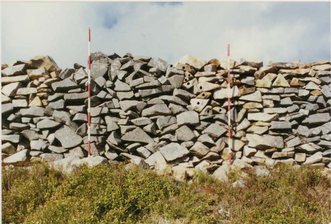
Plate 60 G1022/209/15 ; Collapse V1 after conservation.
