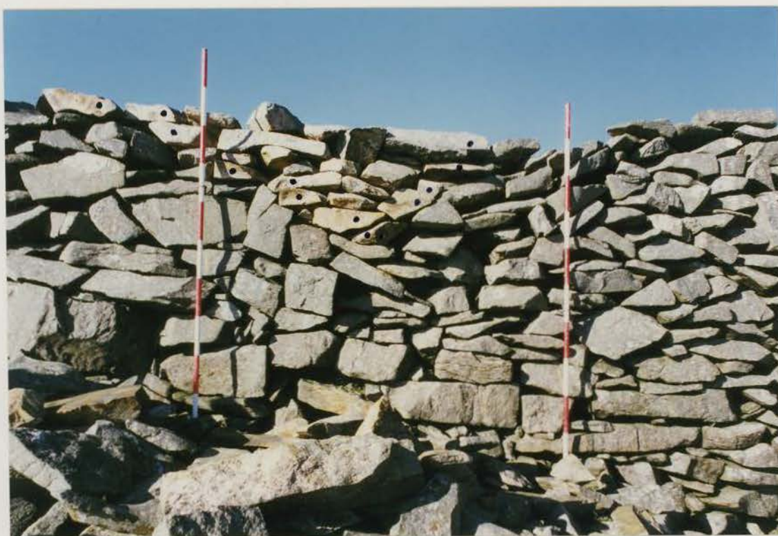
Plate 86 G1022/211/13 ; Collapse X1 after conservation.
