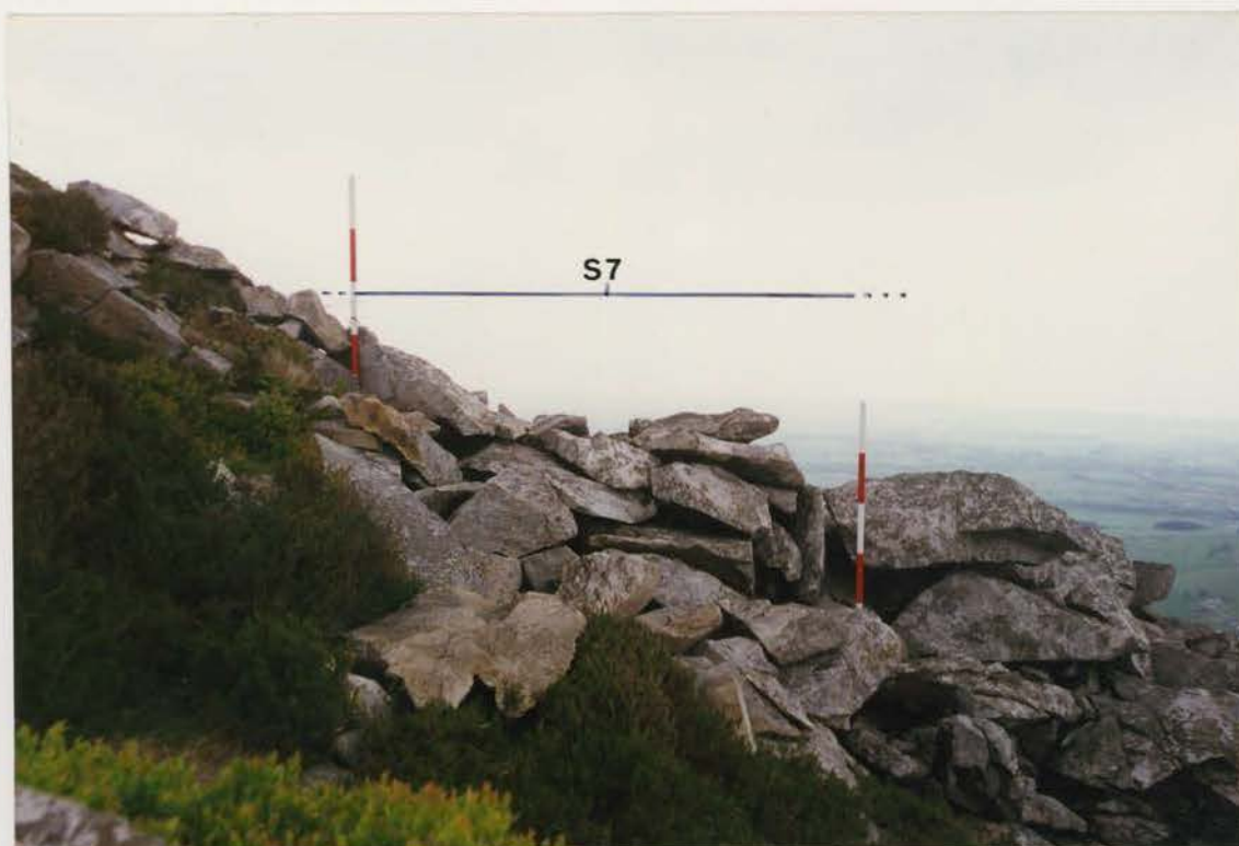
Plate 19 G1022/194/08 ; Collapse S7 before conservation.
