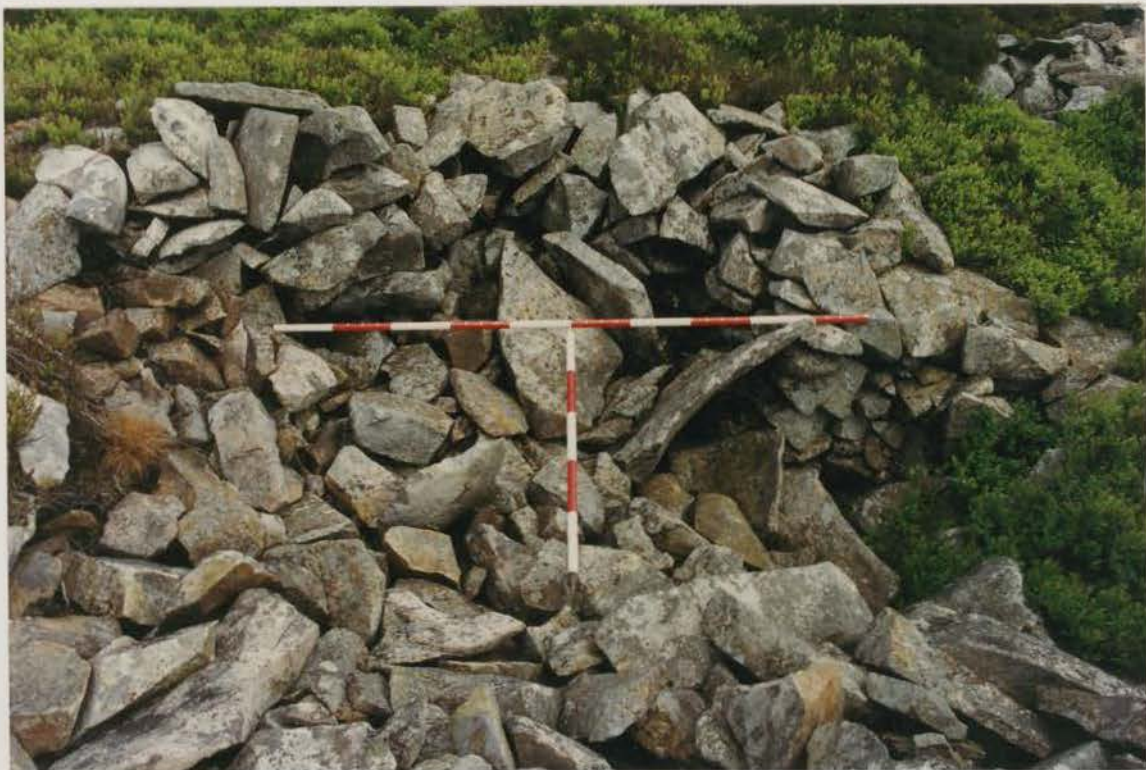
Plate 180 G1022/200/00a; Collapse 106a before conservation.
