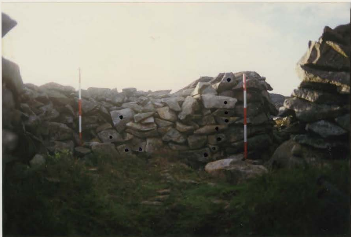
Plate 234 G1022/212/04 ; Collapse 49a after conservation.
