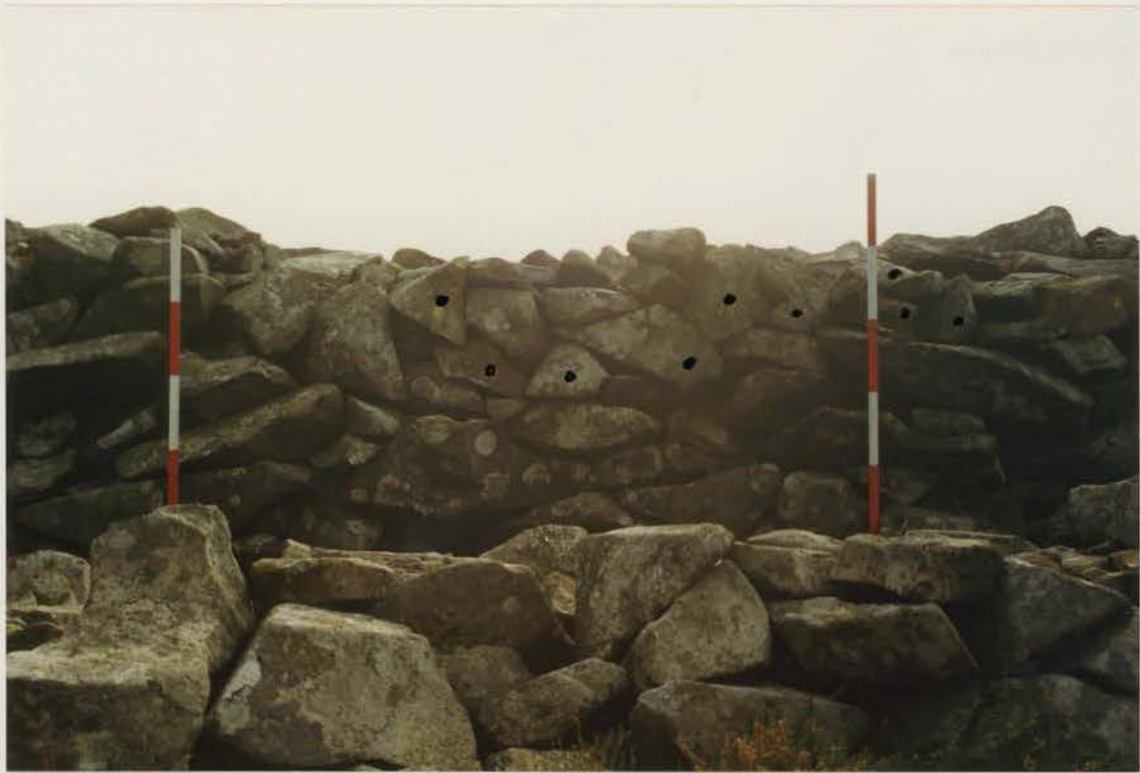
Plate 129 G1022/210/10 ; Collapse W4 after conservation.
