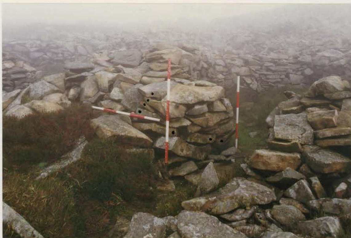
Plate 225 G1022/213/17 ; Collapse 10a after conservation.
