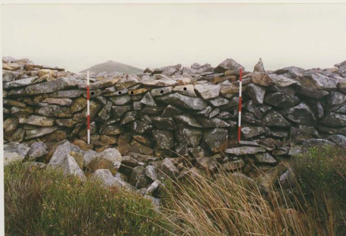
Plate 102 G1022/208/23 ; Collapse V, inner face, after conservation.
