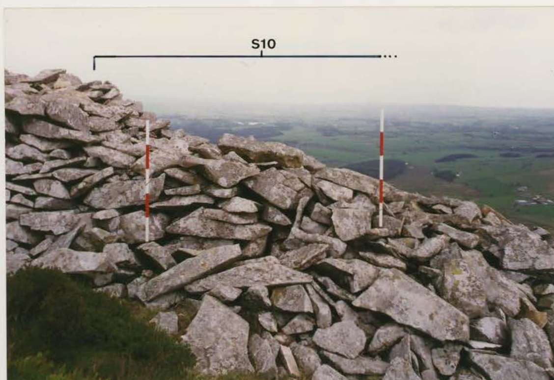
Plate 26 G1022/194/20 ; Collapse S10 before conservation.
