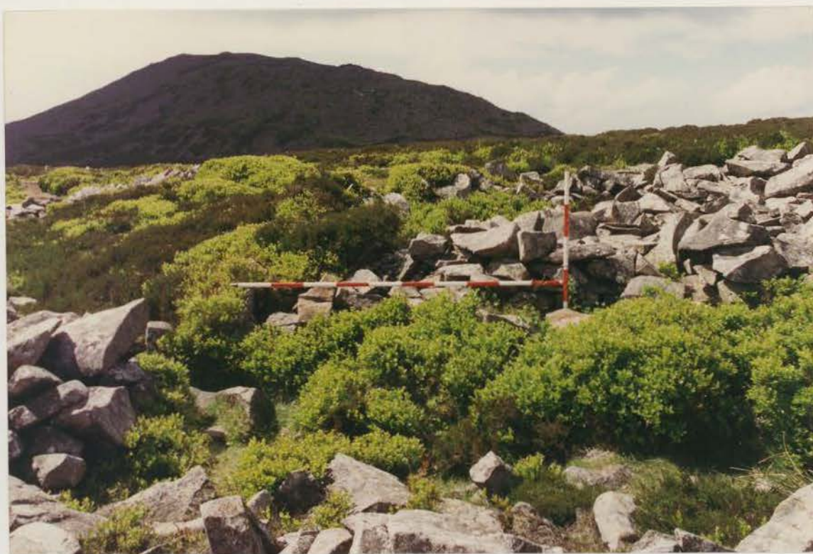
Plate 172 G1022/200/07a; Collapse 45a before conservation.
