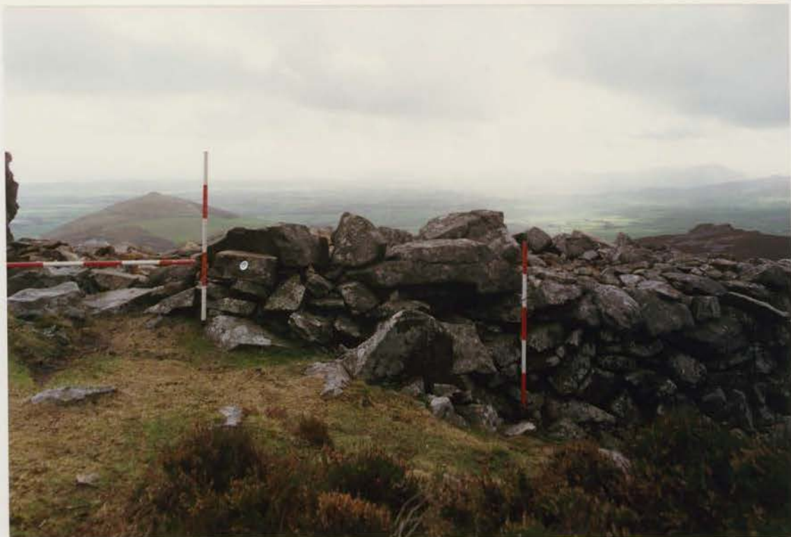
Plate 93 G1022/208/15 ; Collapse U4 after conservation.
