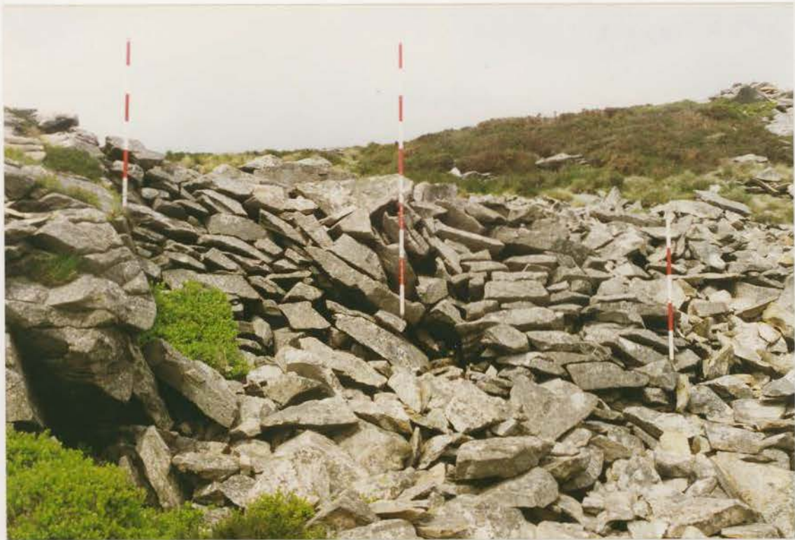
Plate 1 G1022/193/12 ; Collapse S12.
