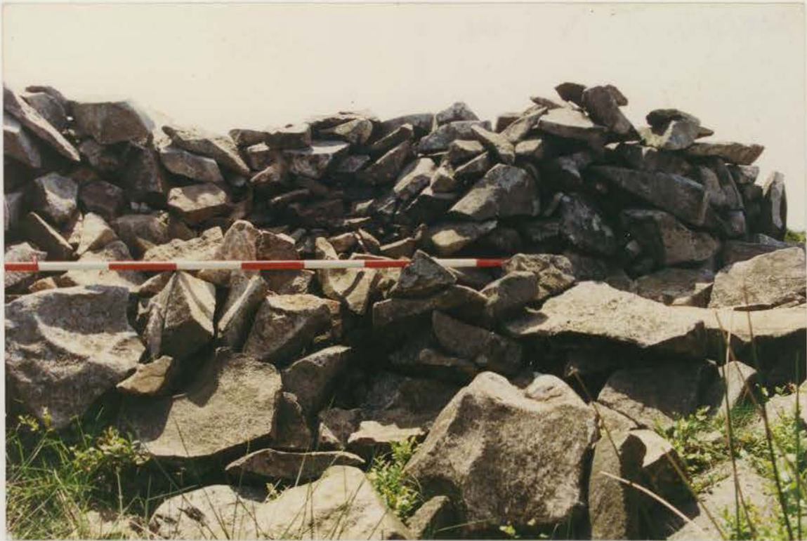
Plate 209 G1022/201/11 ; Collapse 9b (SW.) before conservation.
