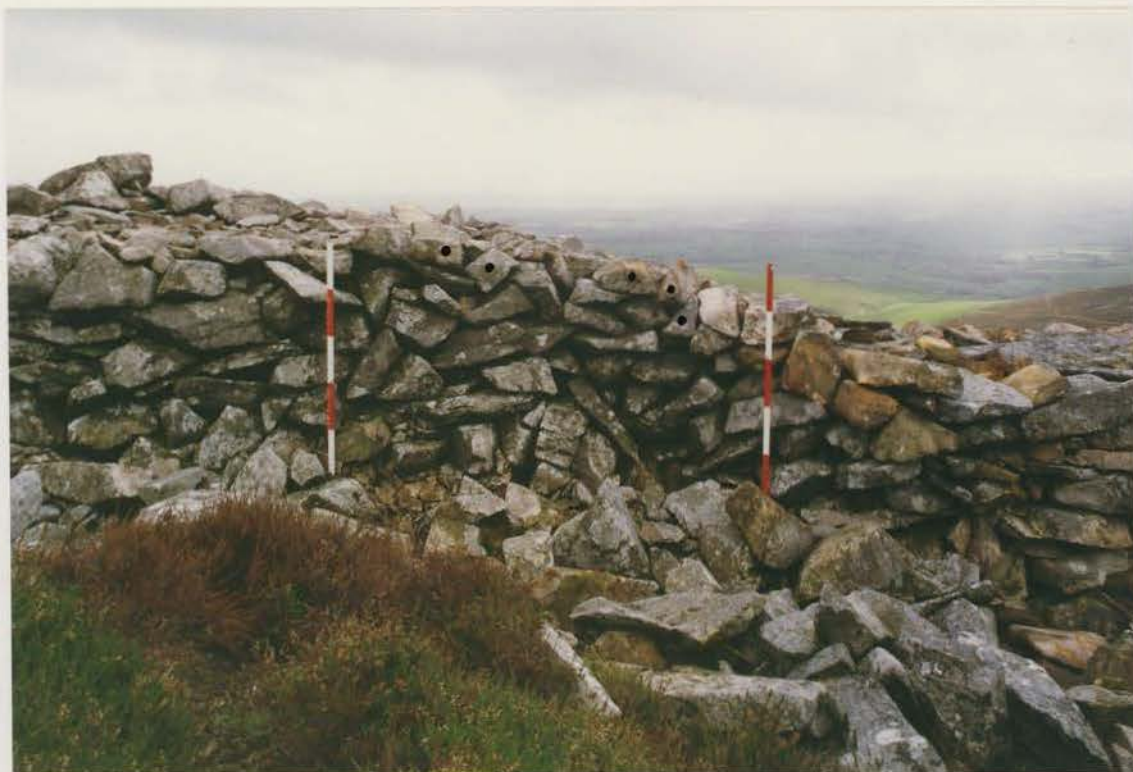
Plate 97 G1022/208/20 ; Collapse U5 after conservation.
