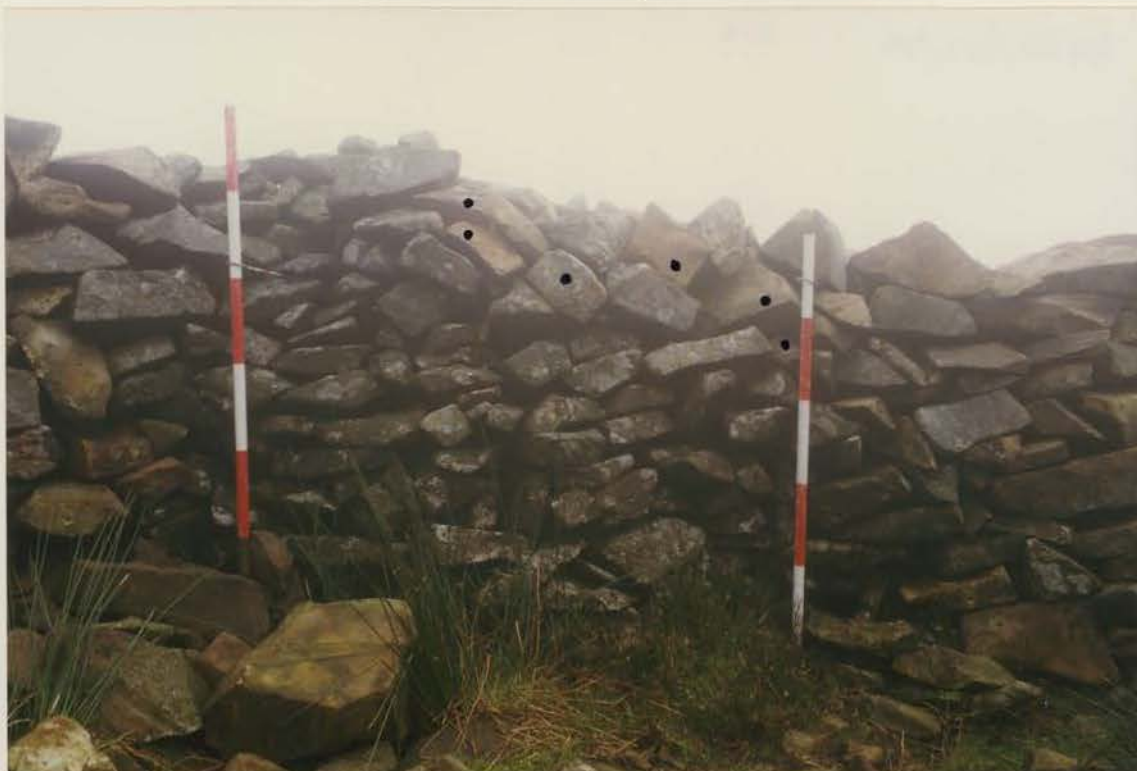
Plate 212 G1022/212/35; Collapse 9b(NE.) after conservation.
