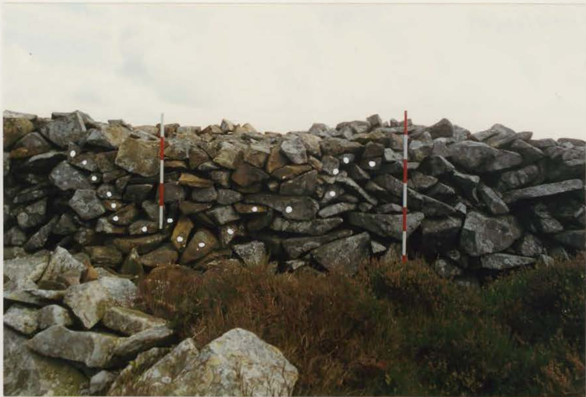
Plate 125 G1022/210/07 ; Collapse W after conservation.
