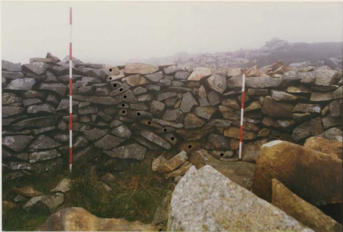
Plate 205 G1022/212/34 ; Collapse 9a, rebuilt masonry.
