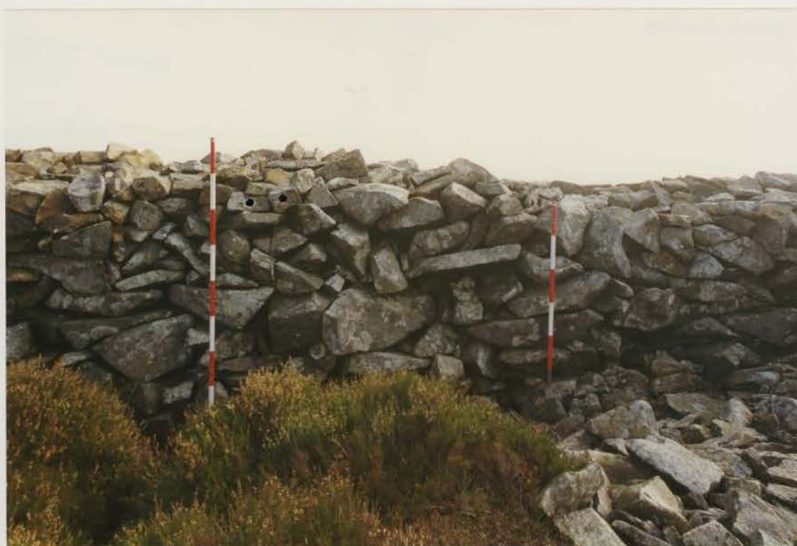
Plate 128 G1022/210/09 ; Collapse W4 after conservation.
