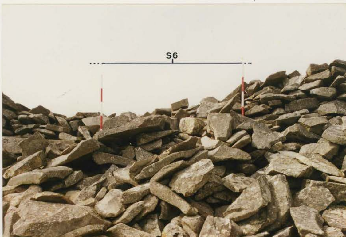
Plate 33 G1022/193/36 ; Collapse S6 before conservation.
