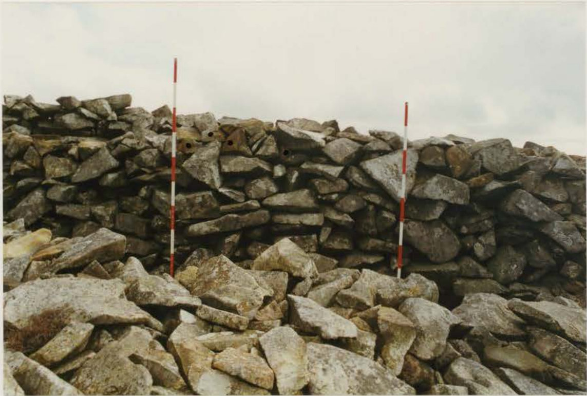
Plate 121 G1022/210/03 ; Collapse V6 after conservation.
