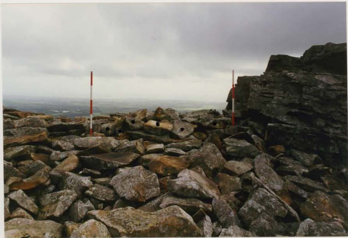
Plate 40 G1022/208/12 ; Collapse S11 after conservation.
