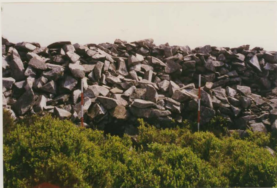
Plate 162 G1022/199/14 ; Collapse 108a before conservation.
