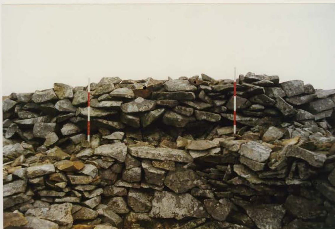
Plate 142 G1022/210/32 ; Collapse X6 after conservation.
