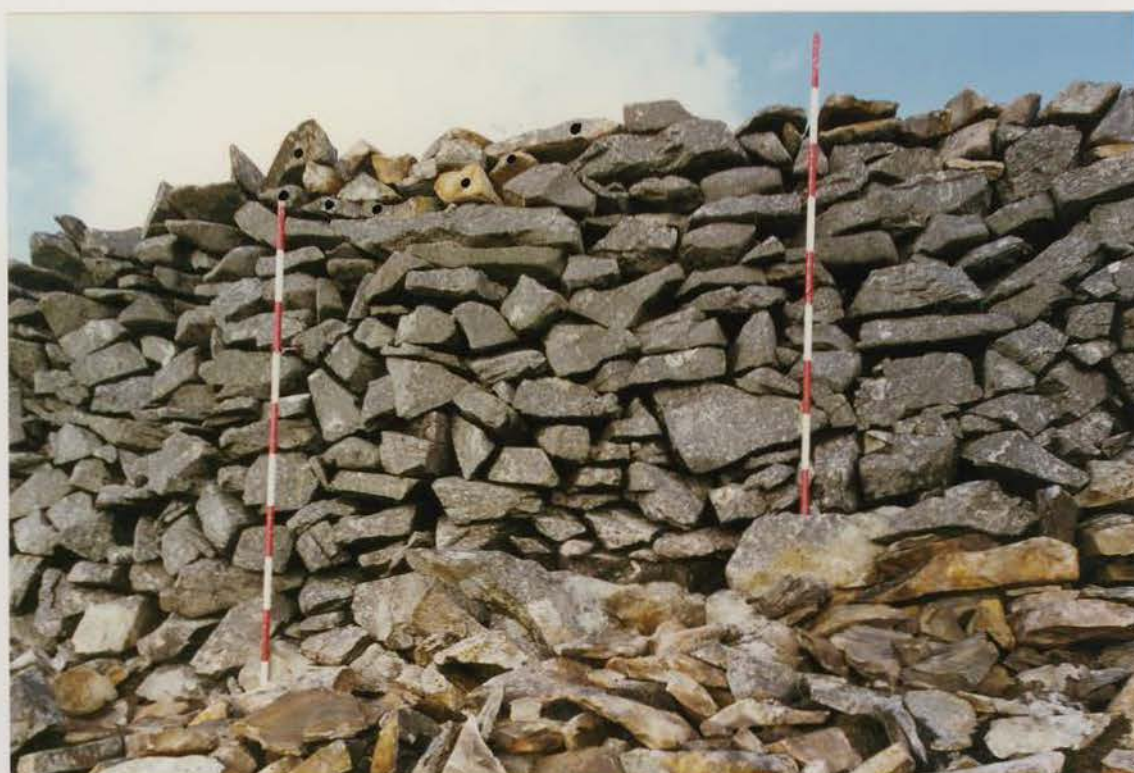
Plate 50 G1022/209/05 ; Collapse U2 after conservation.
