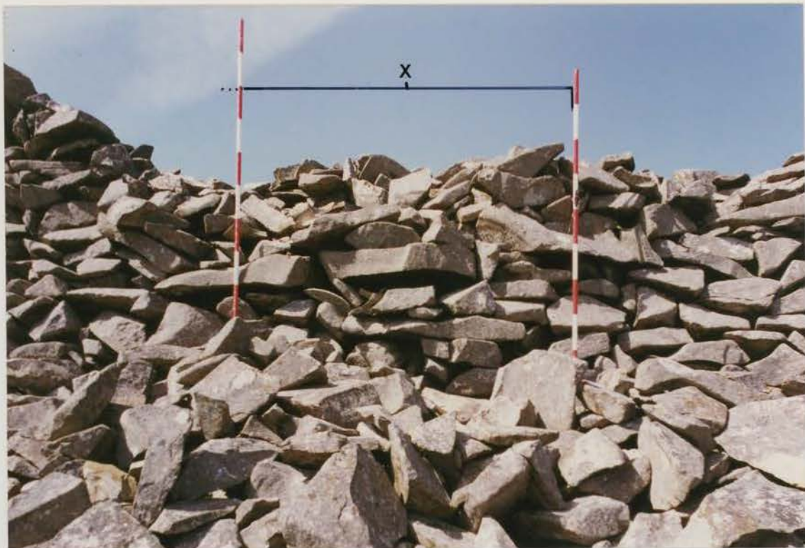
Plate 80 G1022/198/09 ; Collapse X before conservation.
