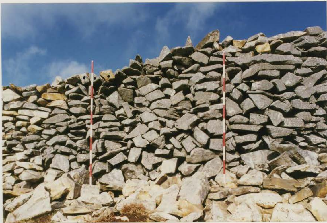
Plate 52 G1022/209/07 ; Collapse U3 after conservation.
