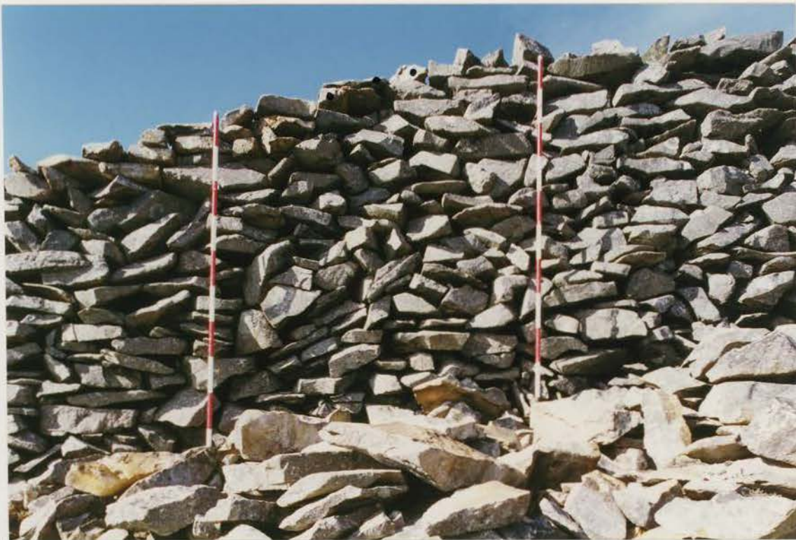
Plate 16 G1022/207/18 ; Collapse S4 after conservation.
