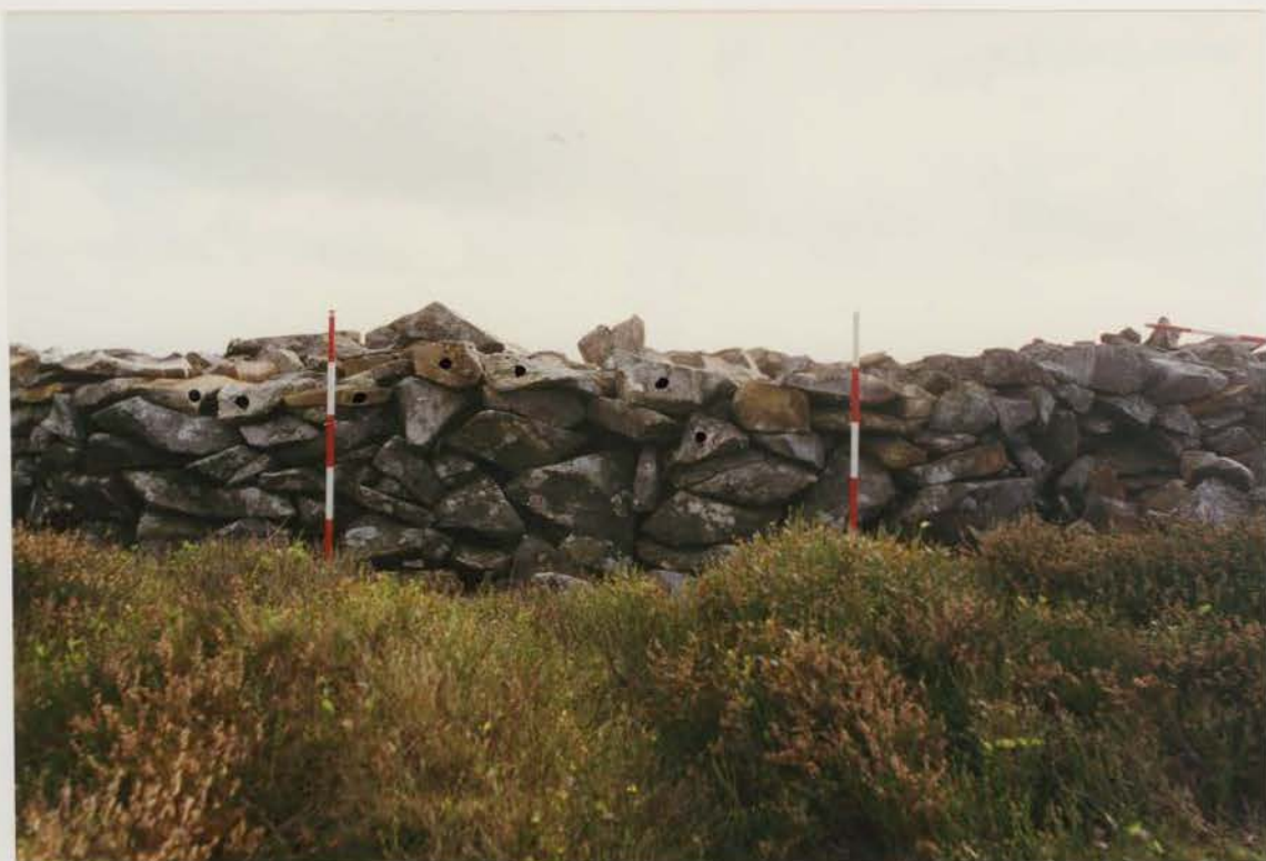
Plate 104 G1022/208/27 ; Collapse V3 after conservation.
