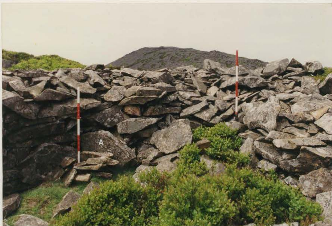
Plate 195 G1022/200/29a; Collapse 41c (SE.) before conservation.
