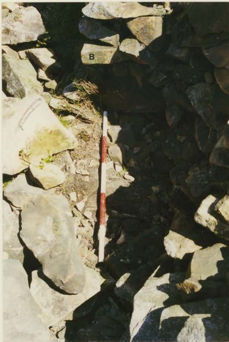
Plate 211 G1022/203/15; Collapse 9b after clearance.
