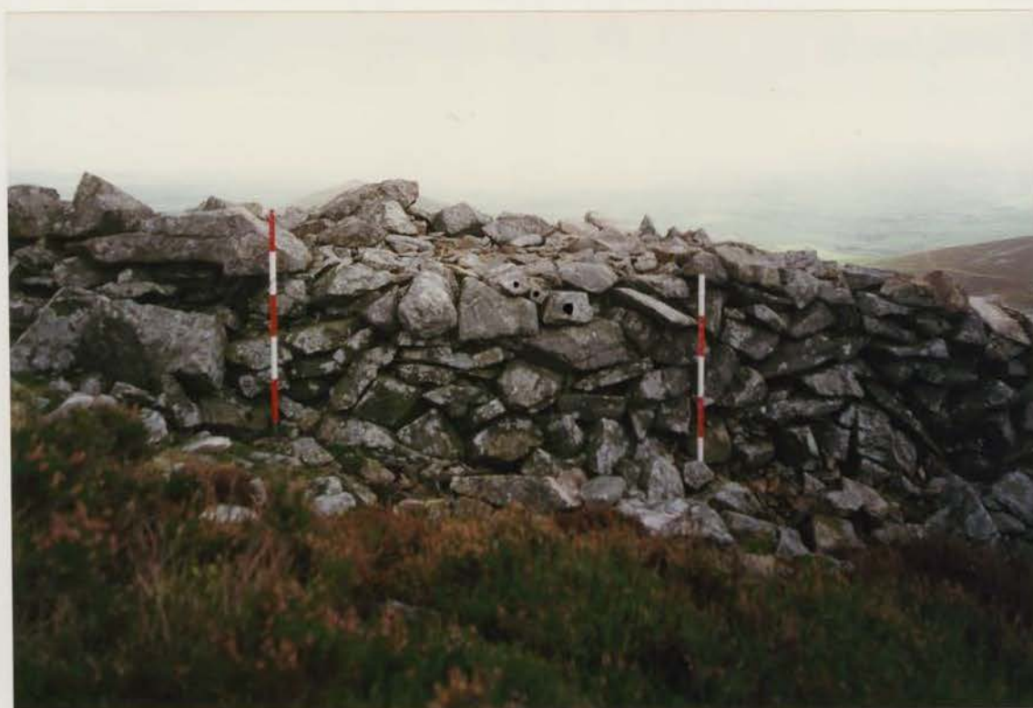
Plate 96 G1022/208/17 ; Collapse U5 after conservation.
