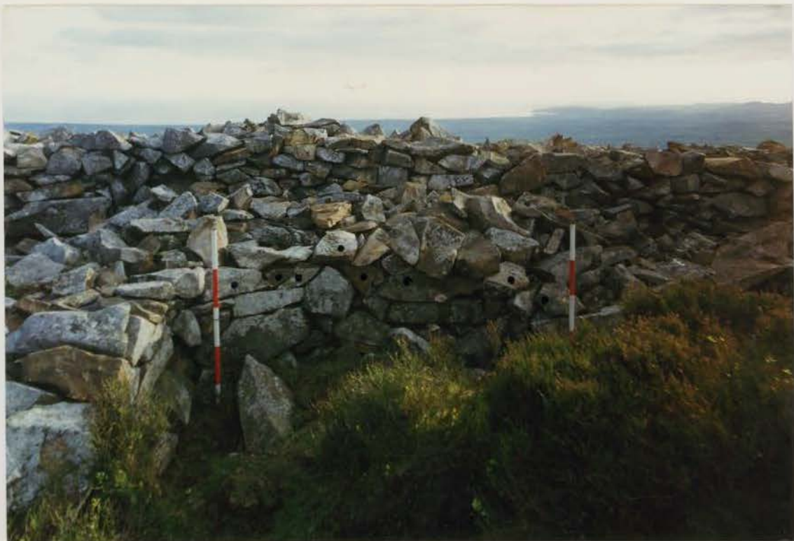
Plate 160 G1022/211/36a; Collapse 45Ad after conservation.
