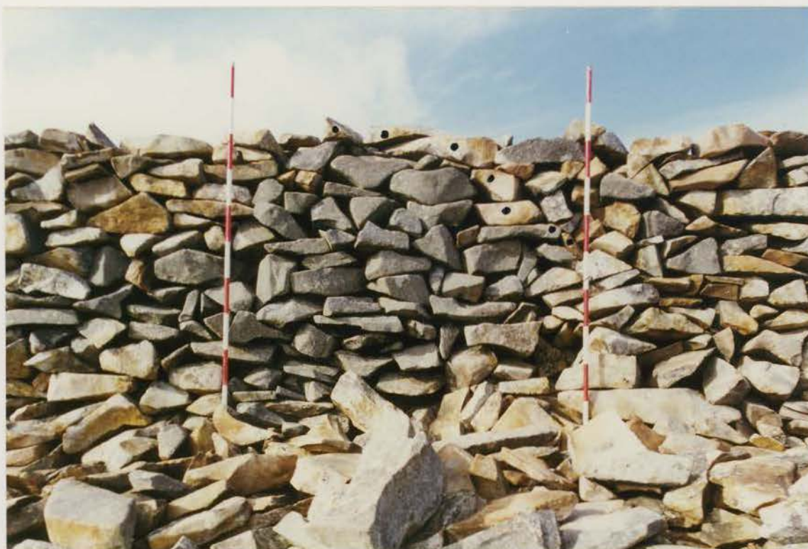
Plate 69 G1022/209/24 ; Collapse V2 after conservation.
