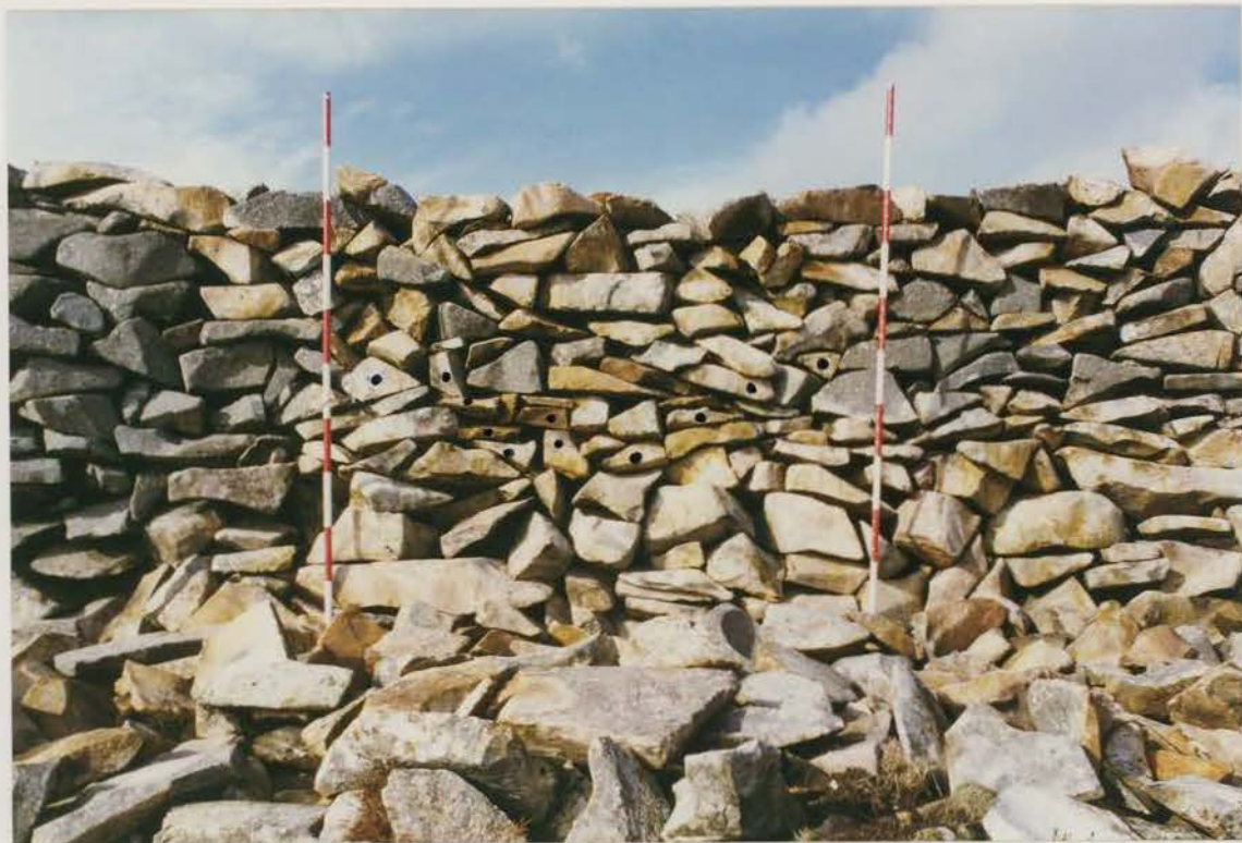
Plate 68 G1022/209/22 ; Collapse V2 after conservation.
