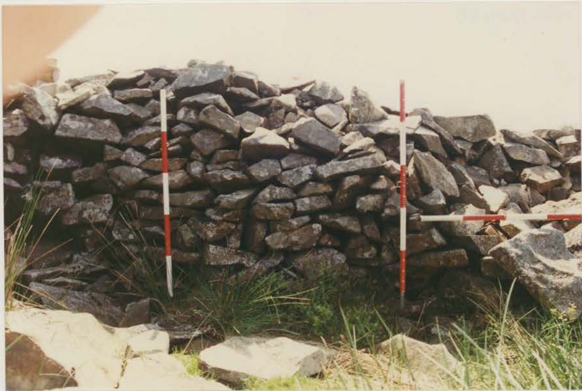
Plate 207 G1022/201/08 ; Collapse 9b (NE.) before conservation.
