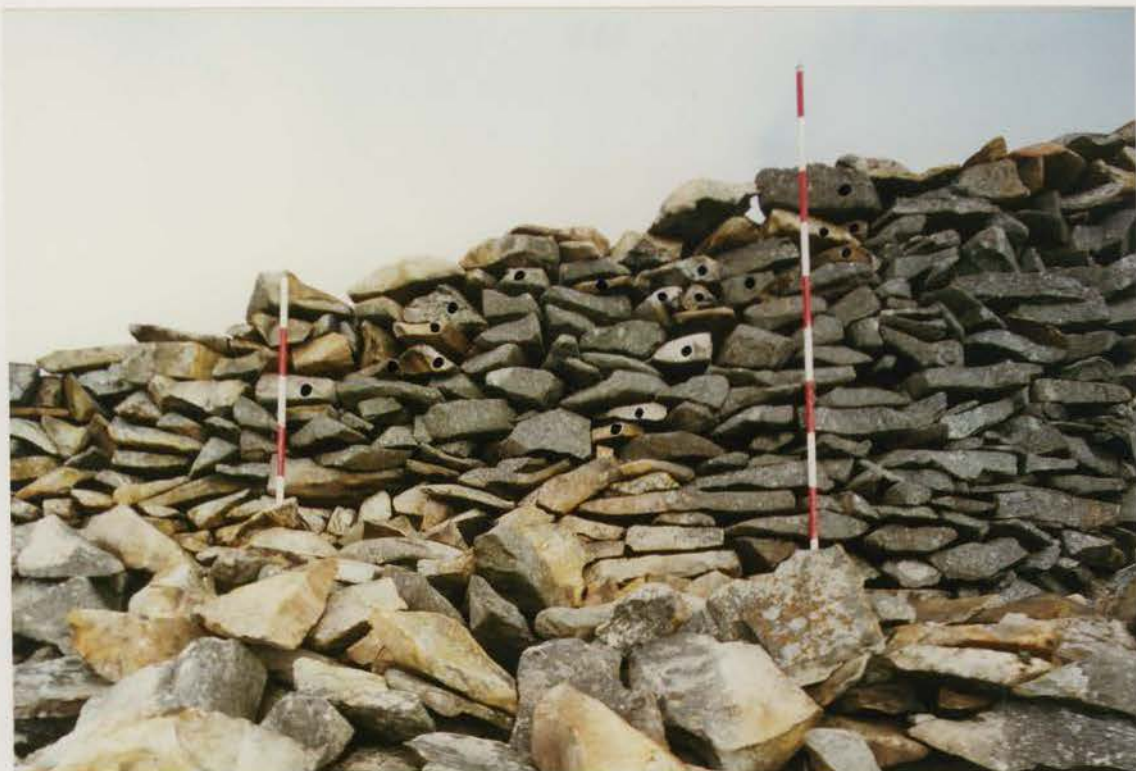
Plate 43 G1022/207/21 ; Collapse S6 after conservation.
