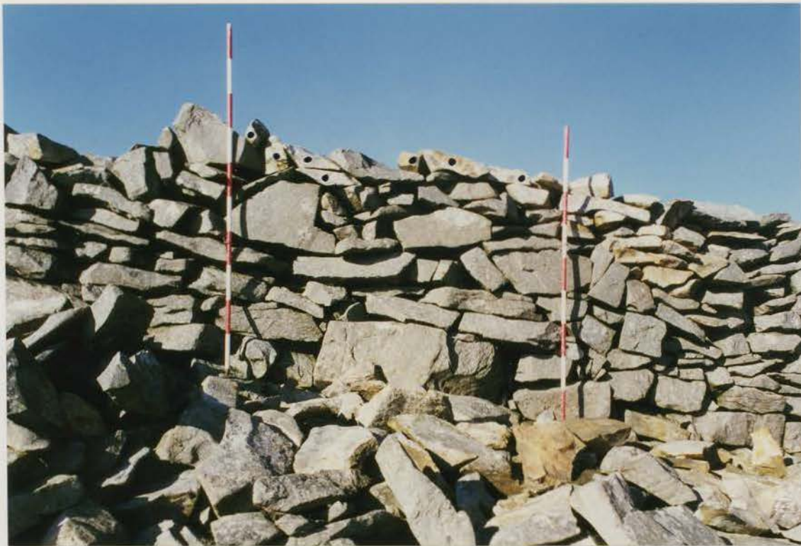
Plate 89 G1022/211/15 ; Collapse X2 after conservation.
