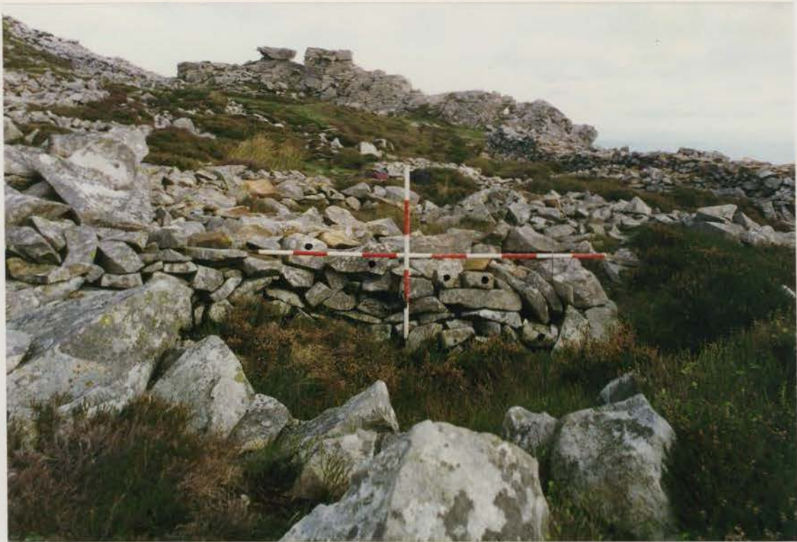
Plate 179 G1022/211/32 ; Collapse 46a after conservation.
