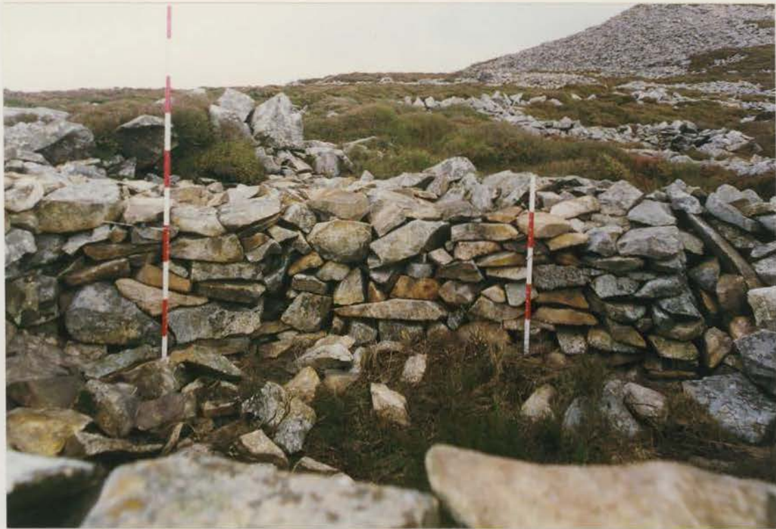
Plate 189 G1022/207/36 ; Collapses 41a and 41b after conservation.
