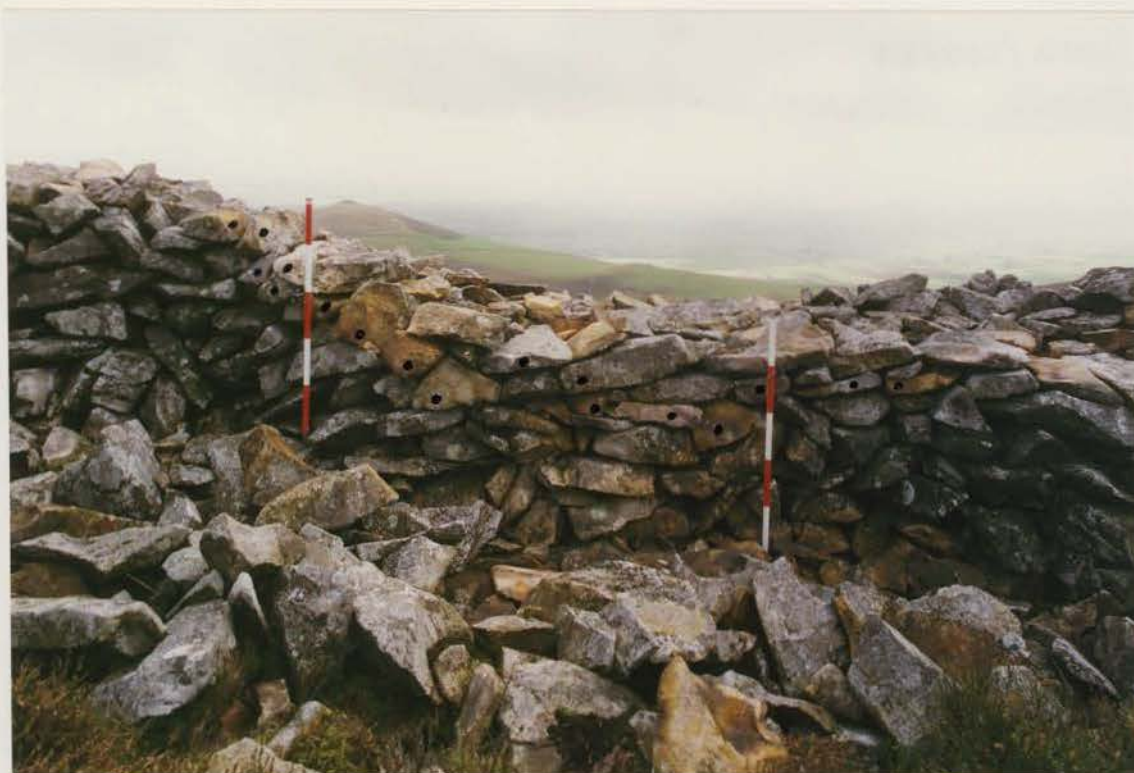
Plate 101 G1022/208/21 ; Collapse V, inner face, after conservation.
