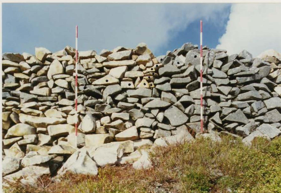
Plate 66 G1022/209/17; Collapse V2 after conservation.
