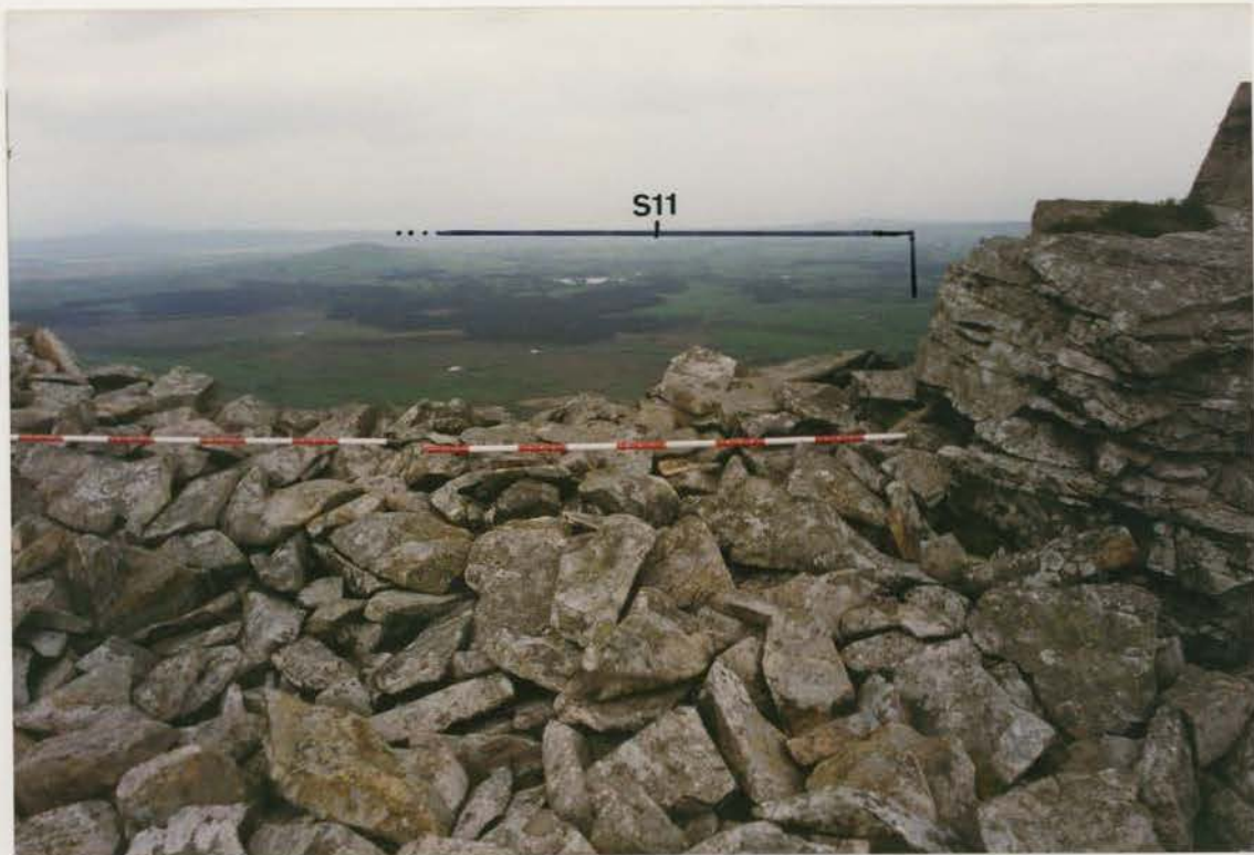
Plate 31 G1022/194/28 ; Collapse S11 before conservation.
