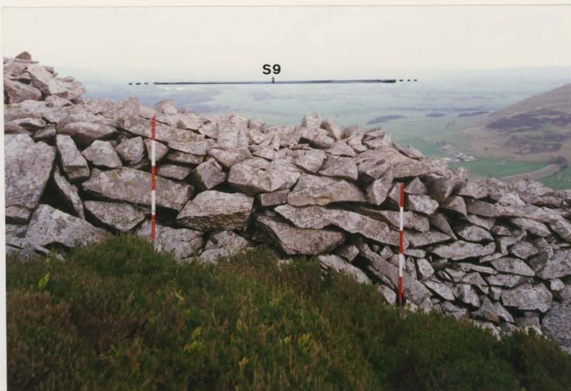
Plate 23 G1022/194/15 ; Collapse S9 before conservation.
