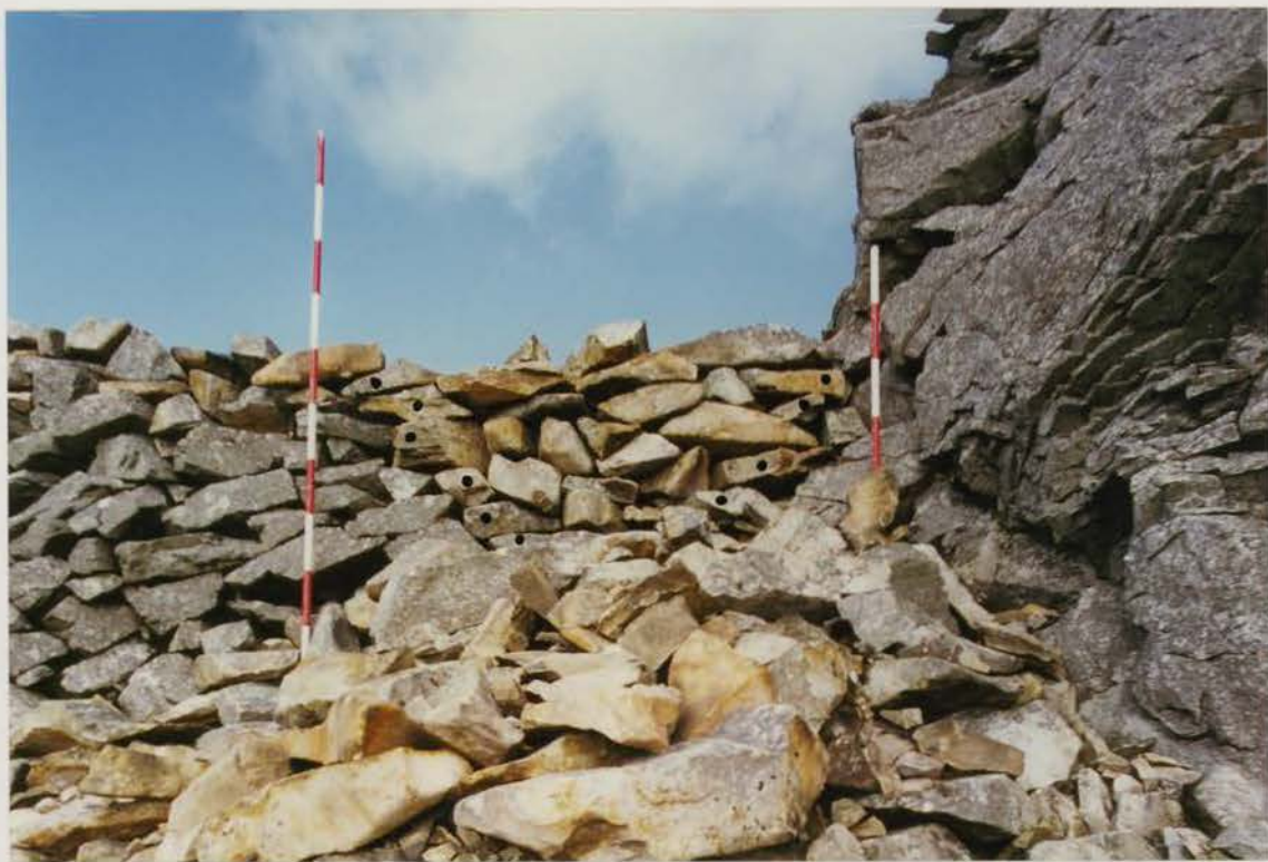
Plate 46 G1022/209/00 ; Collapse U after conservation.
