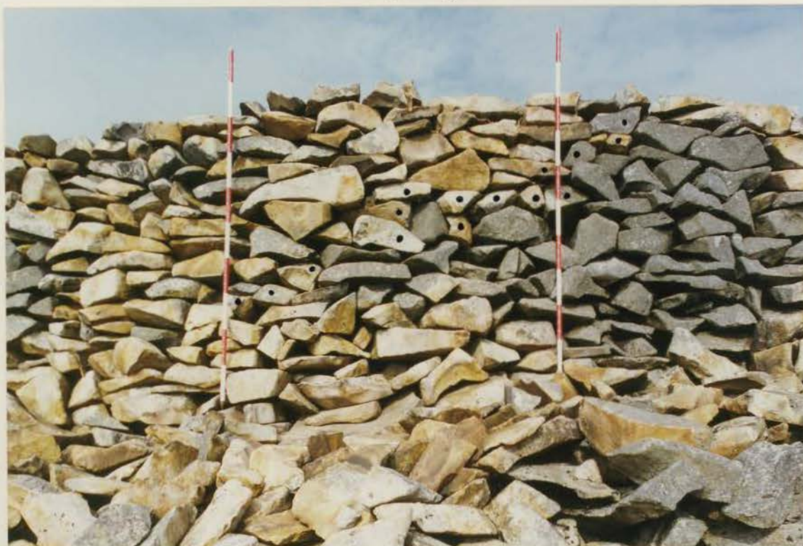
Plate 74 G1022/210/13; Collapse W after conservation.
