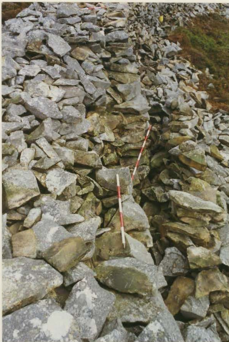
Plate 73 G1022/205/17; Collapse W after clearance.
