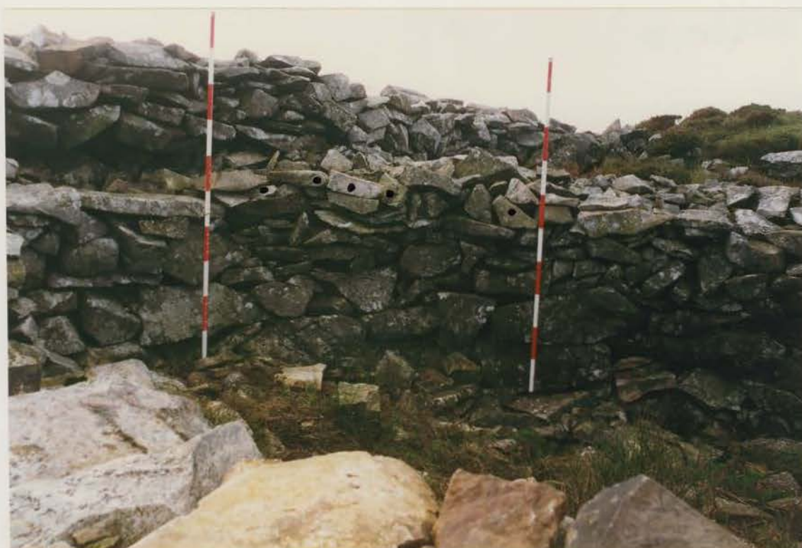
Plate 196 G1022/207/30 ; Collapse 41c (NW.) after conservation.
