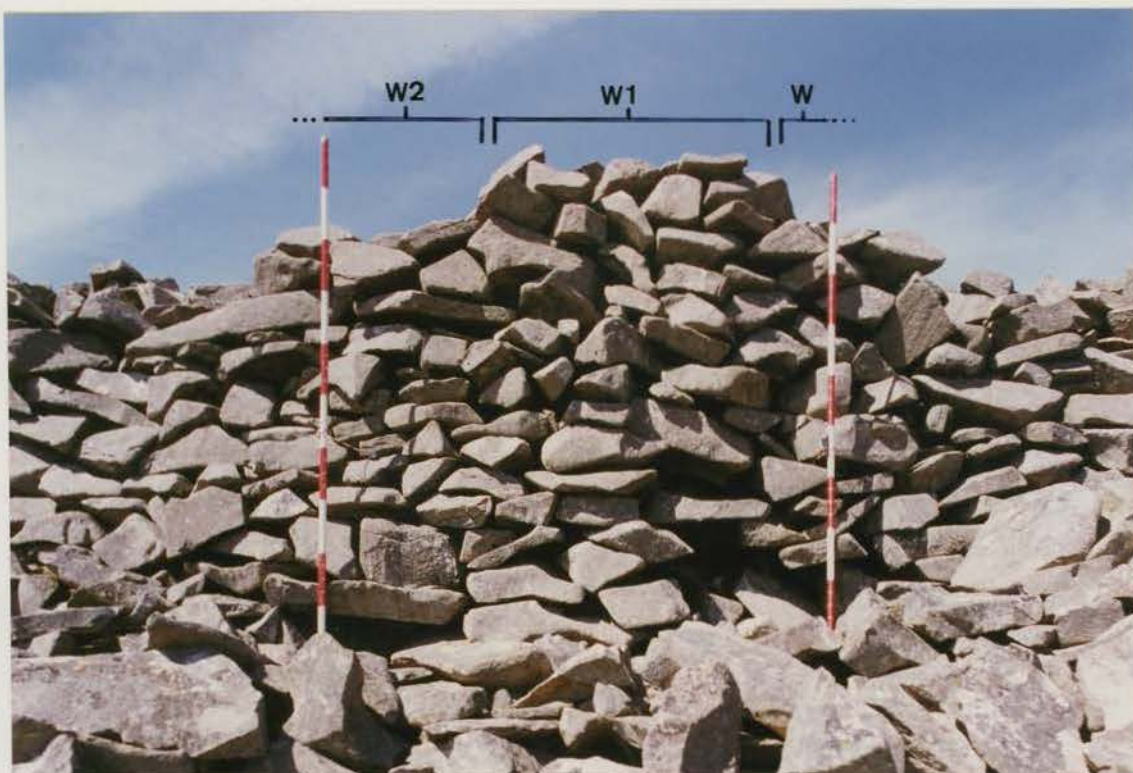
Plate 77 G1022/198/04 ; Collapse W1.
