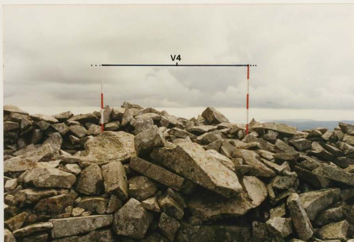
Plate 106 G1022/195/21 ; Collapse V4 before conservation.
