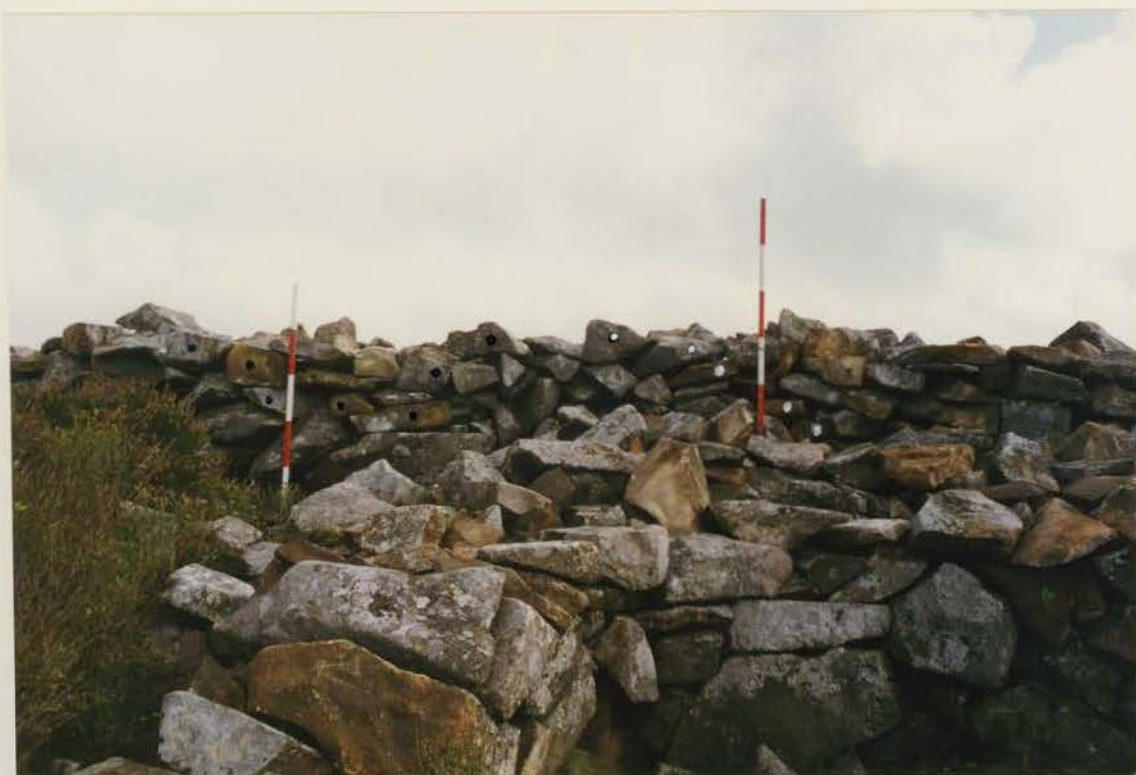
Plate 110 G1022/208/29; Collapse V4, after conservation.
