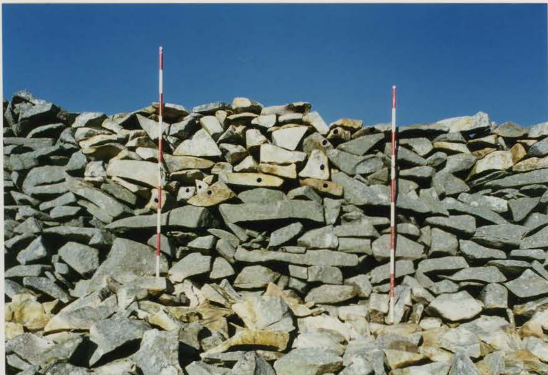
Plate 82 G1022/211/10 ; Collapse X after conservation.
