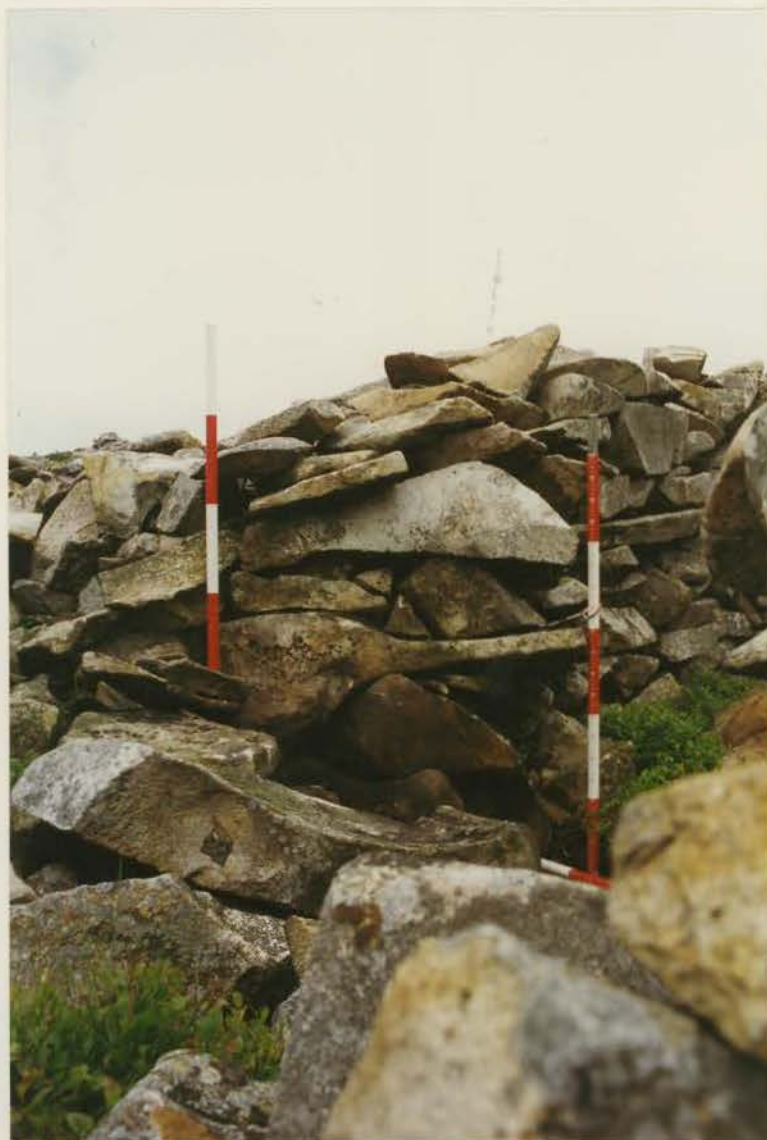
Plate 224 G1022/203/33; Collapse 10a after clearance, showing 'hidden face'.
