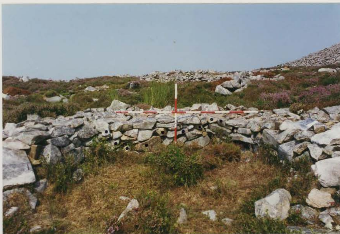
Plate 150 G1022/205/30 ; Collapse 45Aa after conservation.
