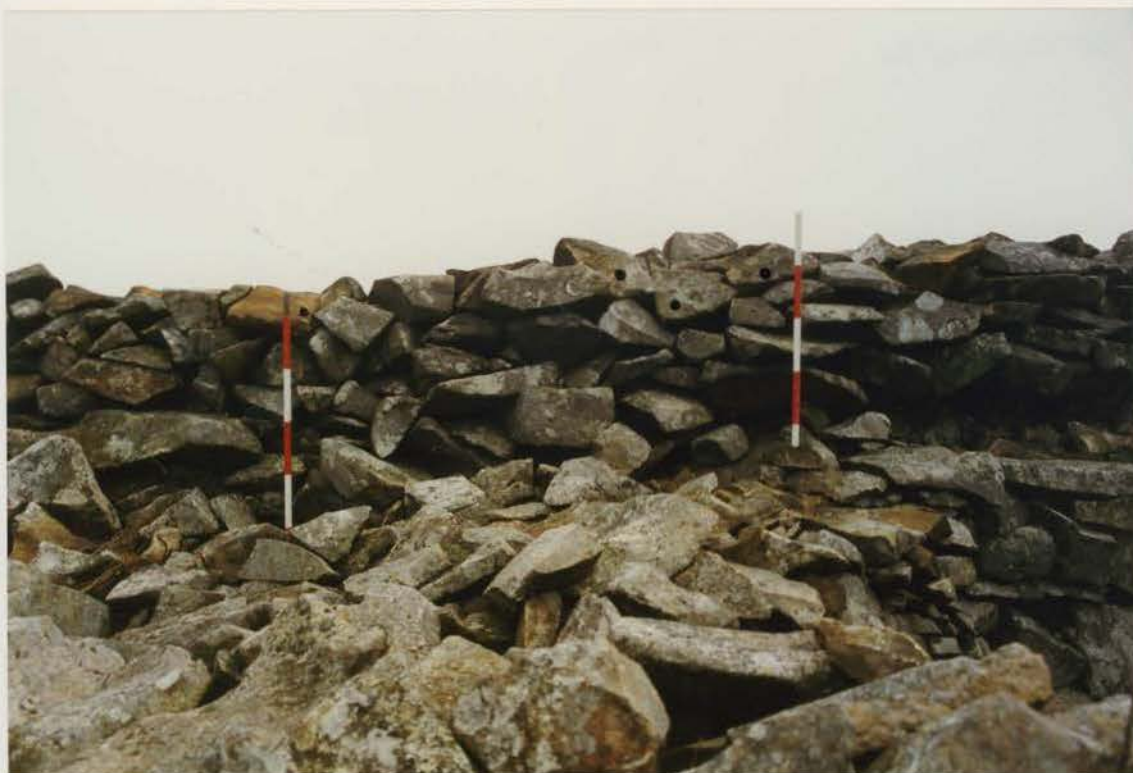
Plate 141 G1022/210/30 ; Collapse X5 after conservation.
