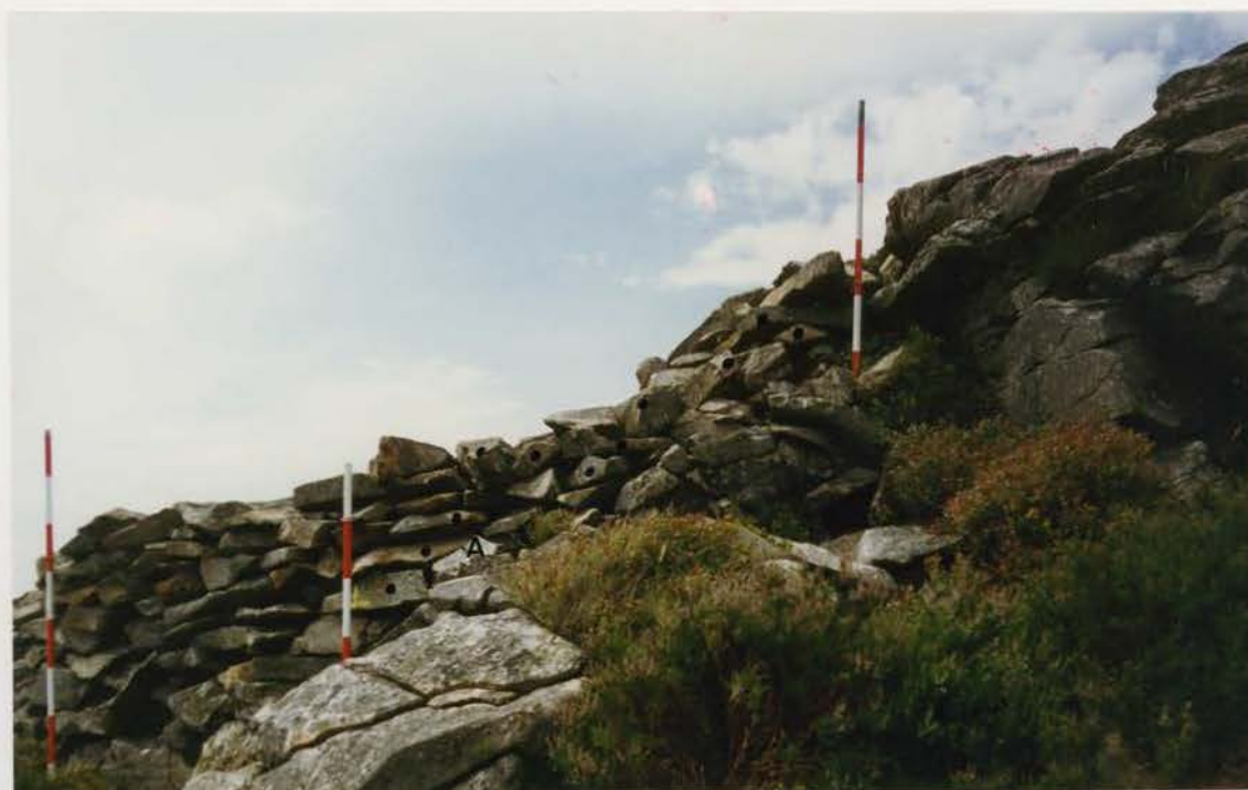
Plate 6 G1022/205/10 ; Collapse S1 after conservation.
