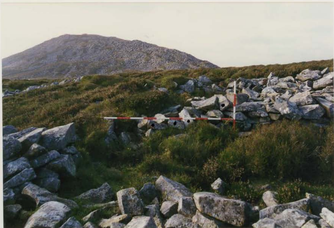
Plate 174 G1022/211/26 ; Collapse 45a after conservation.
