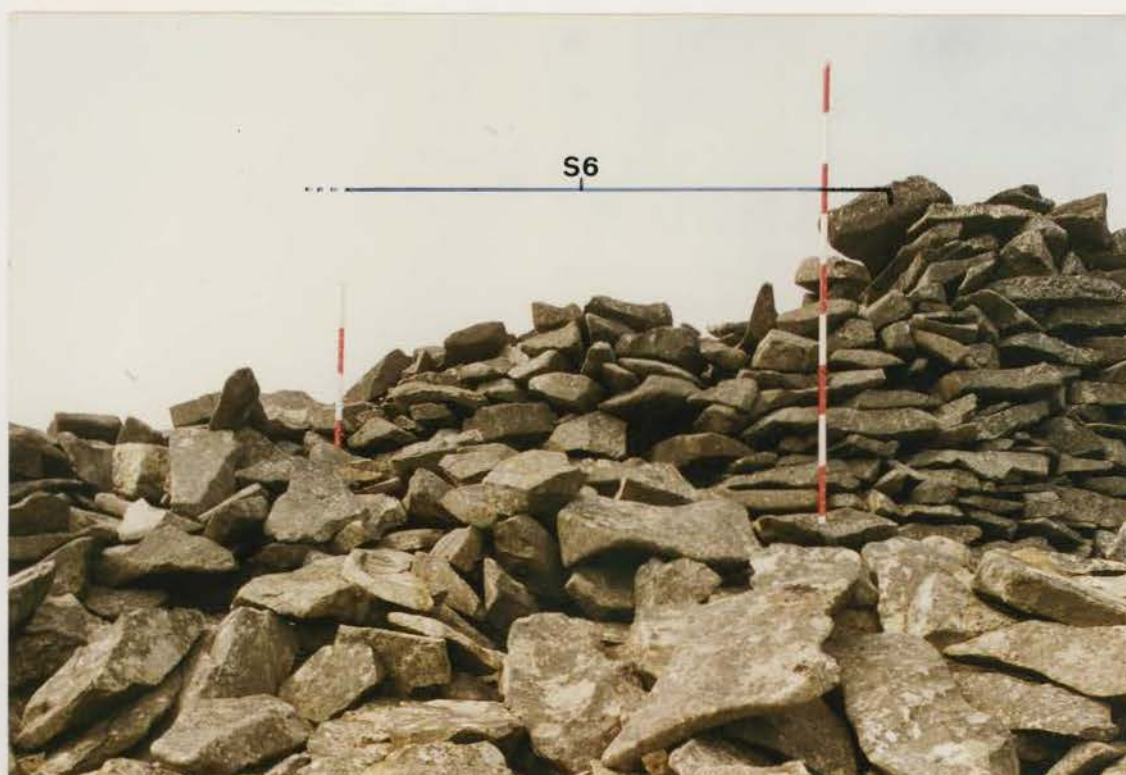
Plate 34 G1022/193/33 ; Collapse S6 before conservation.
