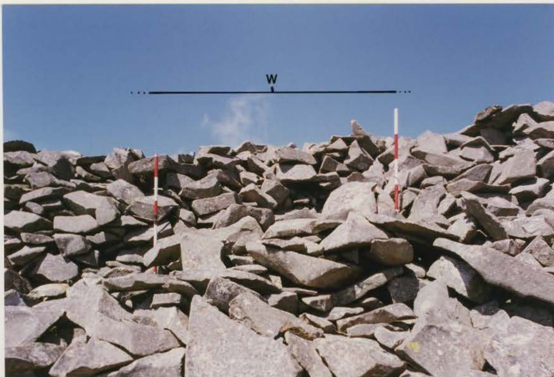
Plate 71 G1022/197/36 ; Collapse W before conservation.
