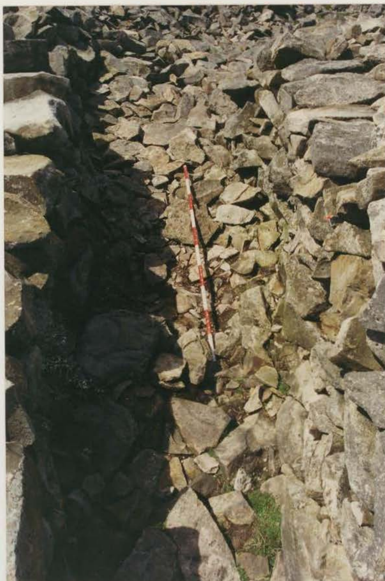
Plate 236 G1022/201/05; SW. entrance, showing erosion to passage floor.
