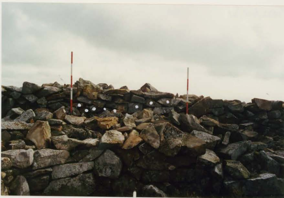
Plate 111 G1022/208/31 ; Collapse V4, after conservation.
