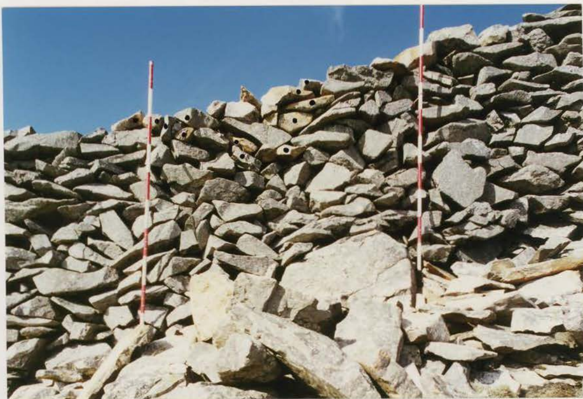
Plate 12 G1022/207/14 ; Collapse S3 after conservation.
