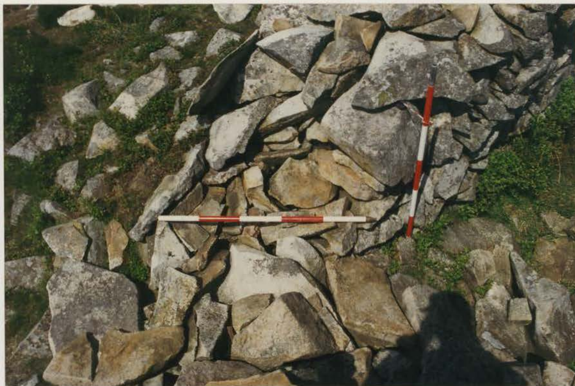
Plate 215 G1022/201/15 ; Collapse 9c before conservation.
