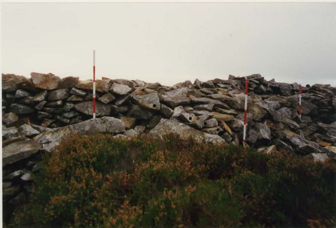
Plate 115 G1022/209/29 ; Collapse V5 after conservation.
