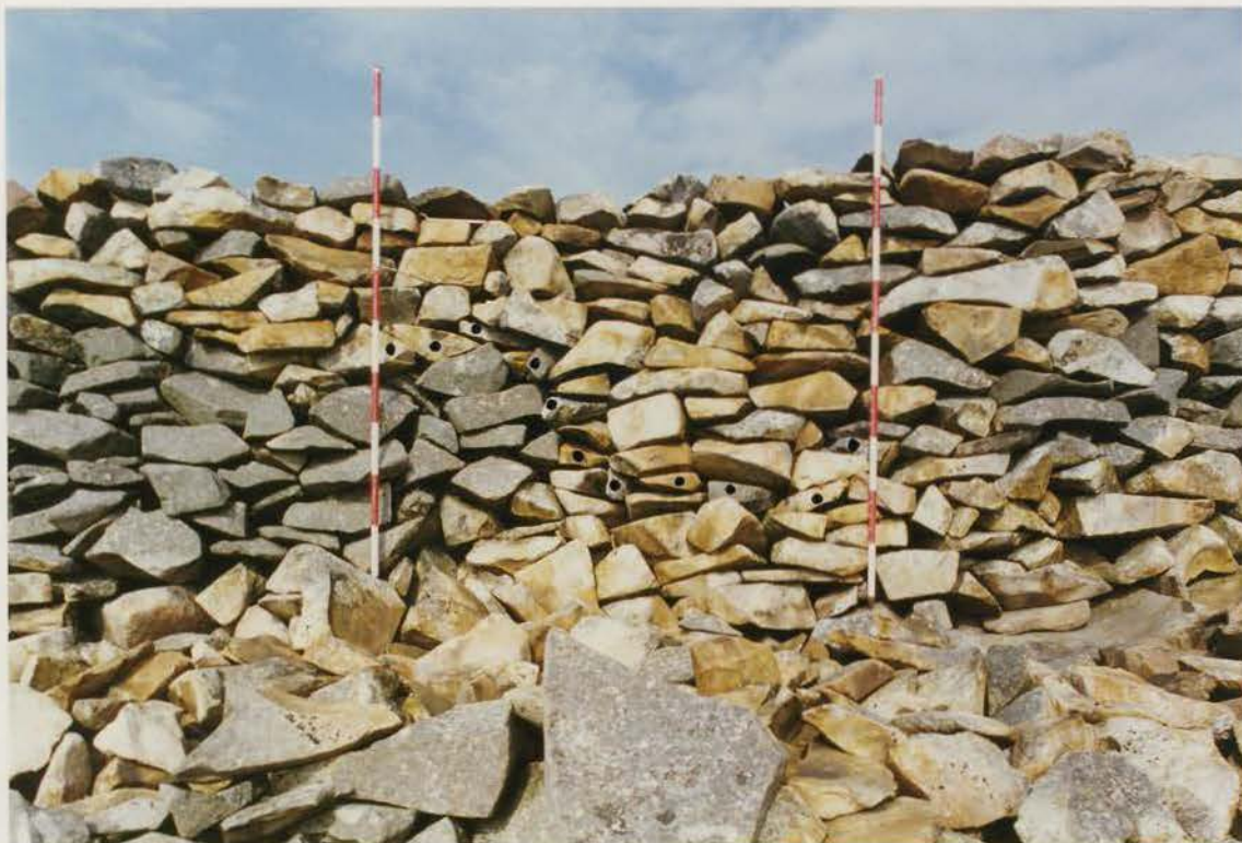
Plate 75 G1022/210/16 ; Collapse W after conservation.
