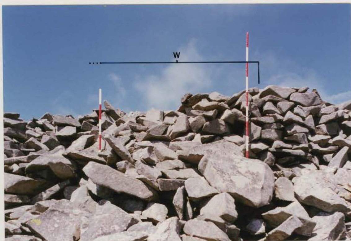
Plate 70 G1022/197/34 ; Collapse W before conservation.
