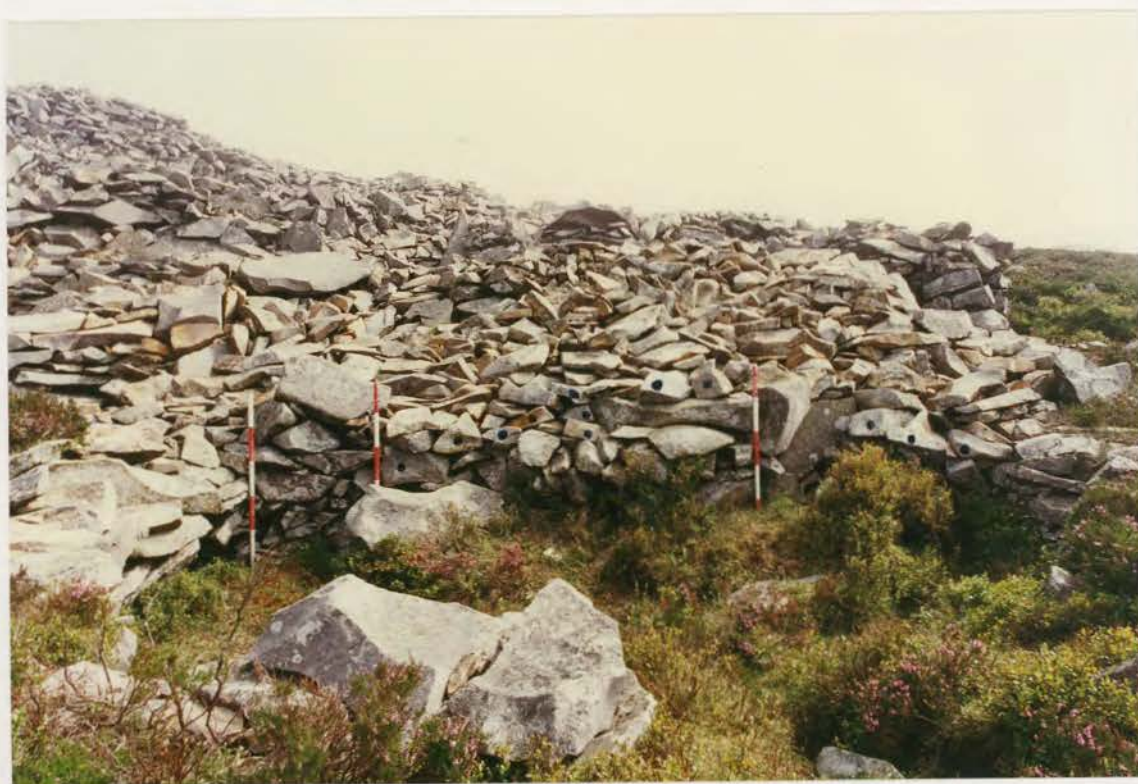
Plate 32. G1022\242\22, collapse 25b after conservation.
