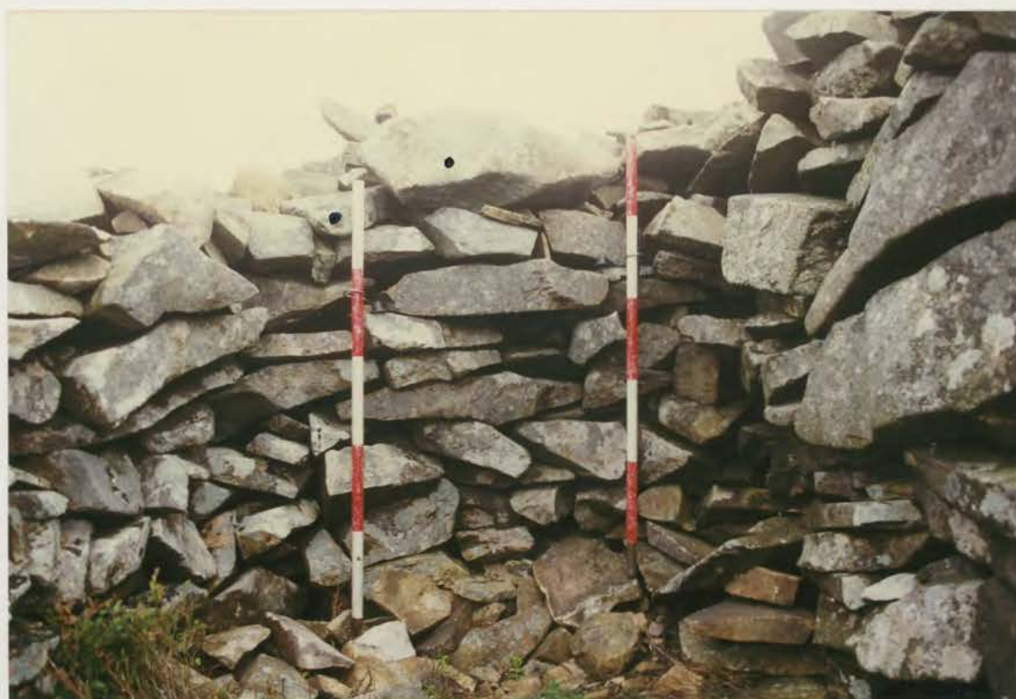
Plate 250. G1022\247\19, collapse 12b after conservation.
