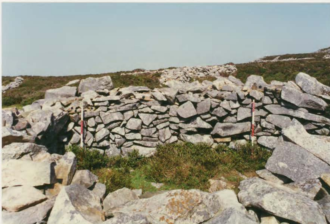
Plate 167. G1022\245\16A, collapse 16d after conservation.
