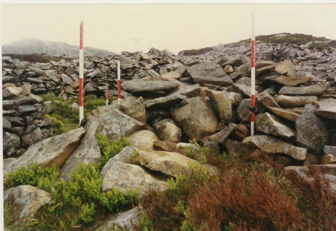
Plate 202. G1022\225\09, collapse 8i before conservation, outer face.
