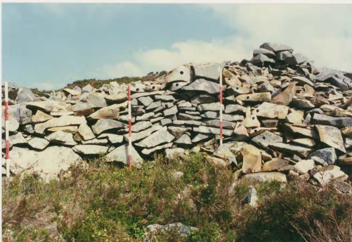
Plate 105. G1022\244\05, collapse 21c after conservation.
