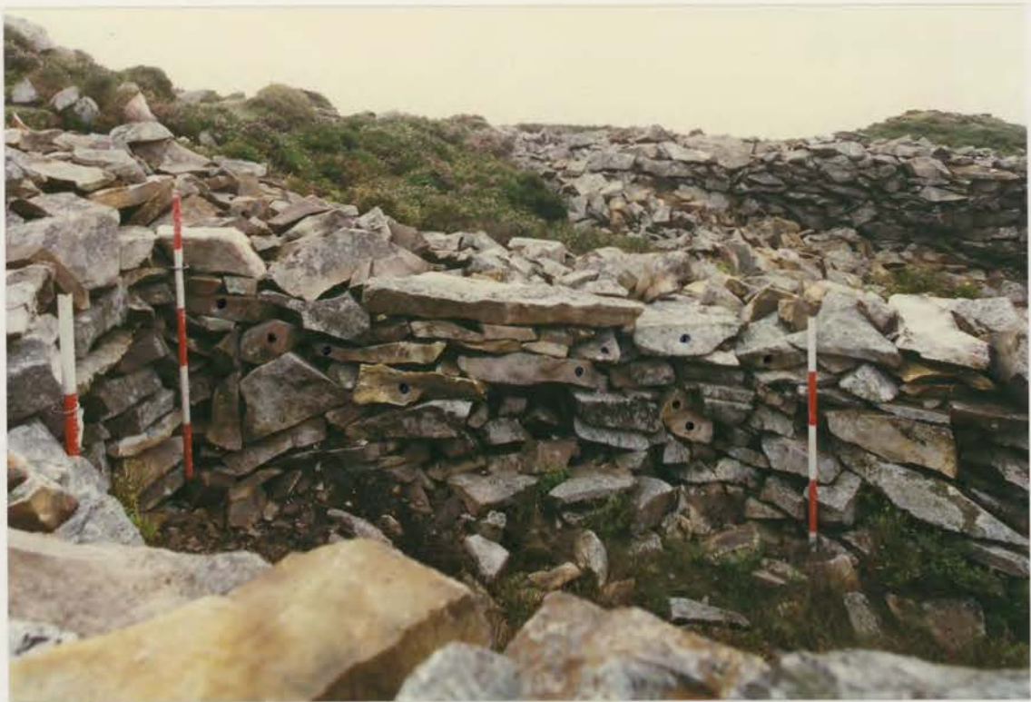
Plate 267. G1022\247\34, collapse 13c after conservation.
