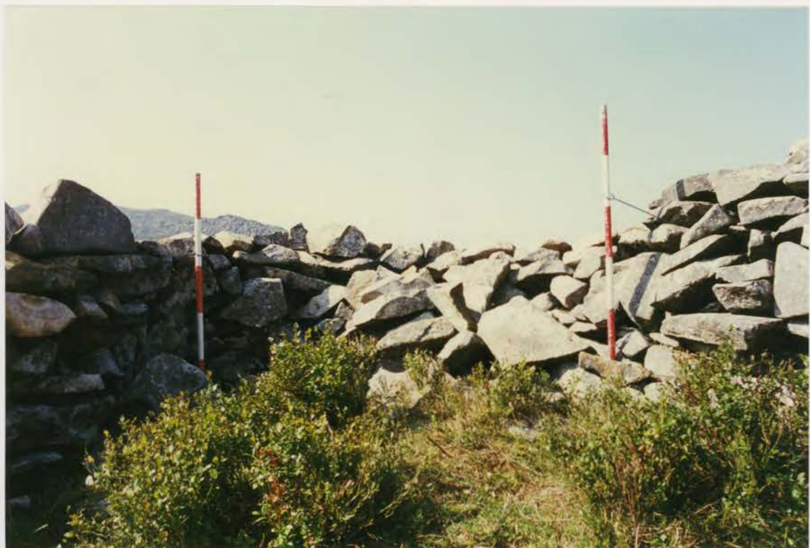
Plate 186. G1022\245\30A, collapse 8c before conservation.
