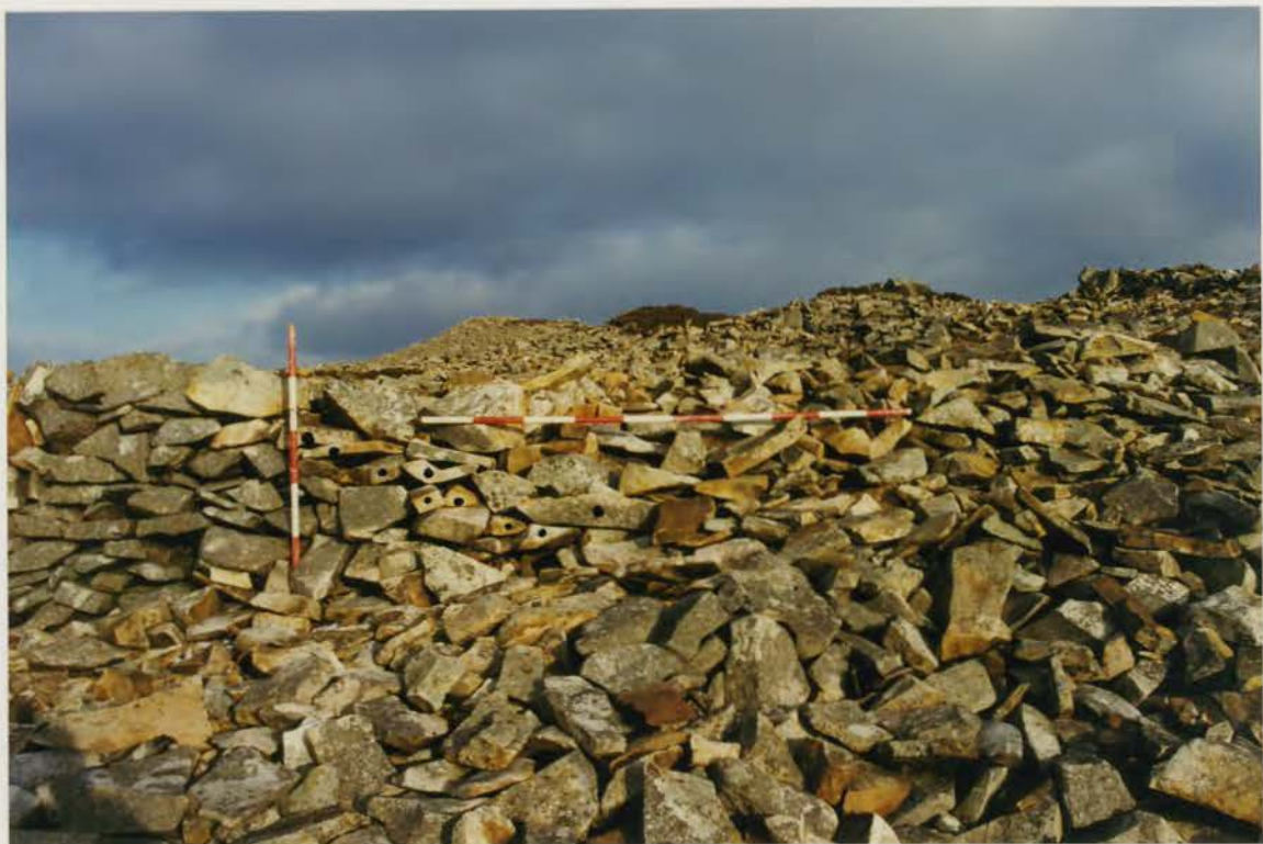
Plate 354. G1022\252\25, collapse 60 after conservation.
