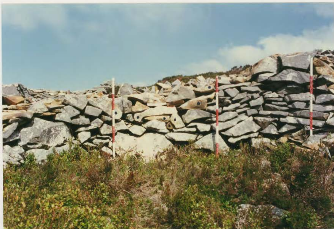
Plate 103. G1022\244\04, collapse 21b after conservation.
