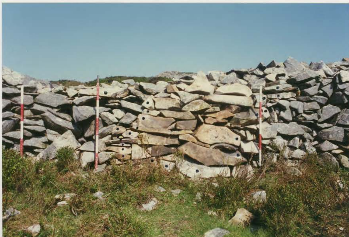
Plate 190. G1022\245\34A, collapse 8e after conservation.
