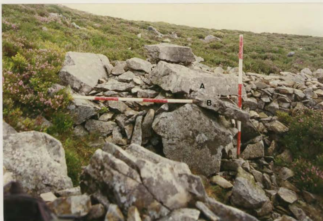
Plate 428. G1022\241\21, collapse 28a before conservation.
