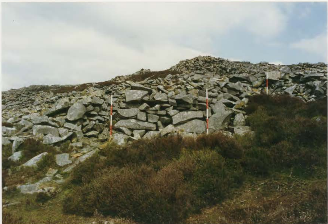
Plate 18. G1022\215\30, collapse 24h before conservation.
