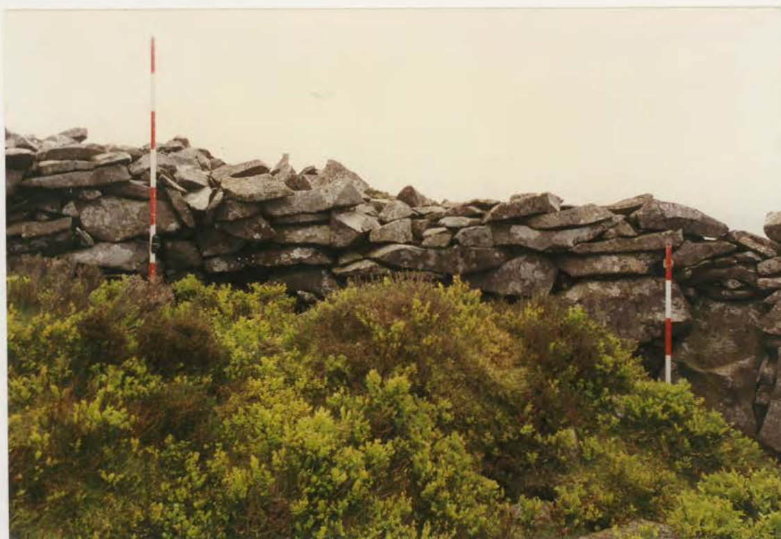
Plate 180. G1022\224\02, collapses 79d and c before conservation.
