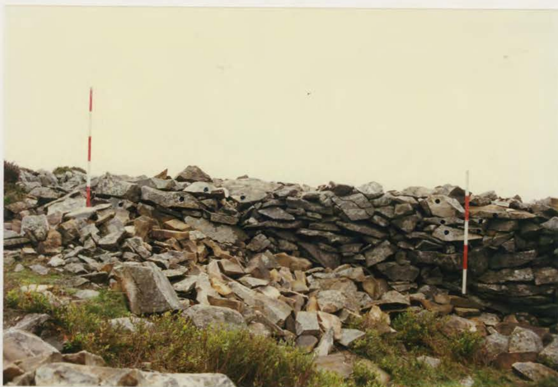
Plate 276. G1022\248\11, collapse 14b after conservation.
