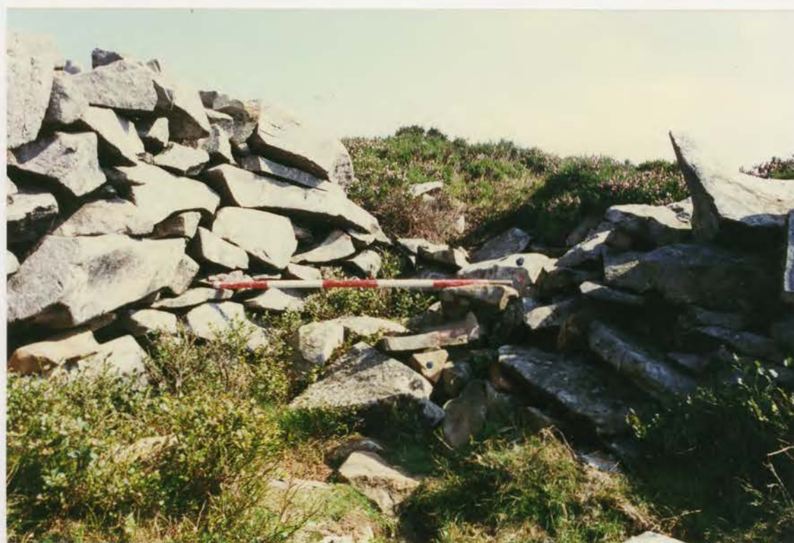
Plate 160. G1022\245\18A, collapse 16a after conservation.
