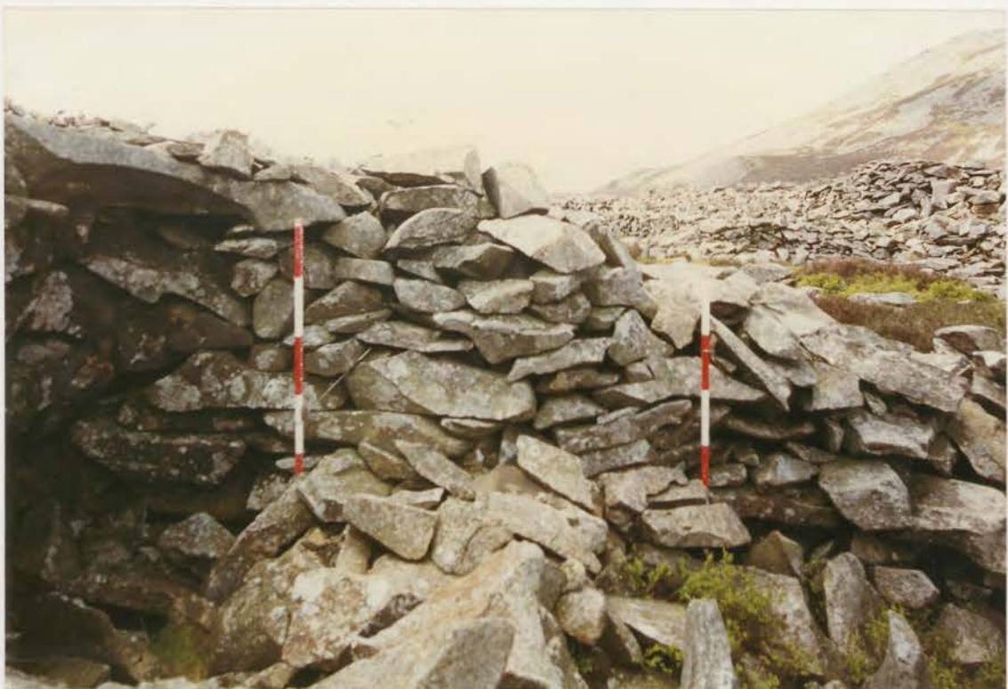
Plate 42. G1022\216\28, collapse 26d before conservation.
