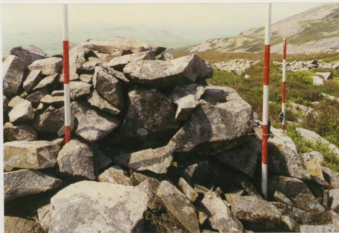
Plate 348. G1022\231\07, collapse 6m before conservation.
