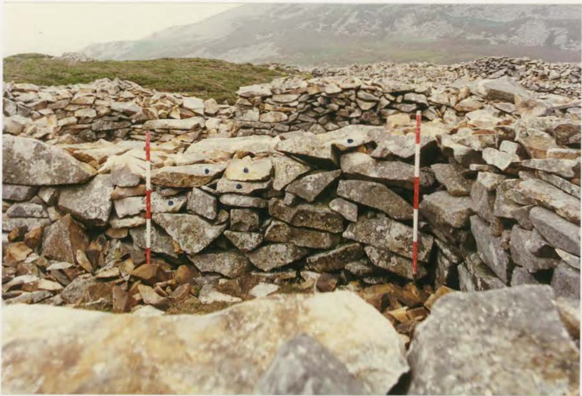
Plate 77. G1022\243\29, collapse 22c after conservation.
