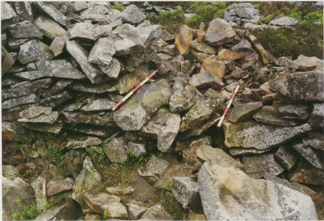
Plate 45. G1022\225\27, collapse 26c after partial clearance.
