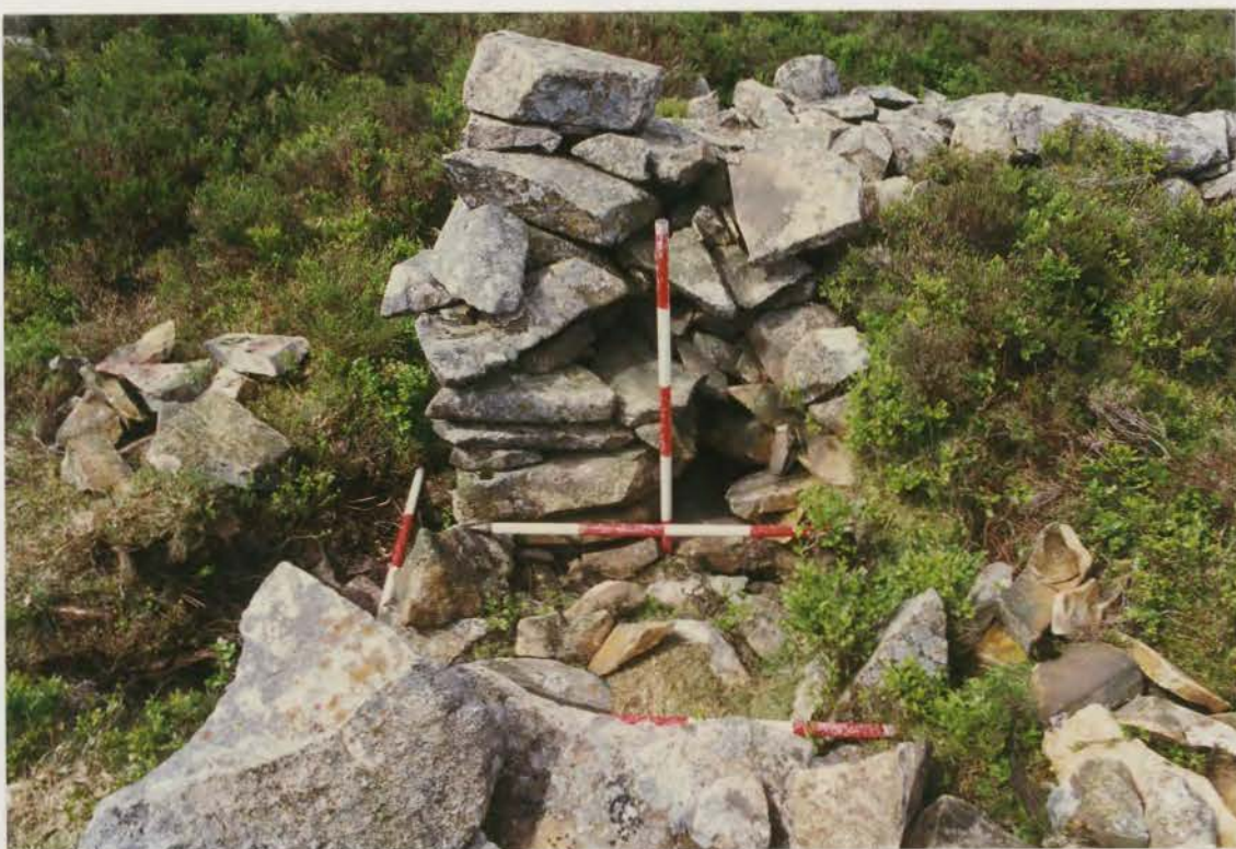
Plate 128. G1022\235\17, collapse 18a before conservation.
