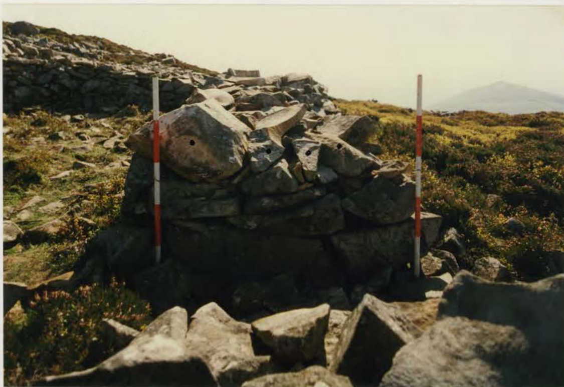
Plate 391. G1022\251\16, collapse 36b after conservation.
