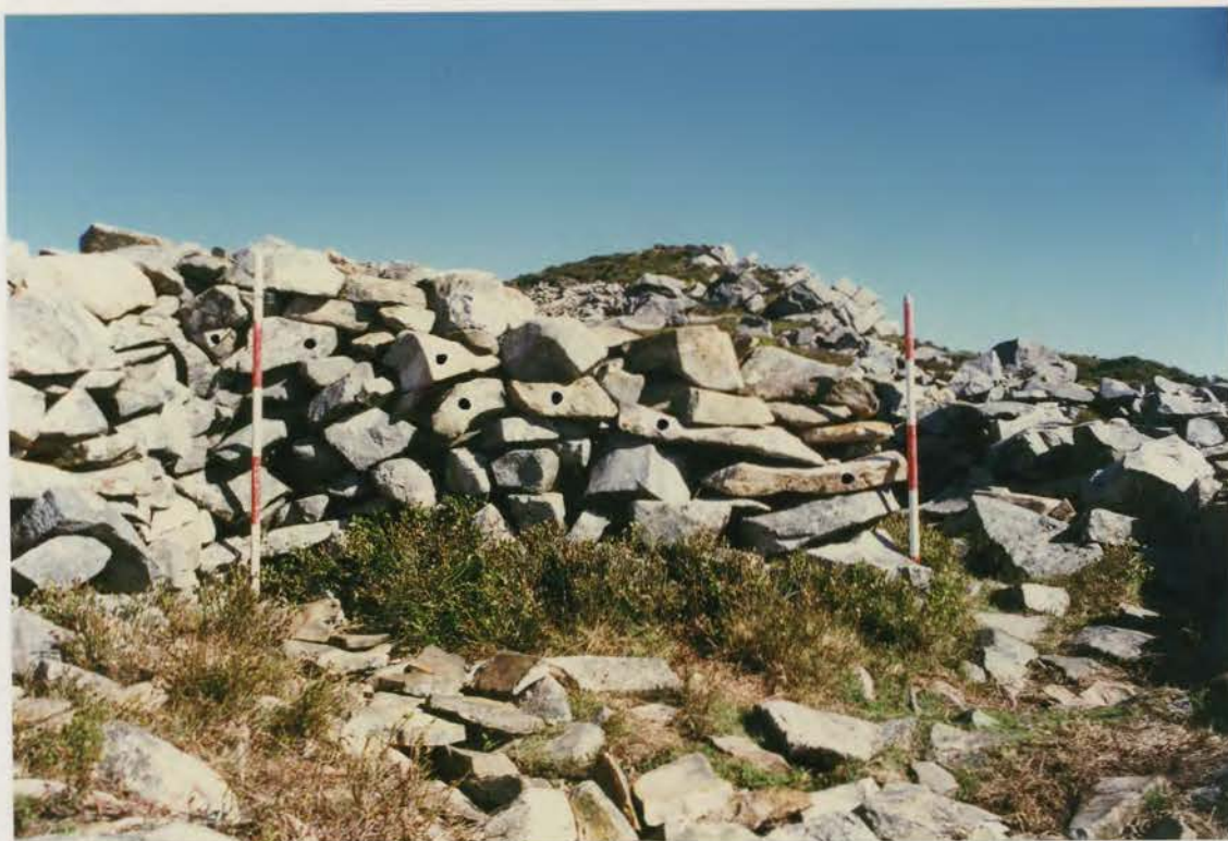
Plate 409. G1022\250\35, collapse 53b after conservation.
