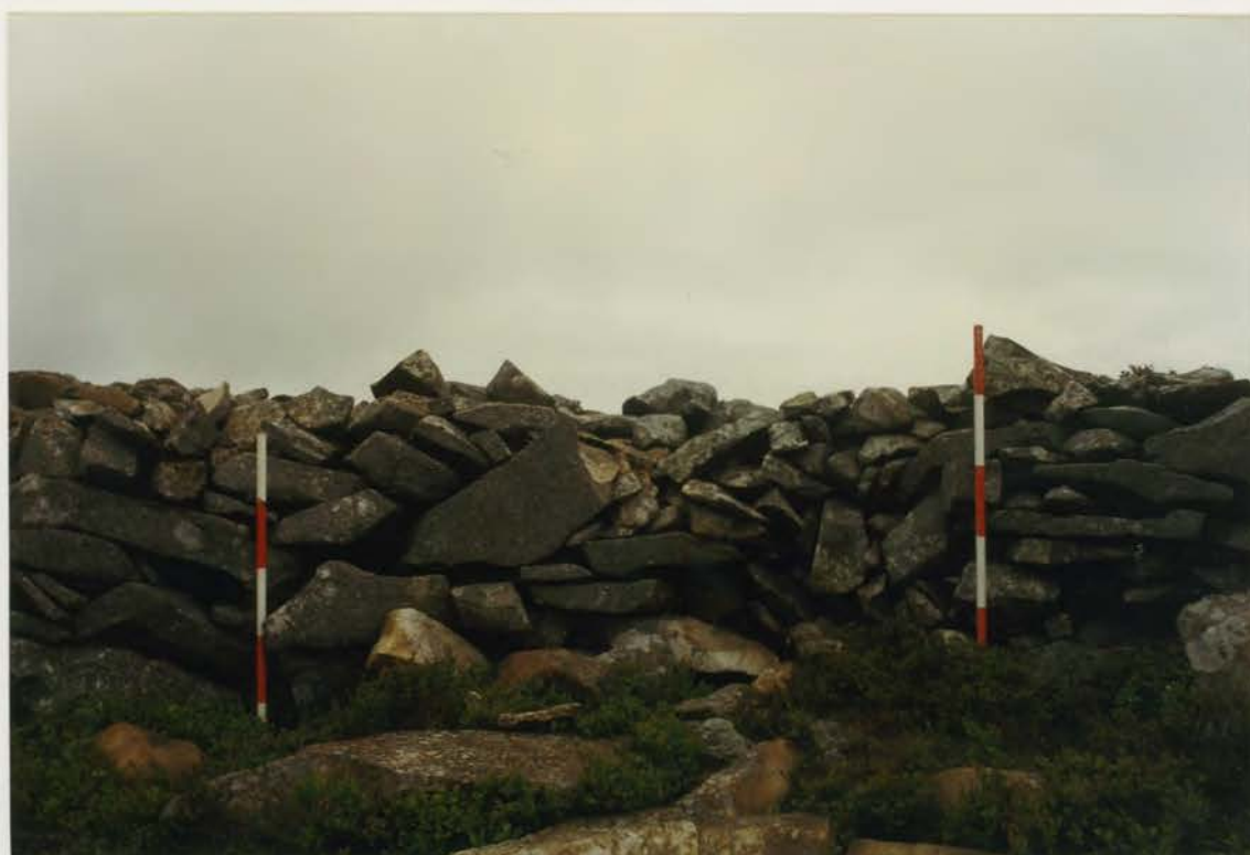
Plate 108. G1022\221\07, collapses 19a and b before conservation.
