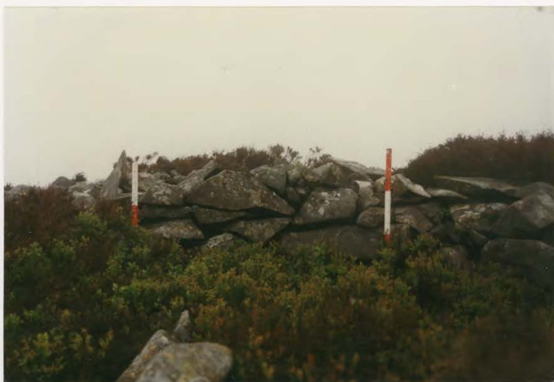
Plate 136. G1022\222\04, collapse 18b before conservation.
