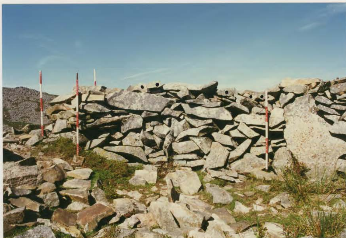
Plate 218. G1022\246\16, collapse 7b after conservation.
