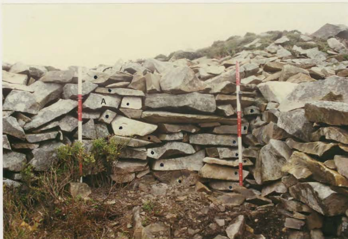
Plate 263. G1022\247\32, collapse 13b after conservation.
