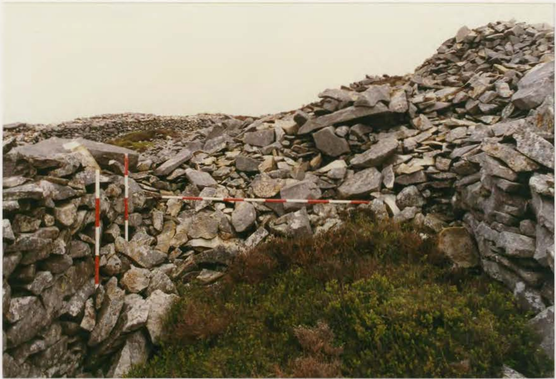
Plate 55. G1022\218\10A collapse 23c before conservation.
