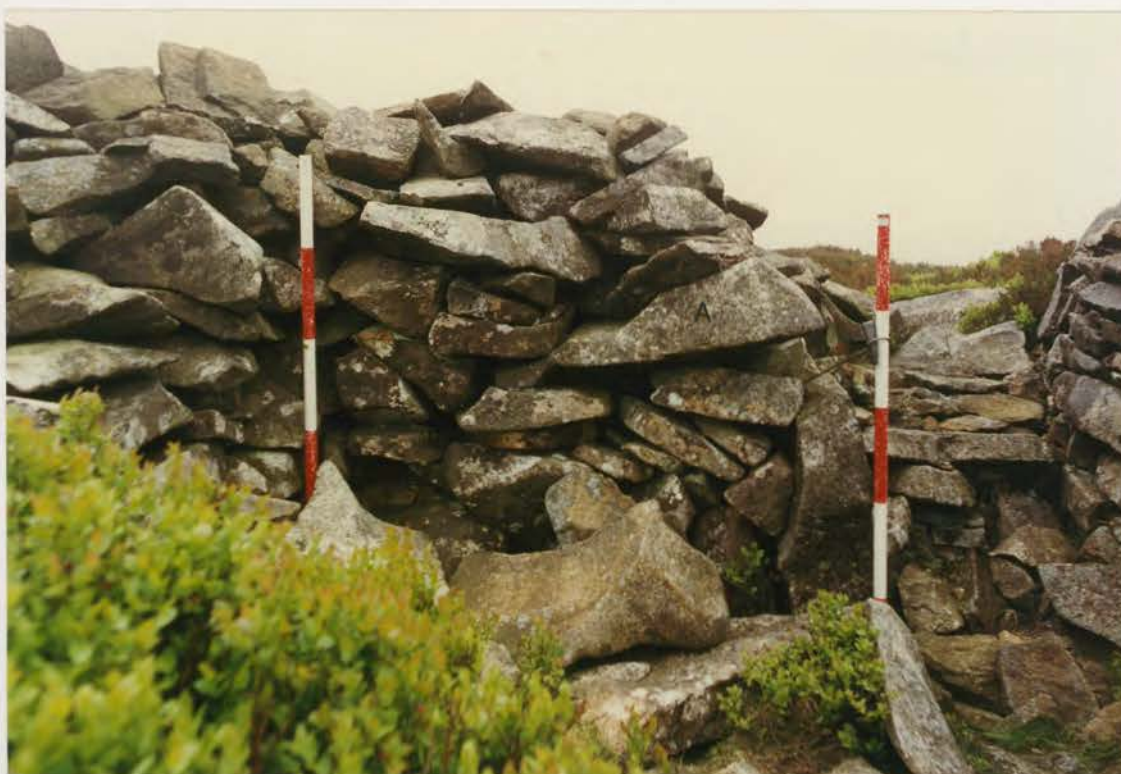
Plate 198. G1022\225\03, collapse 8i before conservation.
