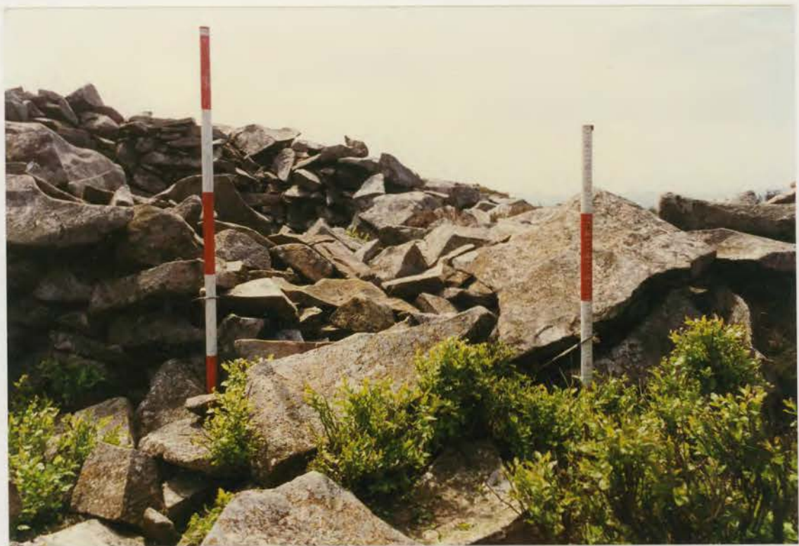
Plate 239. G1022\226\17, collapse 11d before conservation.
