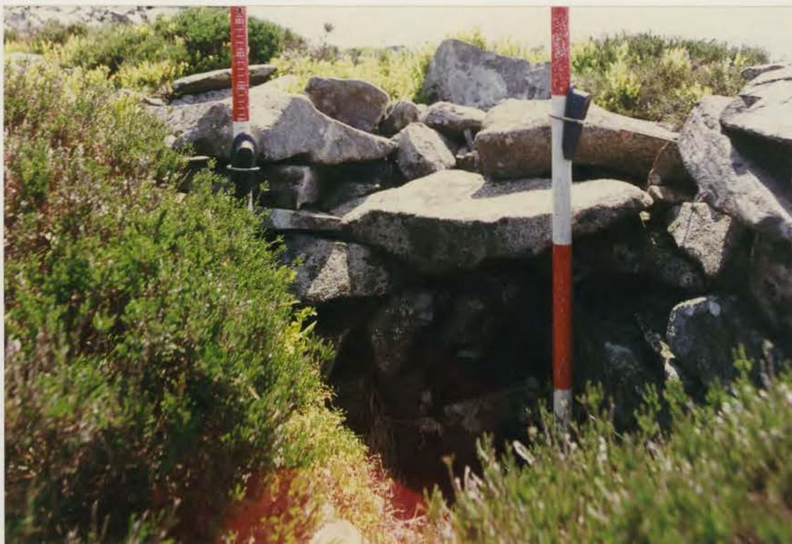
Plate 367. G1022\232\19A, collapse 44a before conservation.
