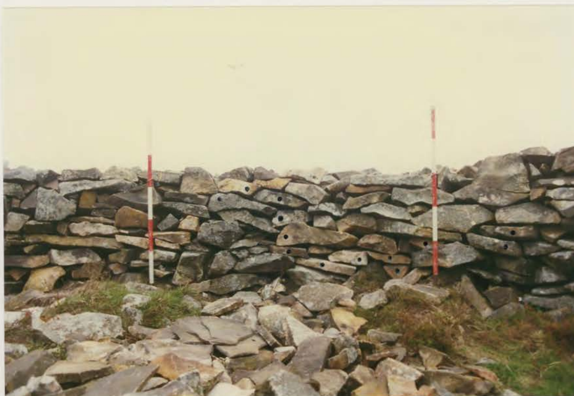
Plate 314. G1022\248\36, collapses 5g and h after conservation.
