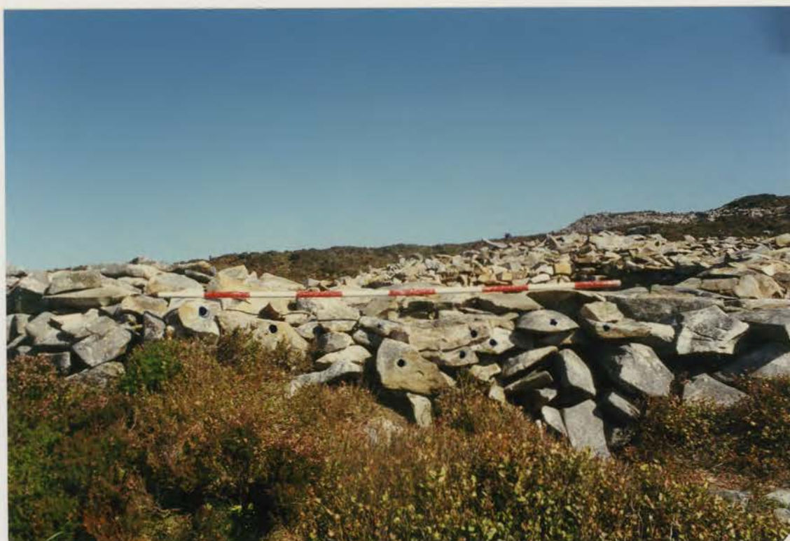
Plate 392. G1022\251\17, collapse 36c after conservation.
