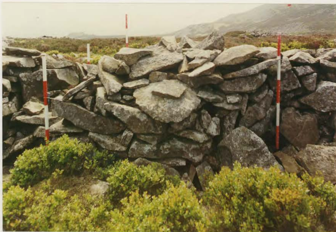
Plate 205. G1022\205\20, collapse 8a before conservation.
