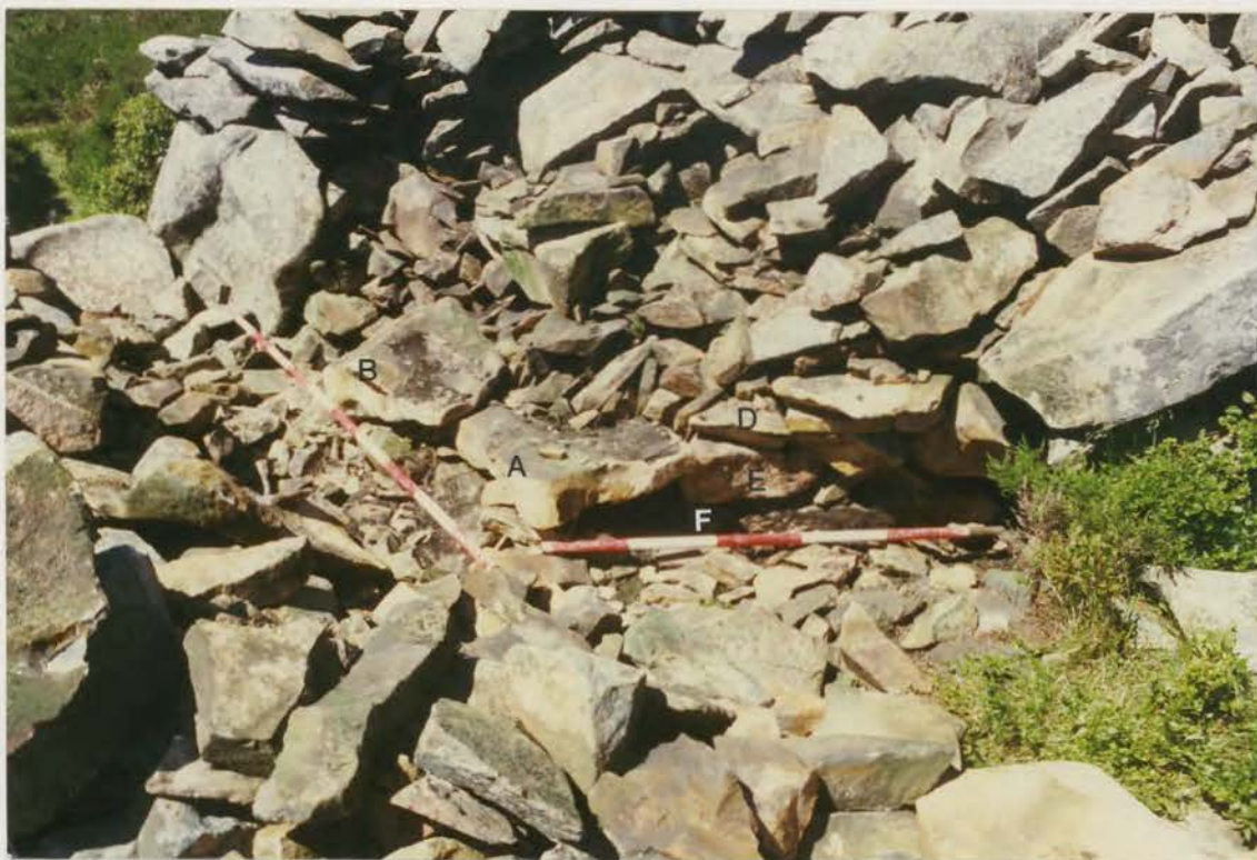
Plate 293. G1022\237\35, collapse 5b after conservation.
