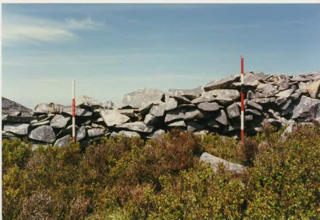
Plate 98. G1022\219\27, collapse 21a before conservation.
