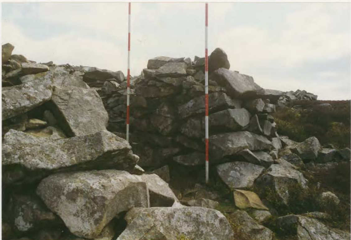
Plate 16. G1022\215\02, collapse 24a before conservation.
