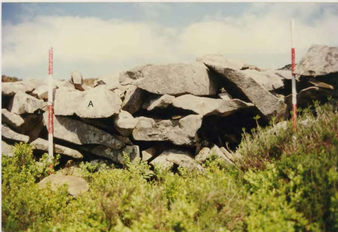
Plate 373. G1022\233\03, collapse 40a before conservation.
