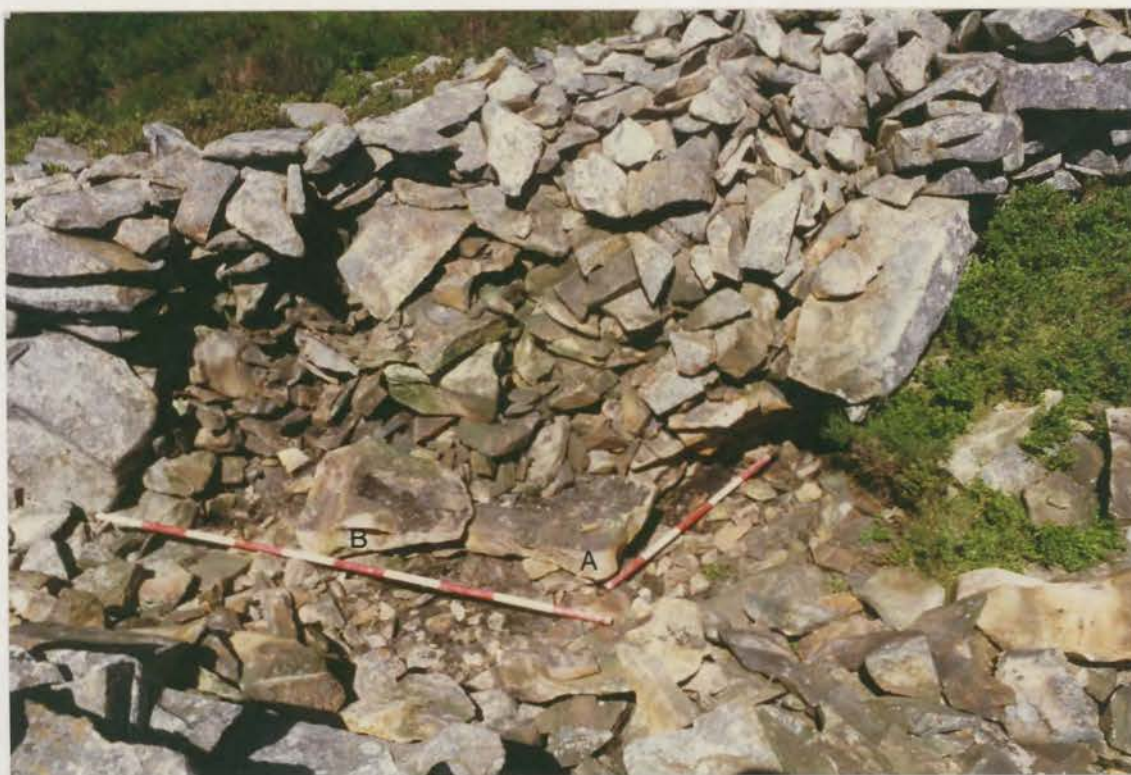
Plate 292. G1022\237\33, collapse 5b after conservation.
