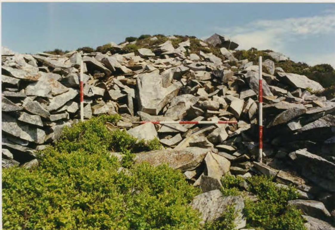
Plate 261. G1022\227\15, collapse 13b before conservation.
