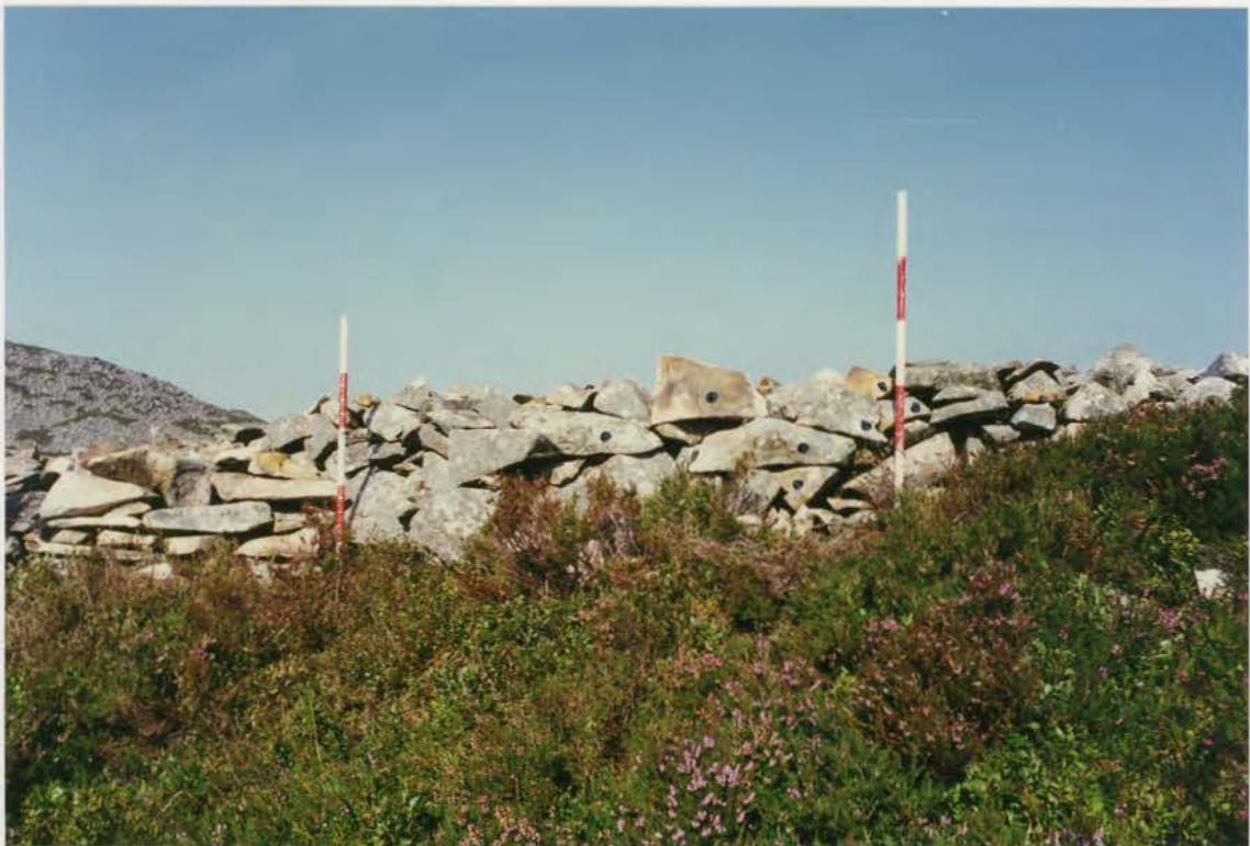
Plate 158. G1022\245\20A, collapse 95c after conservation.
