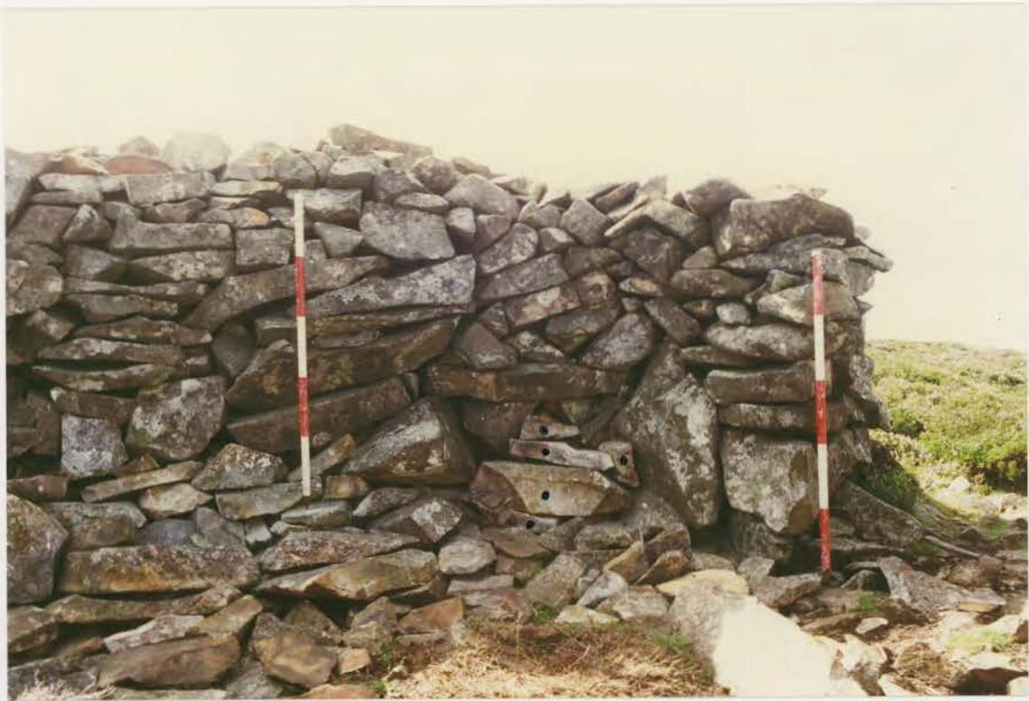
Plate 15. G1022\242\12, collapse 24b after conservation.
