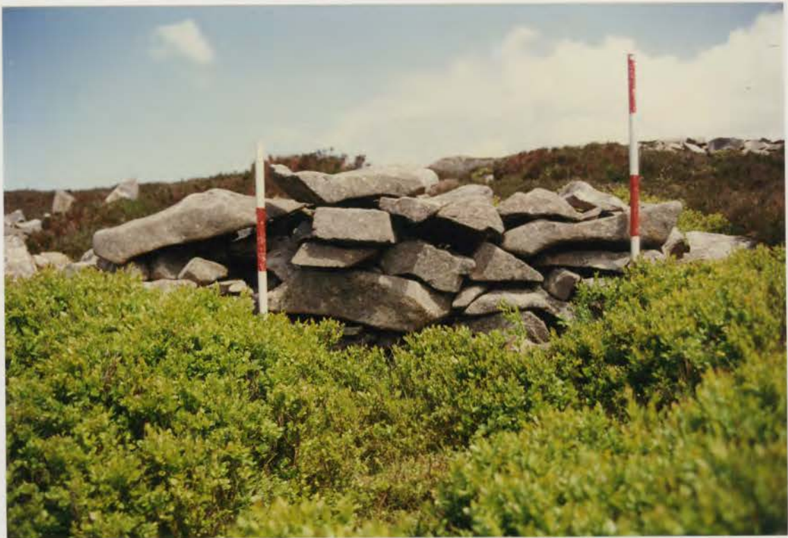
Plate 371. G1022\232\28A, collapse 44d before conservation.
