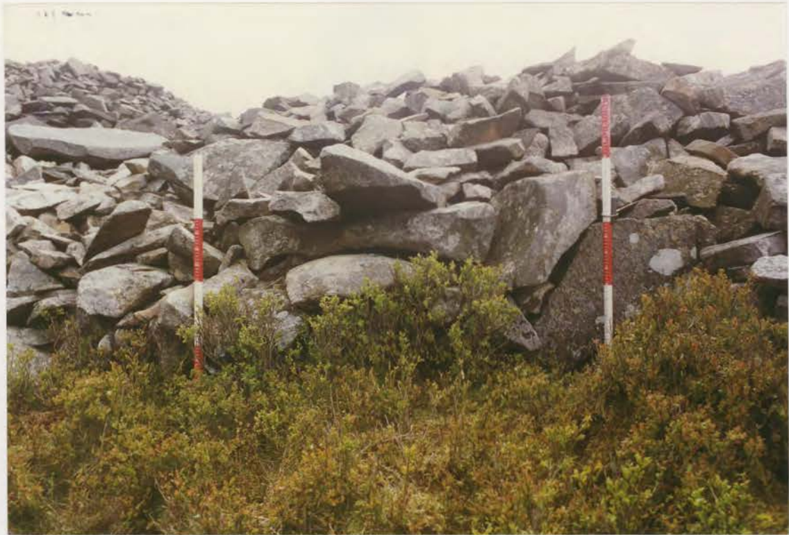
Plate 29. G1022\216\11, collapse 25b before conservation.
