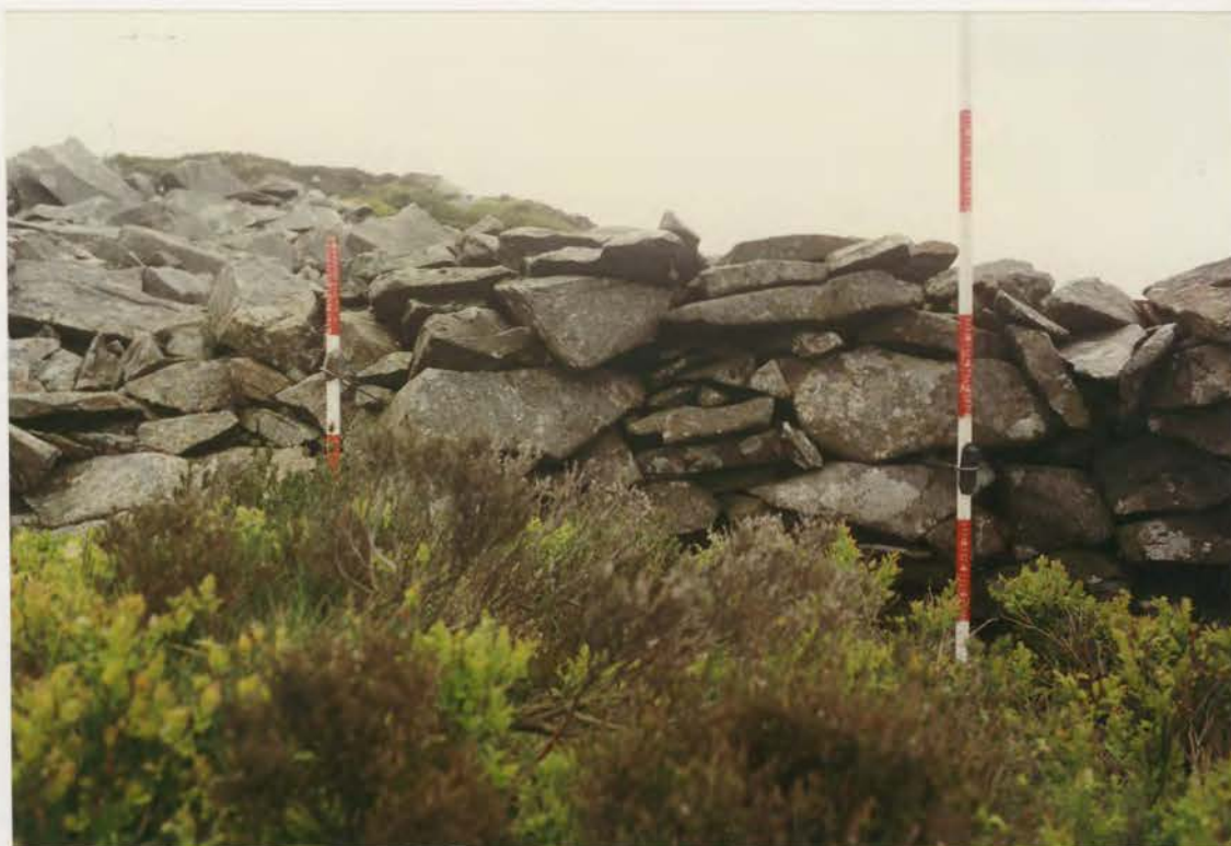
Plate 179. G1022\223\36, collapse 79d before conservation.
