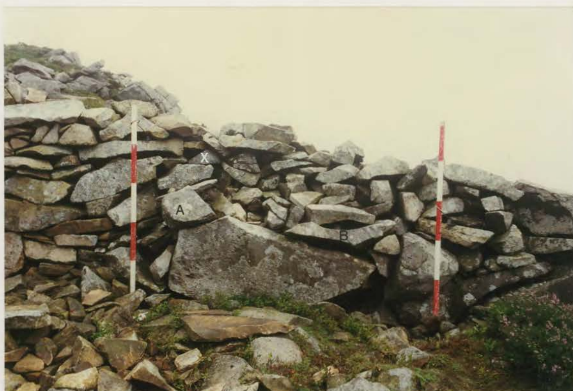
Plate 418. G1022\240\23, collapse 90d before conservation.
