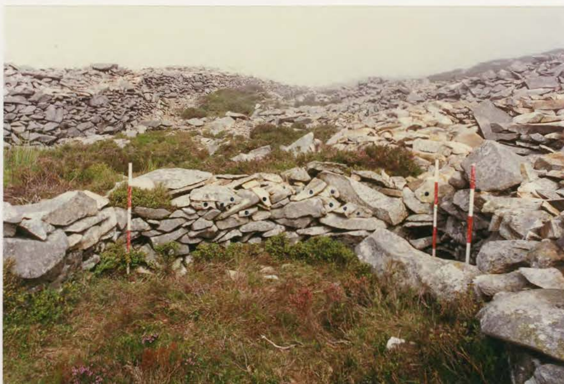
Plate 28. G1022\242\20, collapse 25c after conservation.
