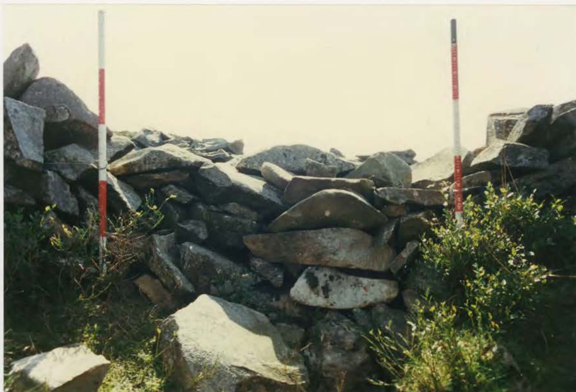
Plate 165. G1022\245\13A, collapse 16b after conservation.
