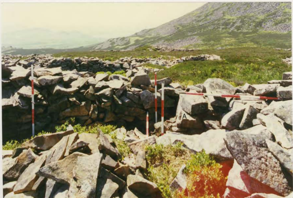
Plate 174. G1022\236\15, collapse 15b after clearance.
