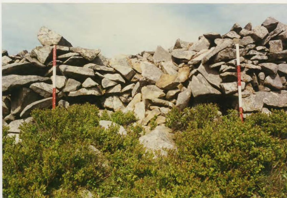
Plate 188. G1022\224\30, collapse 8e before conservation.
