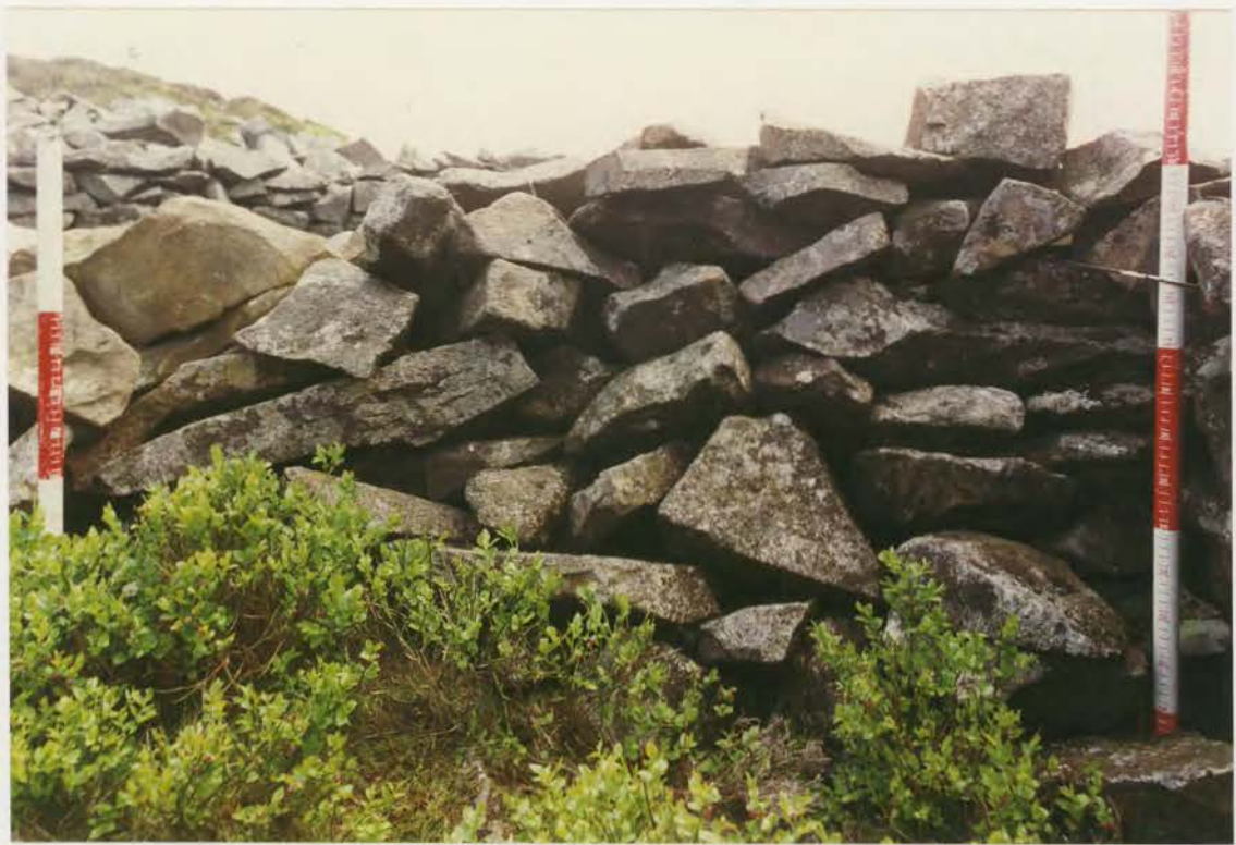
Plate 163. G1022\223\16, collapse 16b before conservation.
