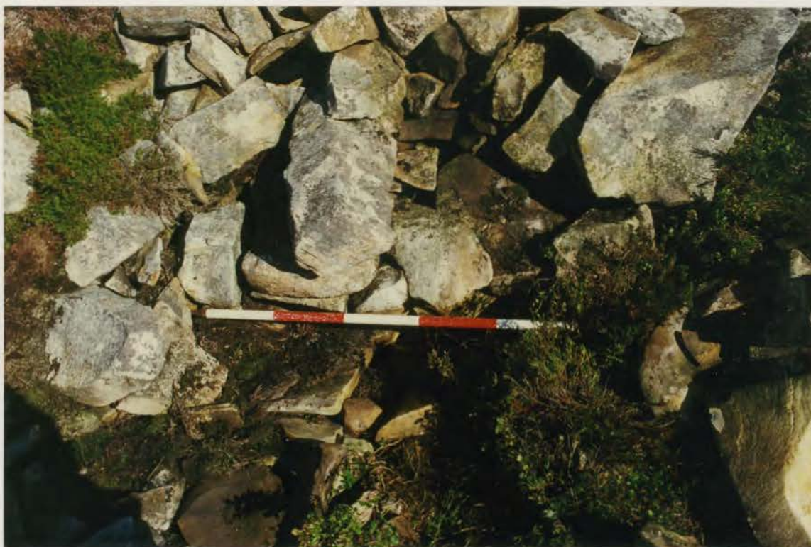
Plate 365. G1022\239\08, collapse 74g after clearance.
