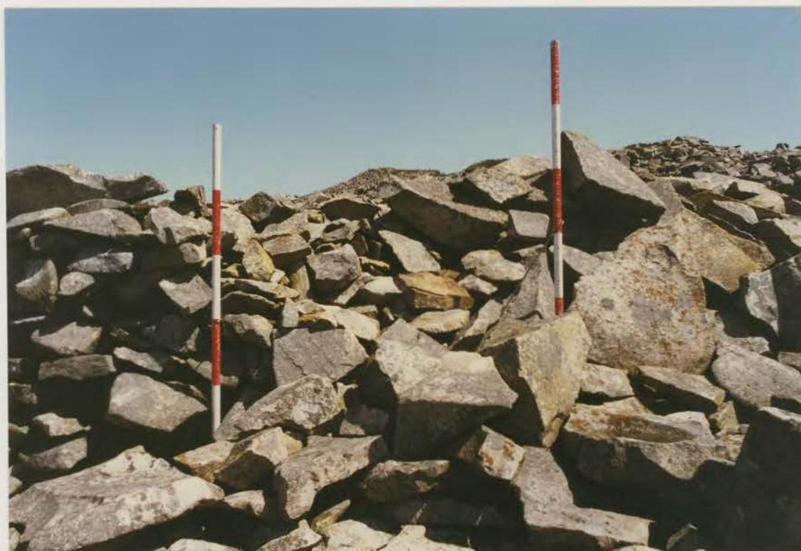
Plate 352. G1022\231\12, collapse 6o before conservation.
