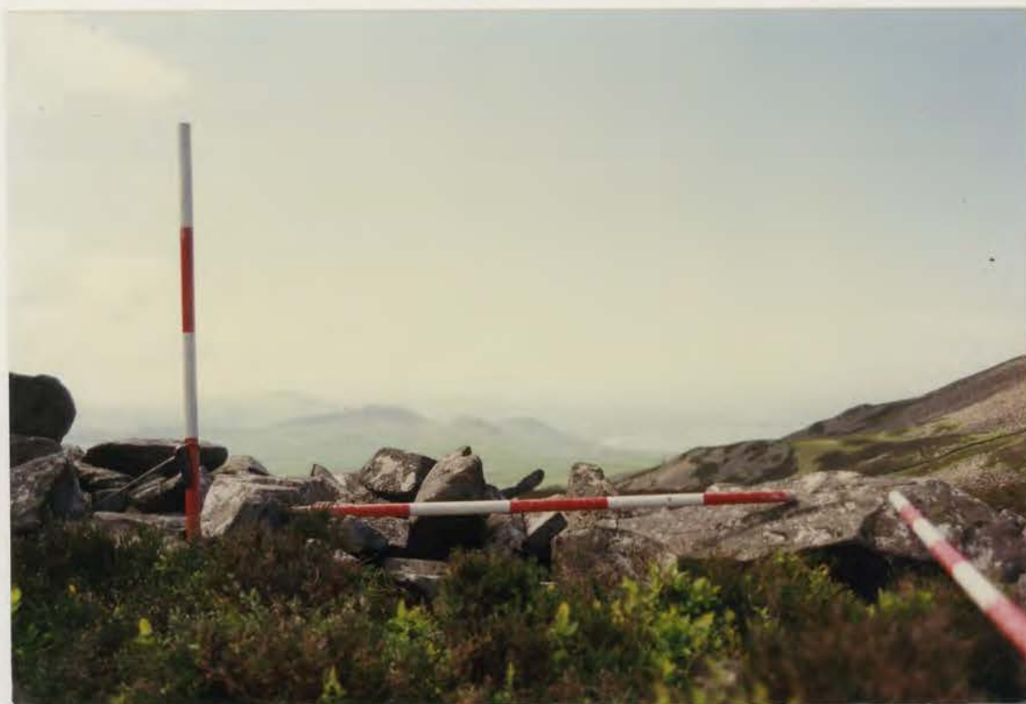
Plate 369. G1022\232\24A, collapses 44b and c before conservation.
