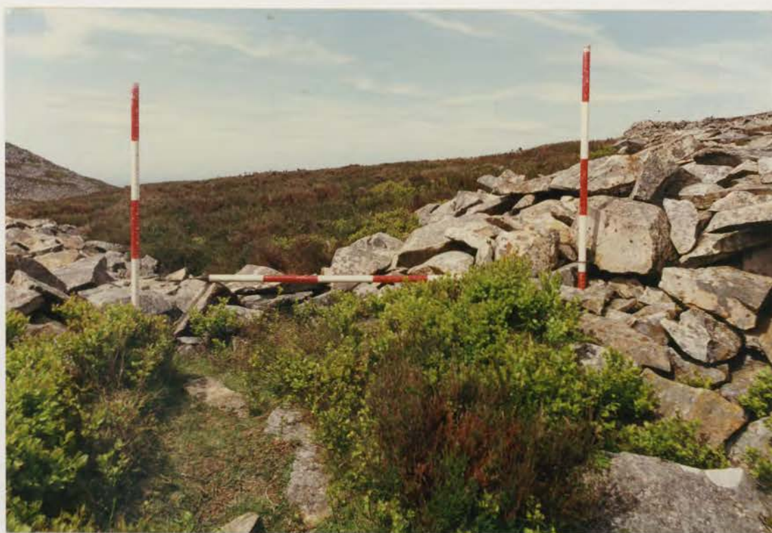
Plate 280. G1022\228\34, collapse 14d before conservation.
