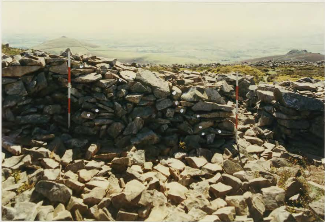
Plate 401. G1022\250\30, collapse 89b after conservation.
