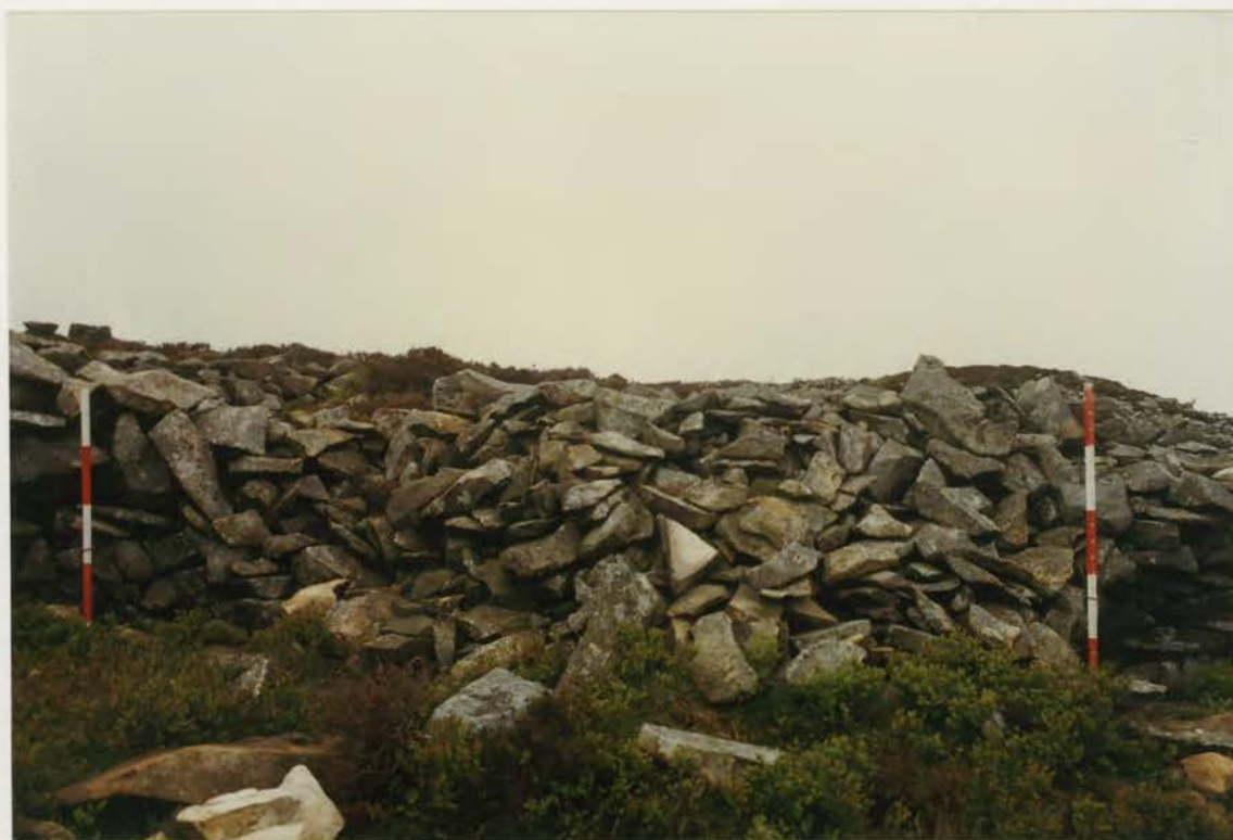
Plate 115. G1022\221\10, collapse 19d before conservation.
