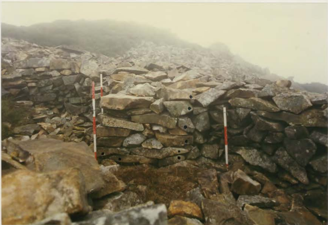
Plate 342. G1022\249\22, collapse 6j after conservation.
