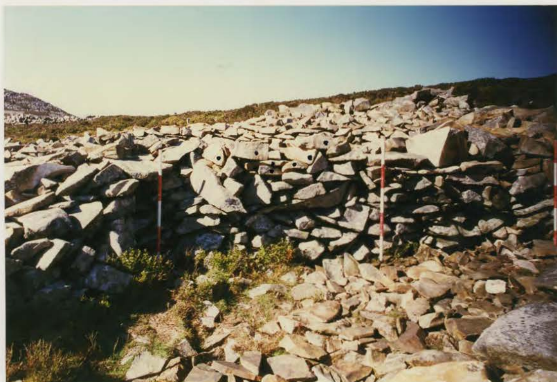
Plate 416. G1022\251\05, collapse 90c after conservation.
