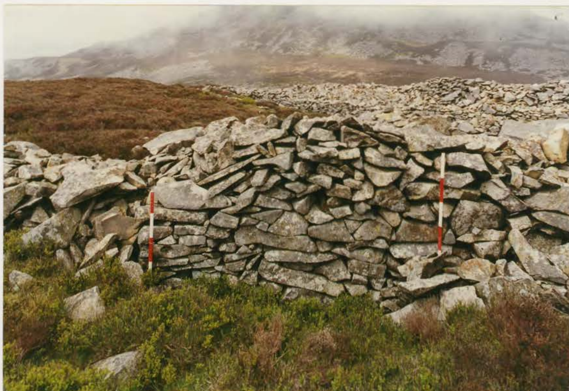
Plate 53. G1022\218\05A, collapse 23a before conservation.
