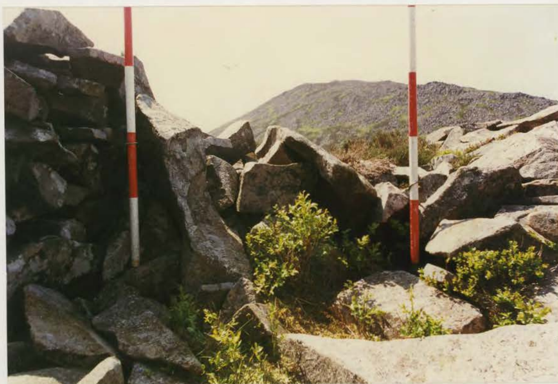
Plate 254. G1022\227\03, collapse 12d before conservation.
