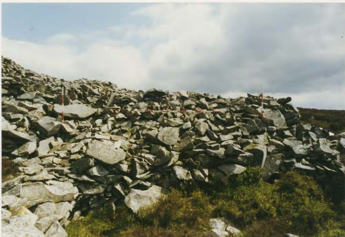
Plate 31. G1022\215\24, collapse 25b before conservation.
