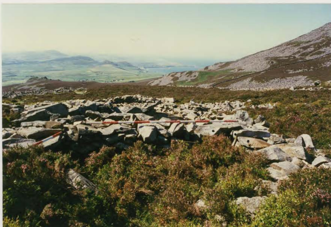
Plate 370. G1022\250\13, collapses 44b and c after conservation.
