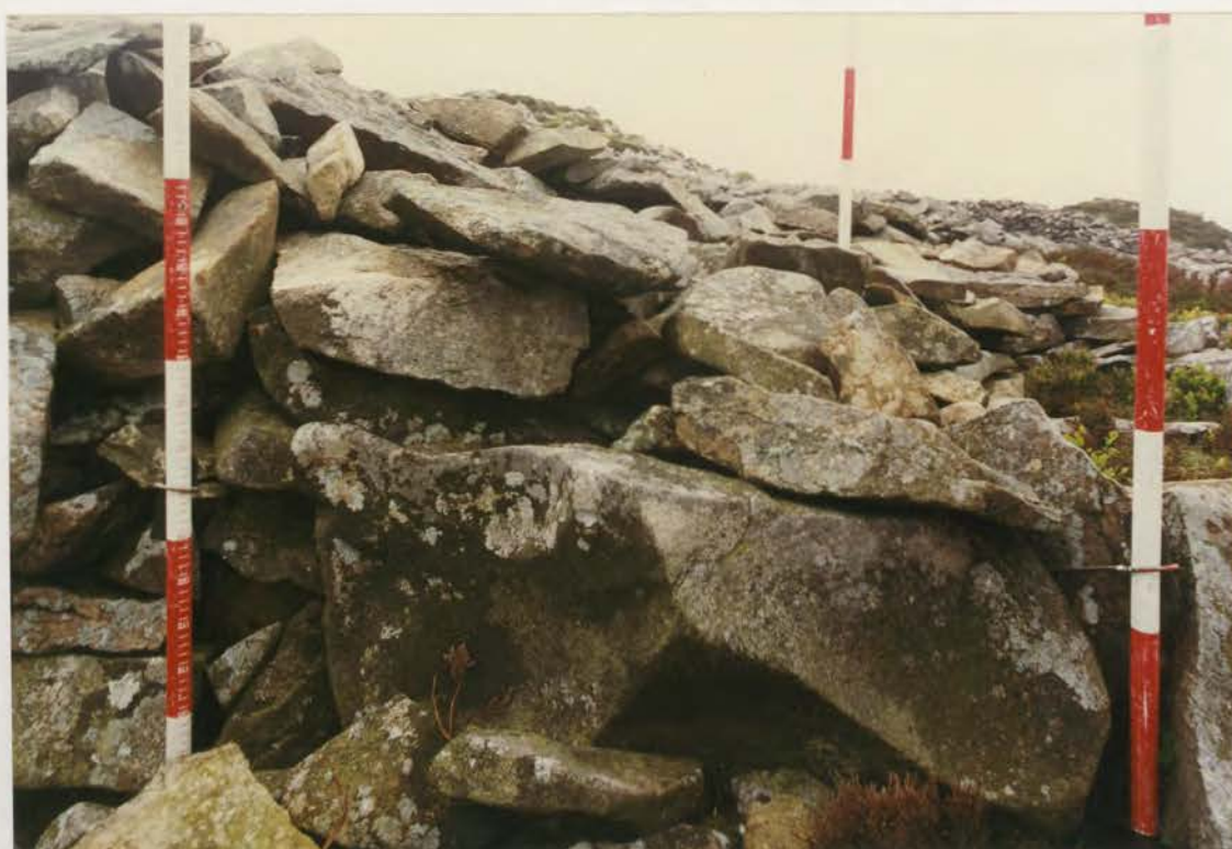
Plate 200. G1022\225\07, collapse 8i before conservation.
