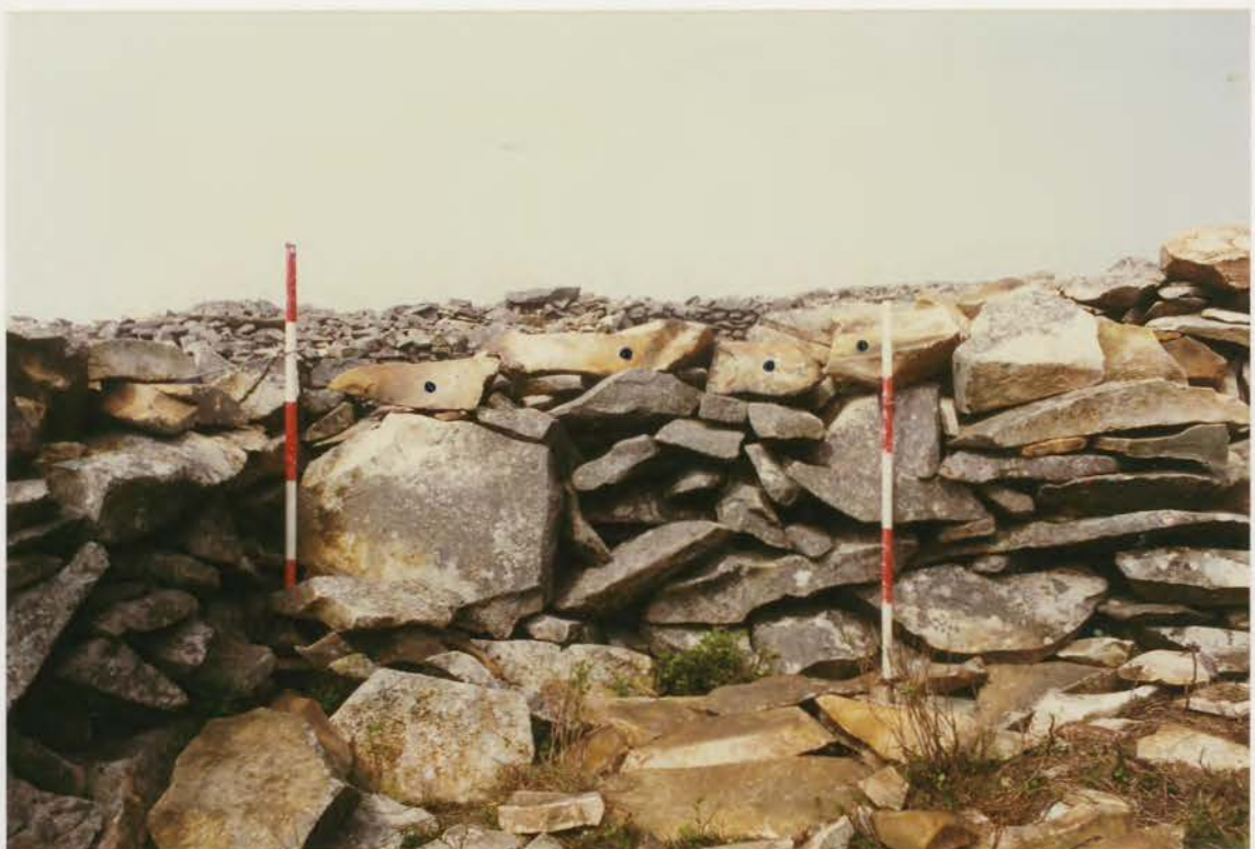
Plate 52. G1022\242\24, collapse 26b after conservation.
