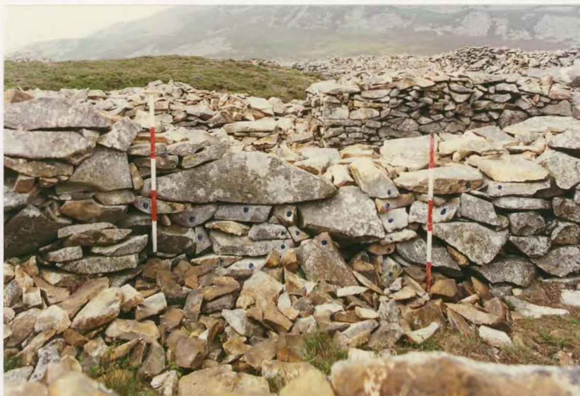
Plate 75. G1022\243\27, collapse 22b after conservation.
