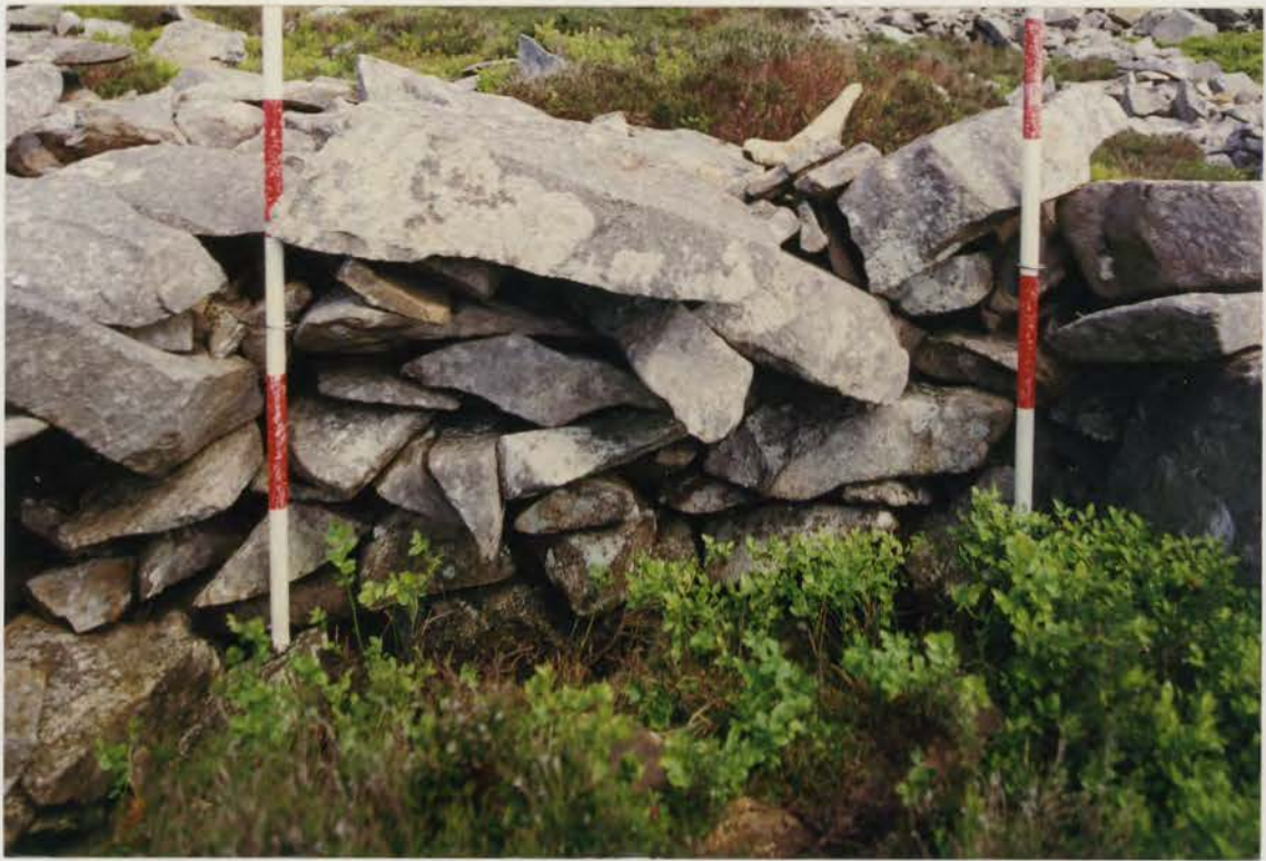
Plate 375. G1022\233\08, collapse 40b before conservation.
