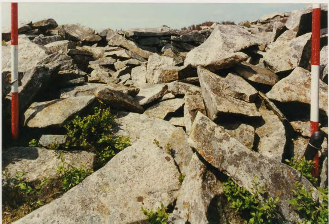
Plate 246. G1022\227\00, collapse 12e before conservation.
