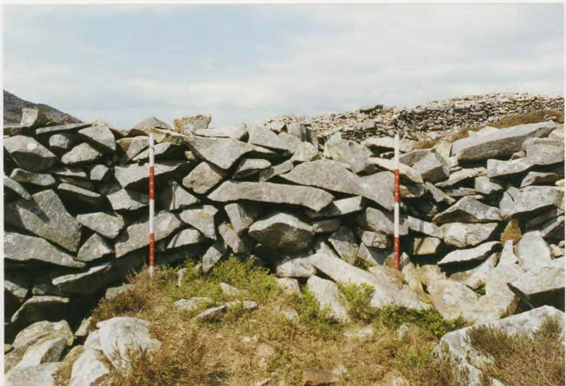
Plate 04. G1022\215\16, collapse 24e before conservation.
