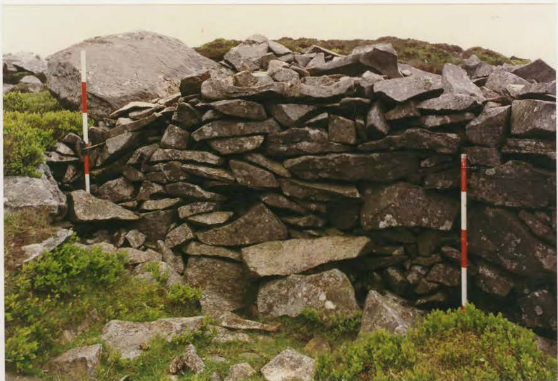
Plate 168. G1022\233\02, collapse 15a before conservation.
