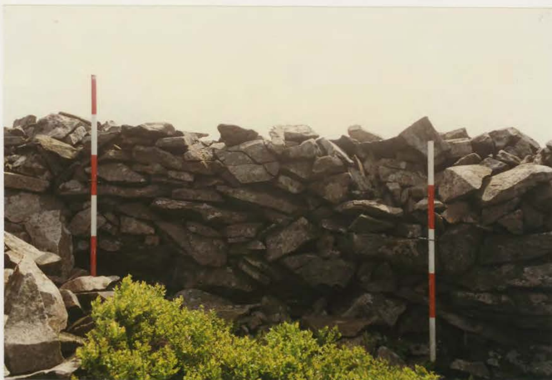
Plate 273. G1022\228\25, collapse 14b before conservation.
