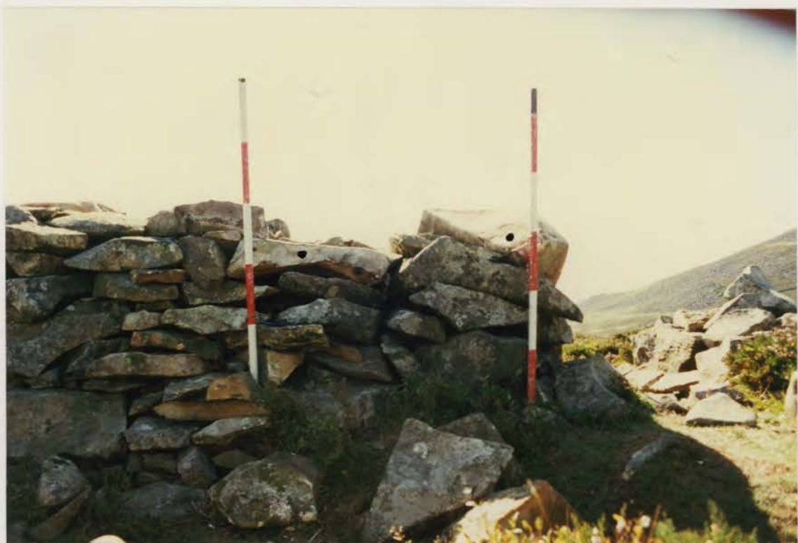
Plate 390. G1022\251\11, collapse 36b after conservation.
