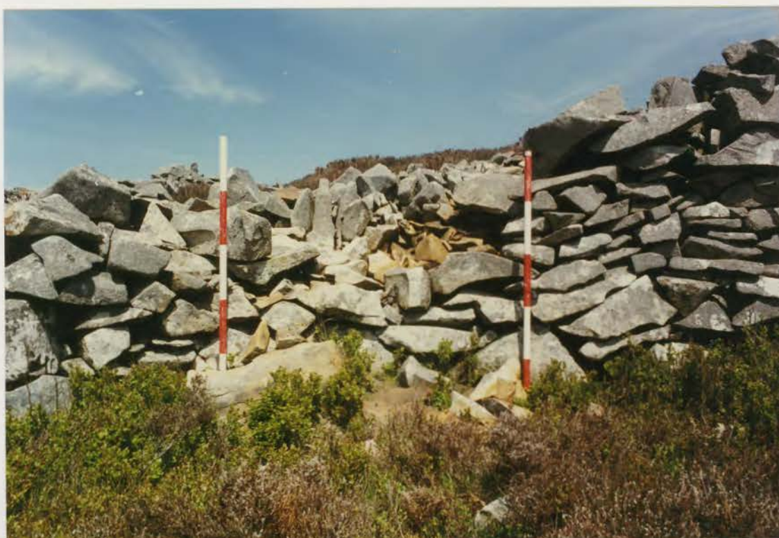
Plate 102. G1022\219\31, collapse 21b before conservation.
