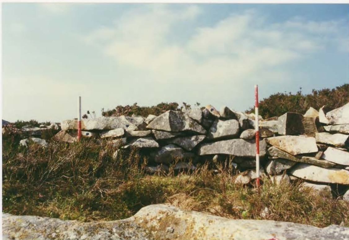
Plate 137. G1022\244\32, collapse 18b after conservation.
