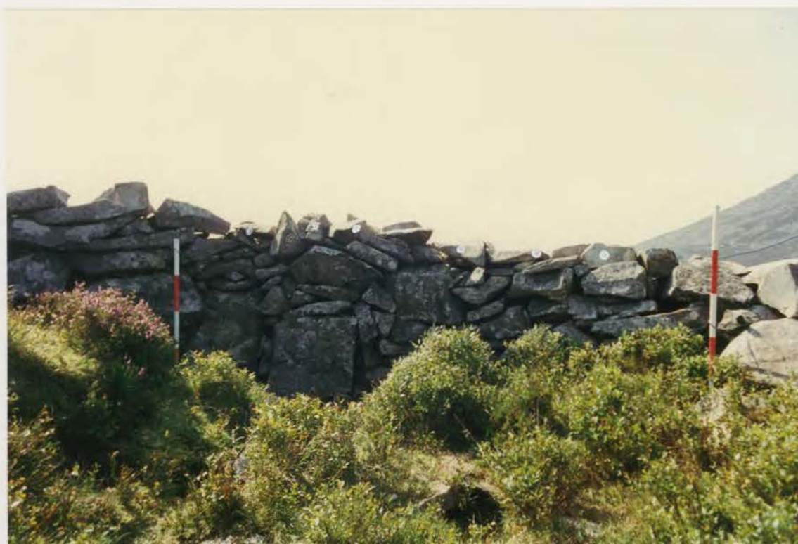
Plate 184. G1022\245\24A, collapse 79c after conservation.
