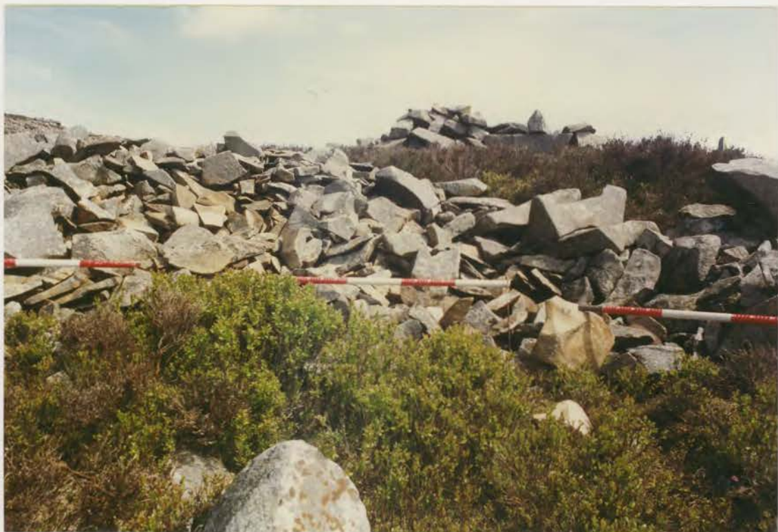
Plate 90. G1022\219\37, collapse 21d before conservation.
