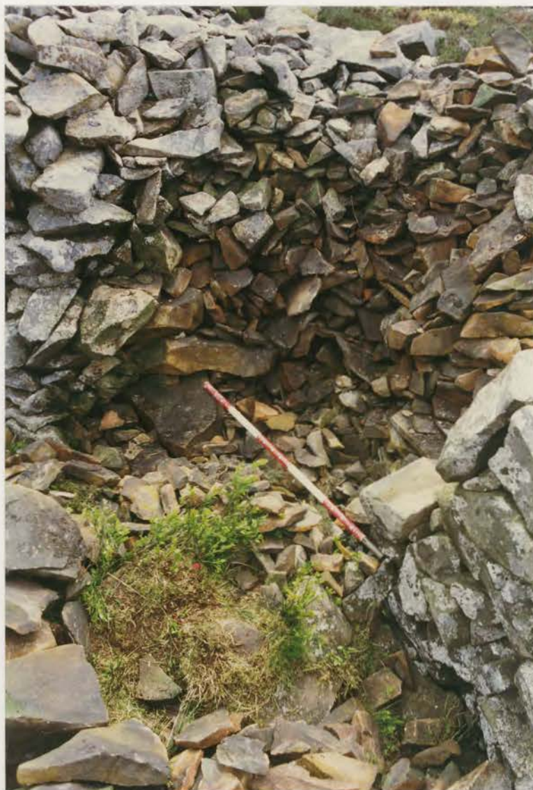
Plate 64. G1022\227\29, collapse 23g after clearance.
