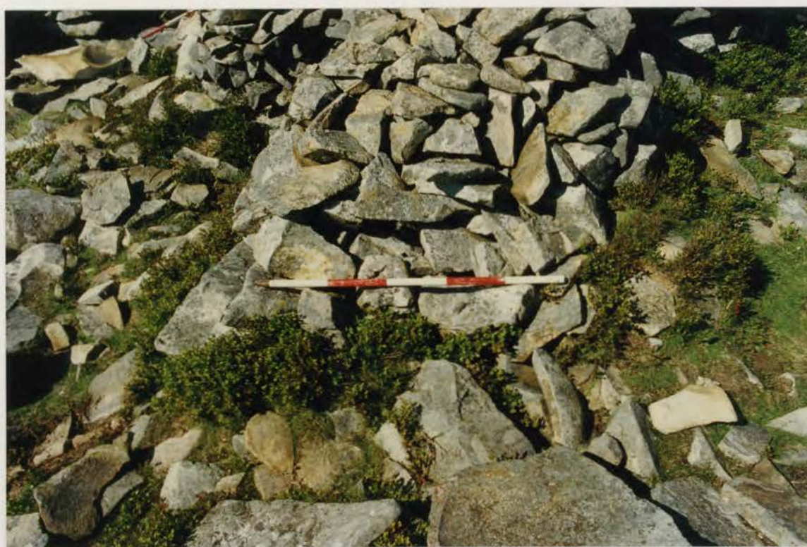
Plate 410. G1022\239\32, collapse 90a before conservation.
