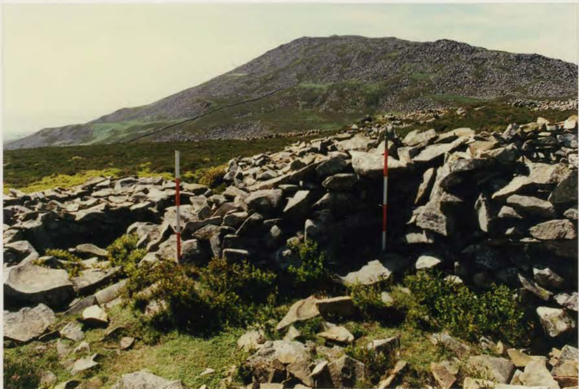
Plate 412. G1022\239\23, collapse 90b before conservation.
