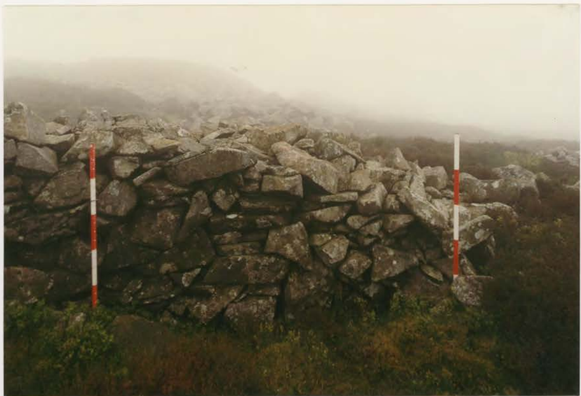
Plate 150. G1022\222\18, collapse 17d before conservation.
