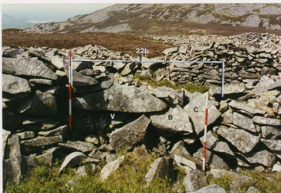
Plate 74. G1022\219\09, collapse 22b before conservation.
