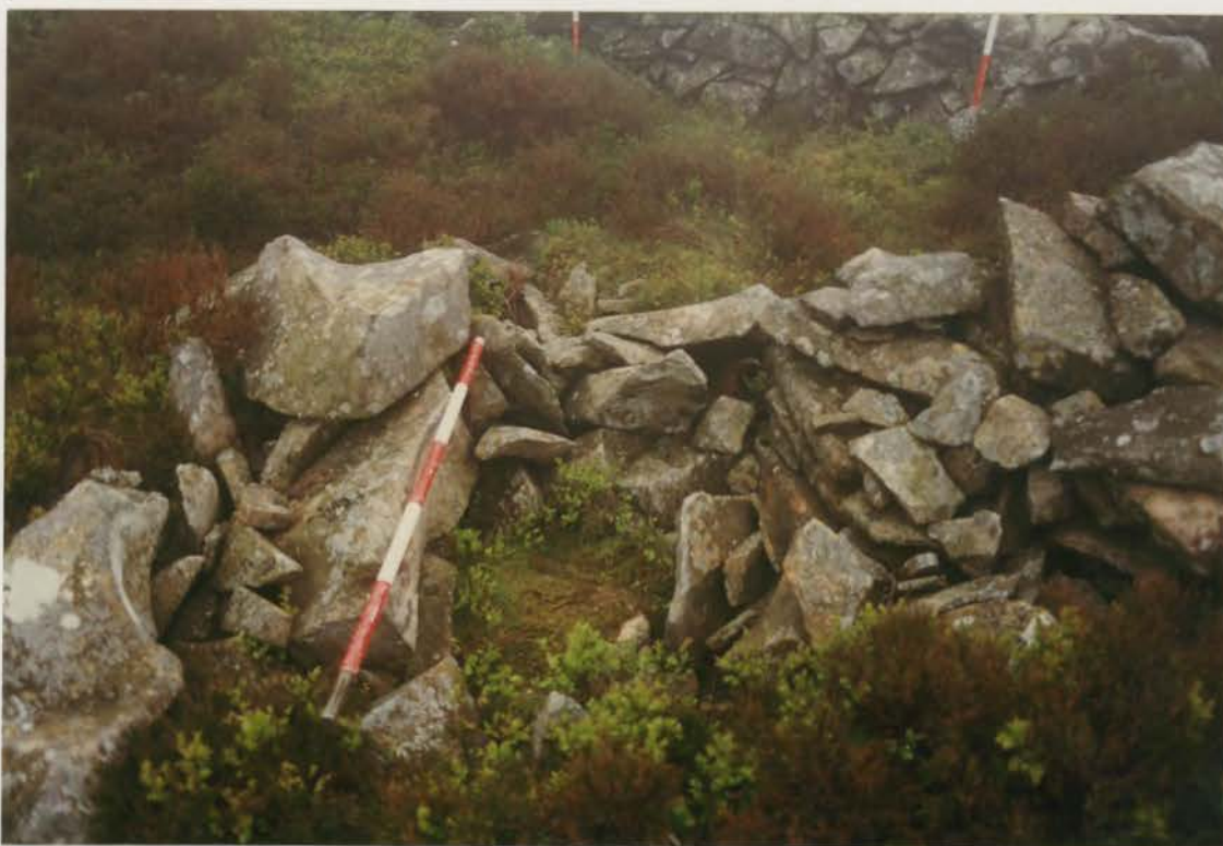
Plate 125. G1022\222\21, collapses 17a, 17e and 18a before conservation.
