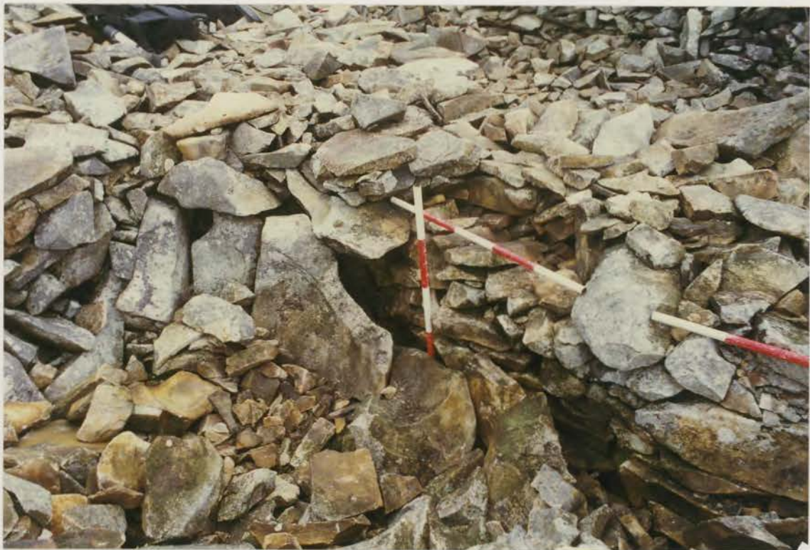
Plate 382. G1022\240\10, collapse 39b after clearance.
