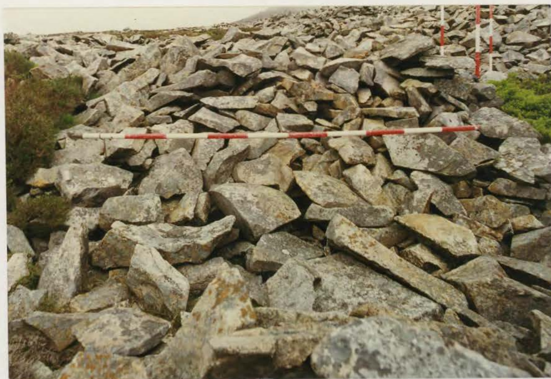
Plate 319. G1022\230\15A, collapse 6a before conservation.
