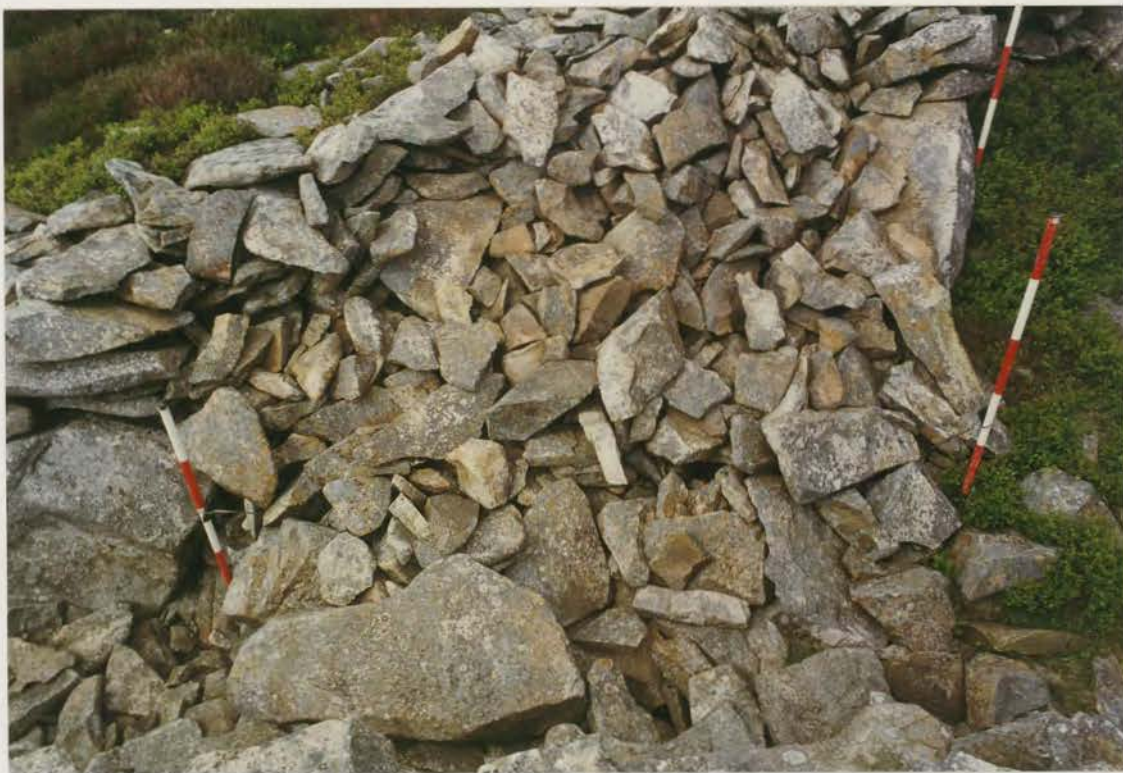
Plate 291. G1022\229\17, collapse 5b before conservation.
