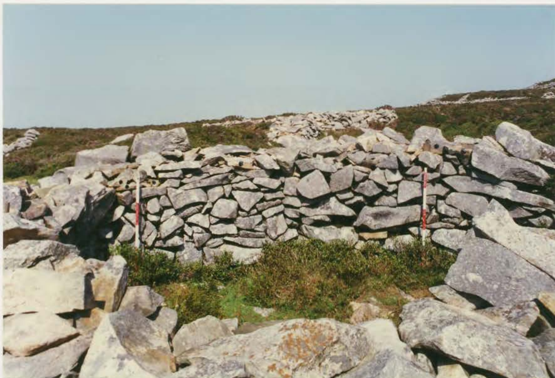
Plate 167. G1022\245\16A, collapse 16d after conservation.
