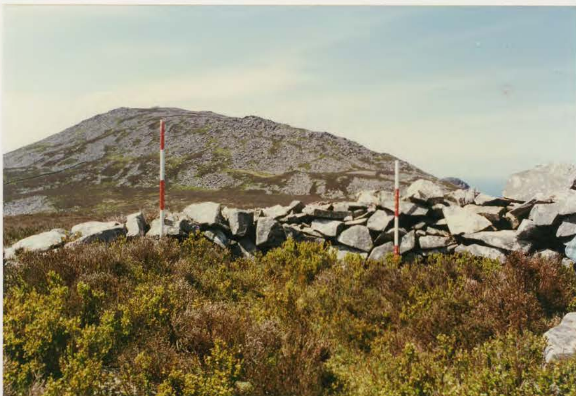
Plate 97. G1022\219\25, collapse 21a before conservation.
