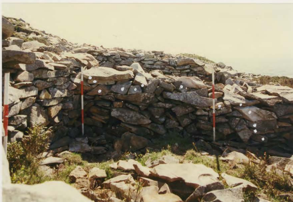
Plate 238. G1022\246\33, collapse 11c after conservation.
