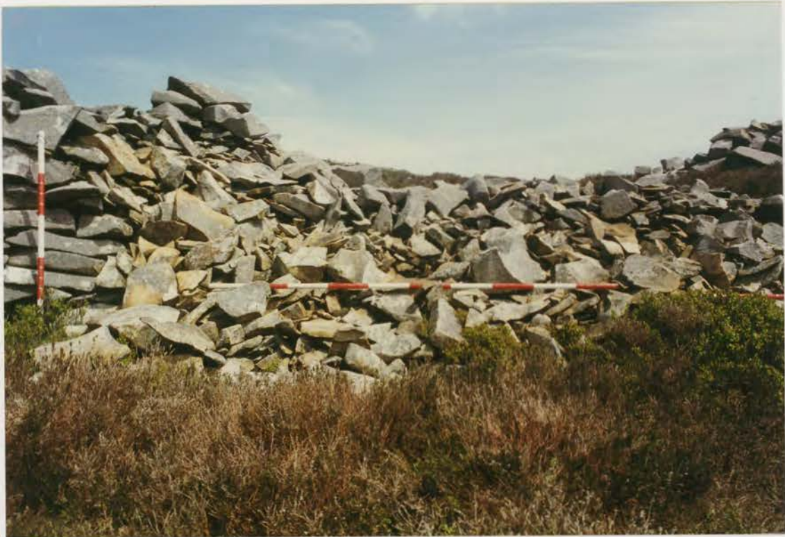
Plate 89. G1022\219\35, collapse 21d before conservation.
