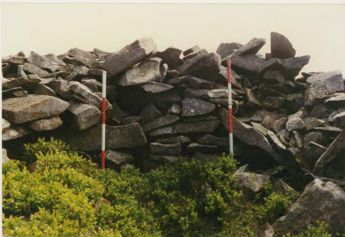
Plate 233. G1022\226\11, collapse 11a before conservation.
