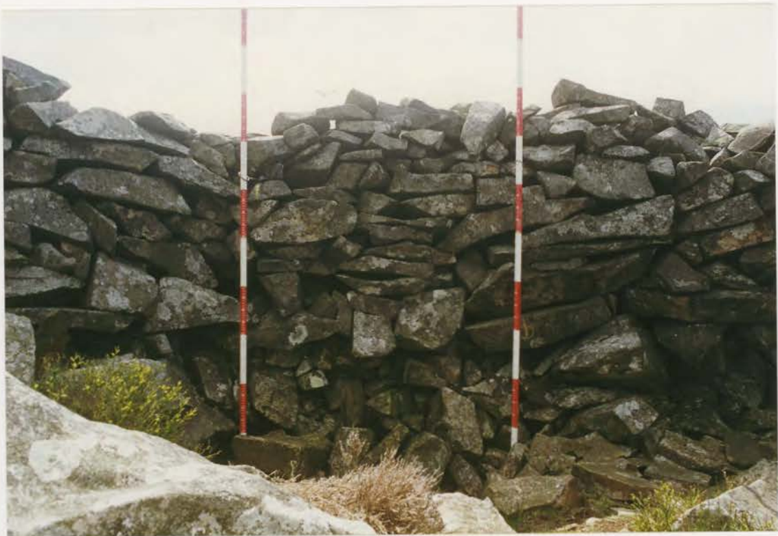
Plate 12. G1022\215\09, collapse 24b before conservation.
