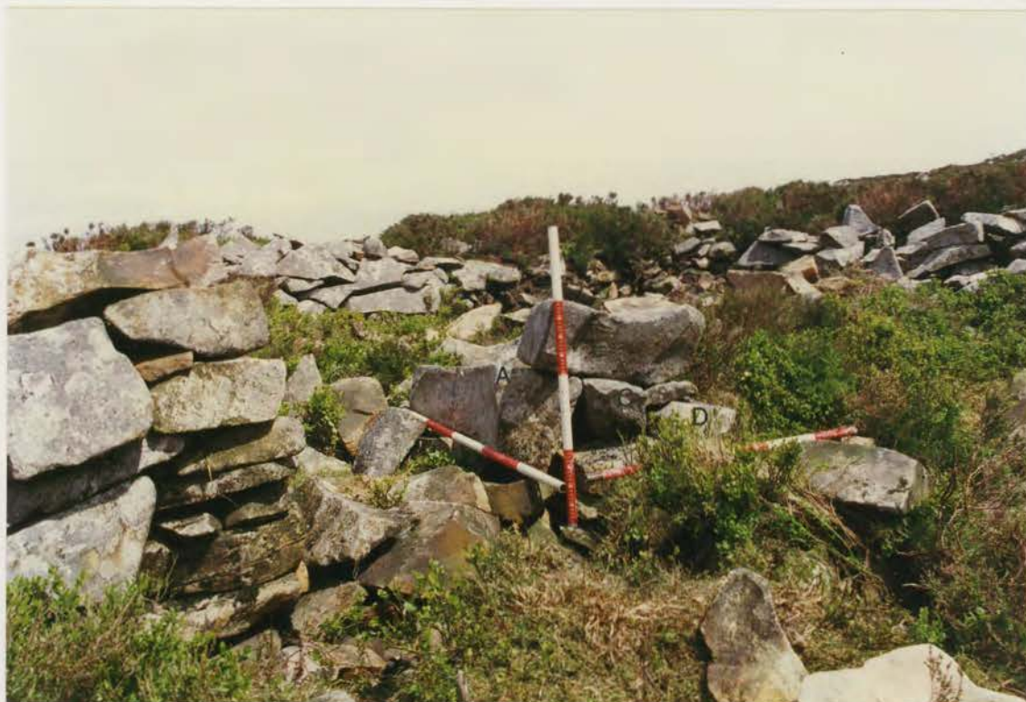
Plate 131. G1022\235\23, collapse 17e before conservation.
