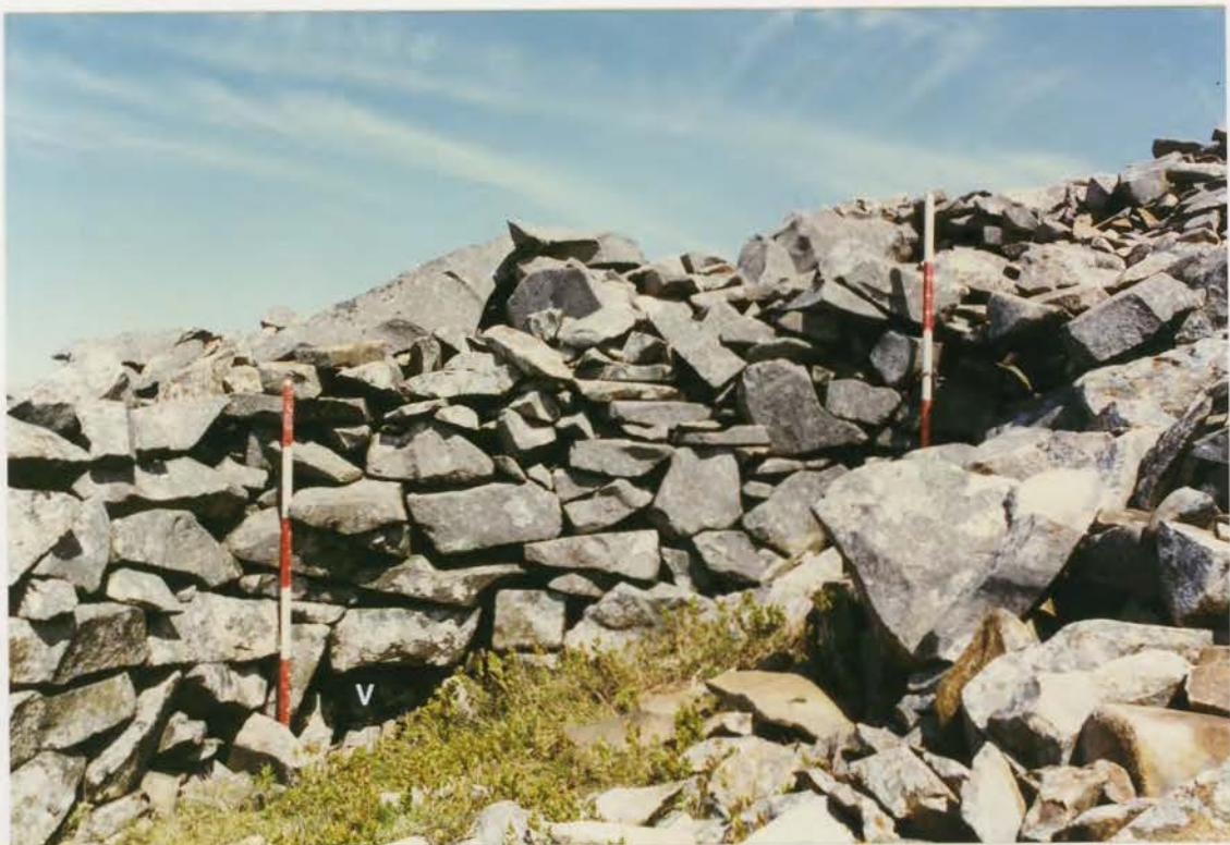
Plate 78. G1022\219\14, collapse 22d before conservation.
