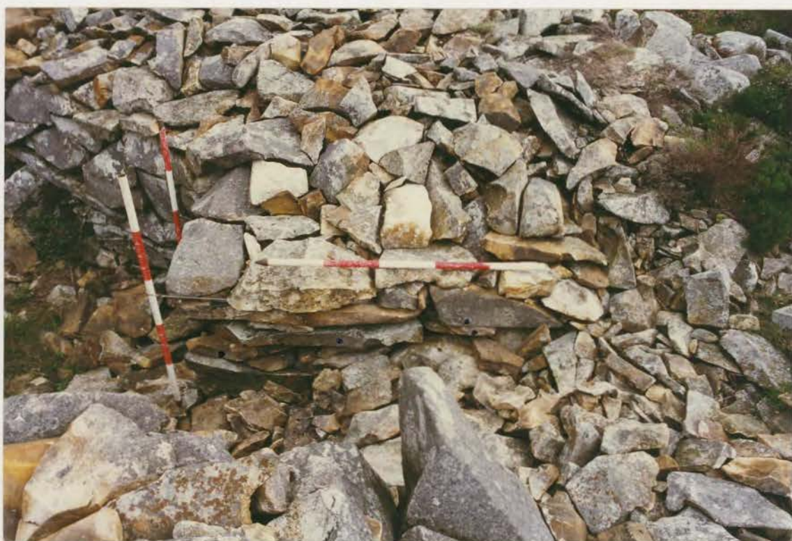
Plate 88. G1022\243\36A, collapse 22h after conservation.
