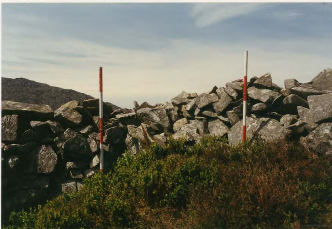
Plate 155. G1022\222\24, collapse 95b before conservation.
