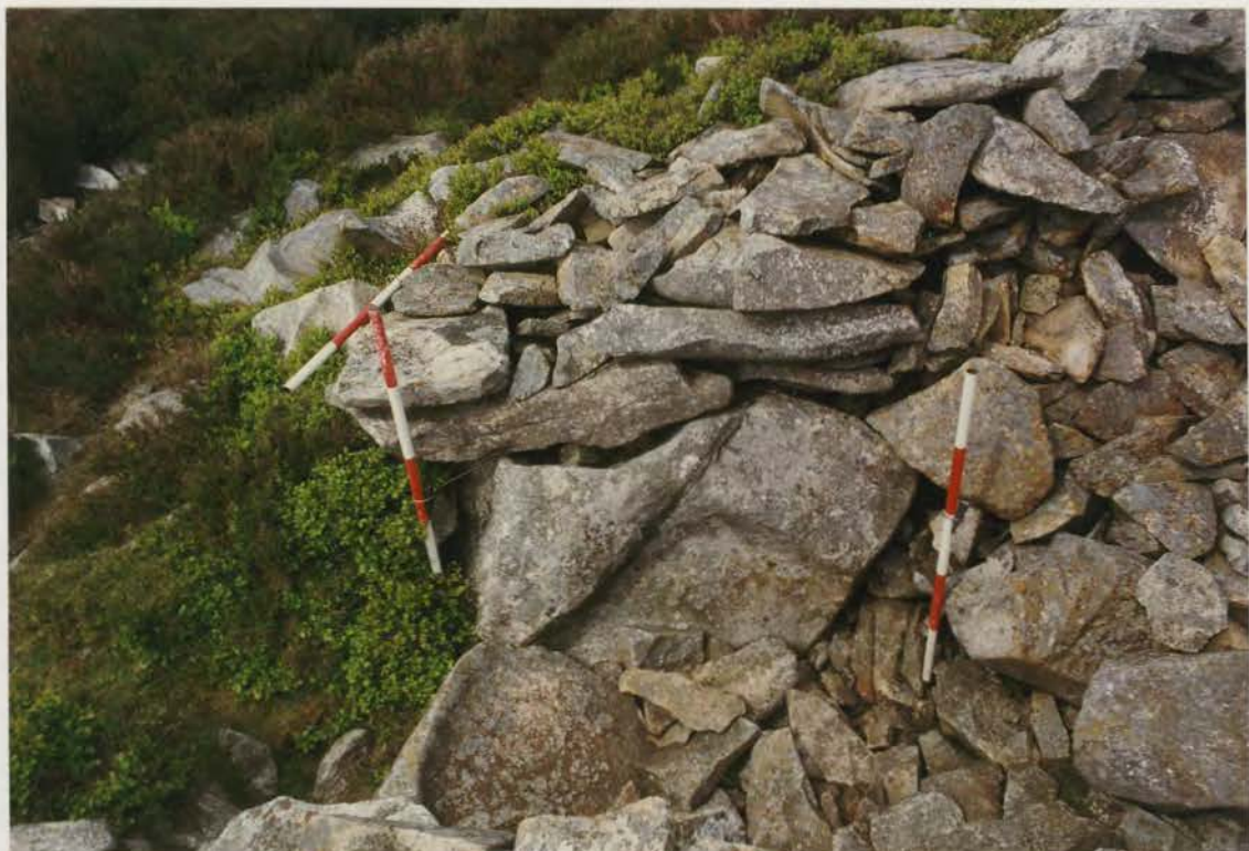
Plate 290. G1022\229\16, collapse 5a before conservation.
