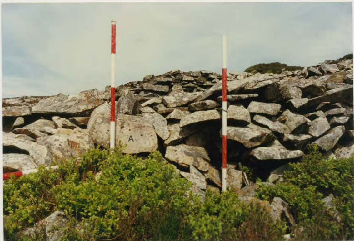
Plate 282. G1022\228\35, collapse 14e before conservation.
