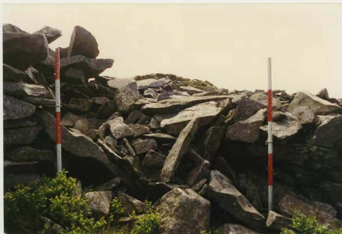
Plate 234. G1022\226\13, collapse 11b before conservation.
