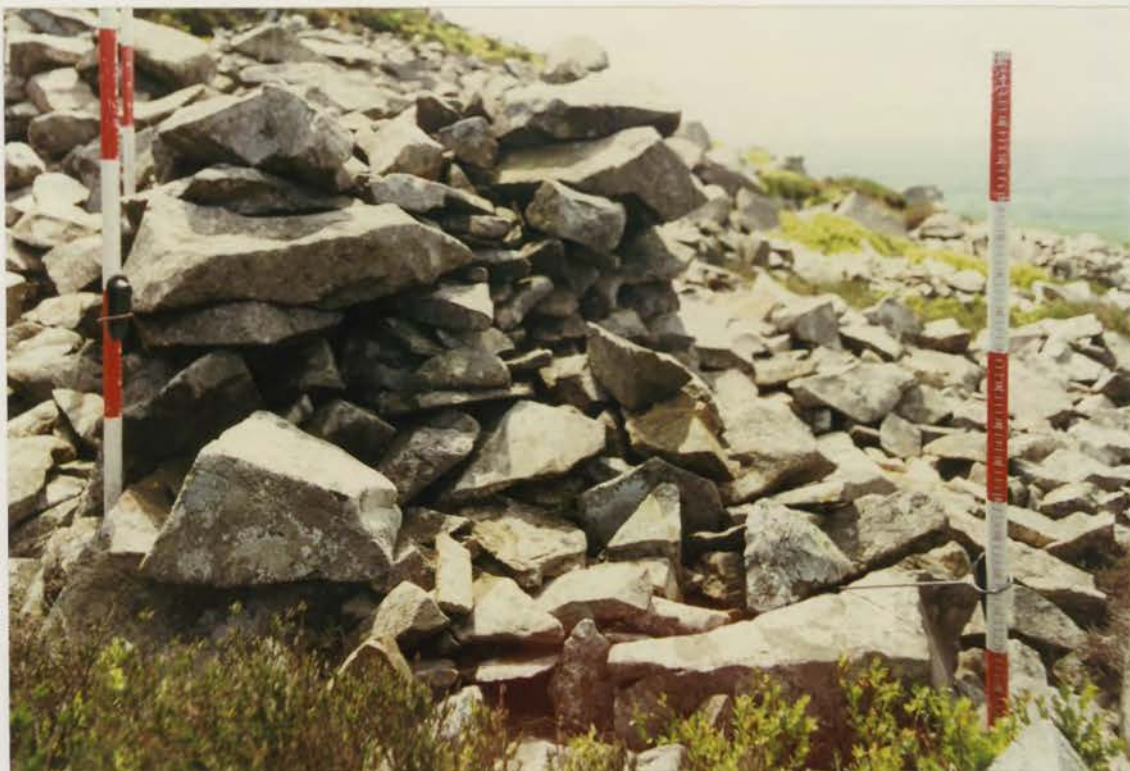
Plate 349. G1022\231\09, collapse 6n before conservation.
