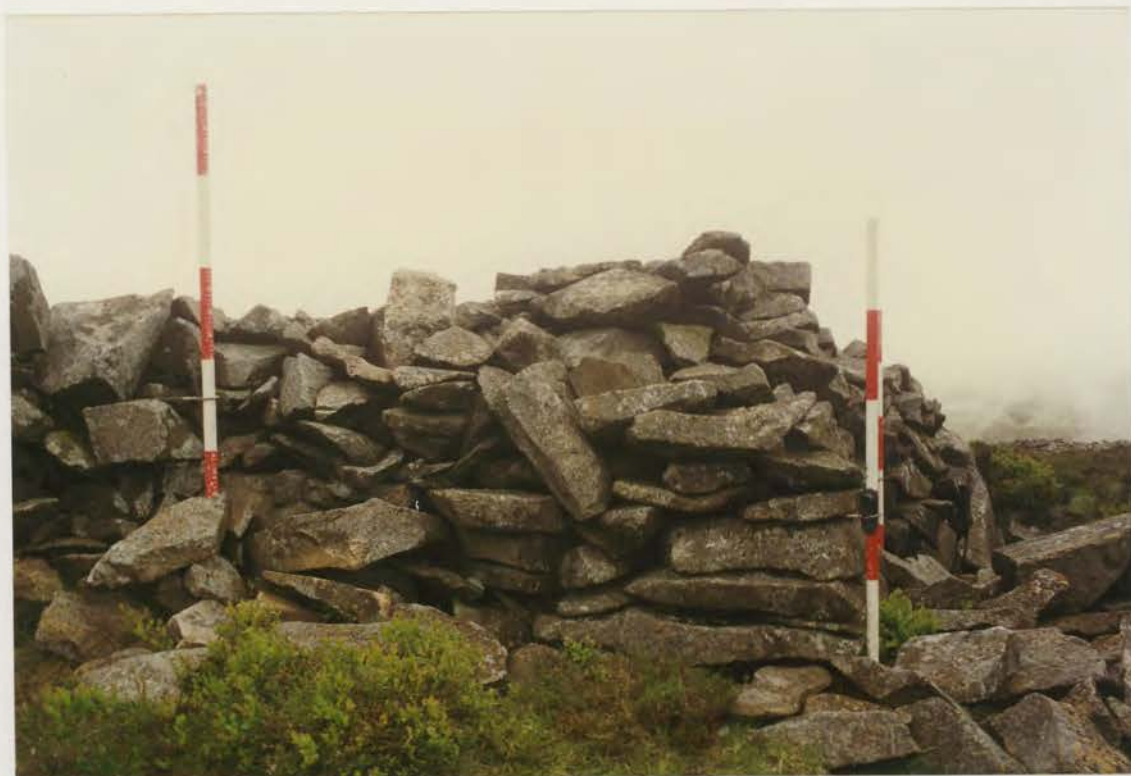
Plate 313. G1022\229\33, collapse 5h before conservation.
