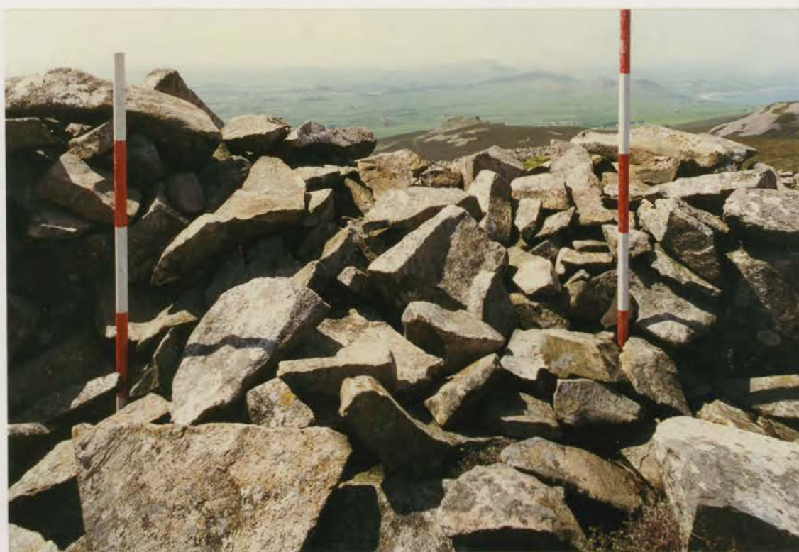
Plate 346. G1022\231\04, collapse 6l before conservation.
