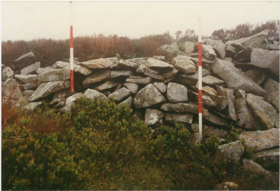
Plate 143. G1022\222\10, collapse 17b before conservation.
