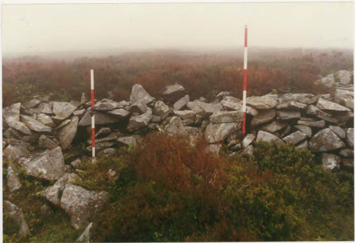
Plate 141. G1022\222\09, collapses 18d and e before conservation.
