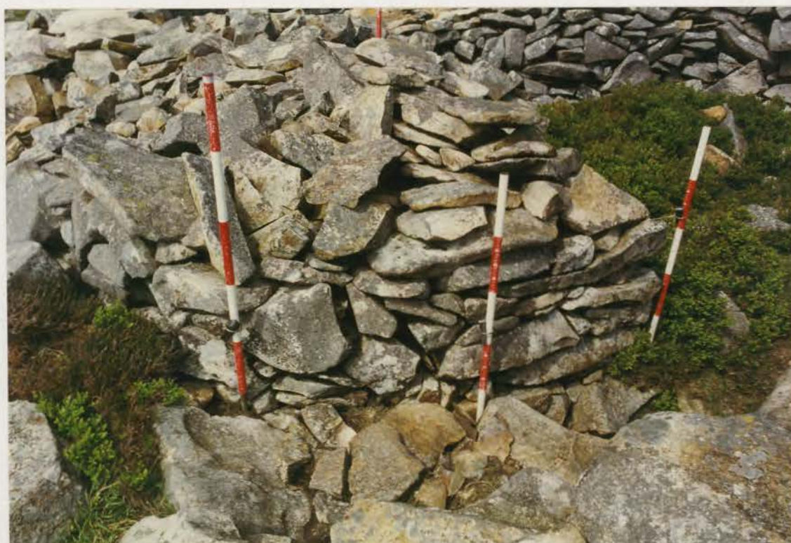
Plate 204. G1022\224\18, collapse 8a before conservation.
