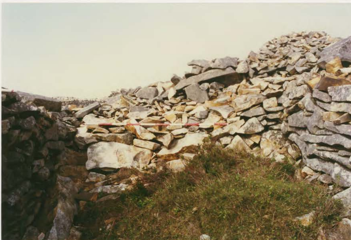
Plate 57. G1022\243\13, collapse 23c after conservation.
