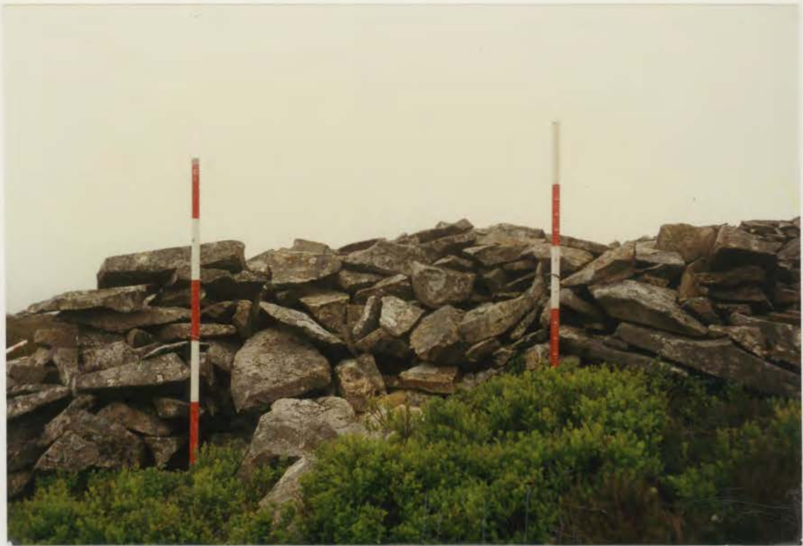
Plate 325. G1022\230\22A, collapse 6d before conservation.
