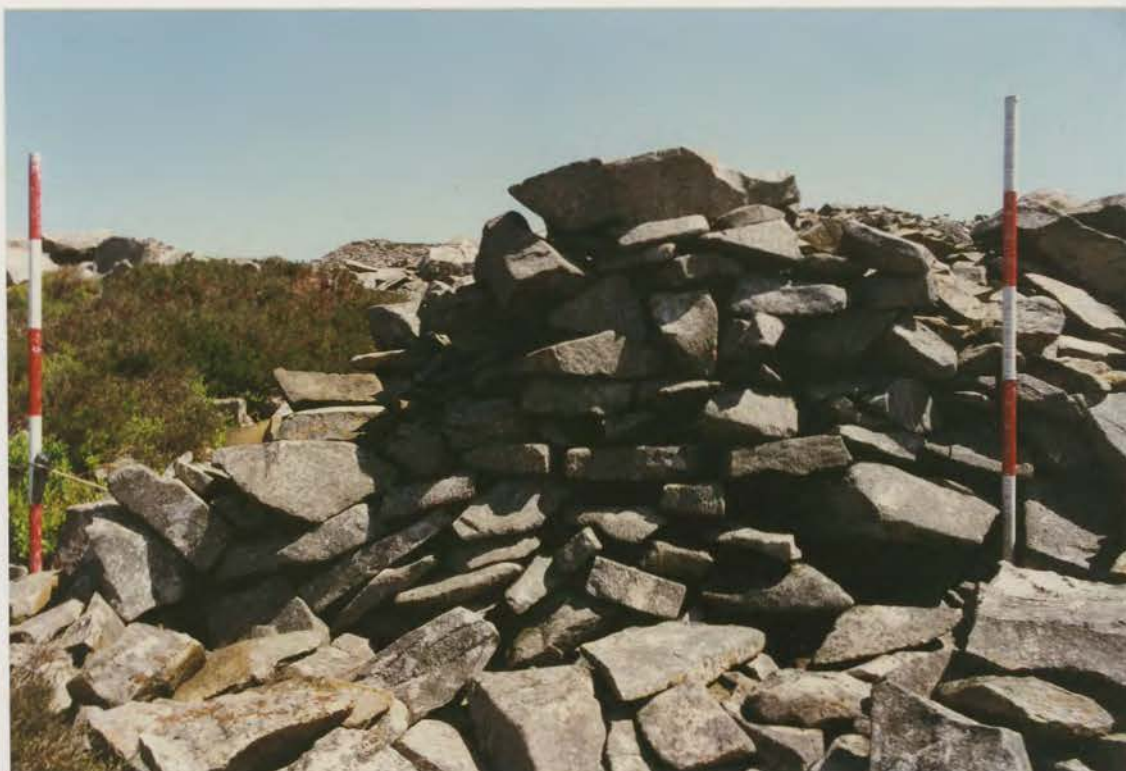
Plate 351. G1022\231\10, collapse 6o before conservation.
