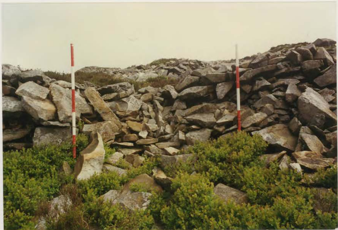
Plate 302. G1022\229\25, collapse 5d before conservation.
