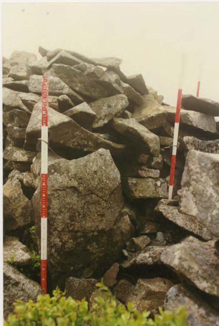
Plate 199. G1022\225\05, collapse 8i before conservation.
