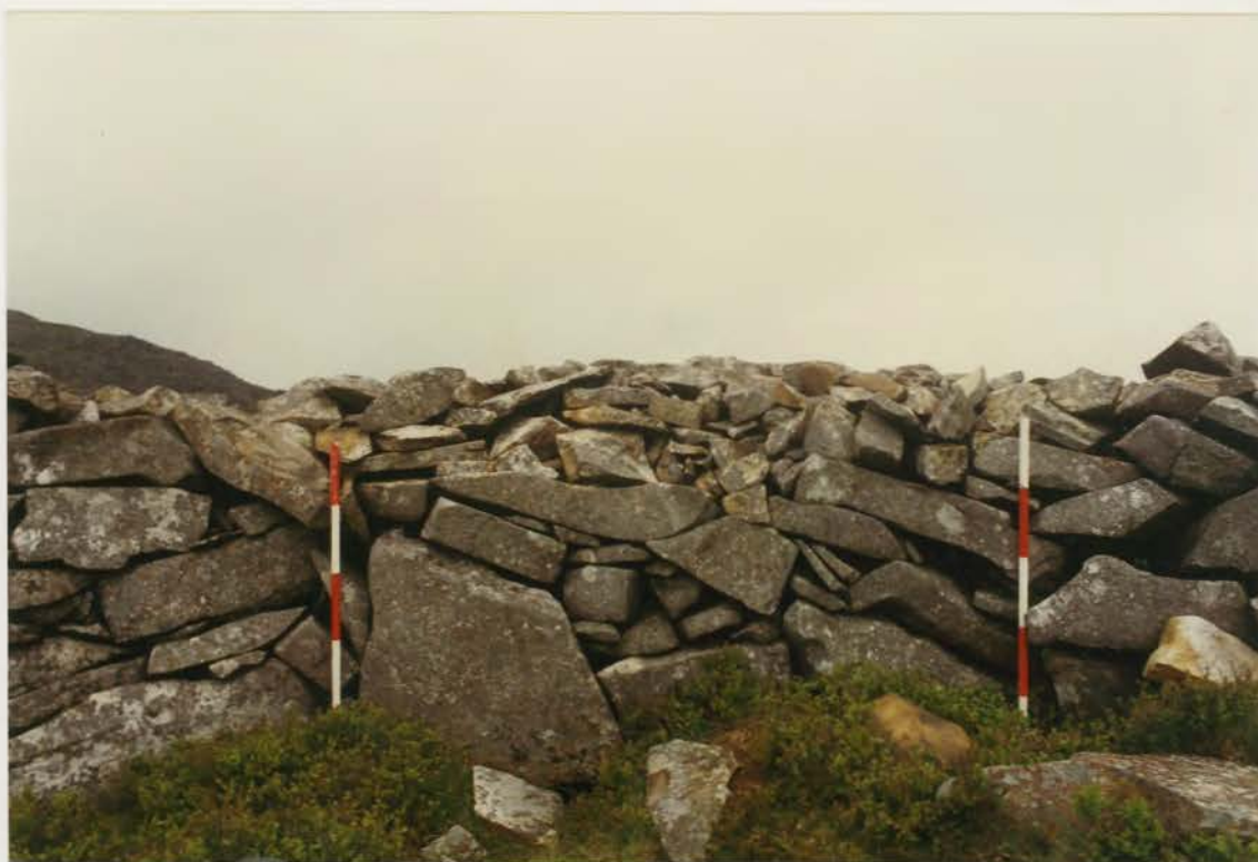
Plate 107. G1022\221\04, collapse 19a before conservation.
