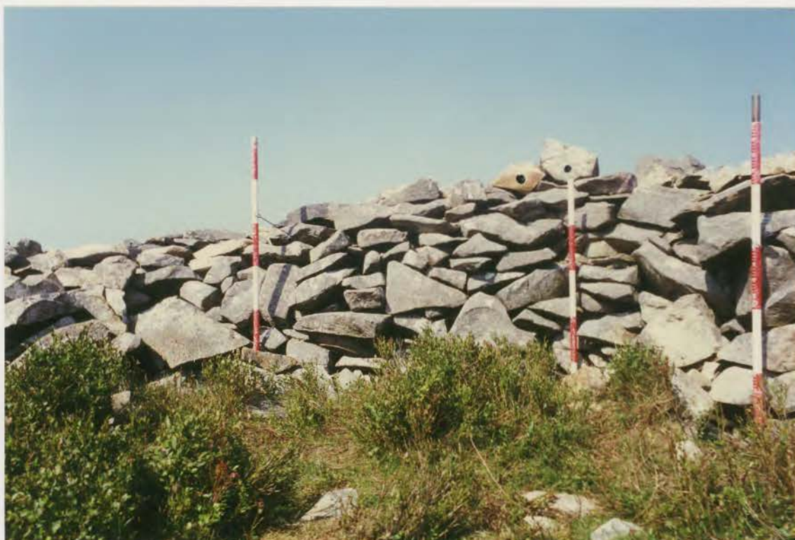
Plate 187. G1022\245\32A, collapse 8d after conservation.
