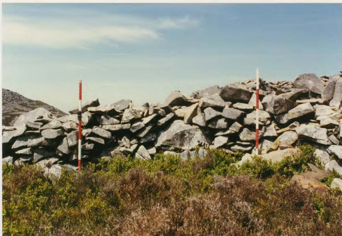
Plate 99. G1022\212\29, collapse 21a before conservation.
