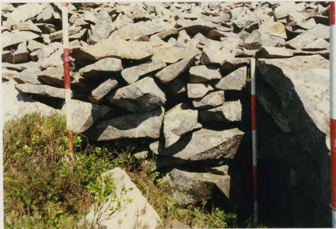
Plate 359. G1022\231\30, collapse 74e before conservation.
