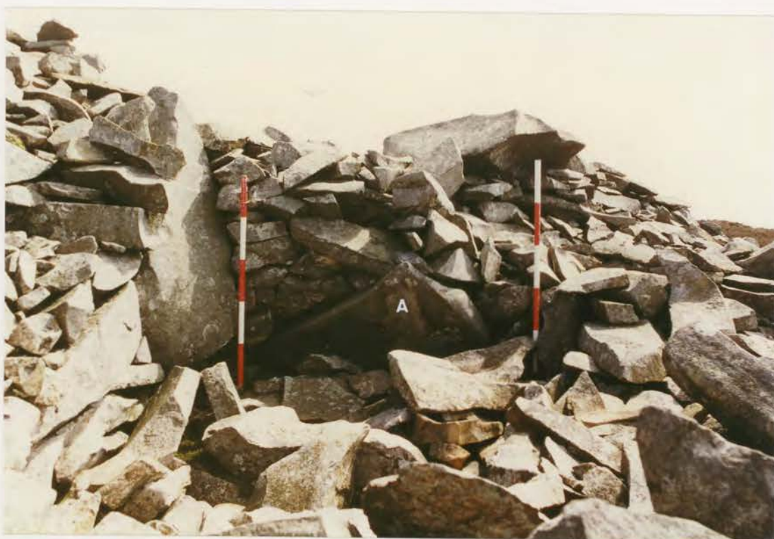
Plate 20. G1022\217\03, collapse 82a before conservation.
