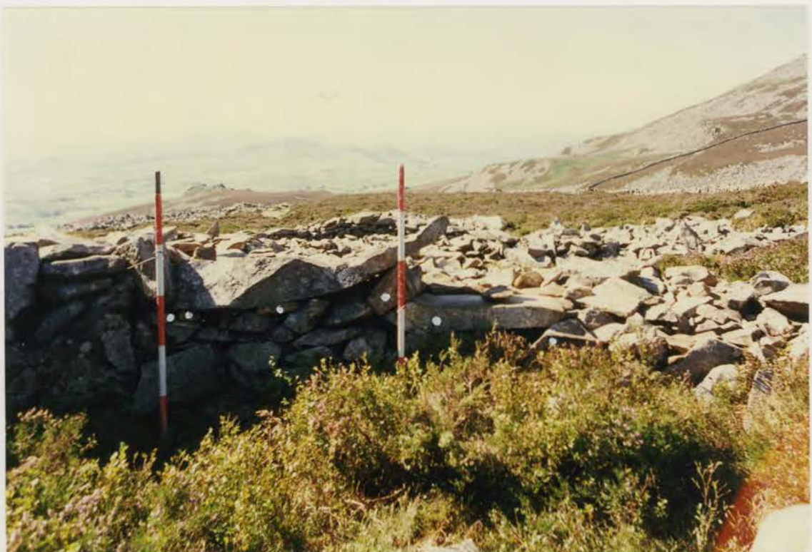
Plate 378. G1022\250\20, collapse 40c after conservation.
