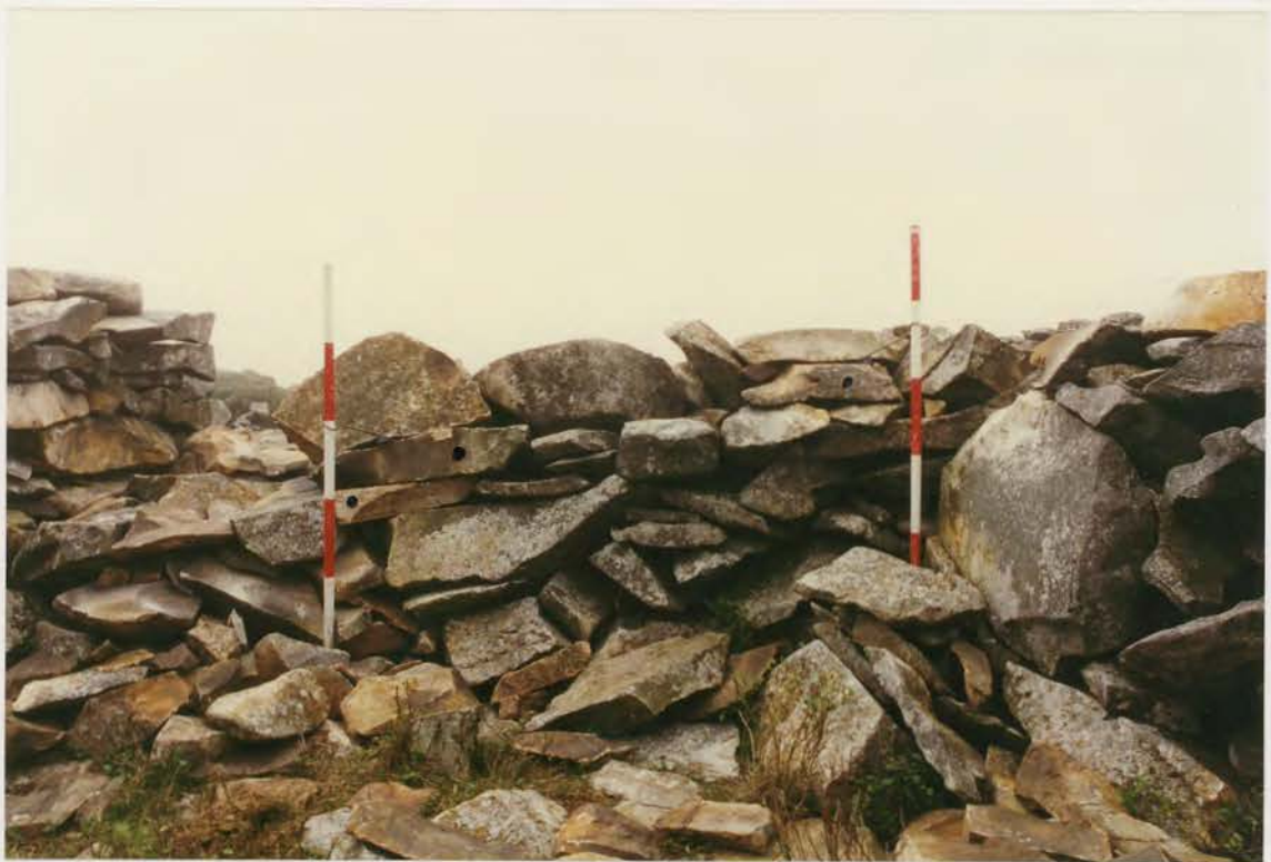
Plate 51. G1022\243\03, collapse 26b after conservation.
