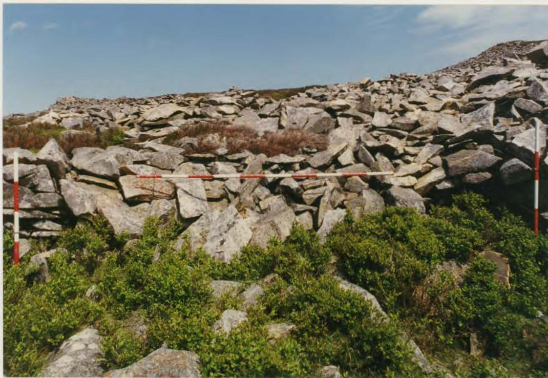
Plate 229. G1022\226\25, collapse 11i before conservation.
