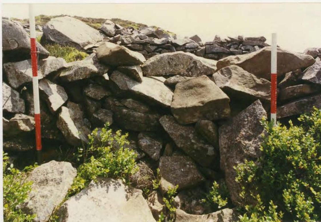
Plate 162. G1022\223\14, collapse 16b before conservation.
