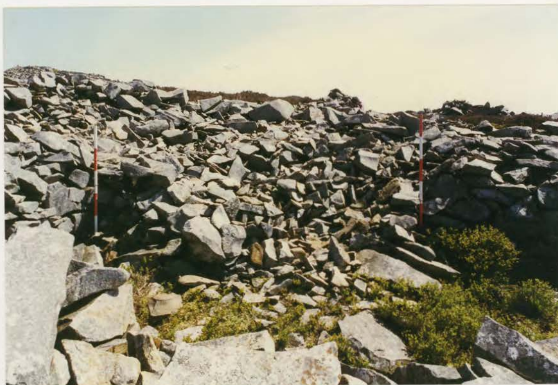
Plate 80. G1022\219\15, collapse 22e before conservation.
