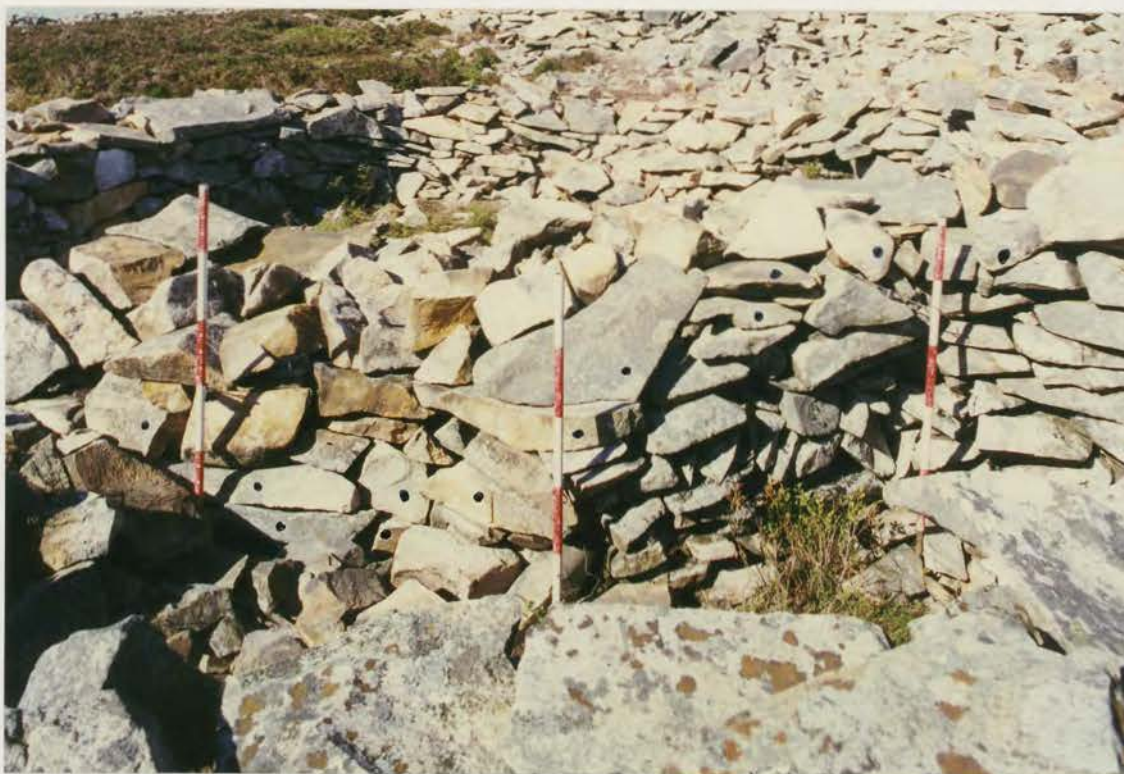
Plate 249. G1022\247\17, collapses 12e and a after conservation.
