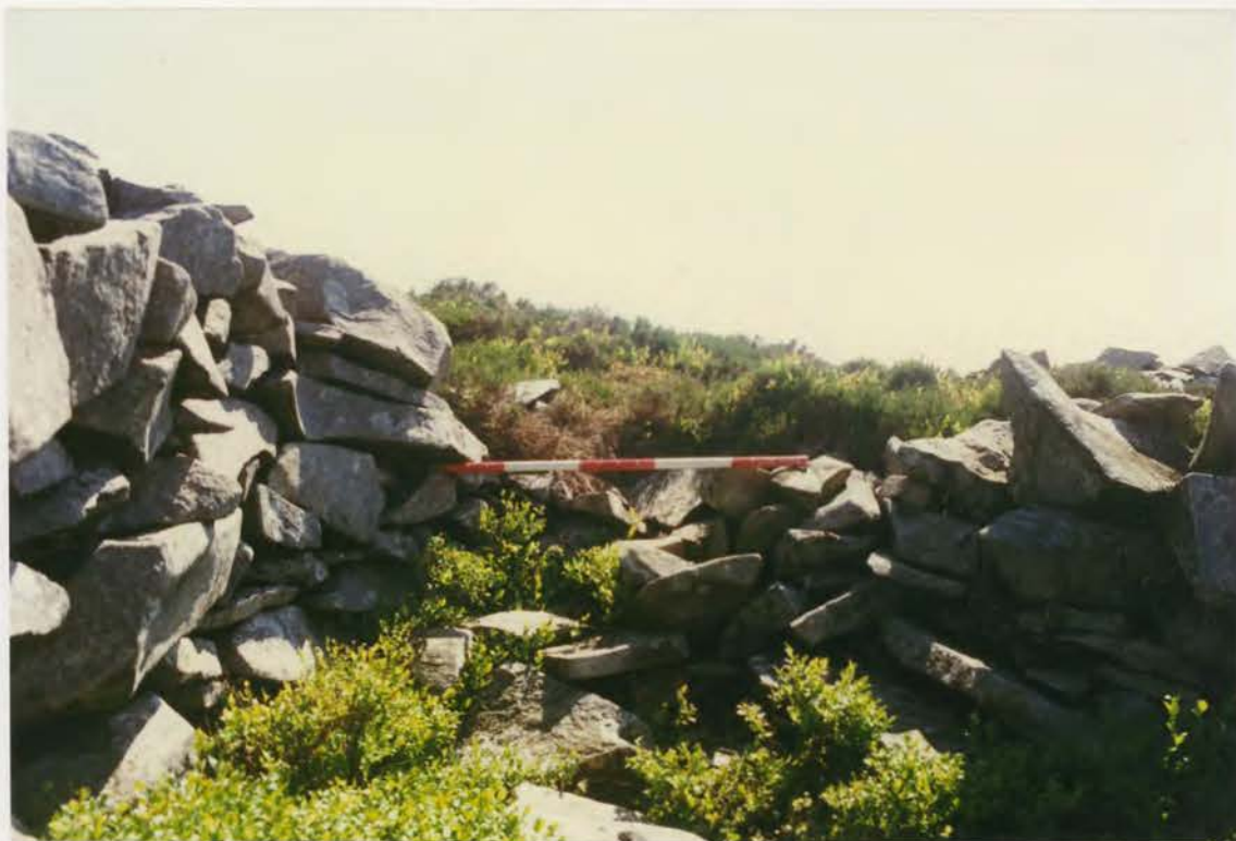
Plate 159. G1022\236\10, collapse 16a before conservation.
