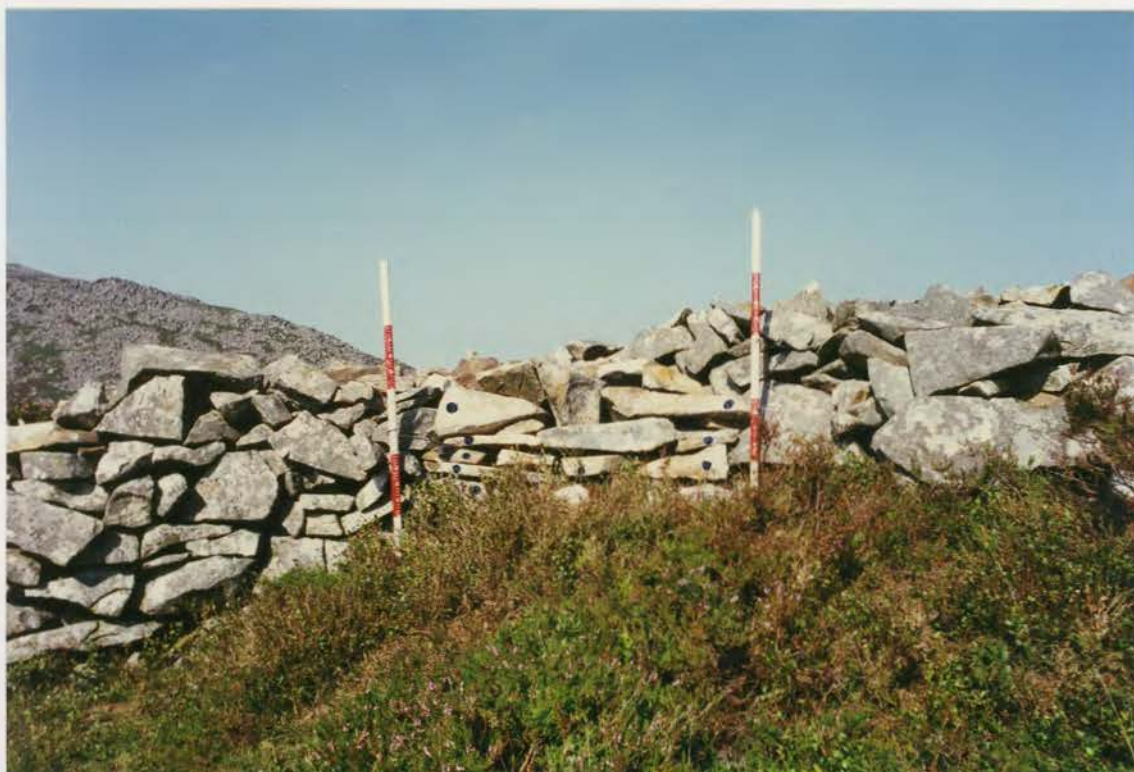
Plate 156. G1022\245\00A, collapse 95b after conservation.
