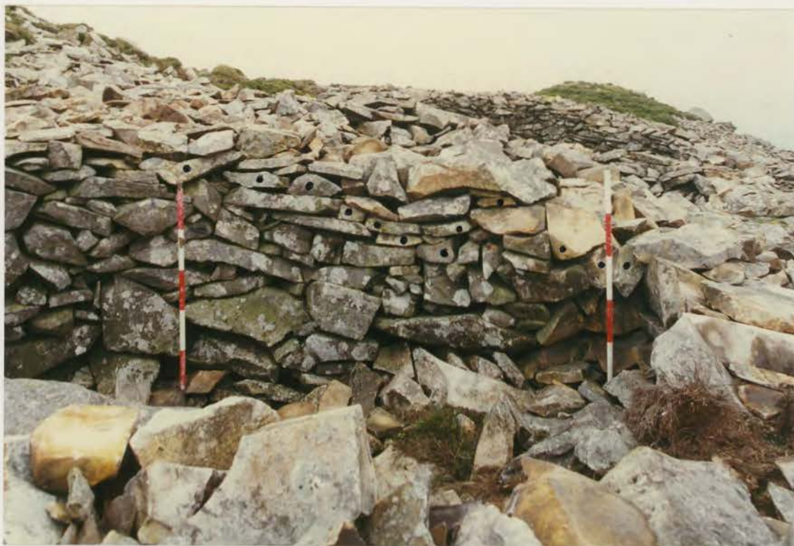
Plate 253. G1022\247\23, collapse 12c after conservation.
