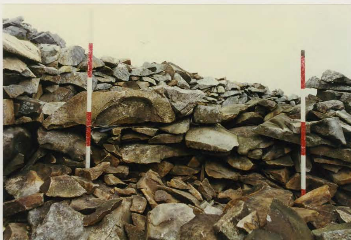
Plate 396. G1022\240\12, collapse 89a after clearance.
