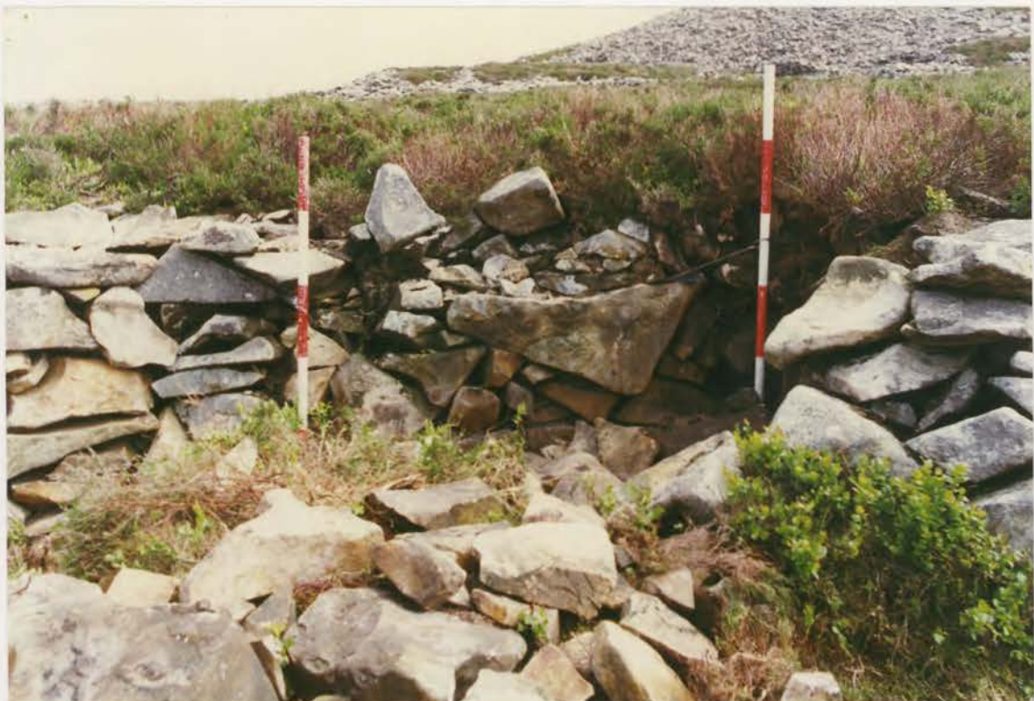
Plate 142. G1022\236\00, collapses 18d and e after clearance.
