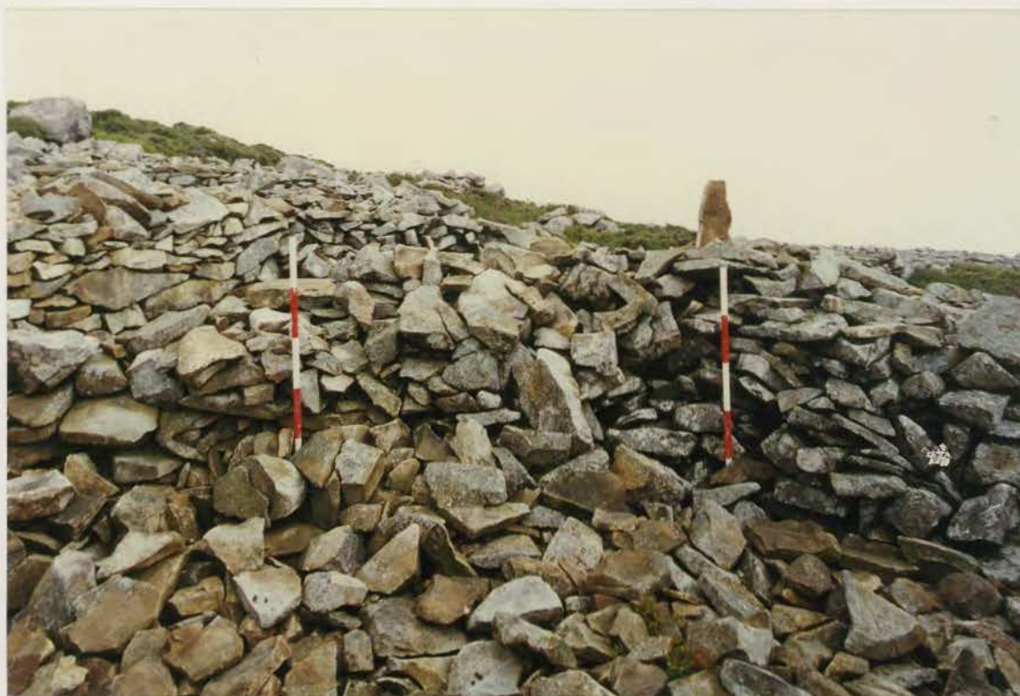
Plate 395. G1022\240\05, collapse 89a before conservation.
