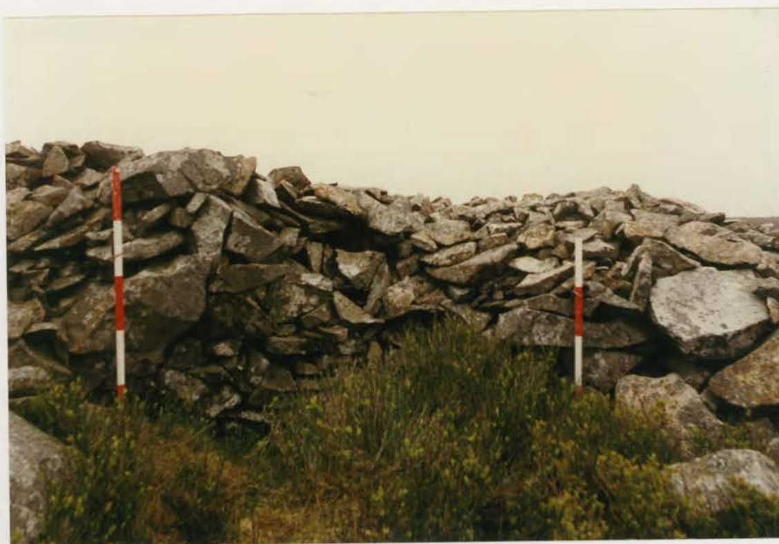
Plate 66. G1022\218\24A, collapse 23h before conservation.
