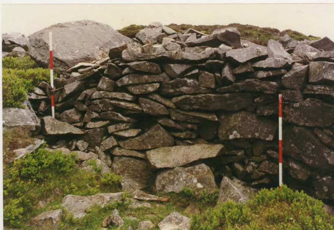
Plate 168. G1022\233\02, collapse 15a before conservation.
