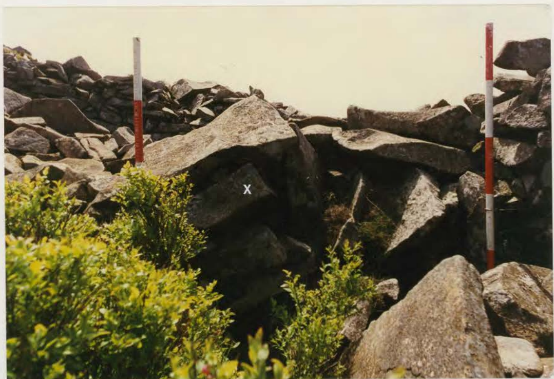
Plate 240. G1022\226\19, collapse 11d before conservation.
