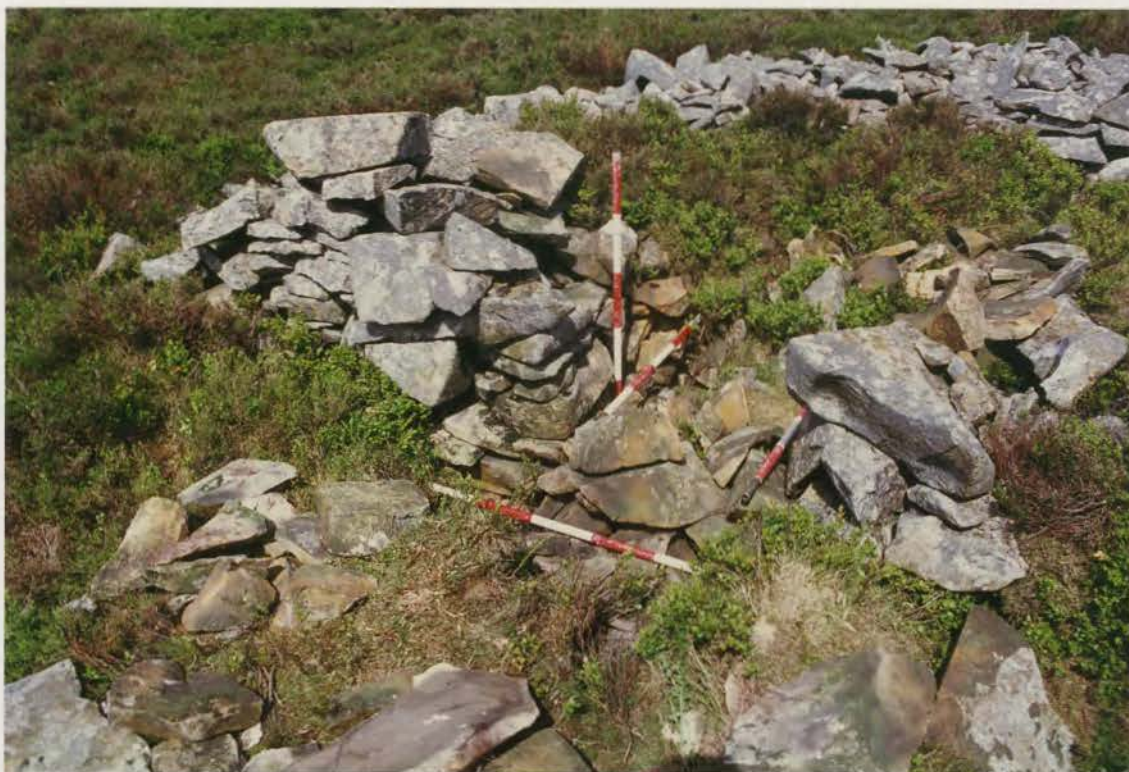
Plate 127. G1022\235\19, collapses 17a, 17e and 18a after clearance.
