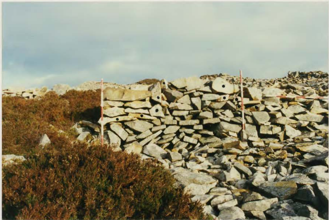
Plate 353. G1022\252\23, collapse 60 after conservation.
