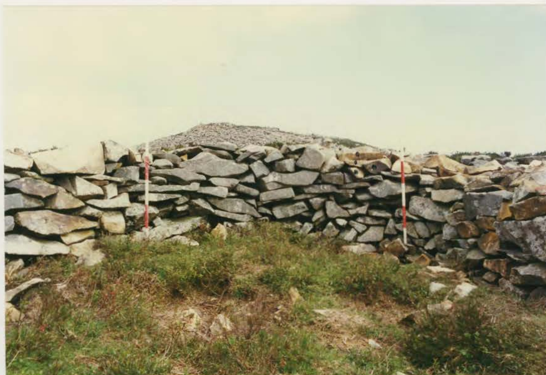
Plate 114. G1022\244\13, collapse 19c after conservation.
