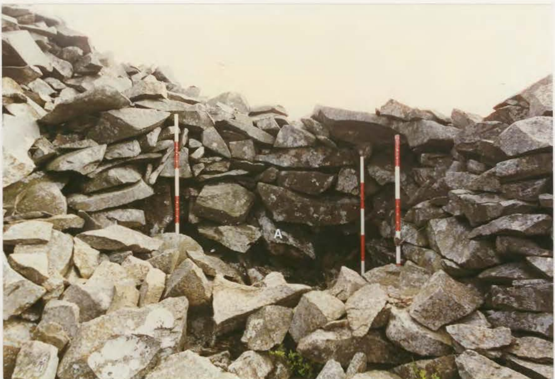
Plate 40. G1022\216\32, collapse 26e before conservation.
