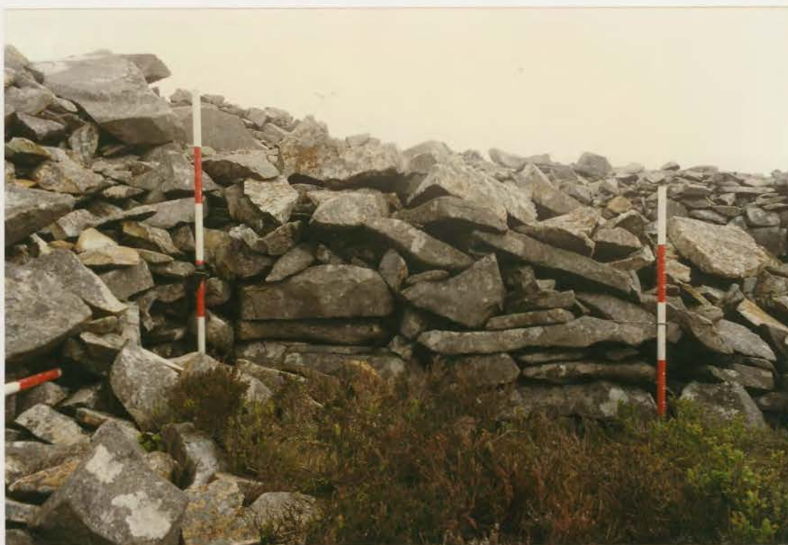
Plate 58. G1022\218\14A, collapse 23d before conservation.
