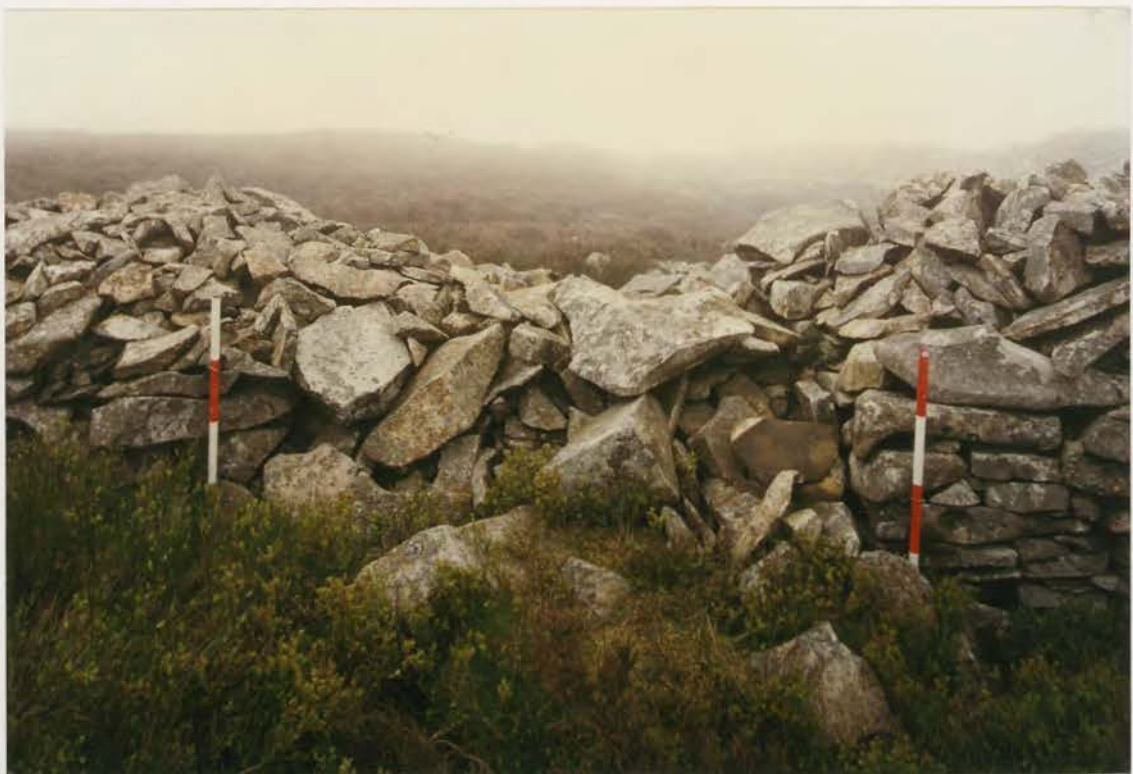
Plate 68. G1022\218\25A, collapse 23i before conservation.
