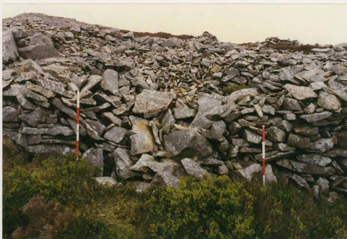
Plate 60. G1022\218\16A, collapse 23e before conservation.
