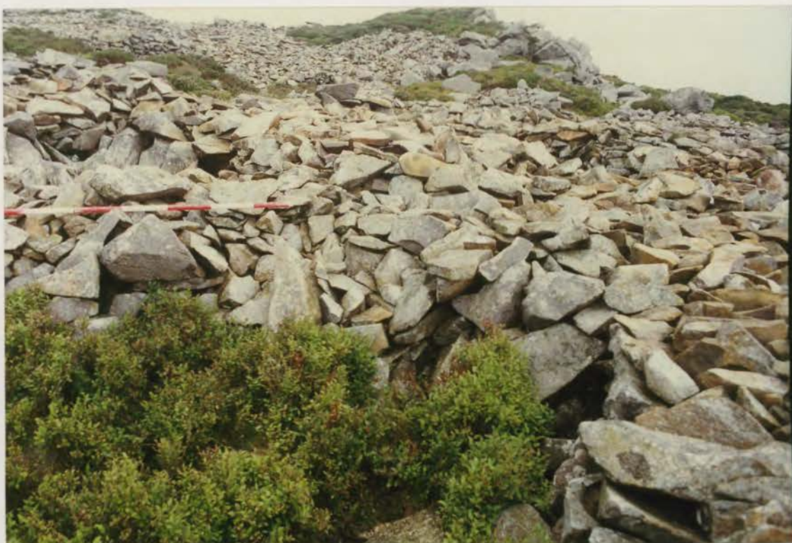
Plate 384. G1022\240\18, collapse 88a before conservation.
