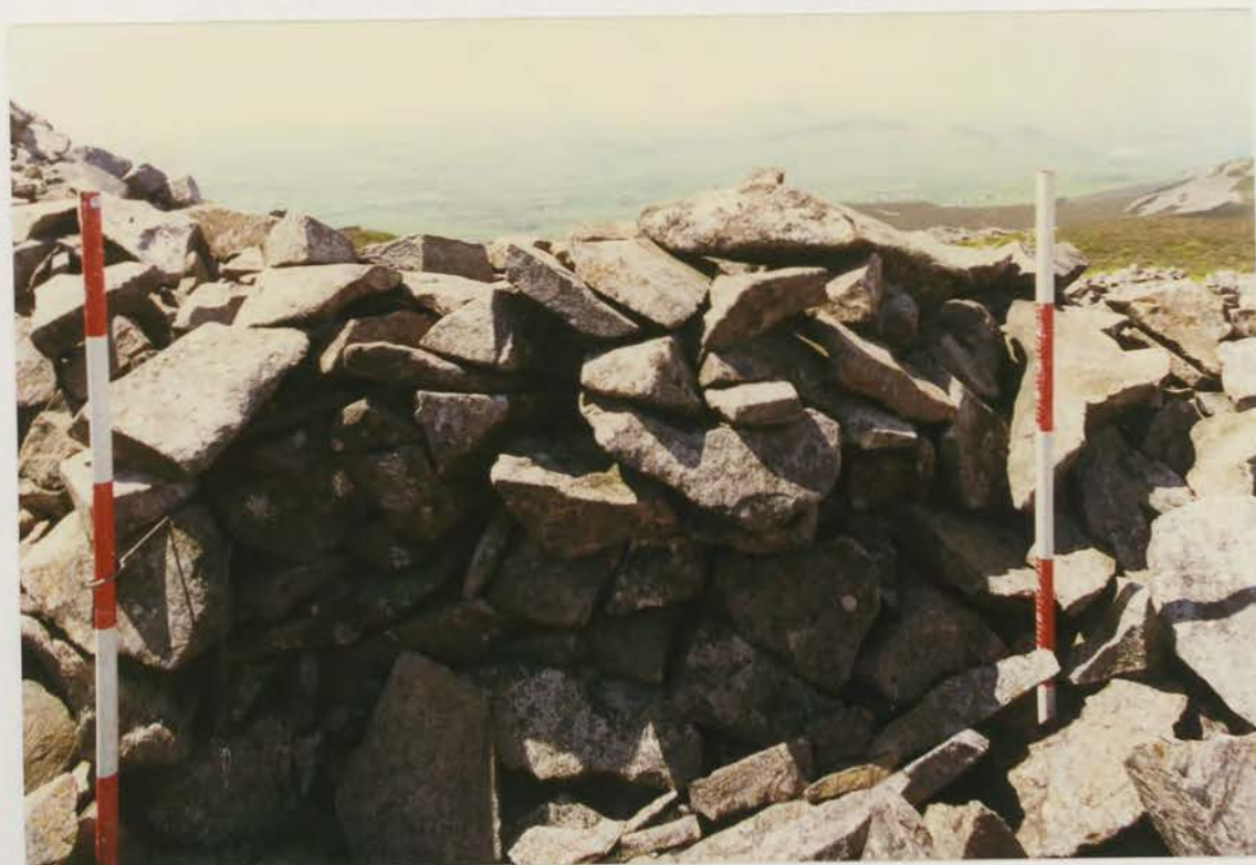
Plate 343. G1022\238\27, collapse 6j showing facing within wall.
