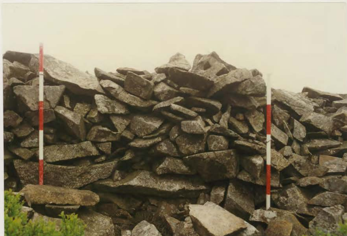
Plate 337. G1022\230\33A, collapse 6i before conservation.
