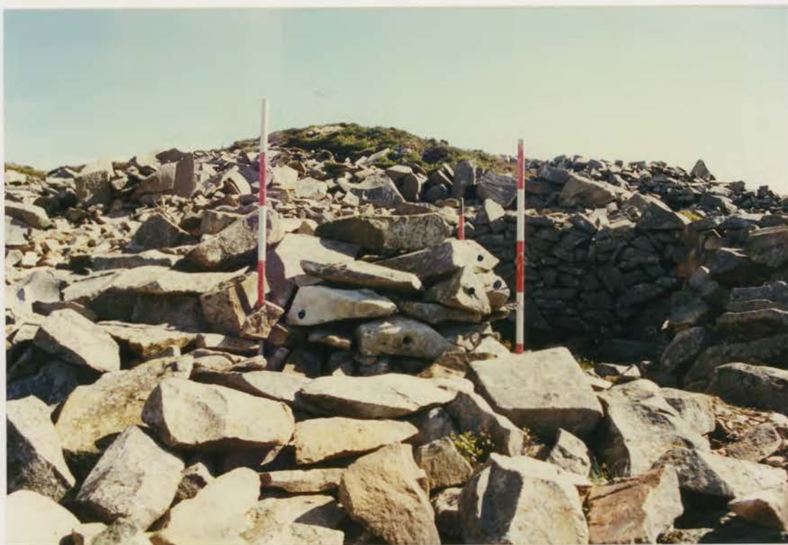
Plate 216. G1022\246\12, collapse 7a outer face after conservation.
