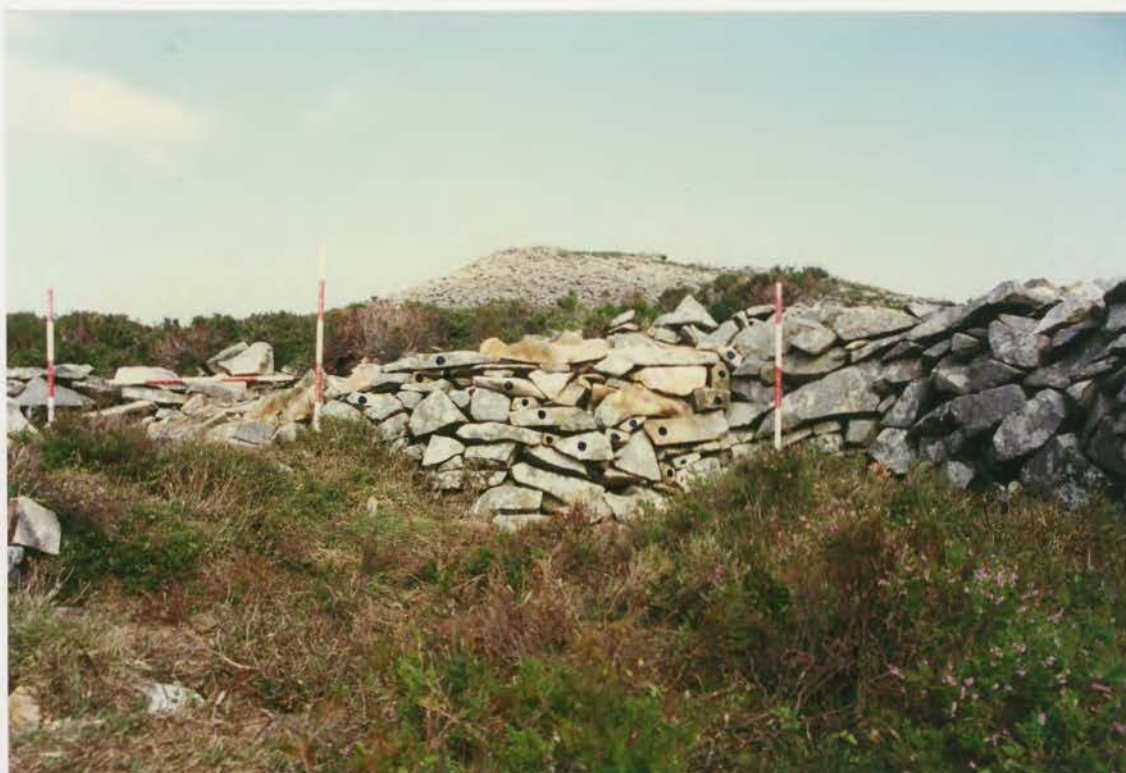
Plate 147. G1022\244\28, collapses 17b and c after conservation.
