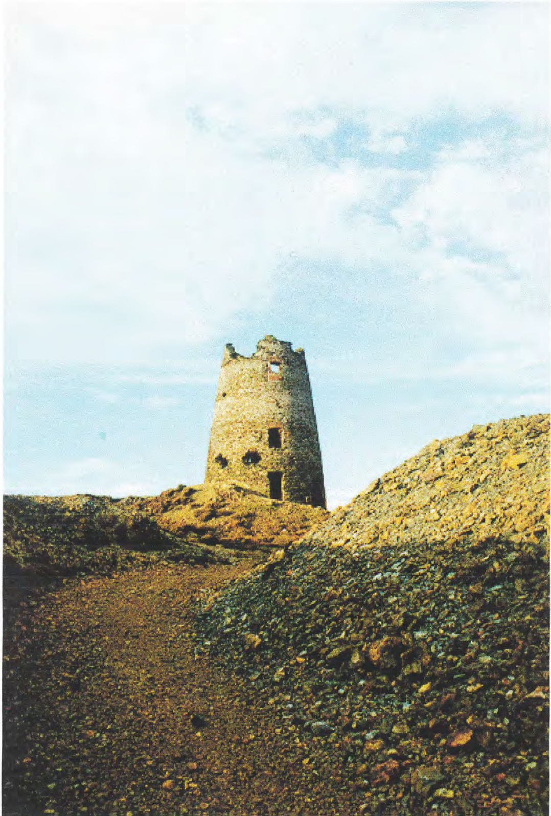
3 The Mona Mine windmill (feature no. 74) was constructed in 1878, and operated a pump by means of 200 feet of flat-rods. It was supplemented from 1880 by a steam engine. Uniquely for Anglesey, it was a five sail mill, and is believed to be the only surviving mine pump windmill in Britain. It is a Scheduled Ancient Monument.
