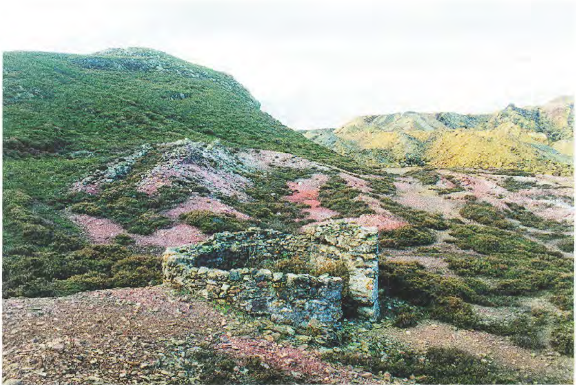
4 The Monna Mine, looking west. In the foreground stand the remains of the magazine (feature no. 293) and beyond a number of the sulphur calcination kilns and their associated stone-built flues (feature nos. 300-303). The distinctive pinkish spoil is a sign of calcination having been carried out.
