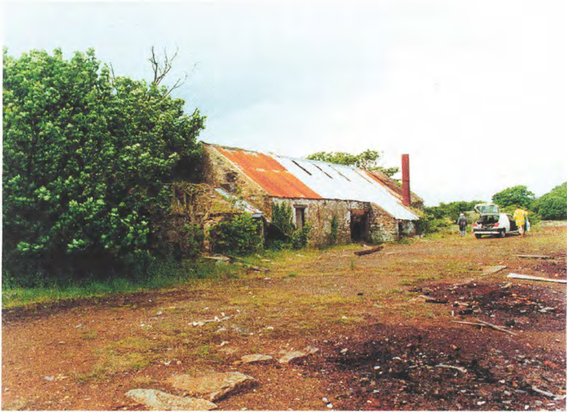
1 The Dyffryn Adda furnace (feature no. 387) was constructed in the early years of the nineteenth century for drying the copper precipitate from the Joint Level which drained both the Parys and the Mona mines. It remained in use until 1958, when the precipitation system was finally abandoned. Its situation near the Amlwch to Llanerchymedd road makes it an easy target for vandals.
