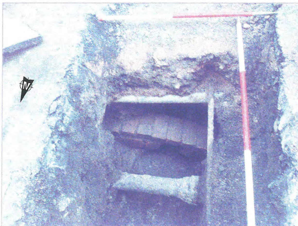
Plate 4. Brick drain visible on the north side of the parapet wall (below)
