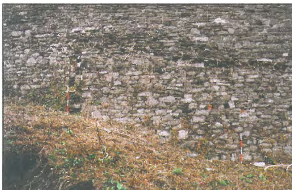
Fig. 12 Conwy town wall, showing 19th century re-facing and bonding for glass-house wall (1m scales 5m apart)
