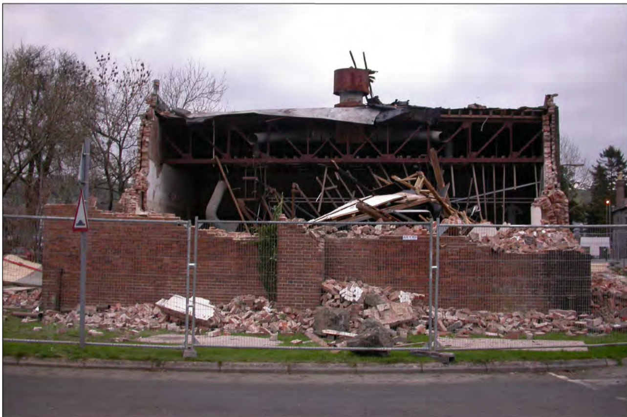
Plate 15. East view of the demolition of the west of the building, including the stage area. Image shows ceiling girders and pipes. G1850/04/04
