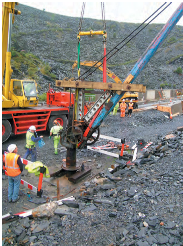
Plate 8 Removal of the upper part of Crane 3(13)
