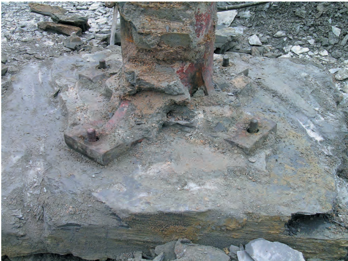
Plate 10 Site 1(13) The crane pillar: flanges and block
