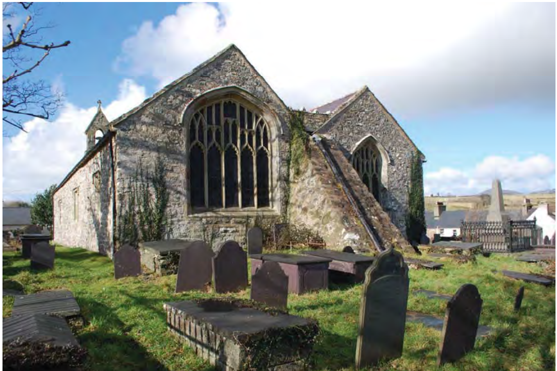
Fig. 11 General view of Abererch Church from the south east. The study area is immediately behind the south wall to the left of the picture.
