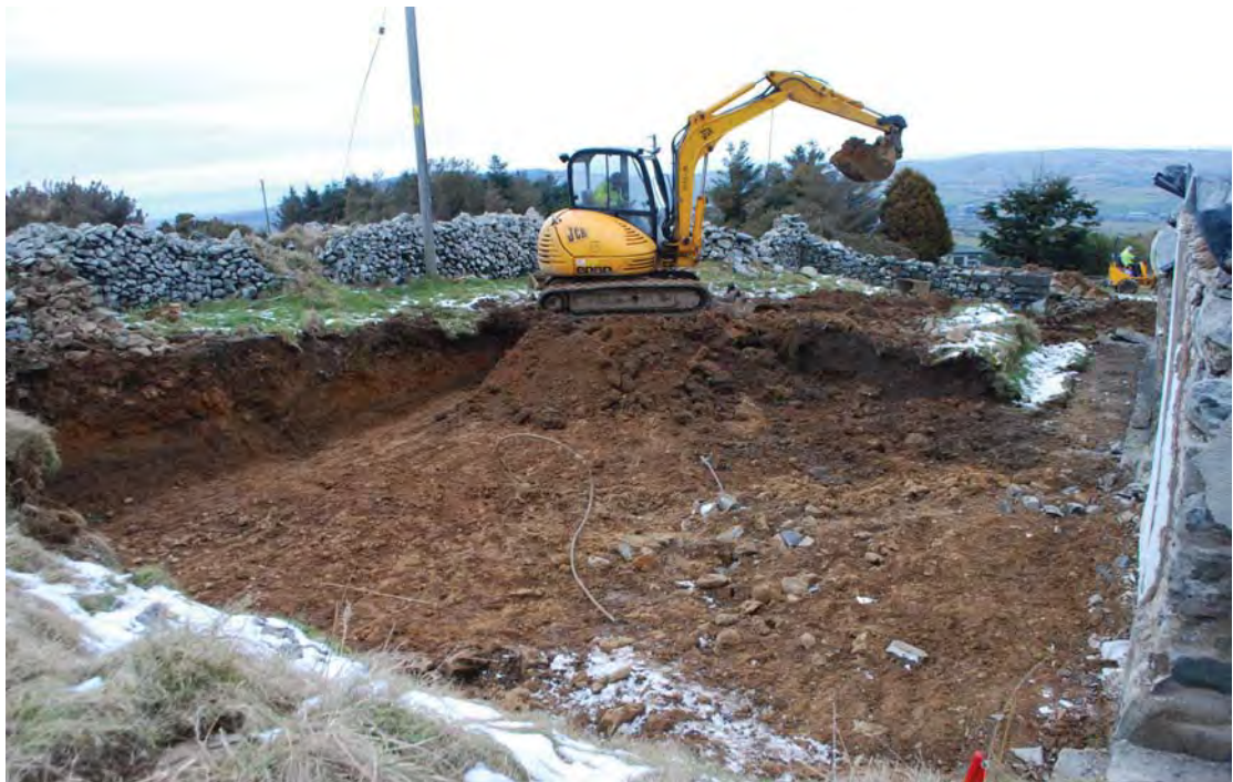
Plate 2 The development plot from the south-west
