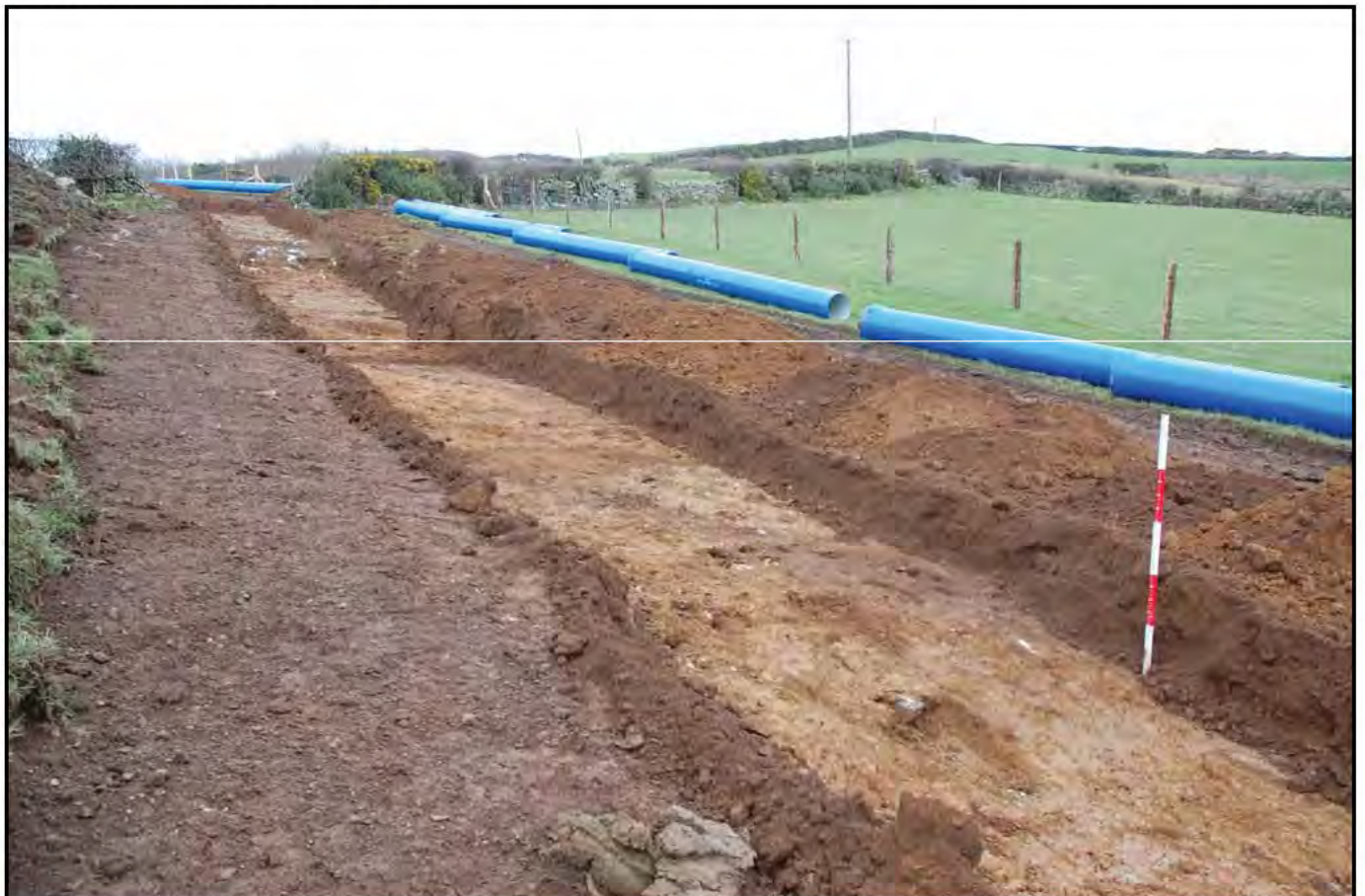
Plate 32 - Llangefni to Penmynydd replacement main: view north at scheme end point, detailing the easement, the strip/map/sample zone and the pipe drop. Note the glacial drift geology at 0.50m below ground surface level. Two post-medieval drainage ditches are visible close to the ranging pole. Bedrock is visible towards top of image. The replacement main terminated at the Penmynydd reservoir.
