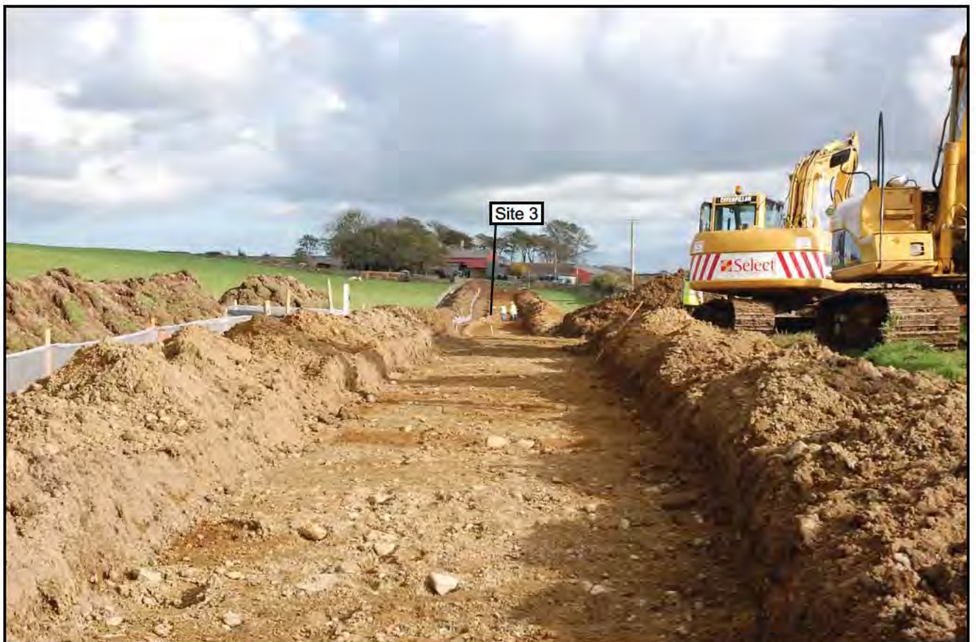
Plate 04 - Gwalchmai to Bodffordd link main: opposite view of Plate 03, looking east, detailing strip/map/sample of pipeline route. Note general location of Site 3 in a low point of the field.
