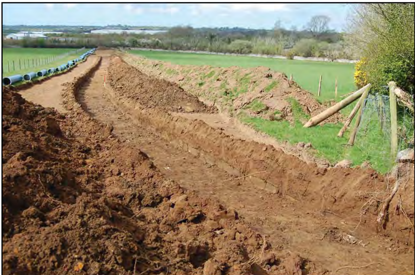
Plate 12 - Llangefni to Penmynydd replacement main: view west of the start of the scheme detailing easement width and strip/map/sample zone. The topsoil was up to 0.40m thick in this area, atop a silt-rich glacial deposit.
