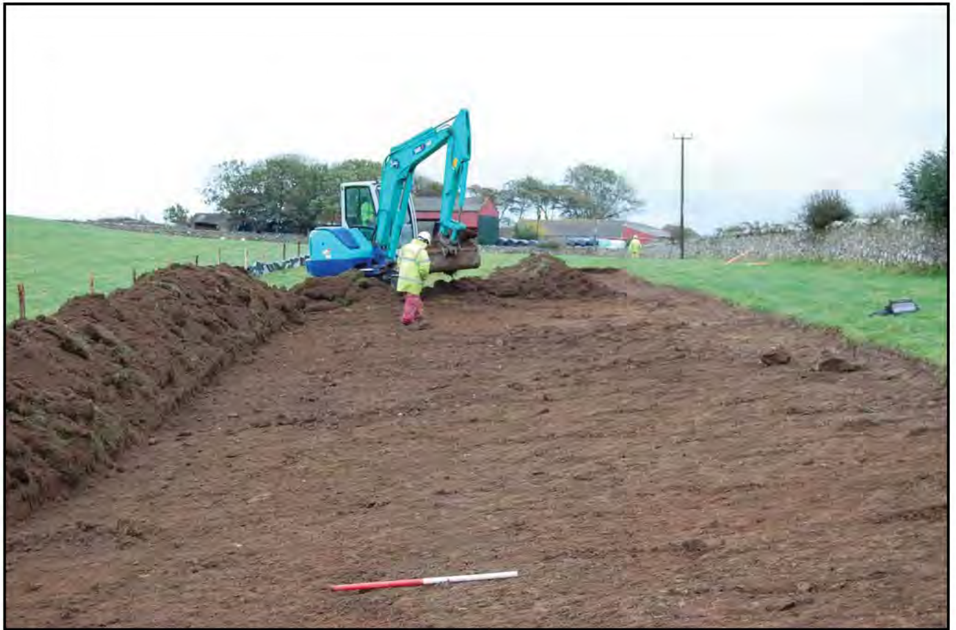
Plate 03 - Gwalchmai to Bodffordd link main: view west toards scheme start point detailing topsoil strip within easement. This field was the location of Site 3 (cf. Plate 04)
