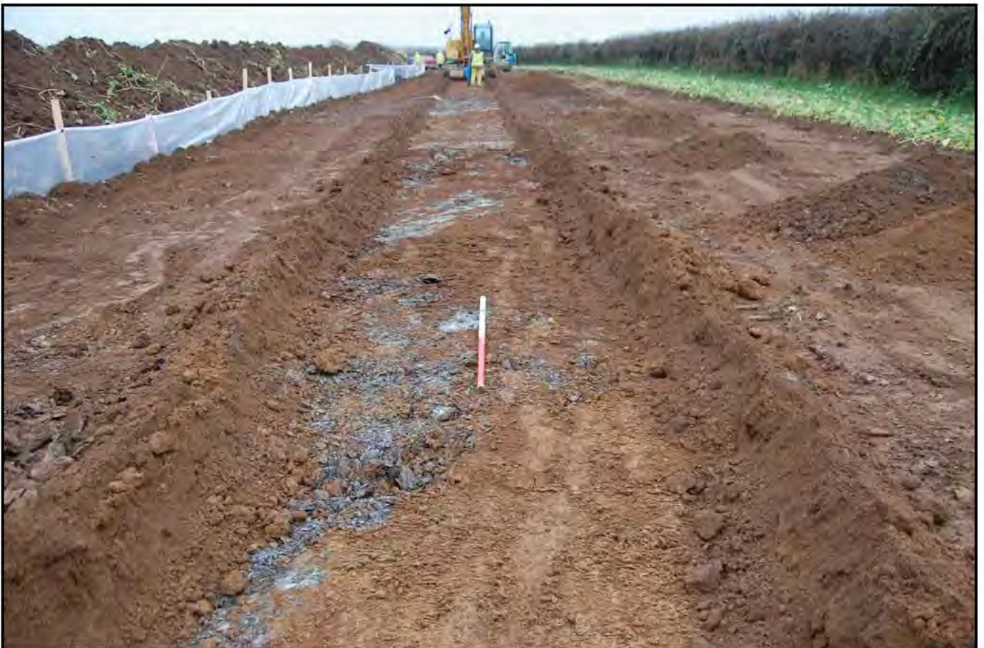
Plate 10 - Gwalchmai to Bodffordd link main: view west of easment and strip/map/sample route detailing the exposed bedrock that characterised the 3.0km point of the scheme.
