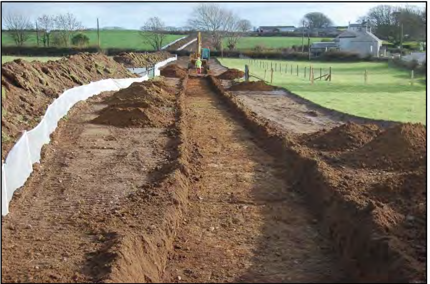
Plate 09 - Gwalchmai to Bodffordd link main: opposite view to Plate 08, detailing easment route and strip/map/sample zone at c.2.5km along the scheme. The geology is visible as a clay-silt drift
