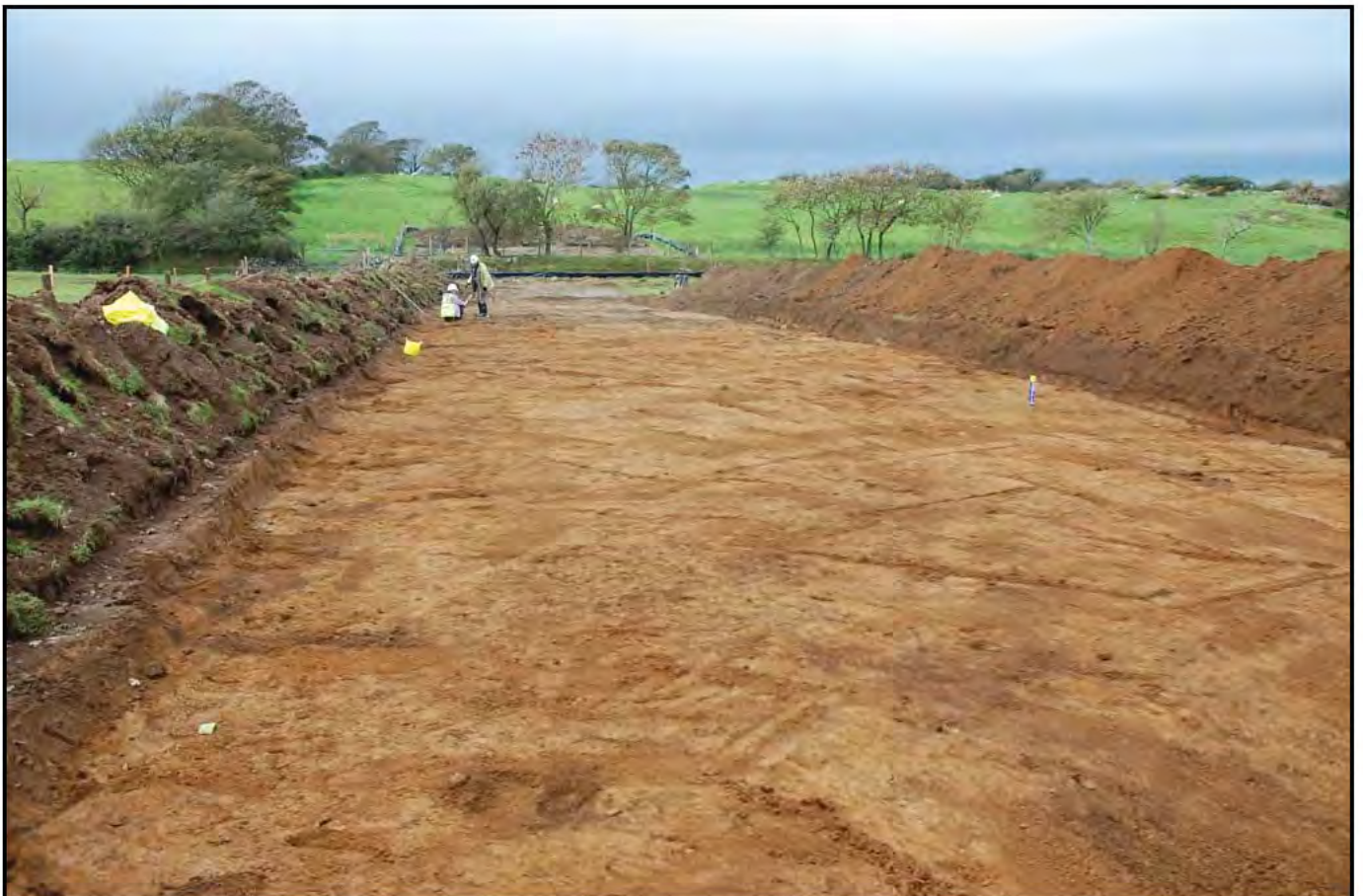
Plate 02 - Gwalchmai to Bodffordd link main: view west of scheme at start point detailing full easement strip. The natural at this location was identified as morrainic drift
