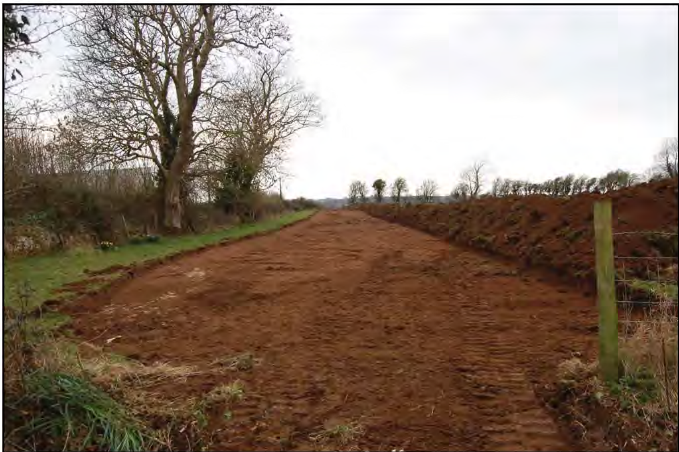
Plate 13 - Llangefni to Penmynydd replacement main: view east from start point during easement strip. Note the natural limestone ridge towards left of image
