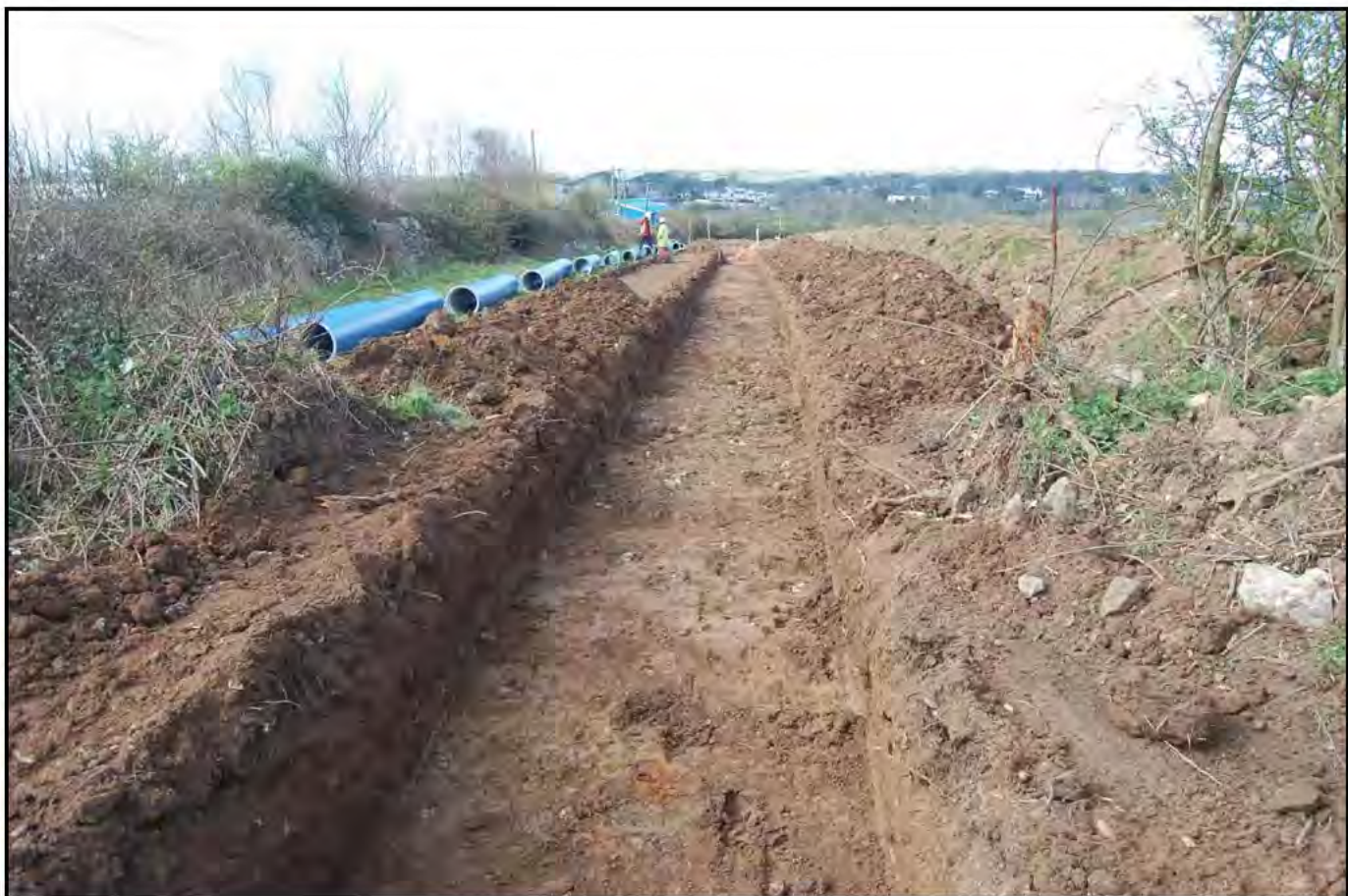
Plate 14 - Llangefni to Penmynydd replacement main: view west towards start of scheme at c.0.5km point detailing strip/map/sample zone, associated depth and exposed natural (clay-silt). Topsoil/Subsoil was up to 0.60m thick at this locaiton. Note replacement main towards left of image.
