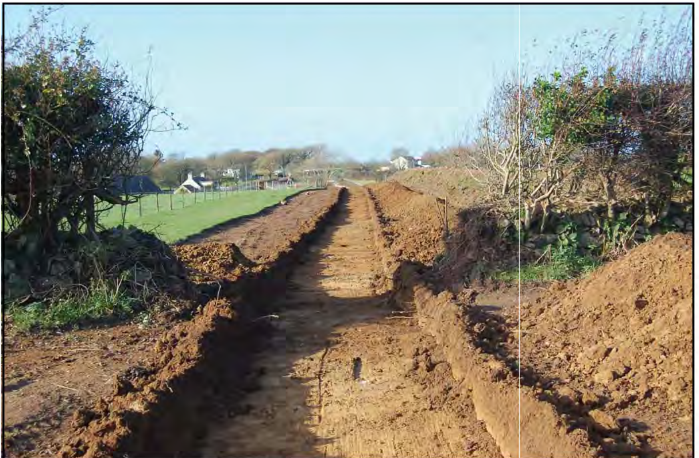
Plate 08 - Gwalchmai to Bodffordd link main: general view west c.2.5km along the scheme detailing easement and strip/map/sample route. The visible geology at this locaiton was a glacial drift.
