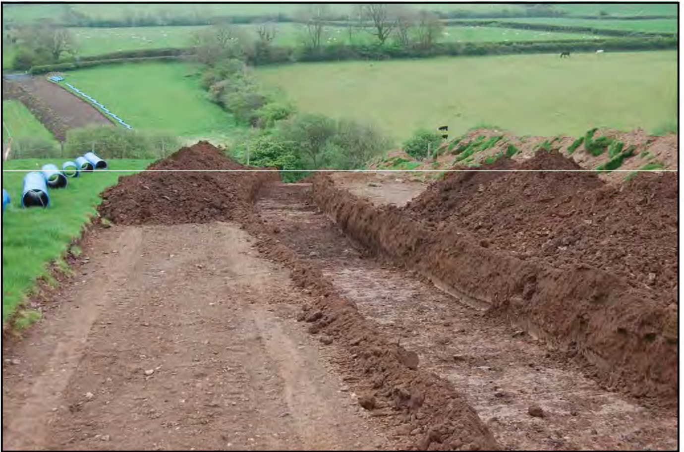
Plate 25 - Llangefni to Penmynydd replacement main: General view east of the scheme c.2.0km along the route, detailing the easement strip, the strip/map/sample zone and the pipe drop. The glacial deposit is visible at the base of the strip/map/sample zone
