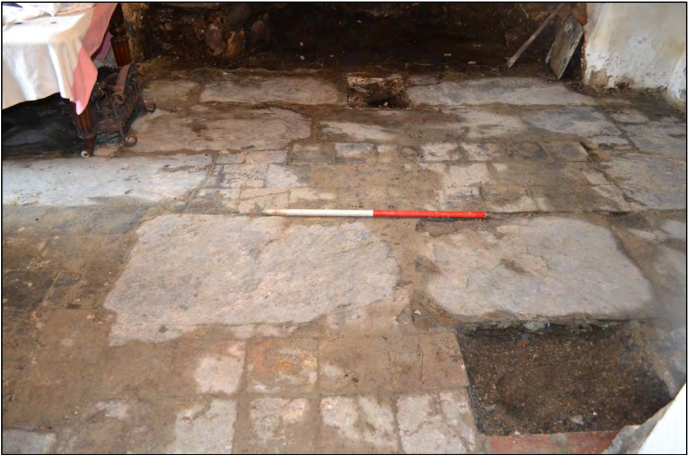
Plate 19: Former Hall floor revealed, from the southeast
