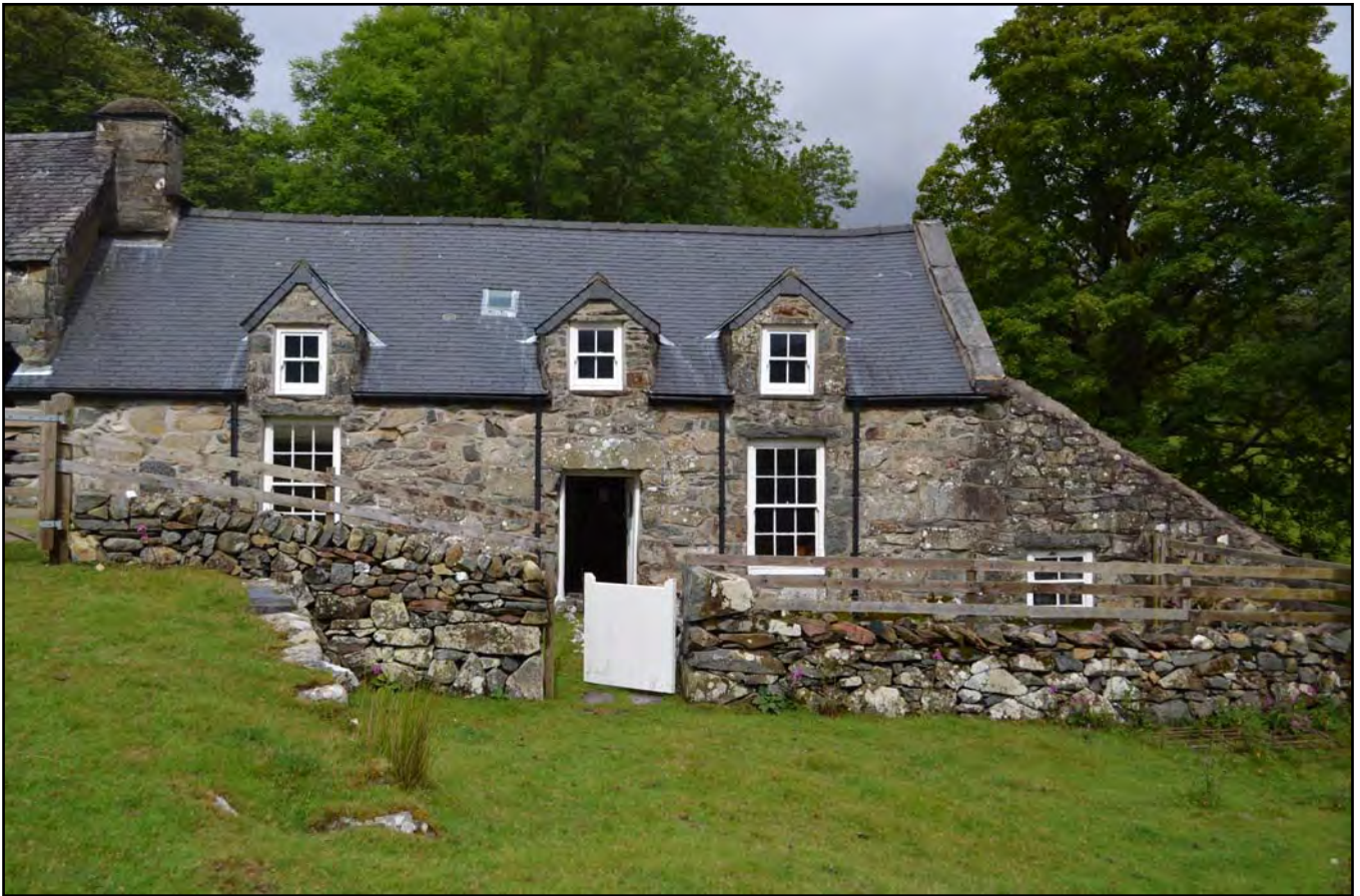
Plate 1: Southeast facing external elevation
