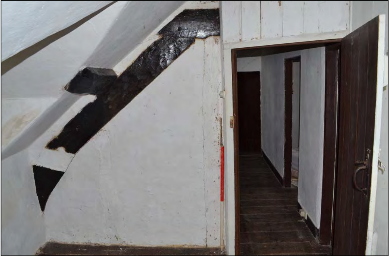
Plate 17: Bedroom 5 showing roof truss from the northeast
