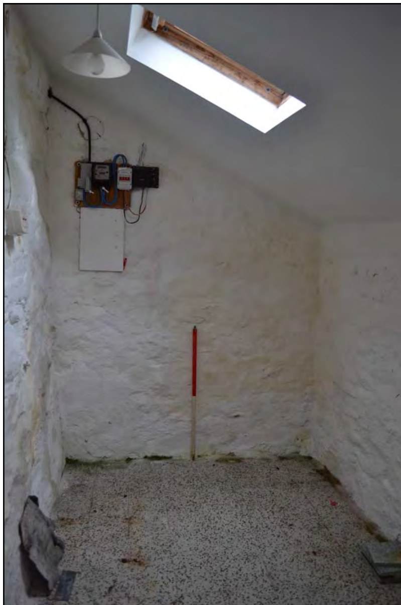
Plate 7: Kitchen from the southwest
