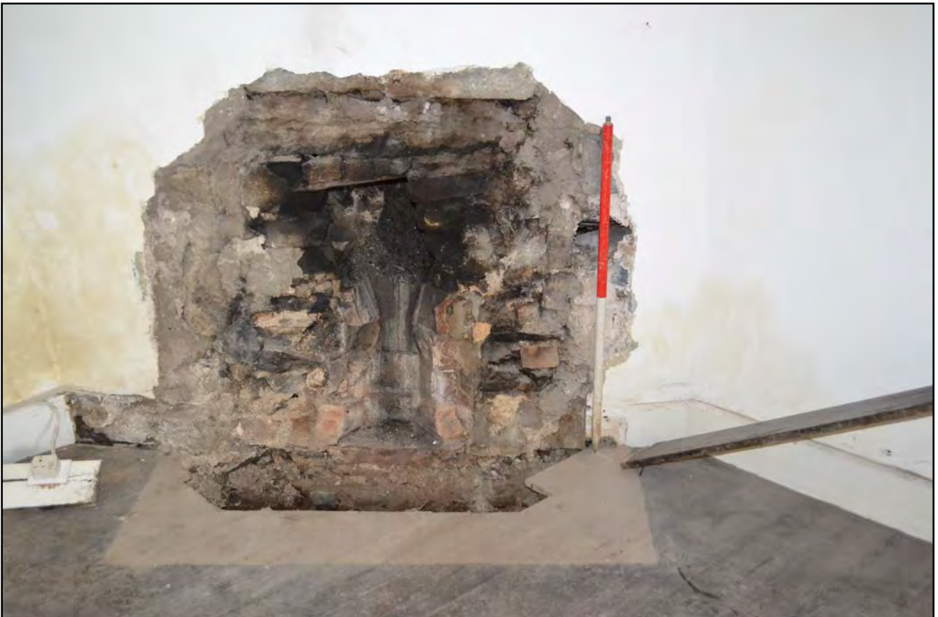
Plate 18: Parlour fireplace removed, from the south
