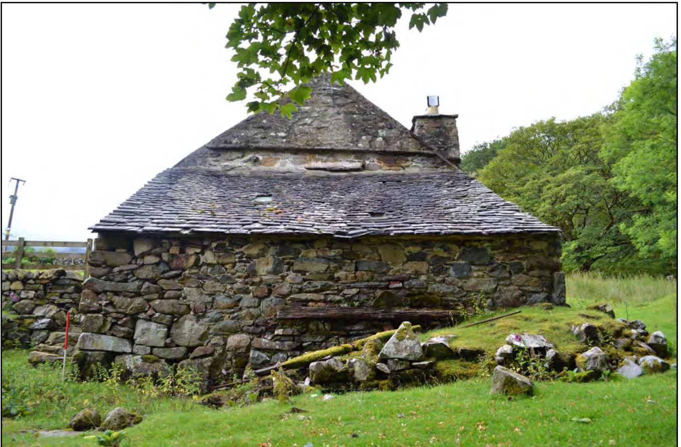
Plate 2: Northeast external elevation showing waterwheel pit
