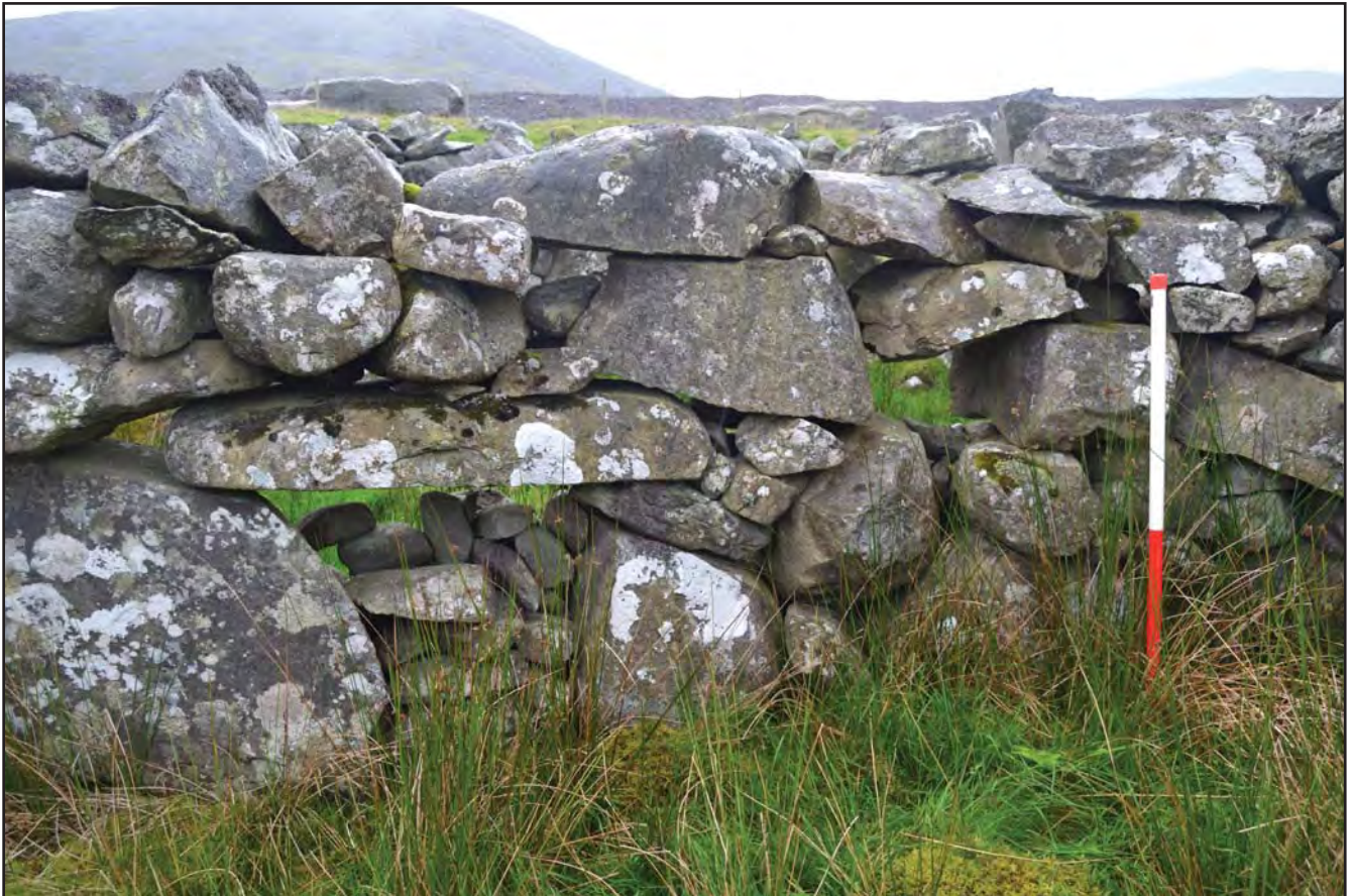
Plate 23. Sheep creep from Cell 11 into Cell 10 blocked with small stones. View from north-west, scale 1m (archive reference: G2534_2023_112)
