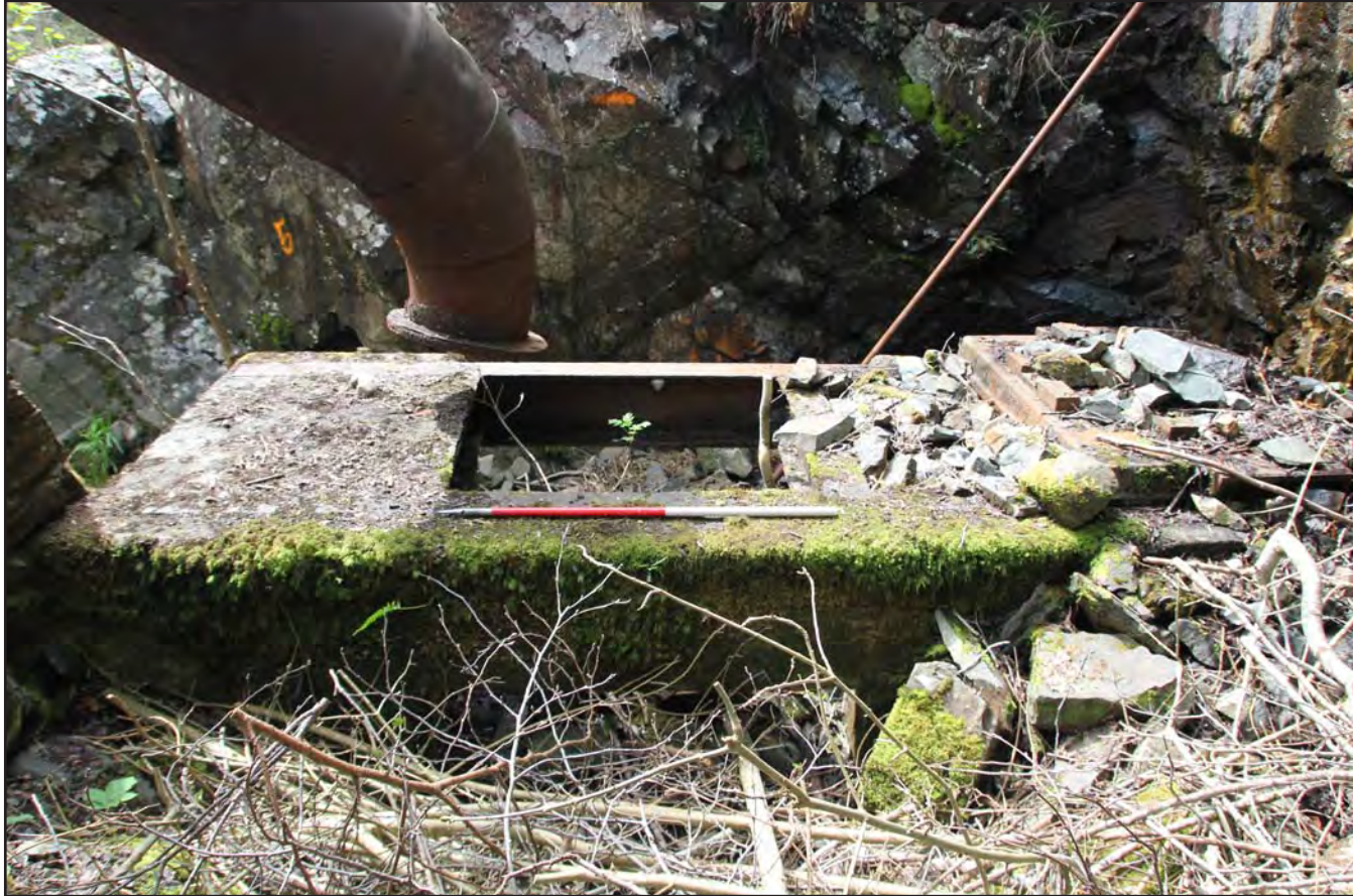
Plate 30: Turbine shaft feature 9 showing Armfield of Ringwood turbine base, from the north. Scale 1.0m.
