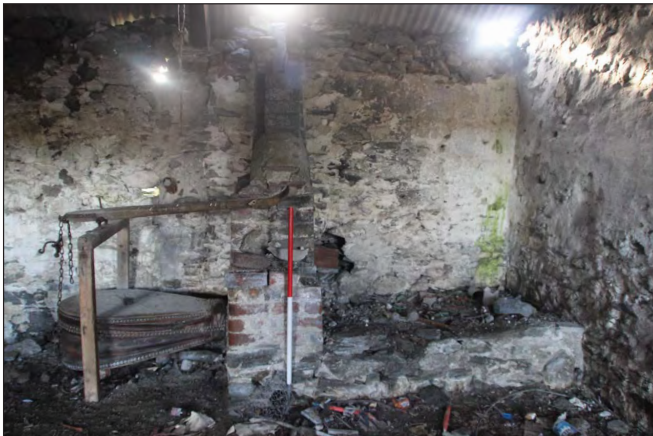
Plate I-11: Cleifiog Fawr Unit 8 forge showing bellows and furnace, from the north. Scale 1.0m.
