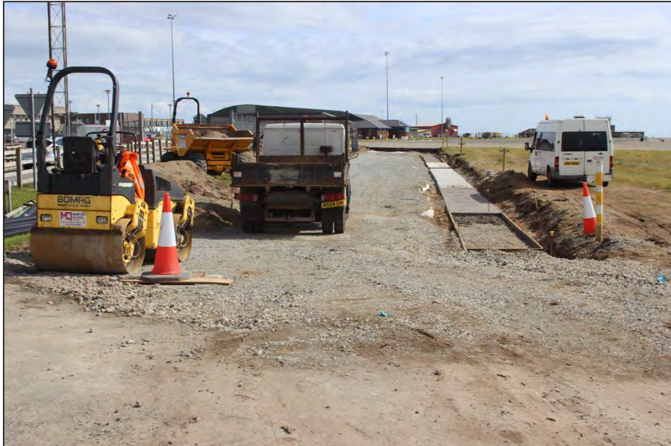
Plate 33: Perimeter road stoned up and concreted (600.0m to 650.0m) - from the north - no scale
