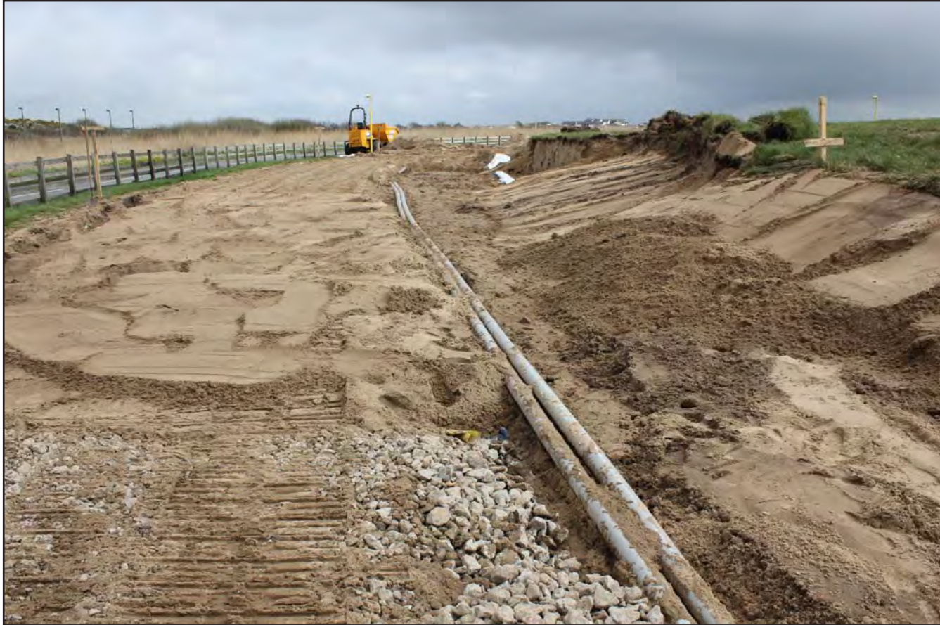
Plate 28: Batter ahead of temporary shut down ahead of reopening of Runway 19 (lowered services also shown) - from the west - no scale
