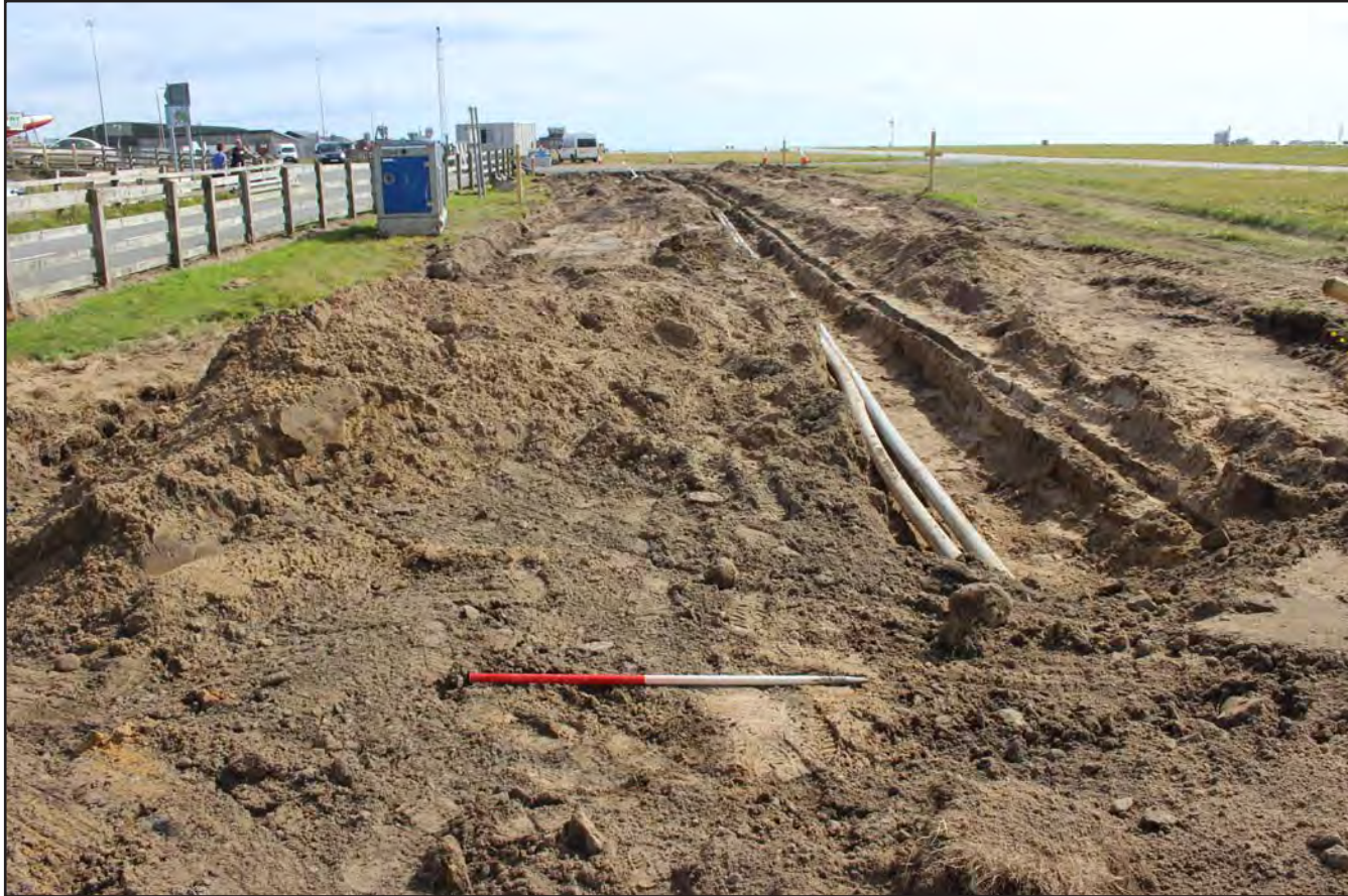
Plate 32: Perimeter road topsoil strip to north of Runway 19 (550.0m to 600.0m) - from the north - 1m scale
