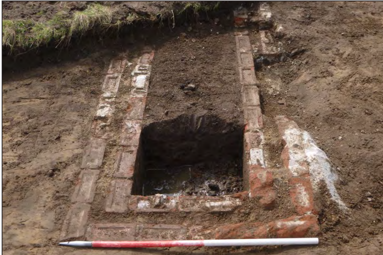
Plate 23: Inspection pit uncovered during CCB excavation - from the north - 1m scale
