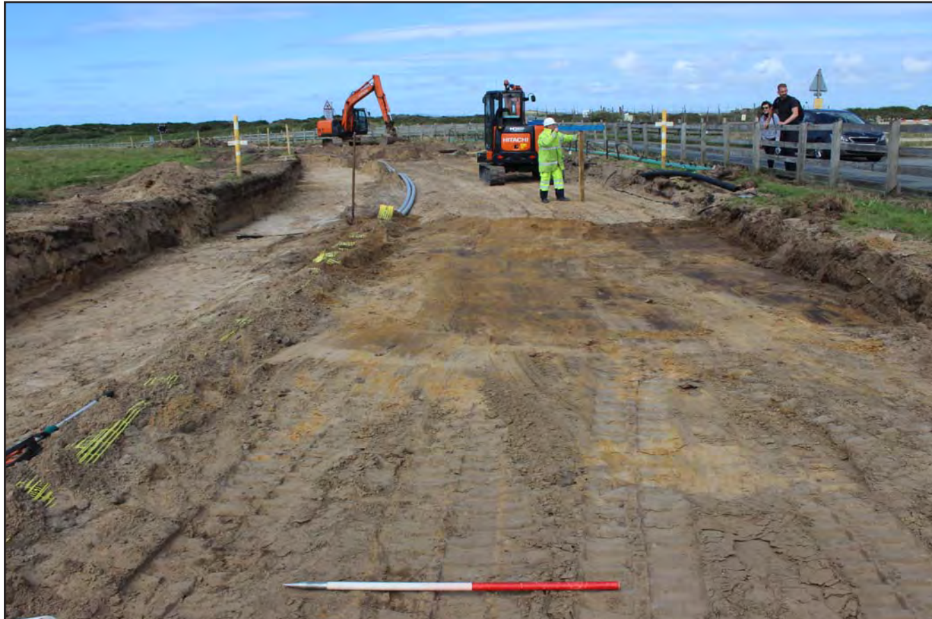
Plate 30: Perimeter road topsoil strip to north of Runway 19 (500.0m to 450.0m) - from the south - 1m scale
