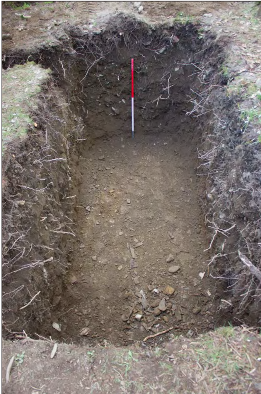
Plate 12: Section shot for septic tank trench, at St. Mary's Church, Church Street, Llanfair Talhaiarn, Conwy - from the east - 1.00m scale
