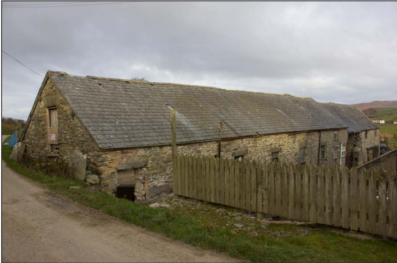
Plate 09: Oblique shot of southern and eastern elevations of outbuilding, at Cefnhirfynydd Isa, Glasfryn, Conwy - from the southeast - no scale
