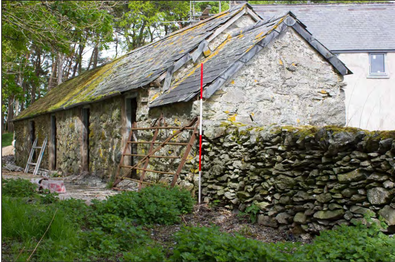
Plate 41: Oblique shot of northwest & southwest elevations of Building 3 - Pigsties at Gaer Gerrig, Llangwm, Conwy - from the southeast - 2.00m scale
