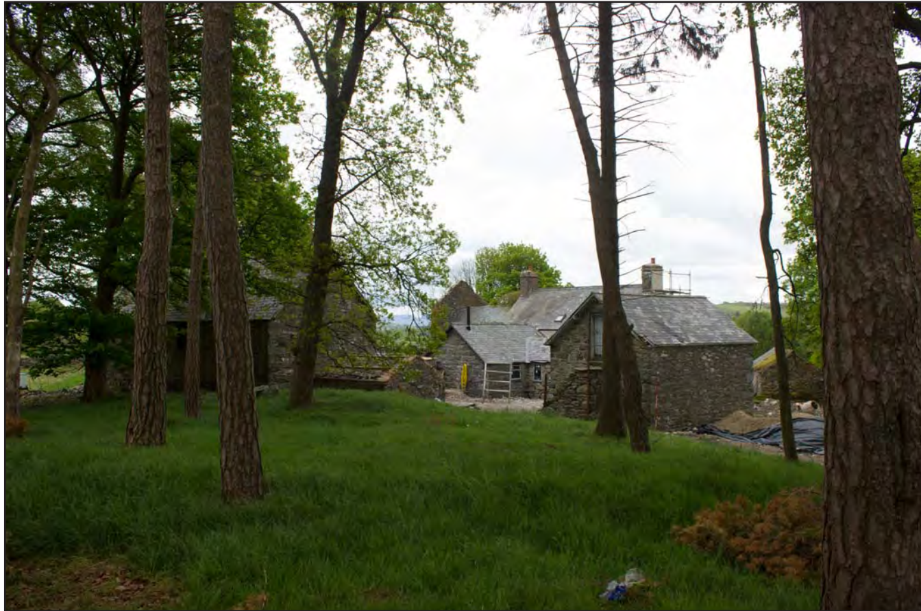
Plate B: Context shot of Gaer Gerrig farm complex - Llangwm, Conwy - from the west-northwest - 2.00m scale
