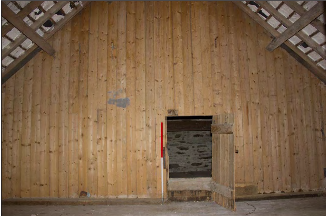
Plate 22: Store 2, First Floor, within Building 1 - Cart and Threshing Barn at Gaer Gerrig, Llangwm, Conwy - from the northeast - 1.00m scale
