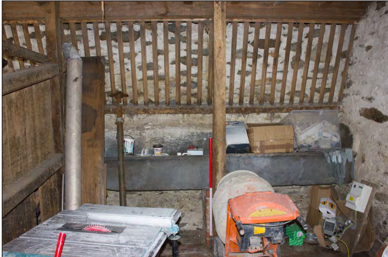
Plate 35: Horse stall (right) within Building 2 - Horse/Pony Stable at Gaer Gerrig, Llangwm, Conwy - from the northeast - 1.00m scale
