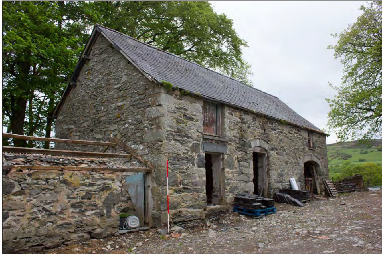
Plate 13: Oblique shot of southwest & southeast elevations of Building 1 - Cart and Threshing Barn at Gaer Gerrig, Llangwm, Conwy - from the southeast - 2.00m scale
