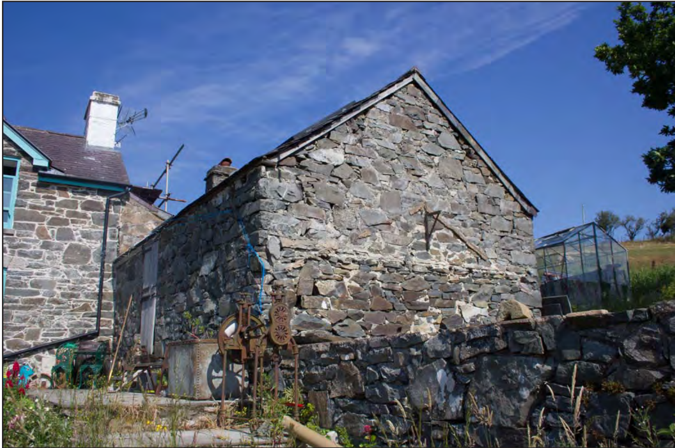
Plate 05: South and east facing external elevations, from the southeast. Scale 1.0m.
