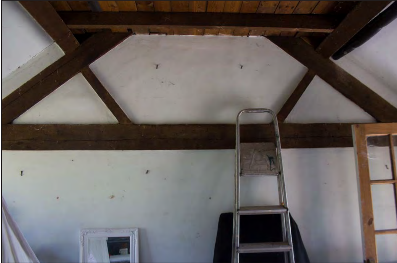
Plate 17: Barn 2 showing truss, from the west.
