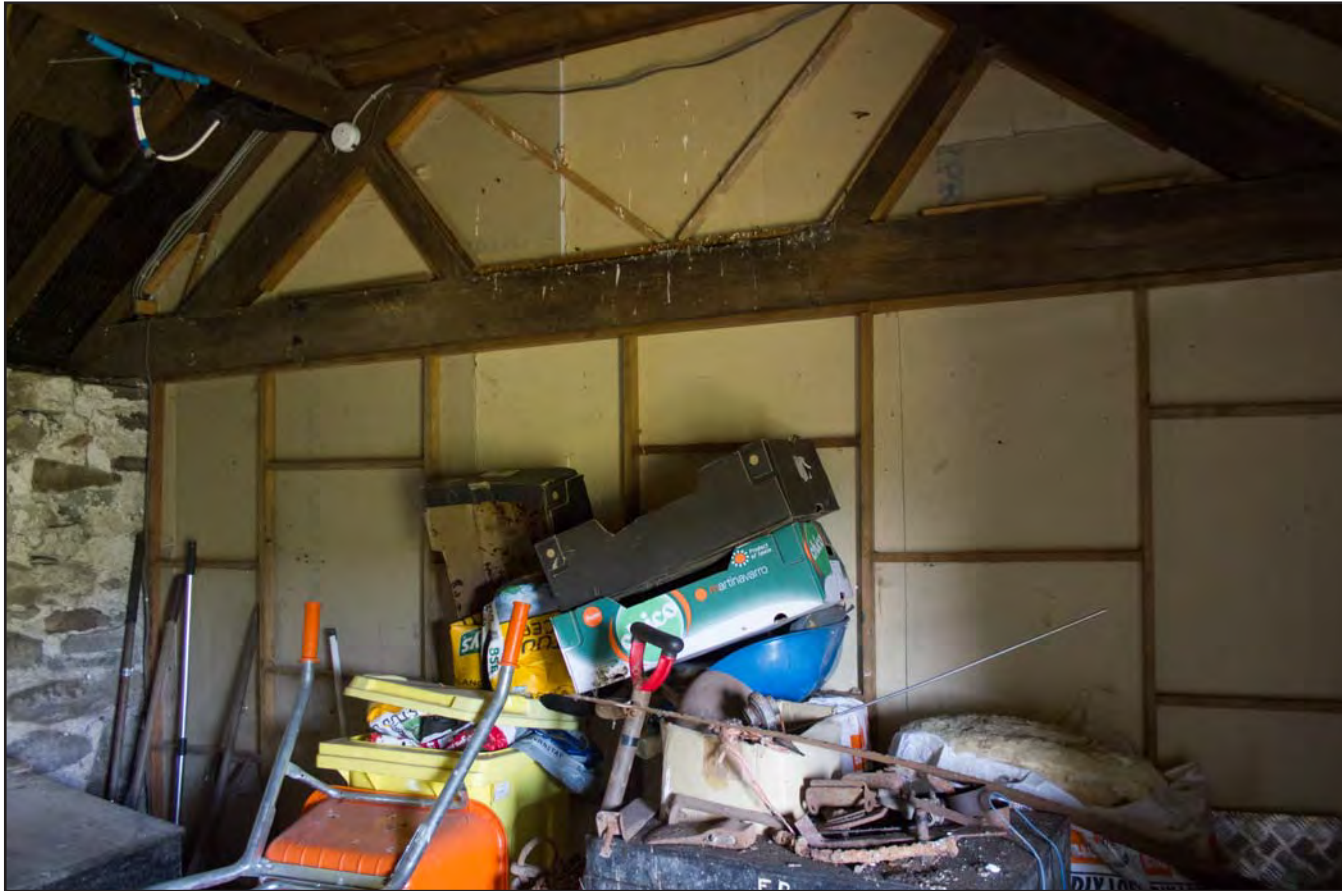
Plate 13: Barn 1 showing truss, from the northeast.
