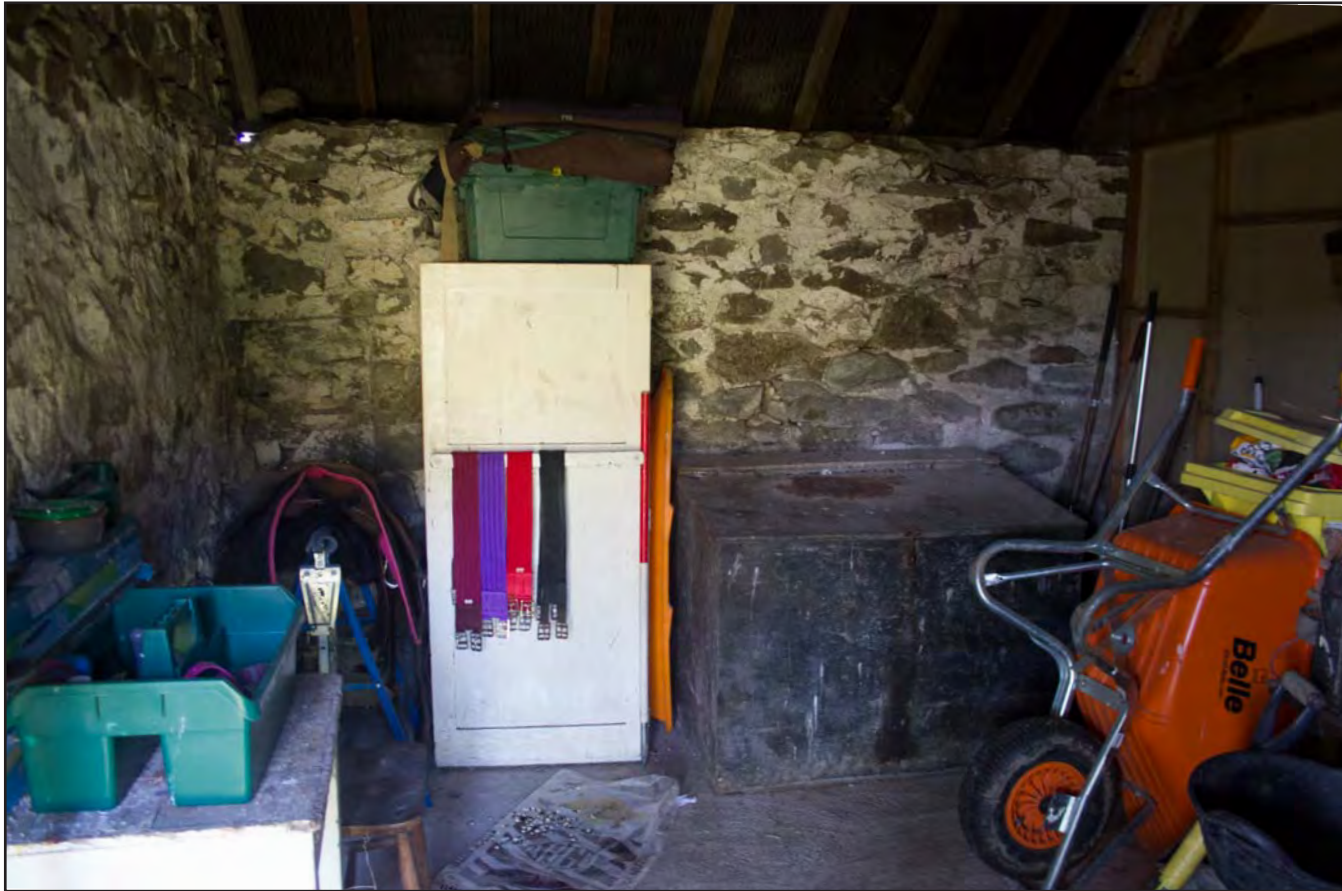
Plate 11: Barn 1, from the north. Scale 1.0m.
