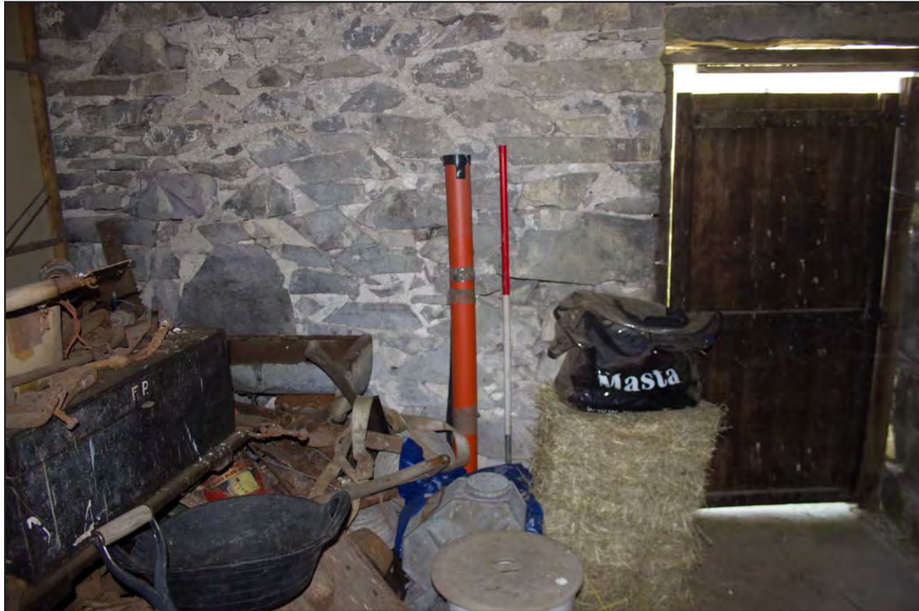
Plate 12: Barn 1, from the south. Scale 1.0m.
