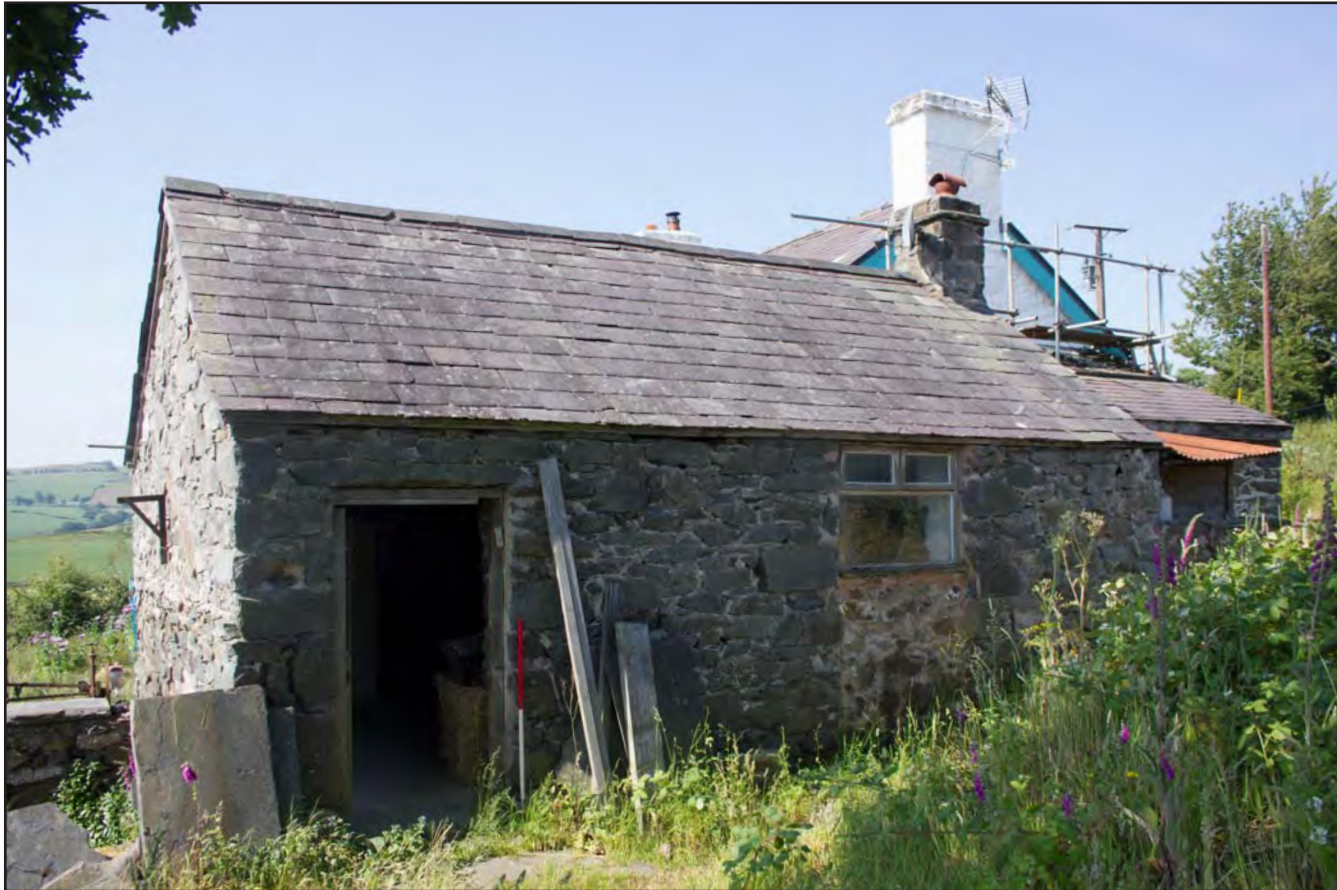
Plate 08: North facing external elevation, from the northeast. Scale 1.0m.
