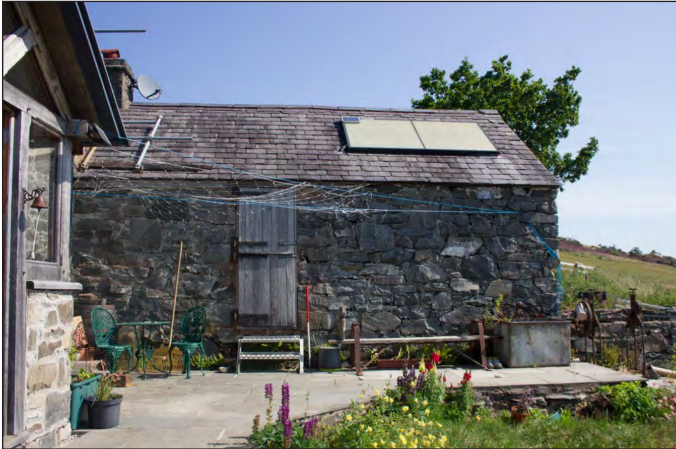
Plate 04: South facing external elevation, from the south. Scale 1.0m.
