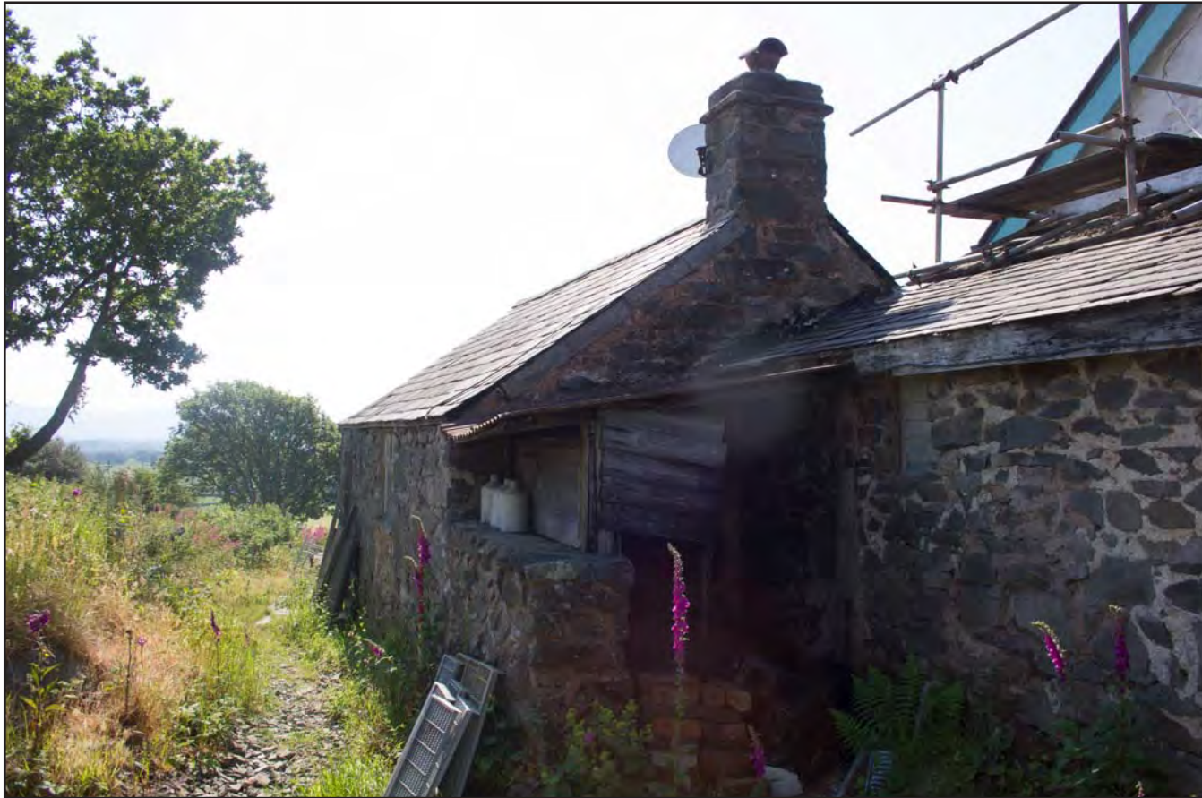
Plate 10: North and west facing external elevations, from the northwest. Scale 1.0m.
