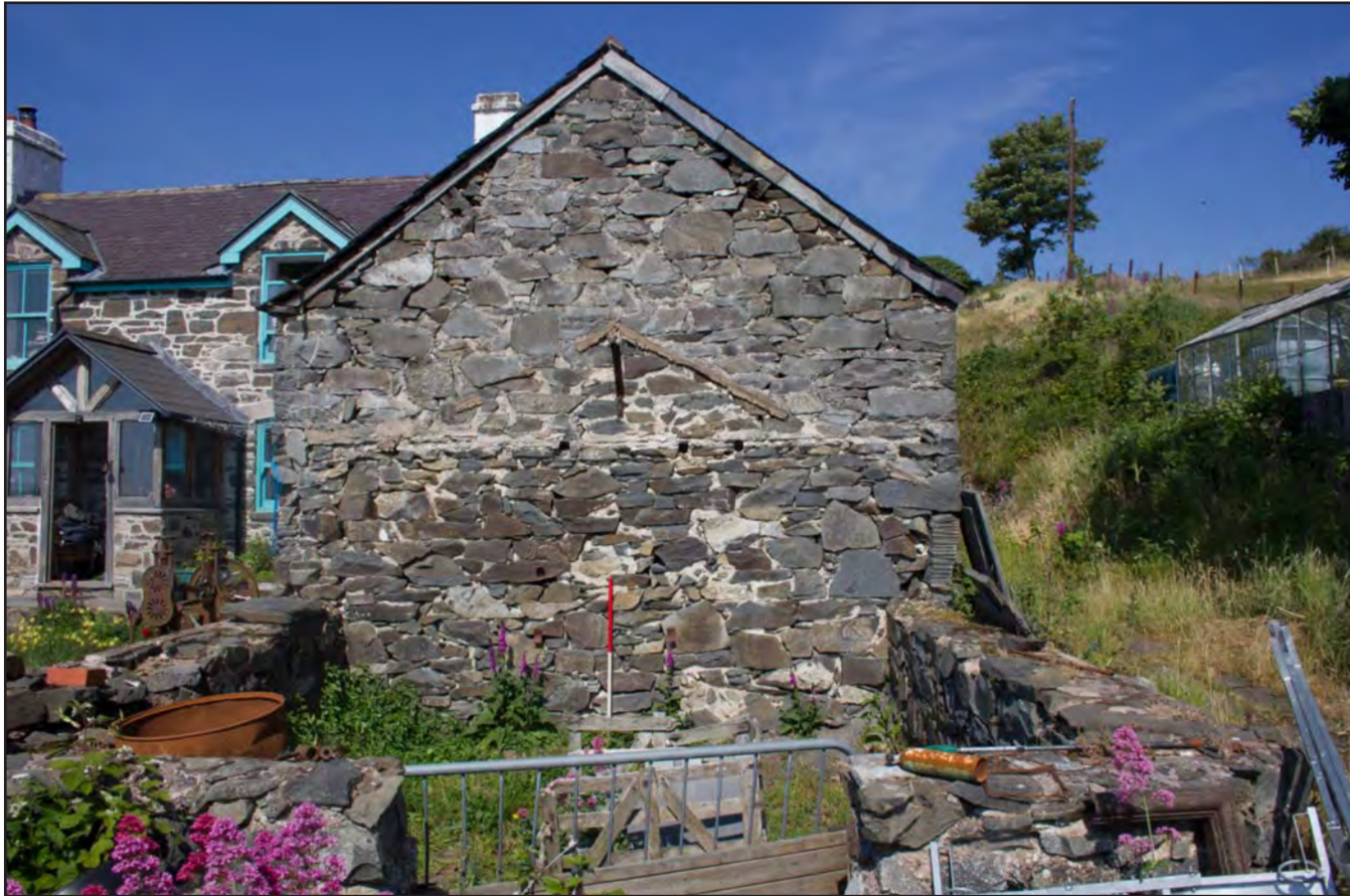
Plate 06: East facing external elevation, from the east. Scale 1.0m.
