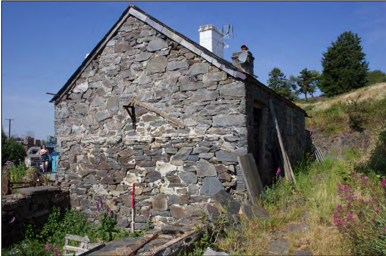
Plate 07: East and north facing external elevations, from the northeast. Scale 1.0m.
