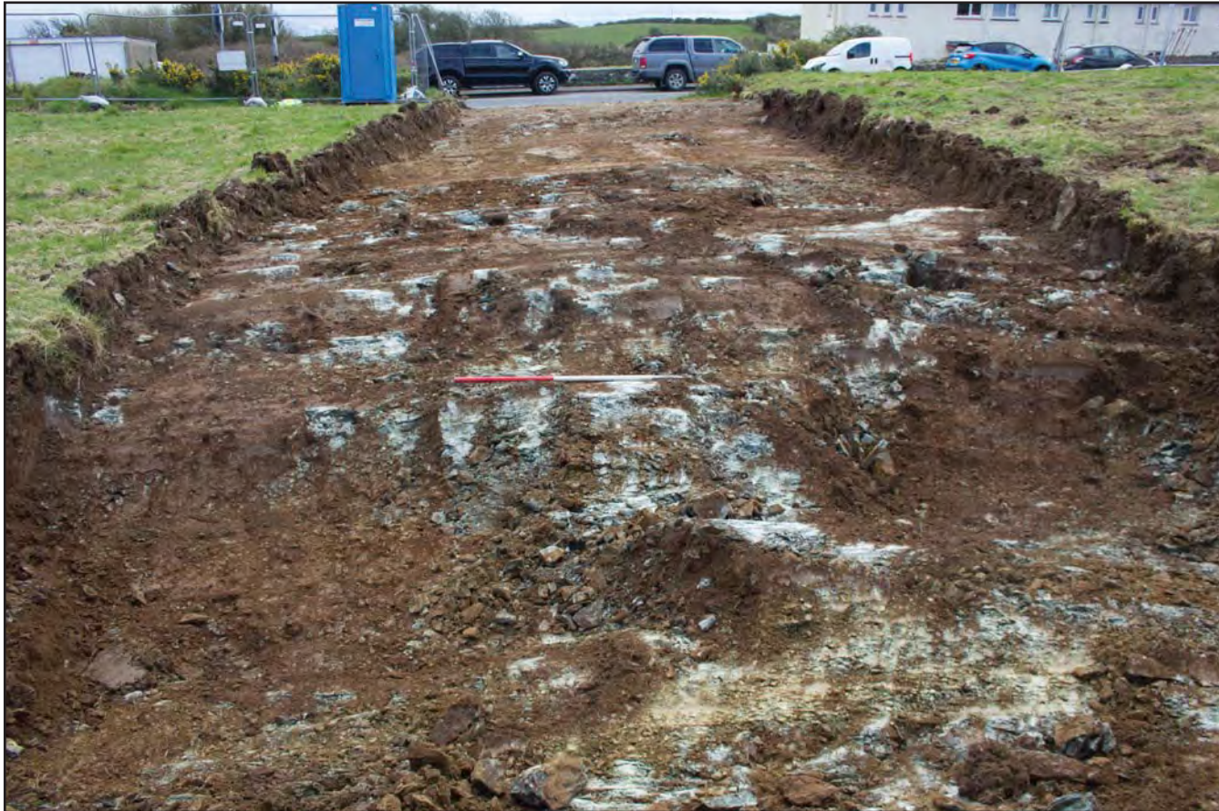
Plate 04: Stripped access / haul route onto Site, from the northwest. Scale 1.0m.
