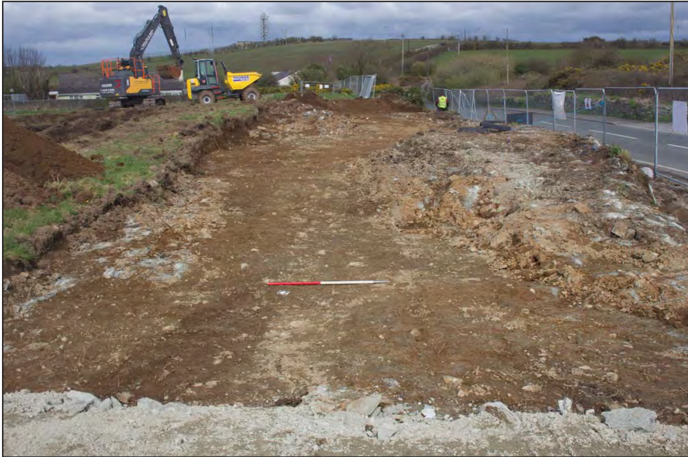
Plate 08: Perimeter Site strip, from the southwest. Scale 1.0m.
