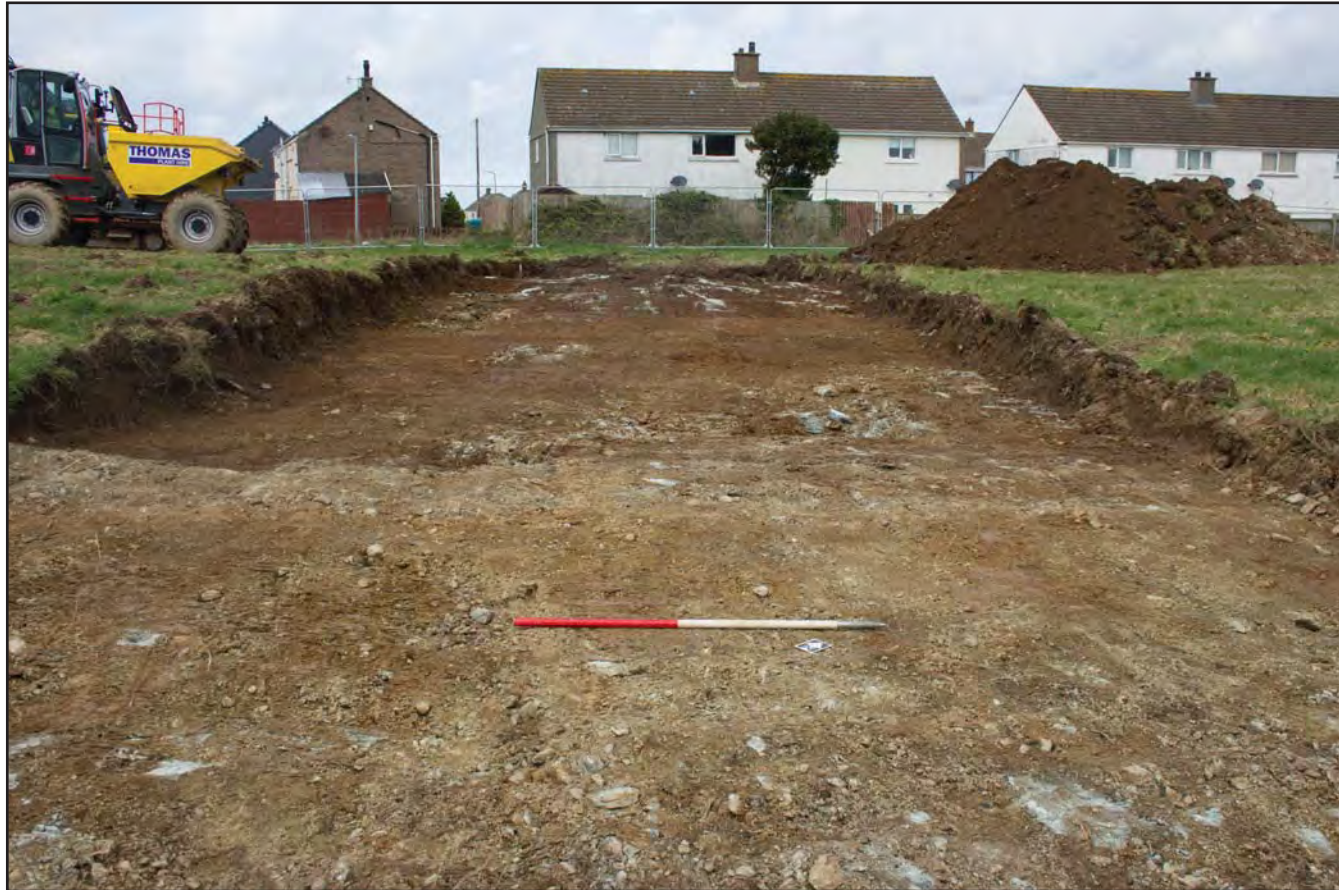
Plate 03: Stripped access / haul route onto Site, from the southeast. Scale 1.0m.
