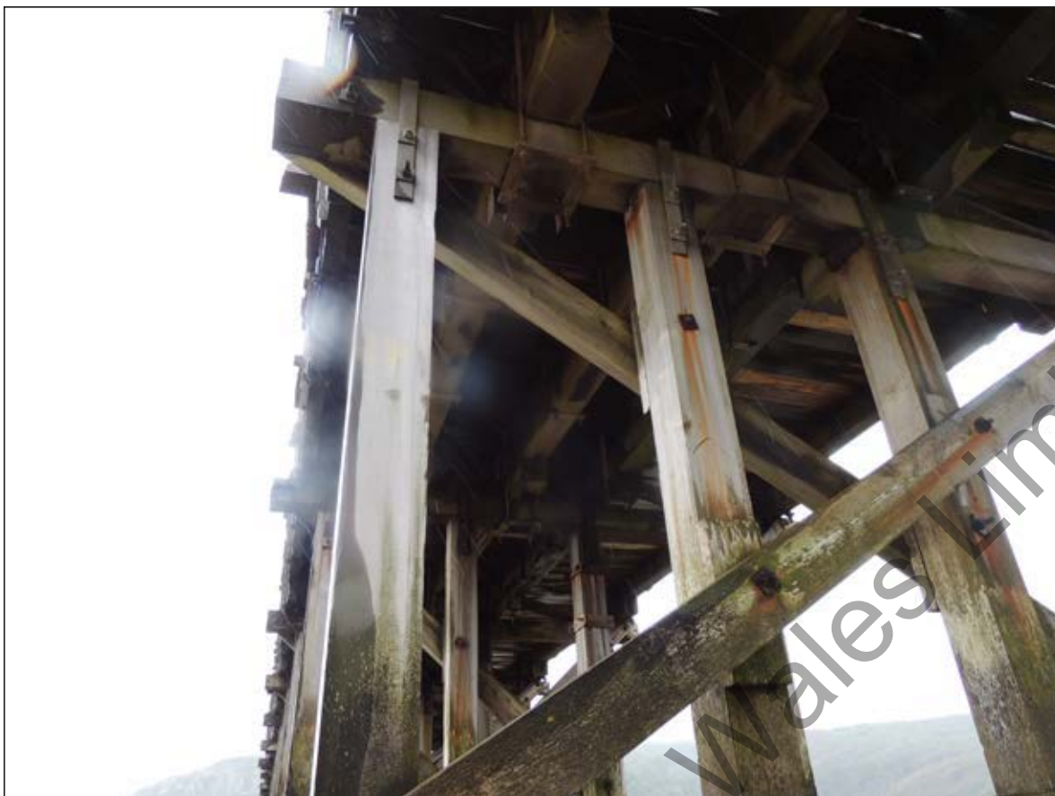
Plate 49. Shot of trestle 26 with replacement verticle piles and galvanised steel straps attached to support beams for transverse deck planks.
