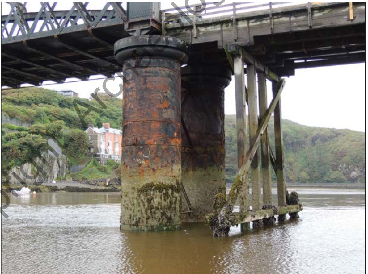
Plate 62. N facing close up of cast iron cylindrical piers.
