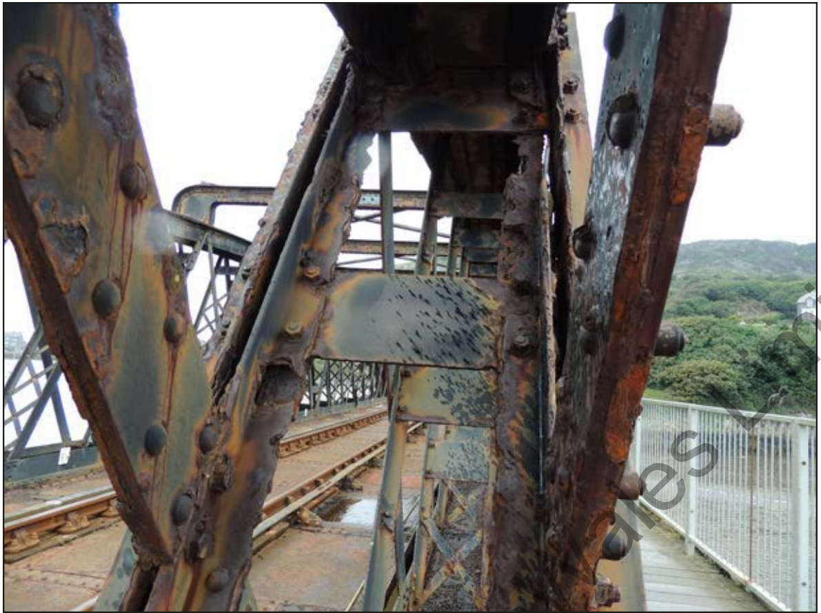
Plate 33. NW facing shot of repairs made to lattice work on the hogback trusses on the span of the viaduct.
