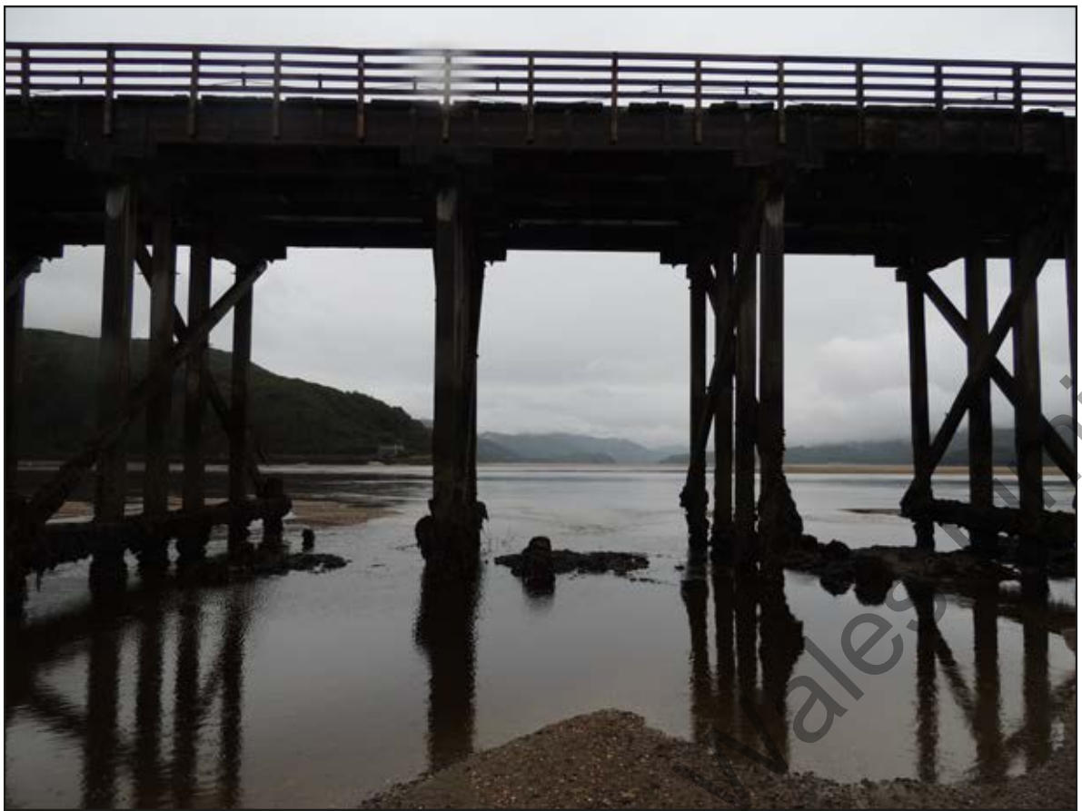
Plate 57. NE facing shot of the remains of old verticle pile stumps under trestle 86, 87, 88.
