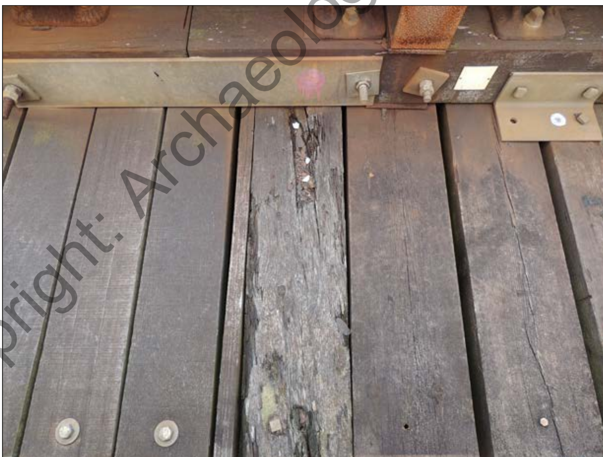
Plate 20. Plan shot of 3 phases of transverse deck plank replacement exemplified by the changing fixtures and preservation of timbers at trestle 50.
