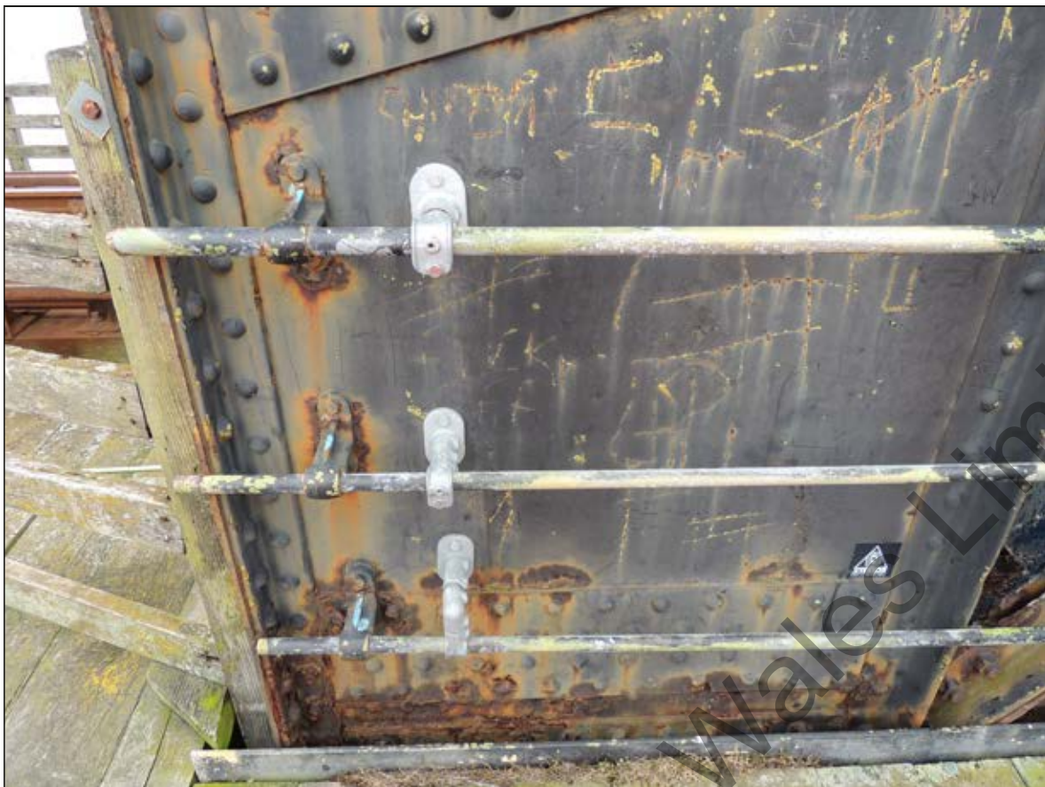
Plate 31. SW facing shot of stainless steel handrail clamps of NE elevation of hogback lattice trusses on the spans of the viaduct.
