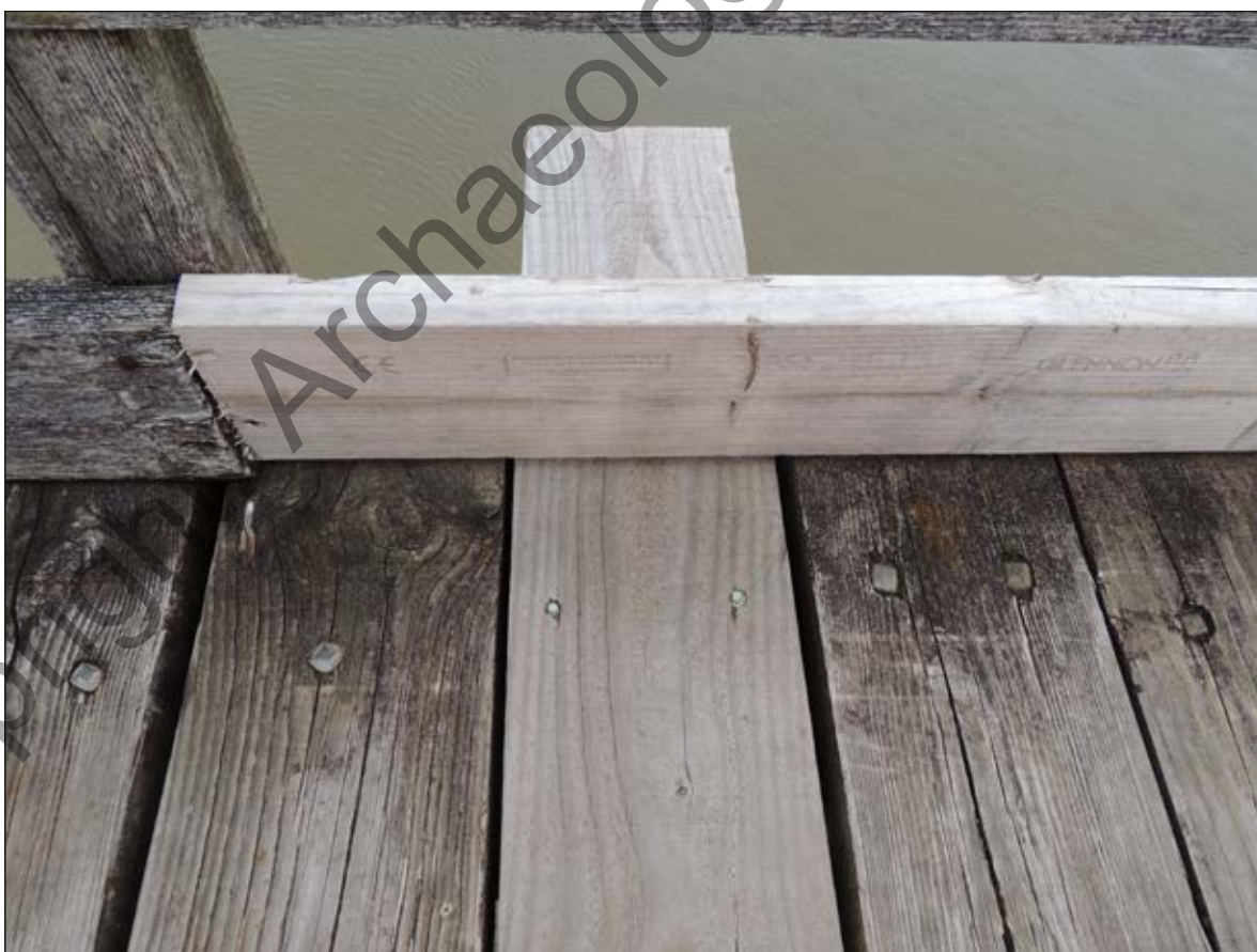
Plate 18. Plan shot of replacement transverse deck planks and kick board on handrail on walkway at trestle 20.
