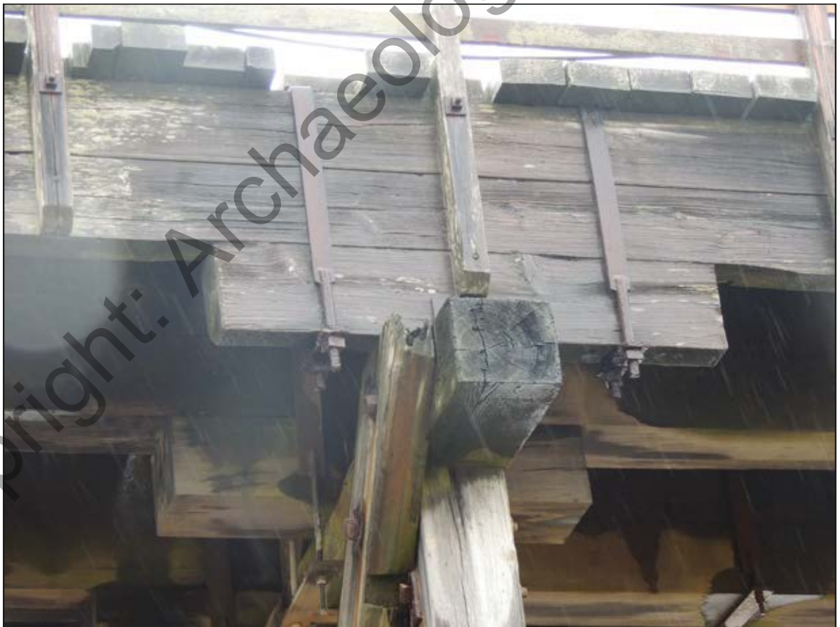
Plate 58. Shot of older steel straps attached to longitudinal outer beam above trestle 86.
