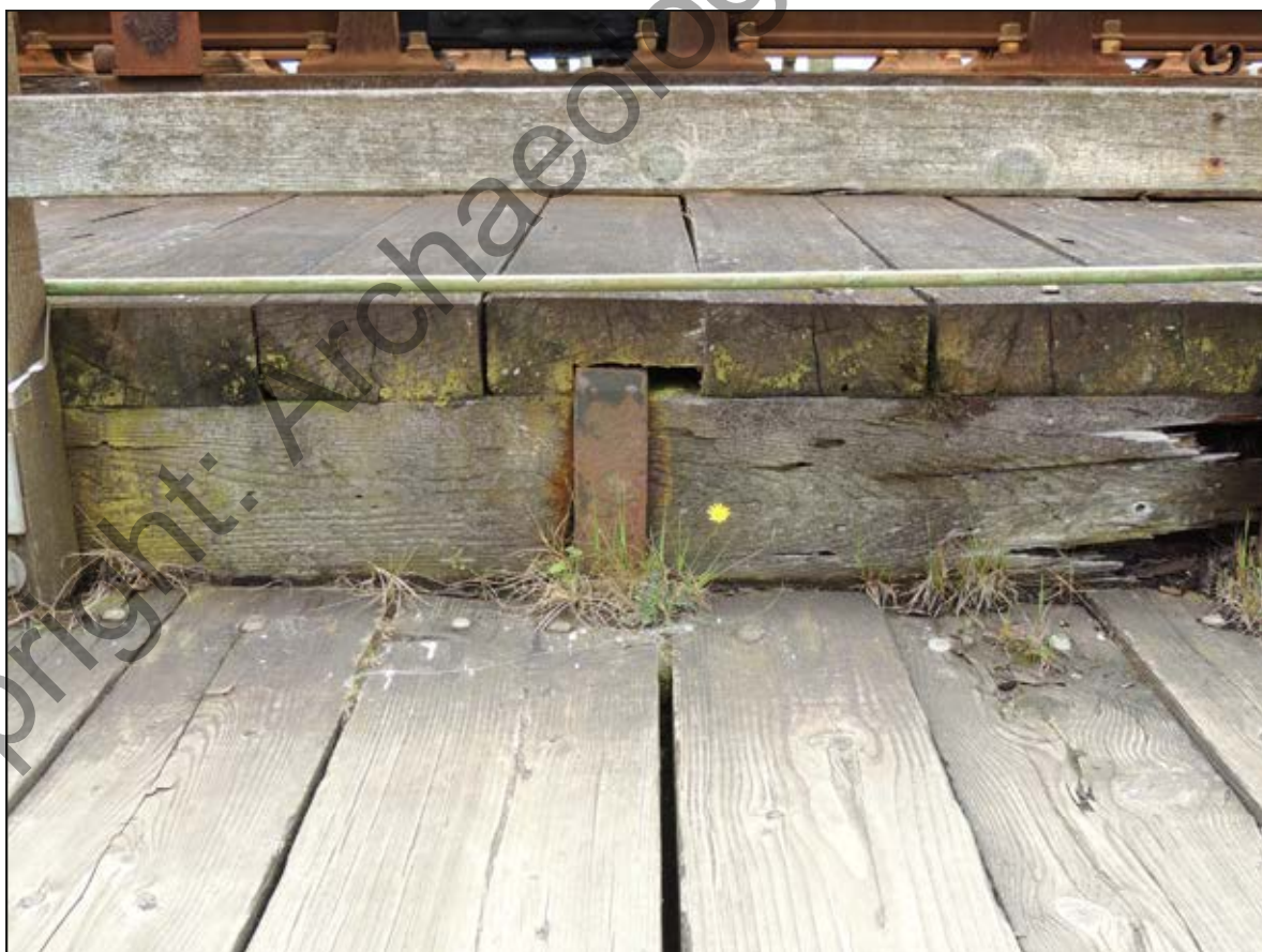
Plate 12. SW facing shot of damaged longitudinal outer beam with metal strap between trestle 5 and 6.
