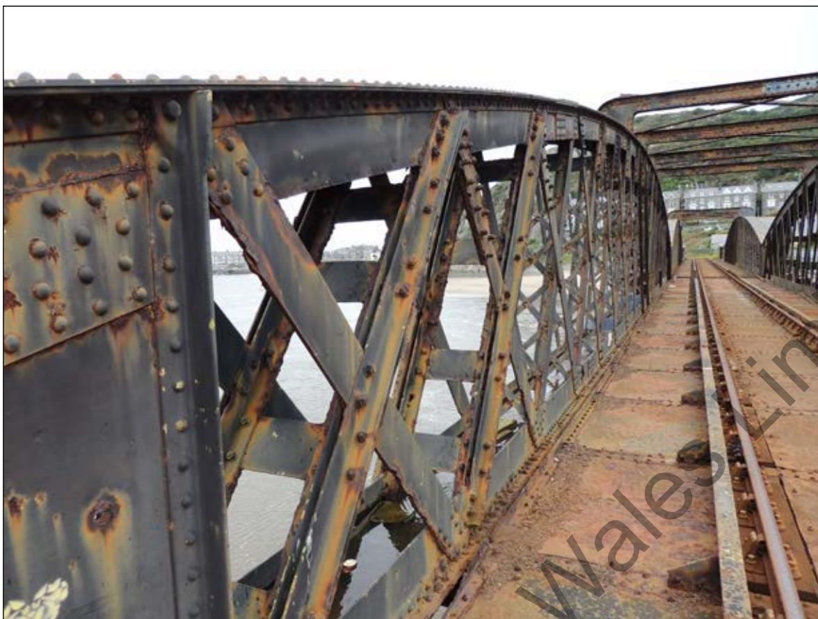
Plate 29. NNW facing shot of hogback lattice trusses on the span of the viaduct.
