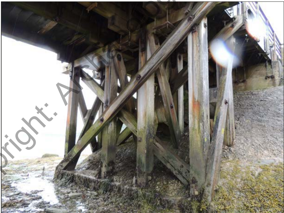
Plate 44. ESE facing shot of trestle 2 showing verticle piles and diagonal beam.
