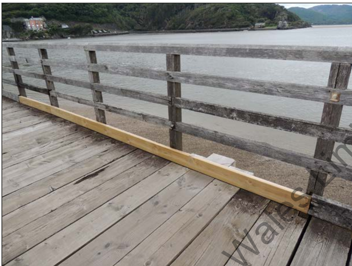
Plate 21. N facing shot of replacement timbers of kickboard on the handrail at trestle 61.
