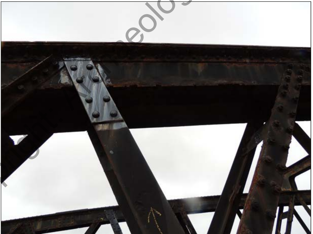
Plate 34. SW facing shot of steel riveted plate added to strengthen the lattice trusses on the NE elevation of the span of the viaduct.
