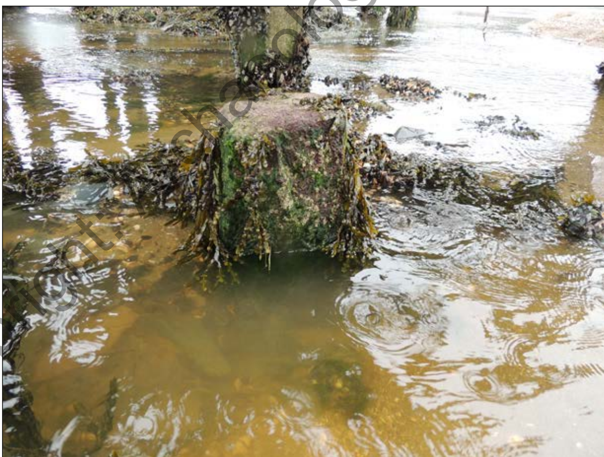
Plate 54. Close up NW facing shot showing remains of central verticle pile stump of trestle 55.
