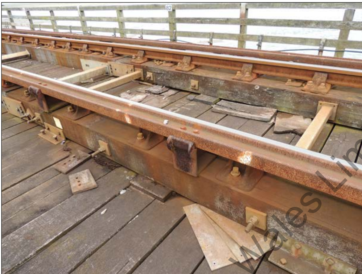
Plate 25. SW facing shot of metal plates and wooden boards supporting transverse deck planks at trestle 82.
