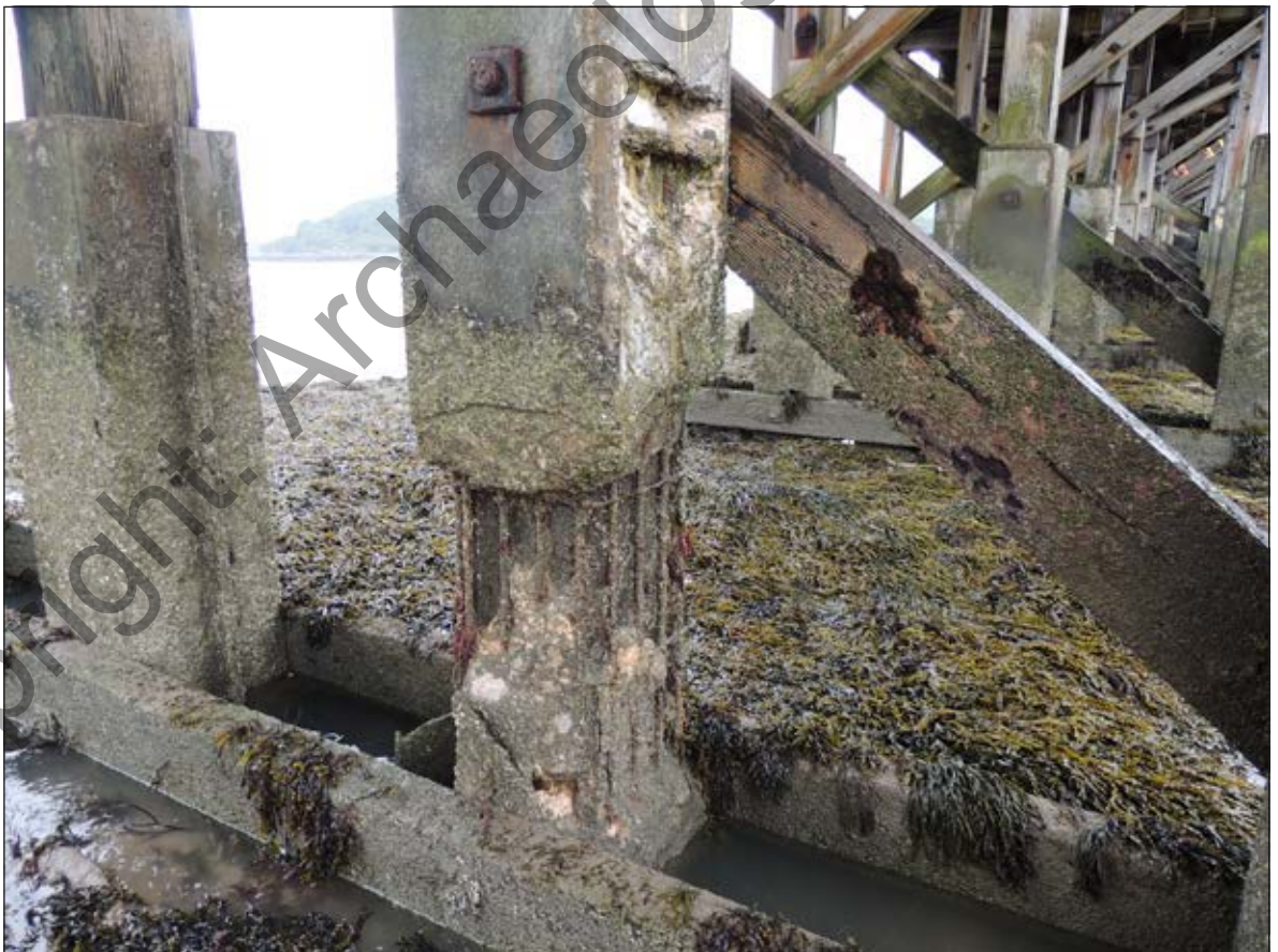
Plate 46. ESE facing shot of damaged reinforced concrete pile casing with exposed rebar of trestle 13.
