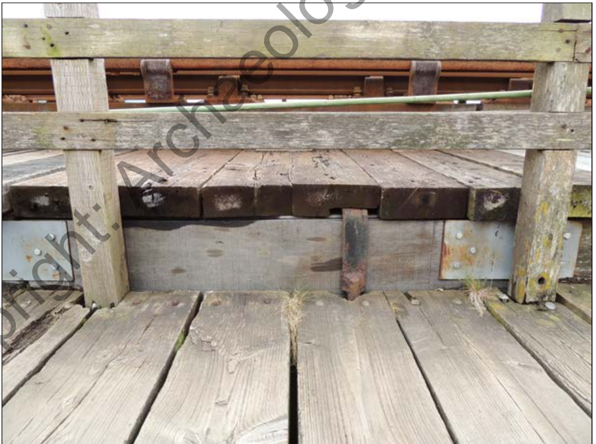
Plate 14. SW facing shot of replacement longitudinal outer beam and metal strap with metal plate reinforcements inbetween trestle 12 and 13.
