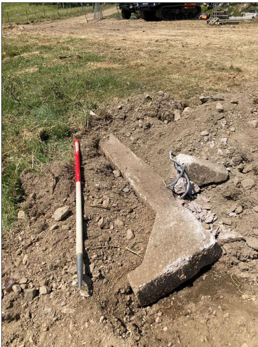
Plate 71. Reinforced prefabricated concrete pillar. Roadway between D and E.
