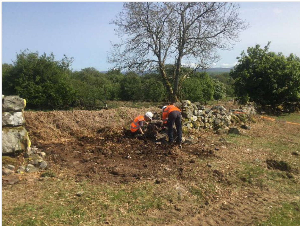
Plate 39. Deconstruction of wall [600] being carried out by hand.
