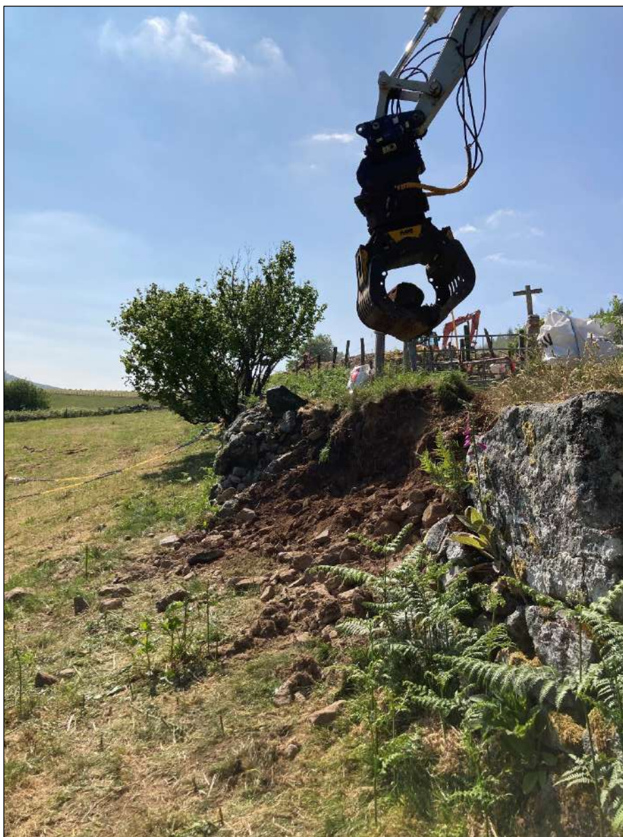
Plate 43. Deconstruction of wall [700] with the hydraulic grab.
