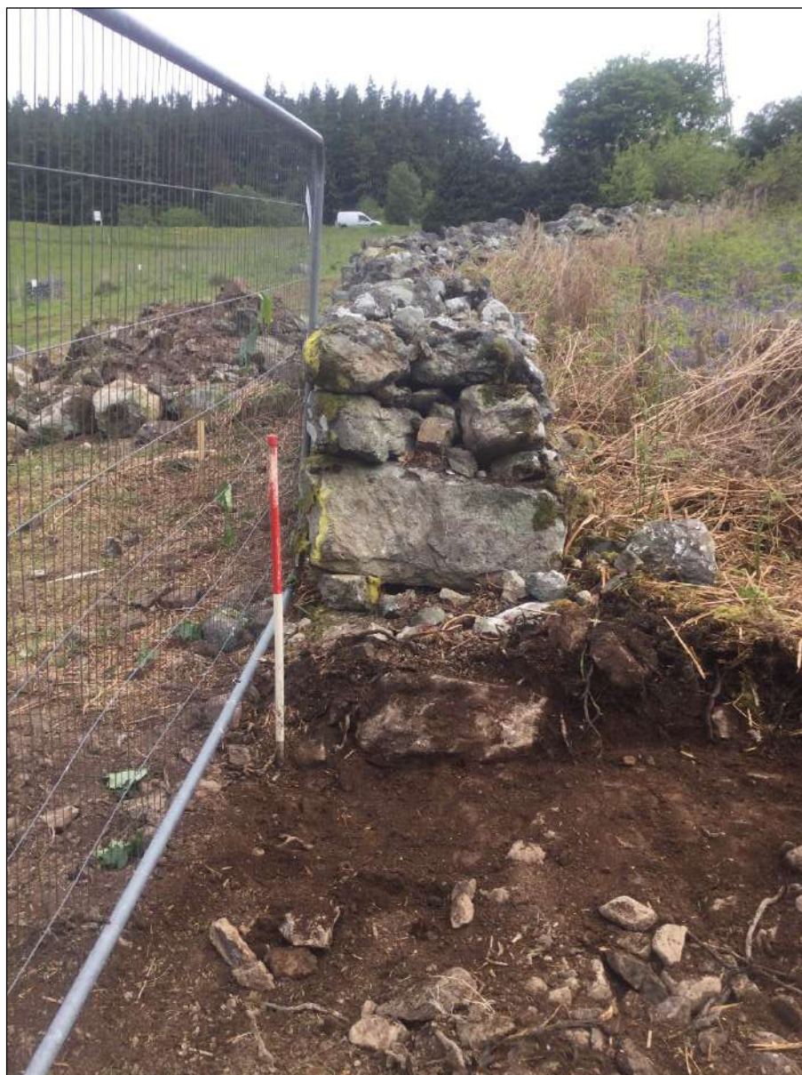
Plate 40. South-facing section of wall [600] showing traditional dry stone build.
