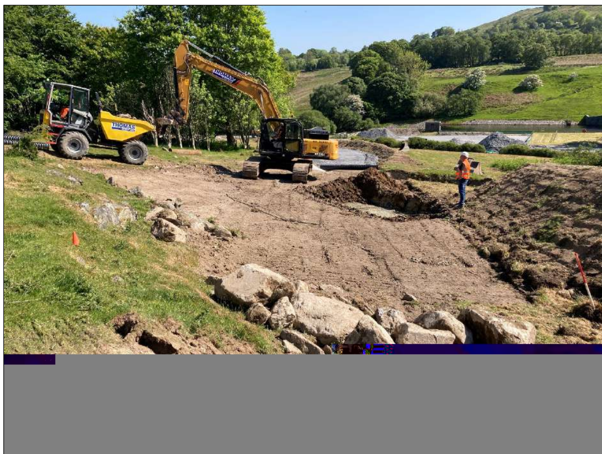
Plate 11. Roadway between B and C under construction.
