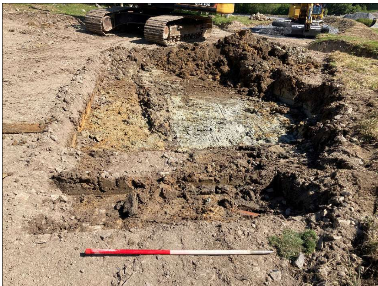
Plate 12. Sondage dug within roadway to judge ground conditions.
