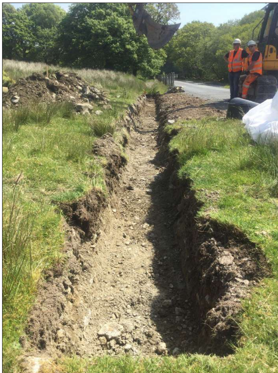
Plate 8. Silt trap at base of Area B, looking east.
