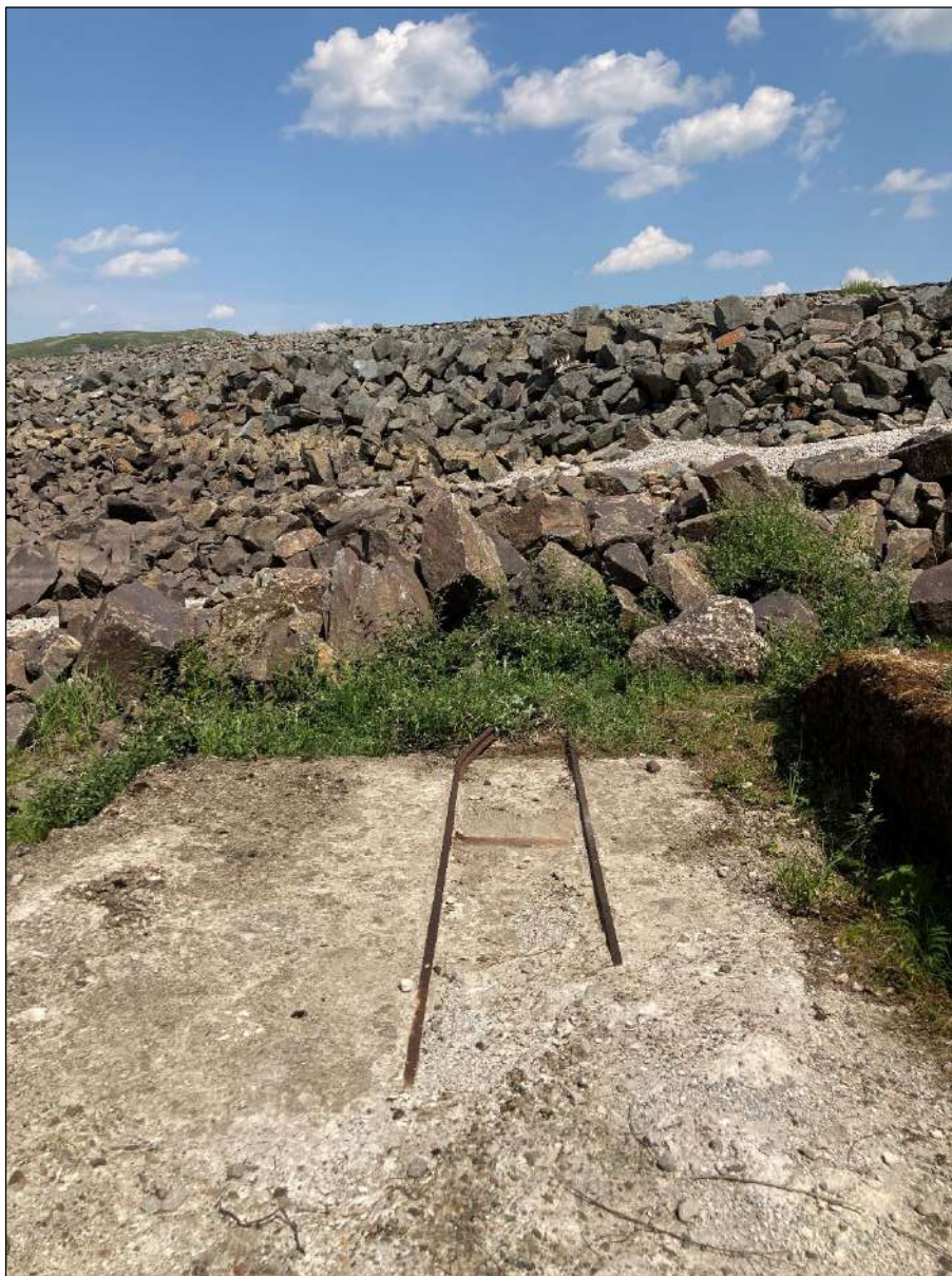
Plate 65. Remains of boggy track used to transport material during construction of the reservoir, exposed during the work.
