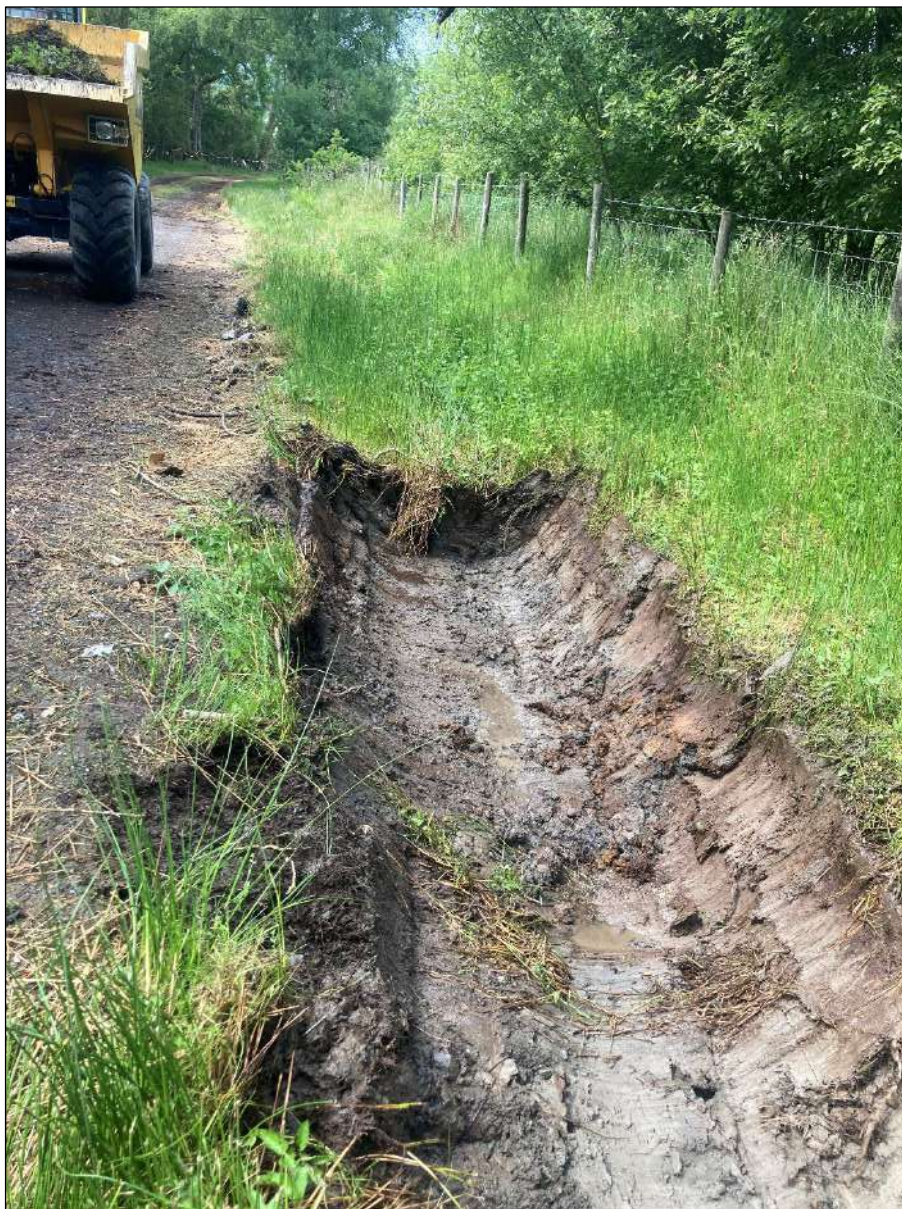
Plate 34. Excavation of the road gullies along the haulage road.
