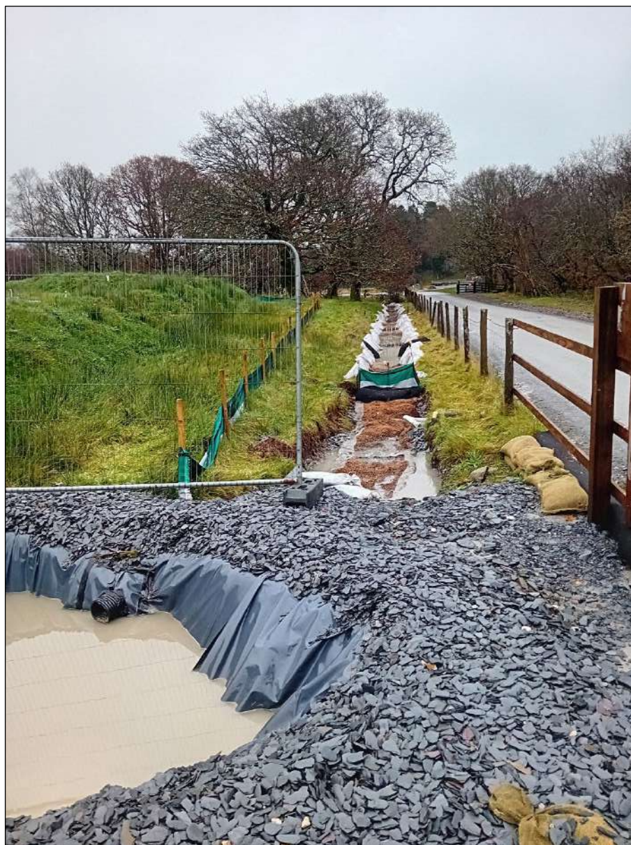
Plate 10. The silt trap at sign off.
