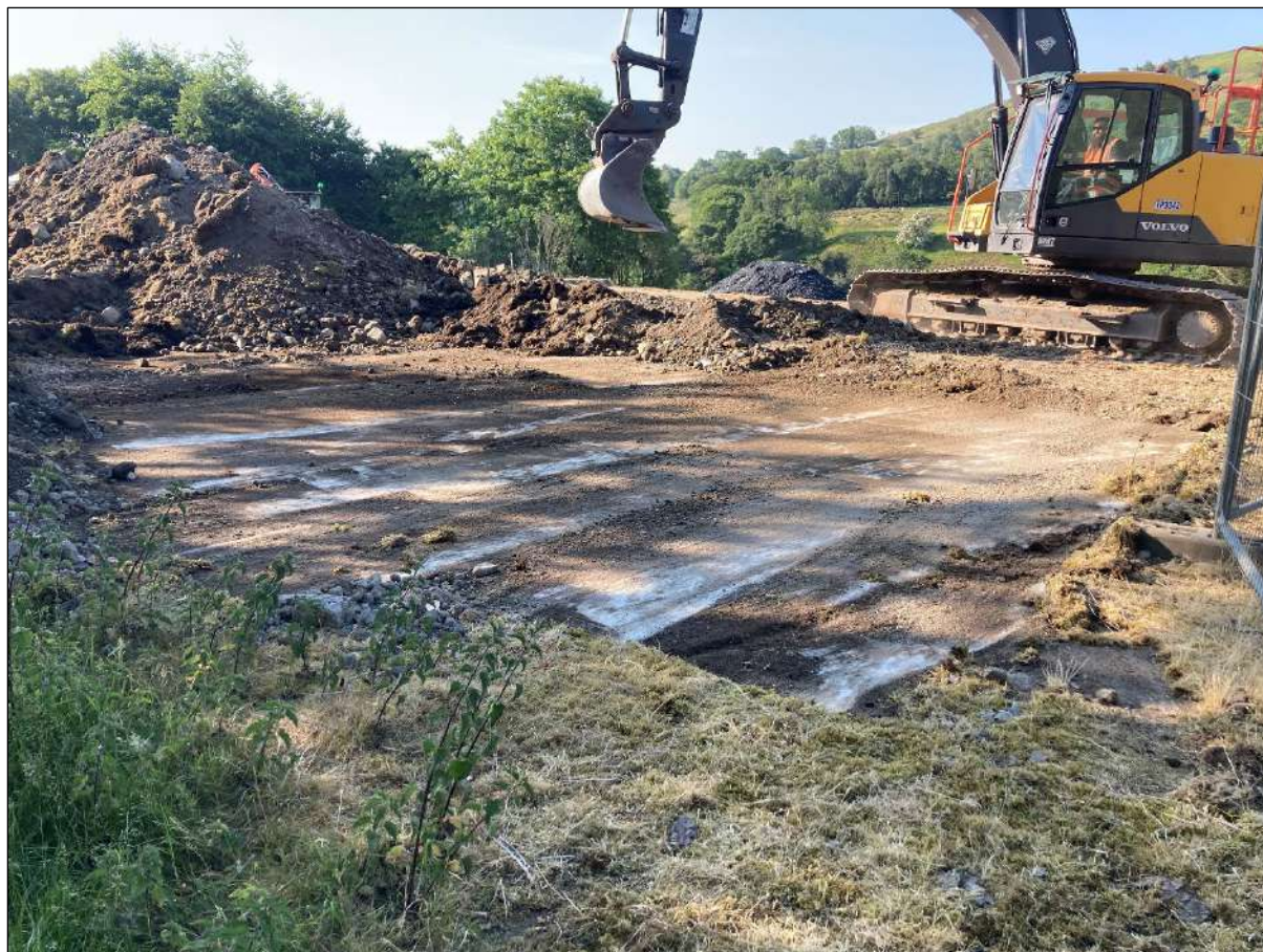
Plate 17. Exposure of concrete apron [302] in Area C.
