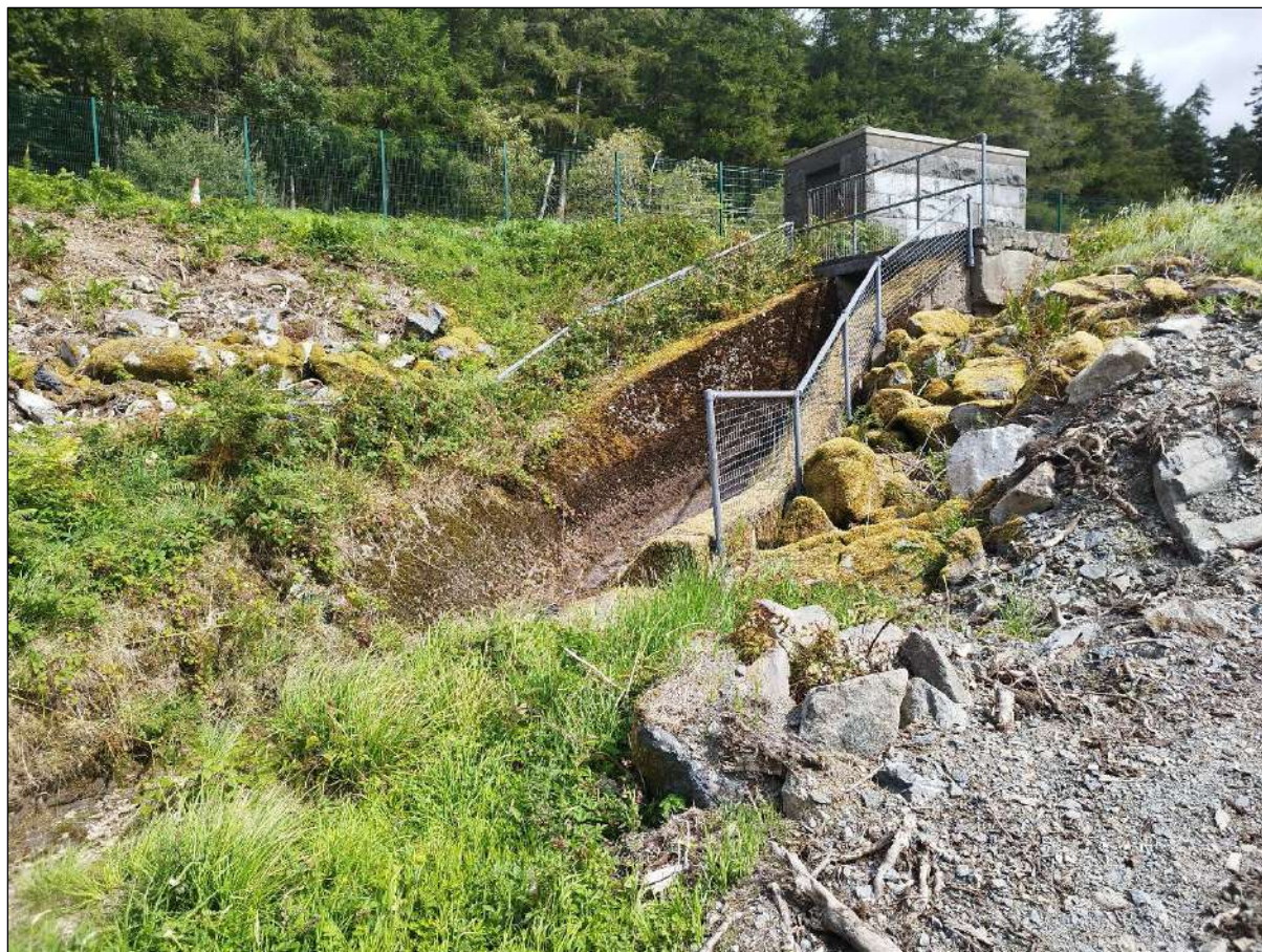
Plate 62. The original spillway for the reservoir, after clearance.
